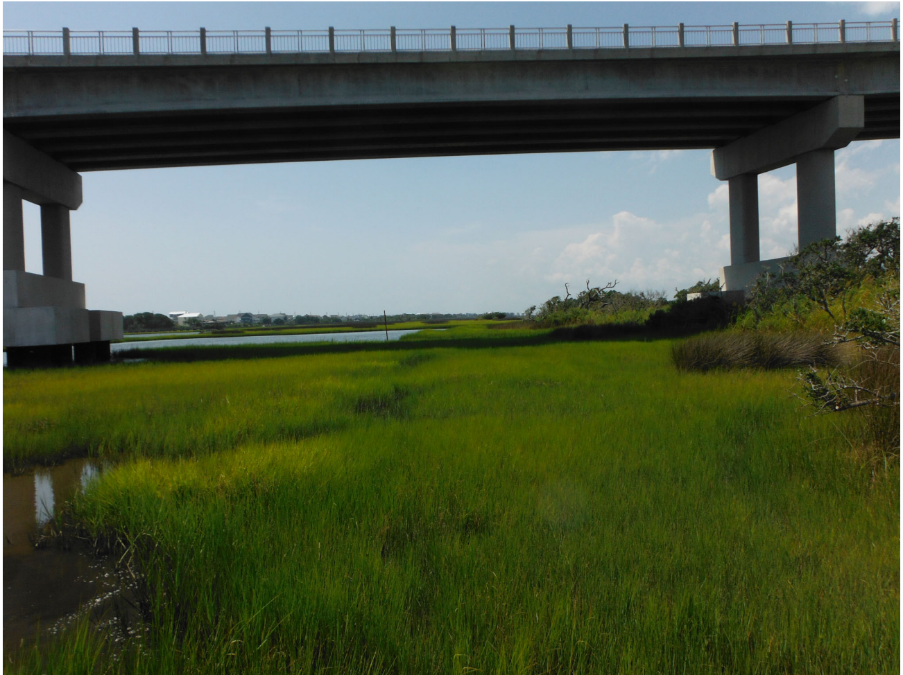
PP# 7 (Geotech area adjacent to Surf City Park)
