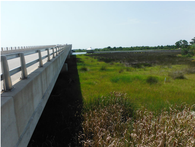
PP# 1 Site 4 (temporary work bridge)
