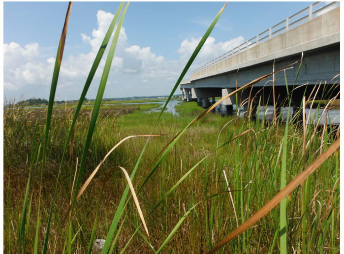
PP#2 Site 4 (temporary work bridge)
