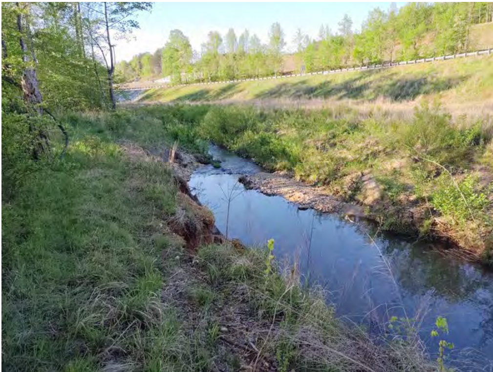
Looking South Downstream through End of Destabilized Streambank
