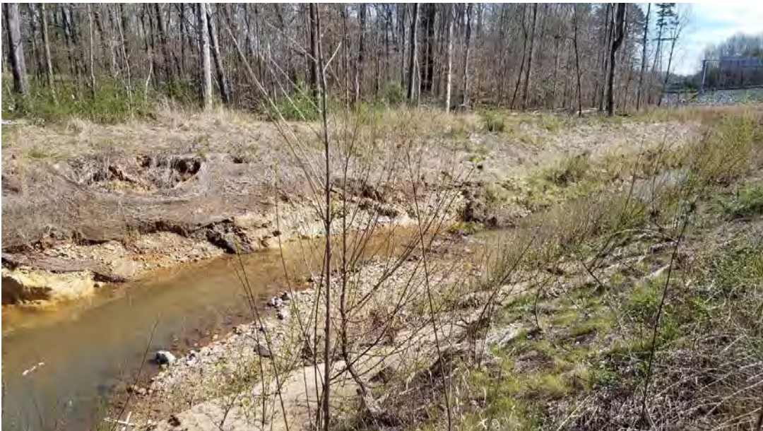
Looking East at Streambank Destabilization below Cross Vane 1 – 3/26/20
