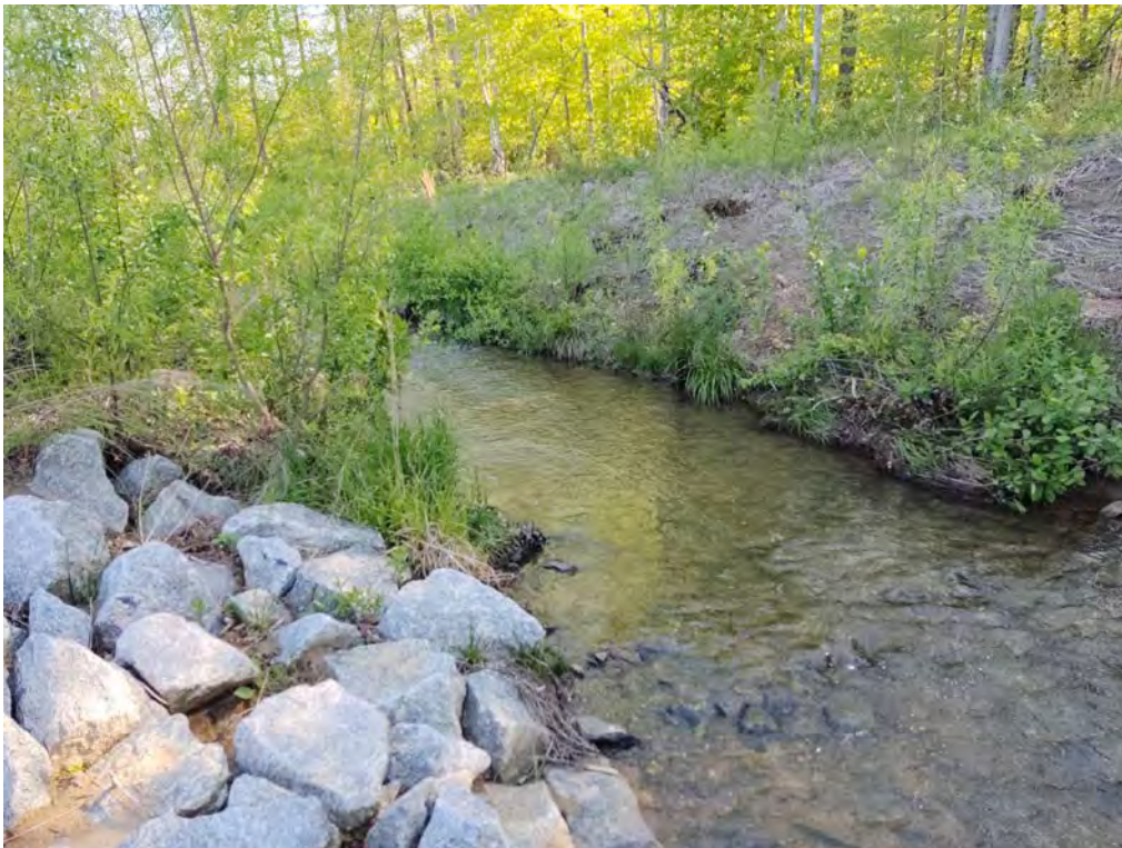
Looking North (Upstream) from End of Channel Relocation Rip Rap on Left is “Plug” of Old Stream Channel
