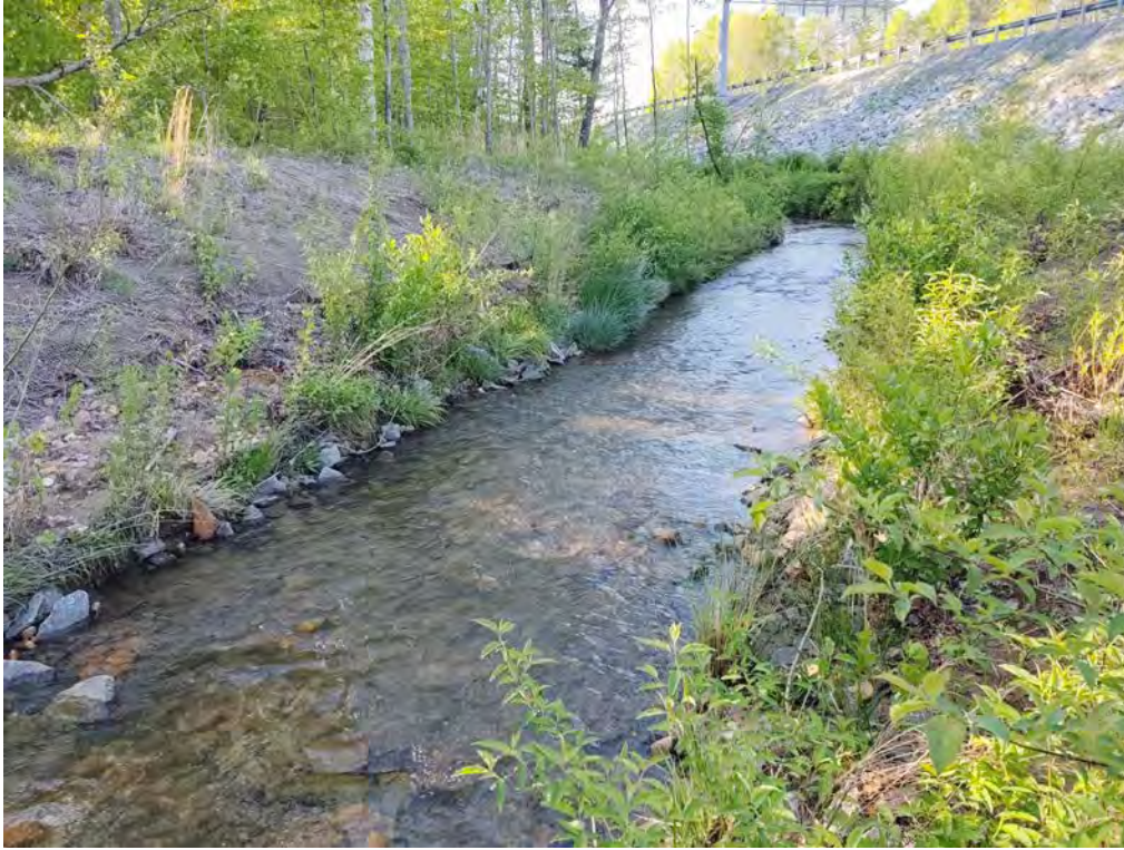
Continue Looking South – Downstream to End of Relocation
