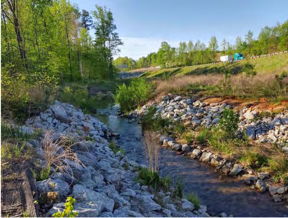
Looking Downstream from Culvert Outlet
