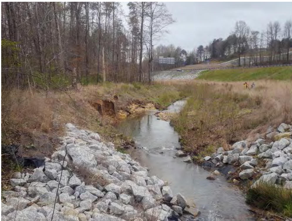
Looking South at Streambank Destabilization below Cross Vane 1 – 3/26/20
