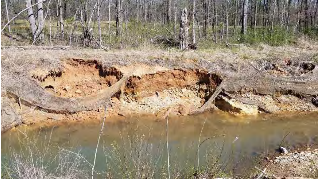
Looking East at Streambank Destabilization below Cross Vane 1 – 3/26/20
