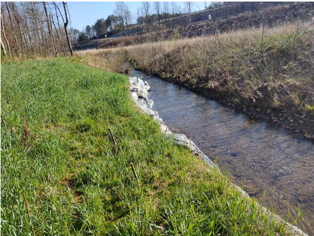
Looking Downstream After Repairs – 4-2-2021
