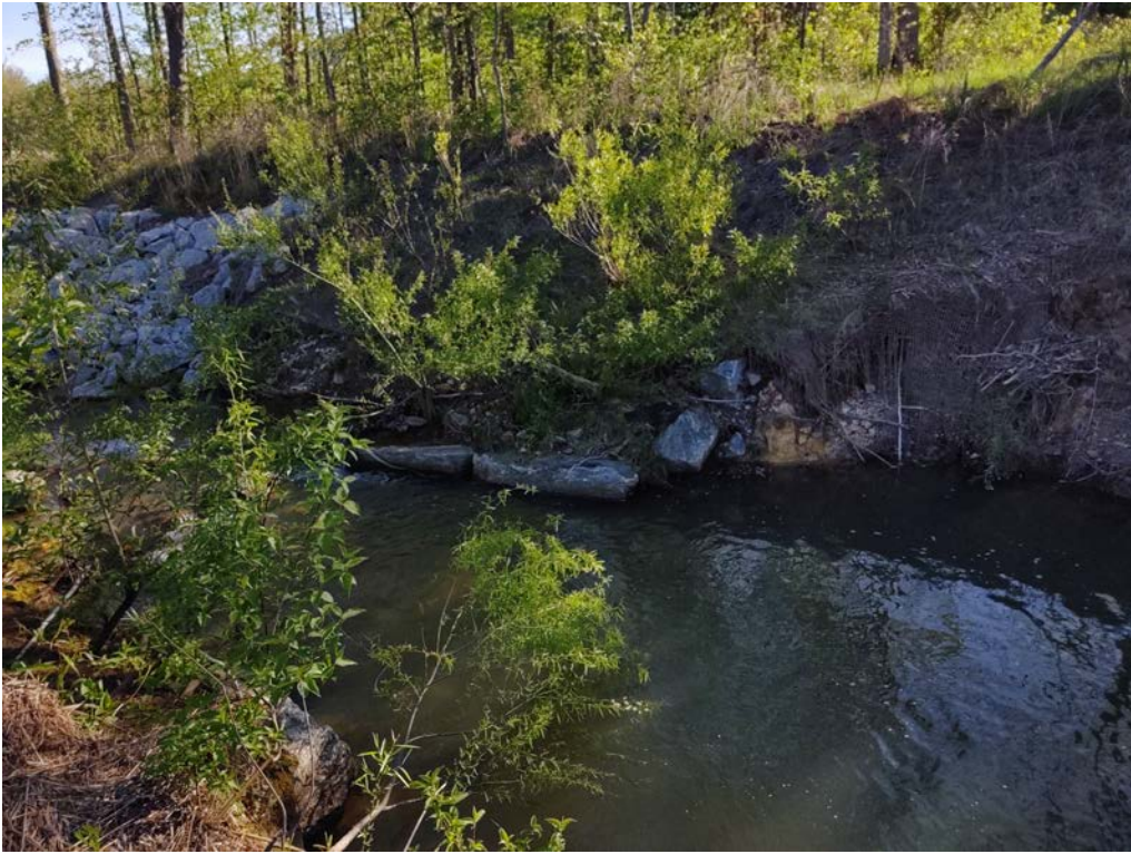
Looking East at Upper End of Streambank Destabilization April 2020
