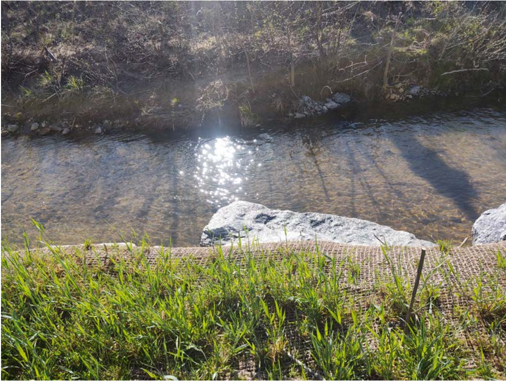
Looking Across Stream from Point 1A After Repairs – 4-2-2021
