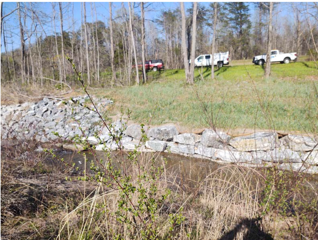
Looking East at Upper End of Streambank Repairs April 2021
