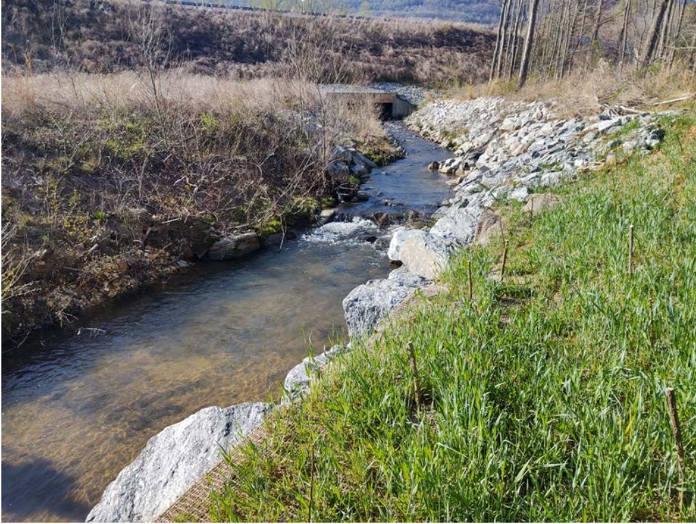
Looking Upstream After Repairs – 4-2-2021
