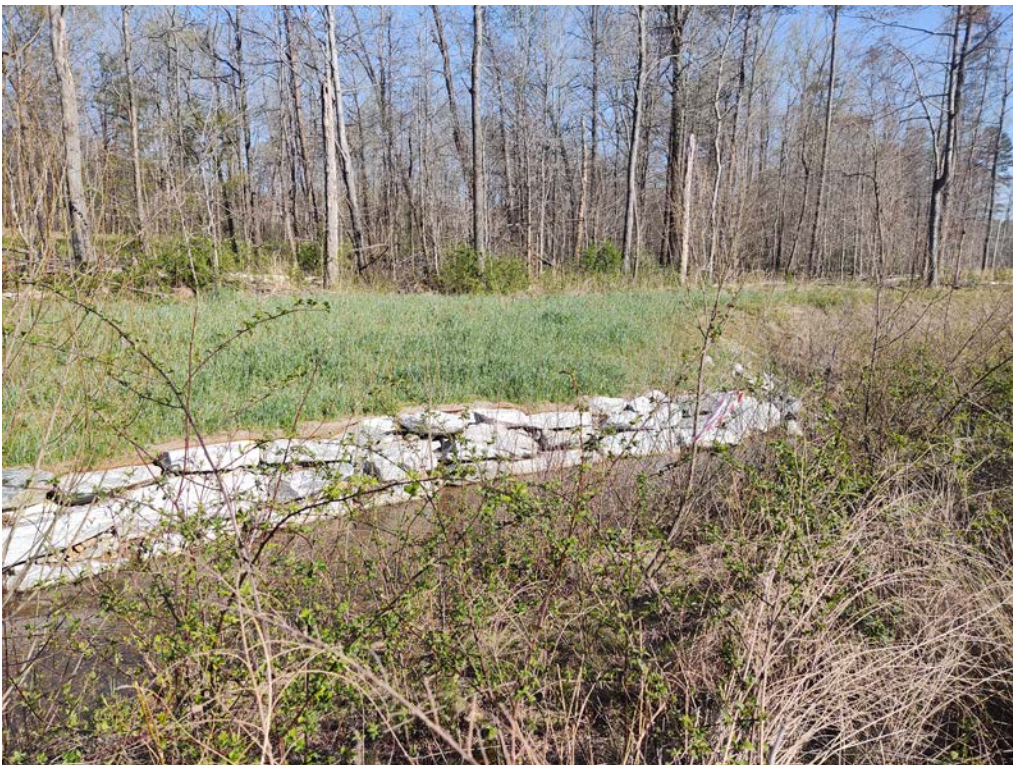
Looking East at Lower End of Streambank Repairs April 2021
