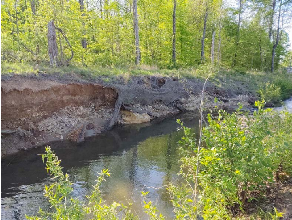
Looking East at Lower End of Streambank Destabilization April 2020
