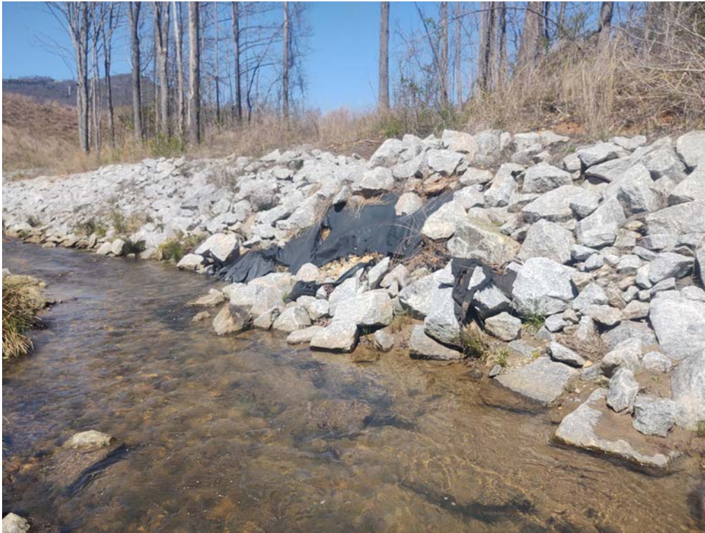
Minor Streambank Scour North of New Boulder Wall
