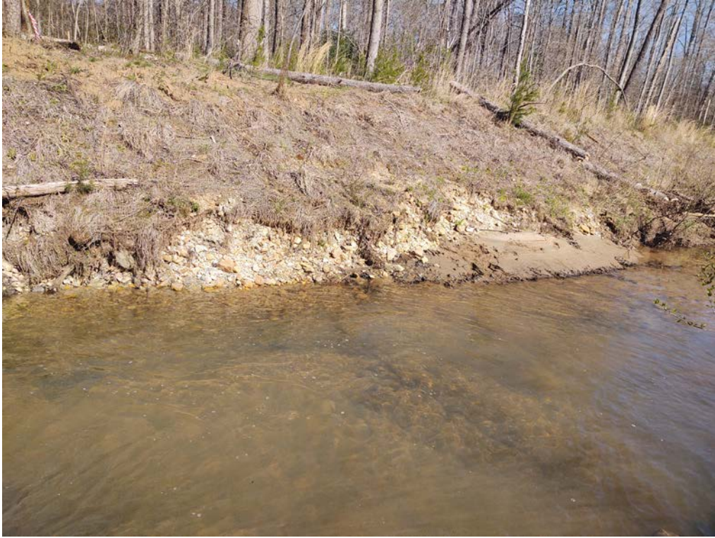
Minor Toe Scour on East Bank Below New Boulder Wall
