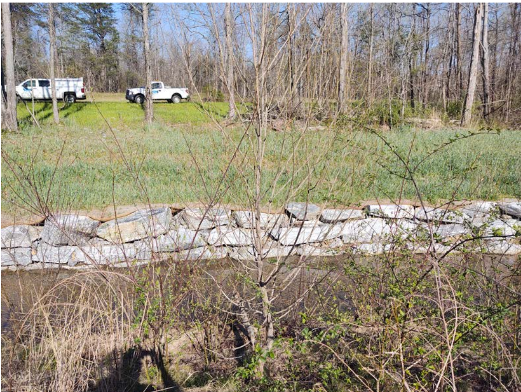
Looking East at Middle of Streambank Repairs April 2021
