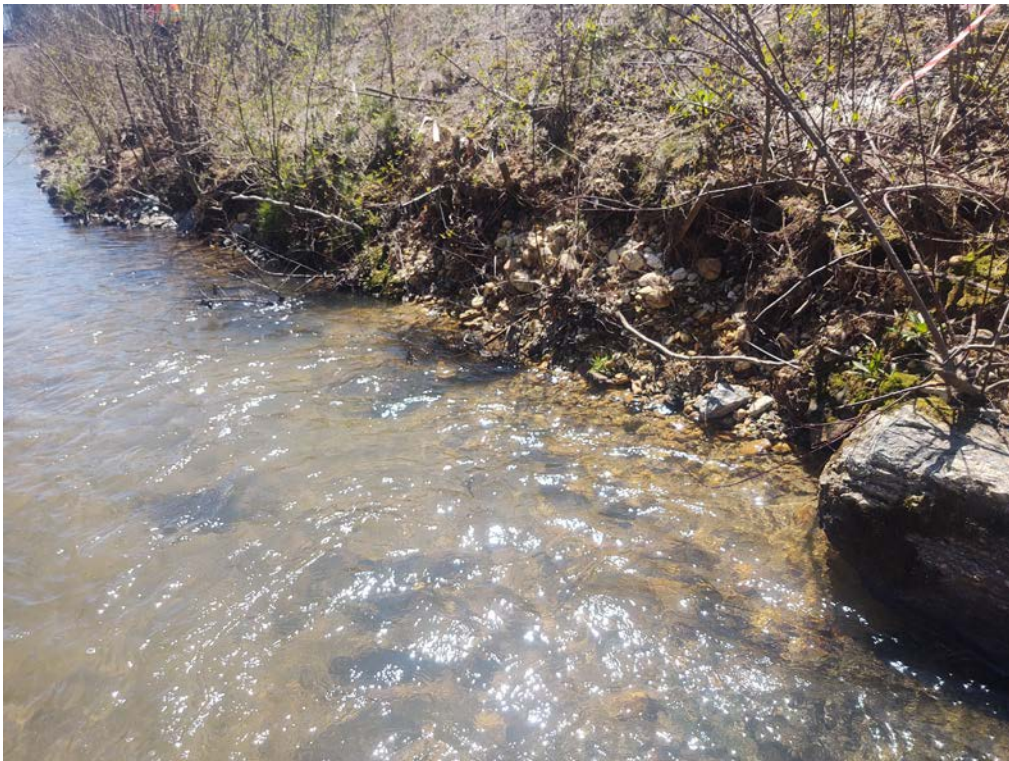
Minor Toe Scour on West Bank of Cross Vane 1
