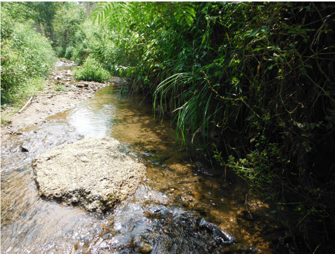
Undercut left bank
