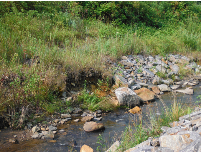
Minor bank scouring along left bank
