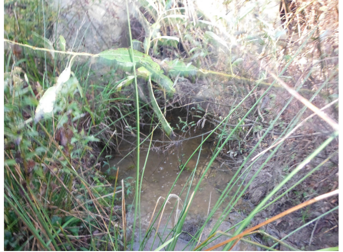
Upper stream looking downstream at pipe inlet
