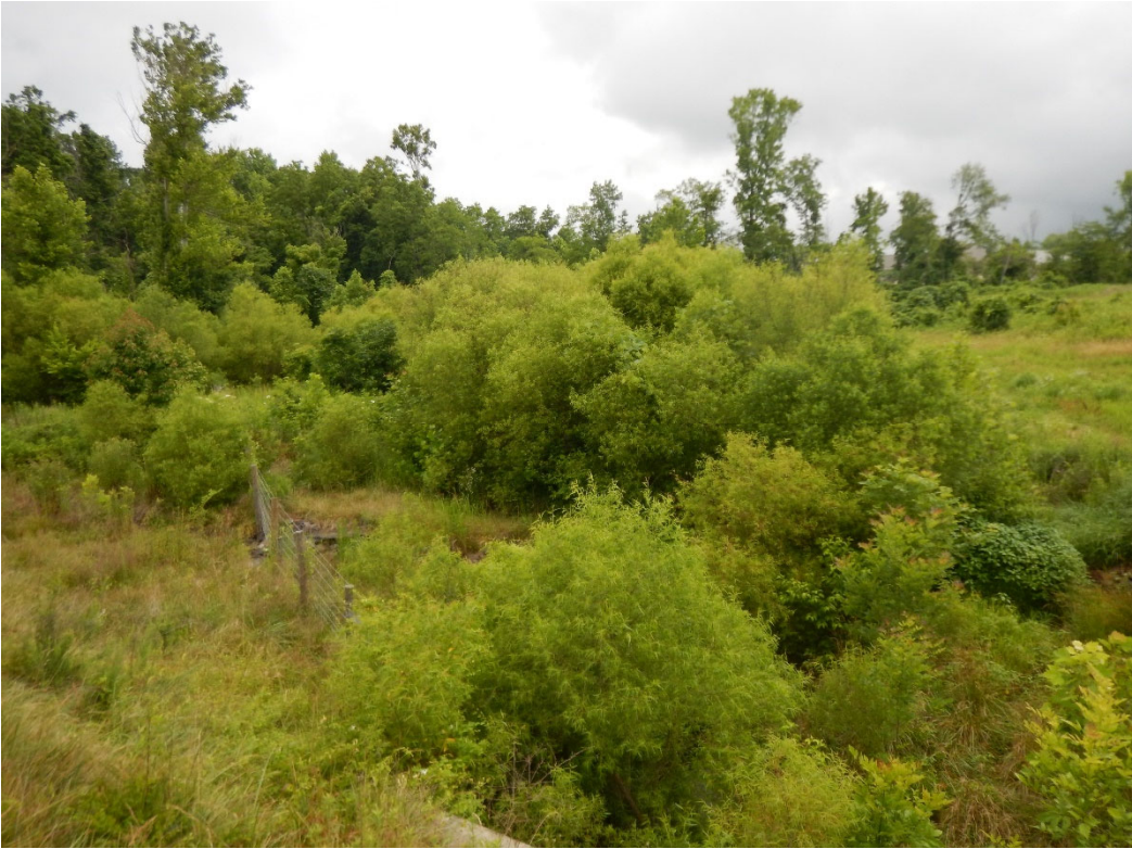
Overview looking upstream from culvert inlet at I-840.
