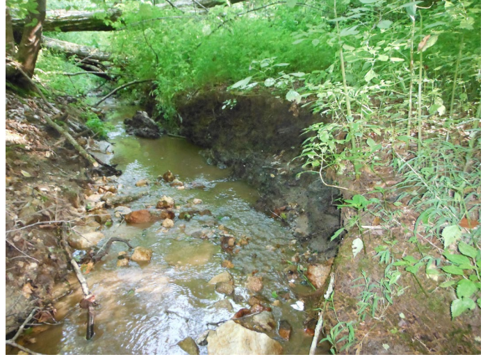
Bank erosion upstream of PP#1
