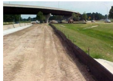
Perimeter Silt Fence
