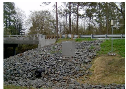
Rock Stabilization
