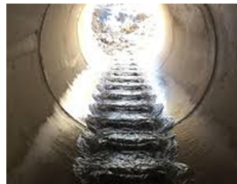
Culvert with Flexi baffles installed
