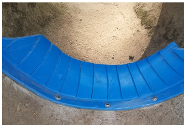
Typical Flexi baffle installed in a culvert
