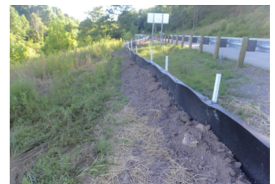
Wildlife barrier fencing (courtesy of ODOT)
