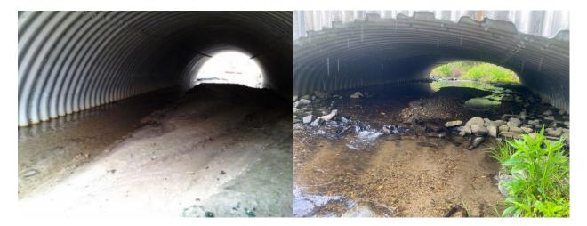
Figures 2 and 3. Wide corrugated metal pipe (Wayne County, SR 1300, Unnamed Tributary) retaining bedload (left) and aluminum box culvert (Transylvania County, #870163, North Prong Glade Creek) with notched sills and baffles buried by bedload (right, note partially exposed sill in photo right).
