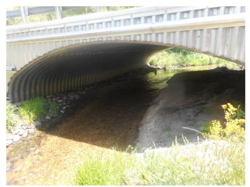
Figure 14. Native material backfilled over rip rap in aluminum box culvert (Henderson County, #440073, Greer Creek).
