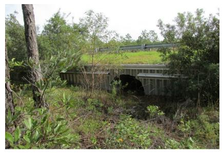
Figure 17. Culvert designed for small and medium animal passage on EF Middleton Blvd. Brunswick County.
