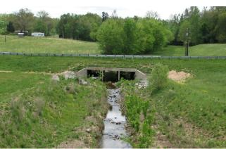
Figures 4 and 5. Benching into box culvert (left, Transylvania County, #870012, Hogsed Creek) and benching with bank sloping (right, Mecklenburg, I-485 vicinity, unnamed tributary).
