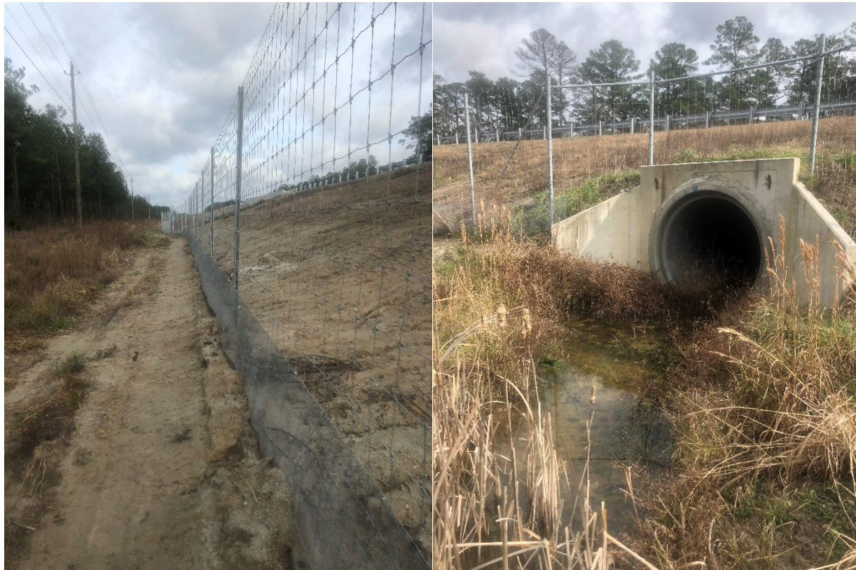
Figures 23 and 24. Woven-wire wildlife fence run (left) and tie into crossing structure (right). US 17 Jones County
