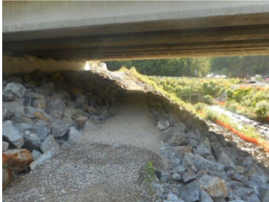
Figure 10. Wildlife pathway or "bench" as built from Figure 9.
