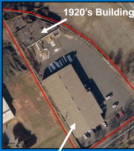
1990 Building - Plumbing Supply
