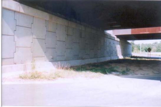
I-540 & Triangle Town Center Constructed 2004 CR \approx 5 \mu\text{m}/\text{yr}
