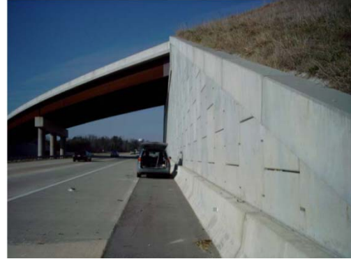
US 1 West - Wake Forest Constructed 2005 CR \approx .25 \mu\text{m}/\text{yr}
