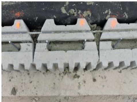
Grout with Vertical & Horizontal Rebar
