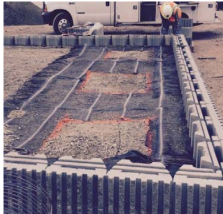
Precut Geogrid Around Shaft Location
