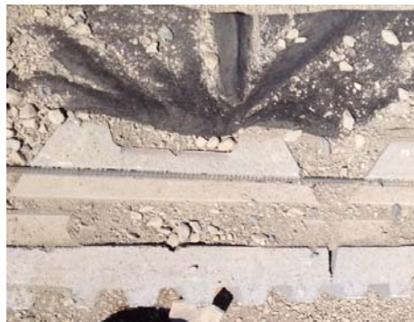
Core Fill and Horizontal Rebar
