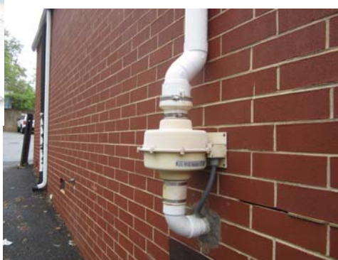
View of vapor mitigation system in on-site building.
