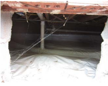
View of vapor mitigation system in on-site building.
