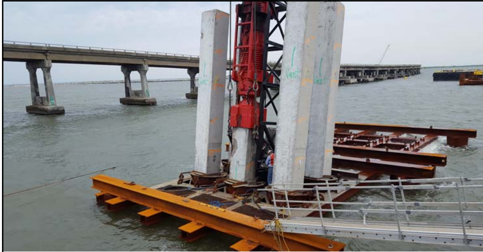
DRIVING 36" SQUARE PILE
