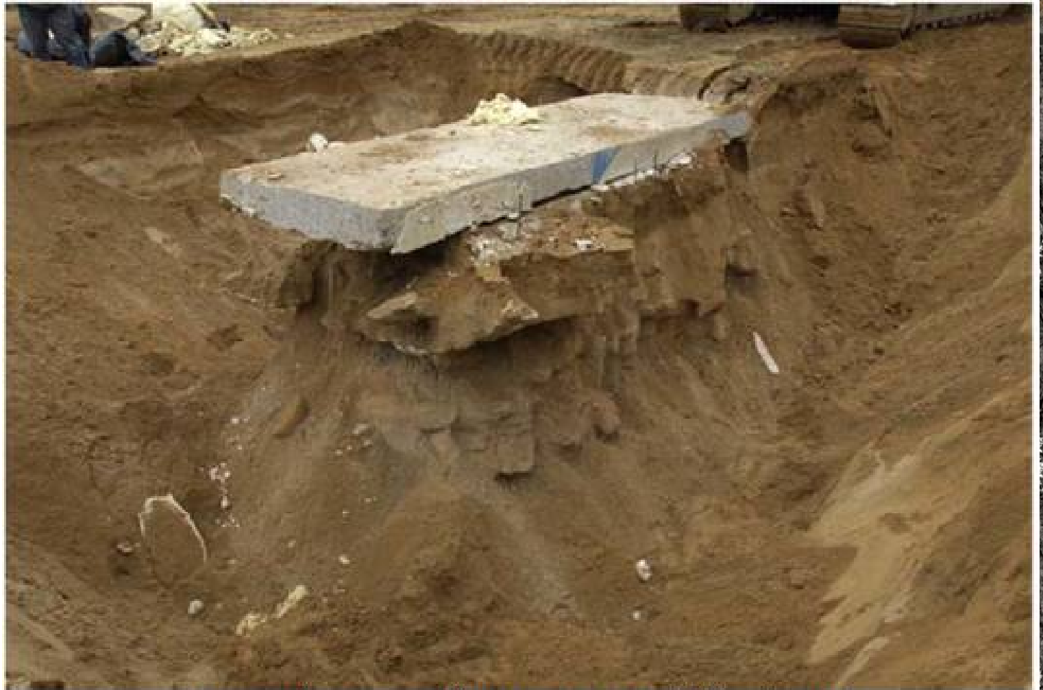
Excavation Revealing ISSBIP-Stabilized Sand
