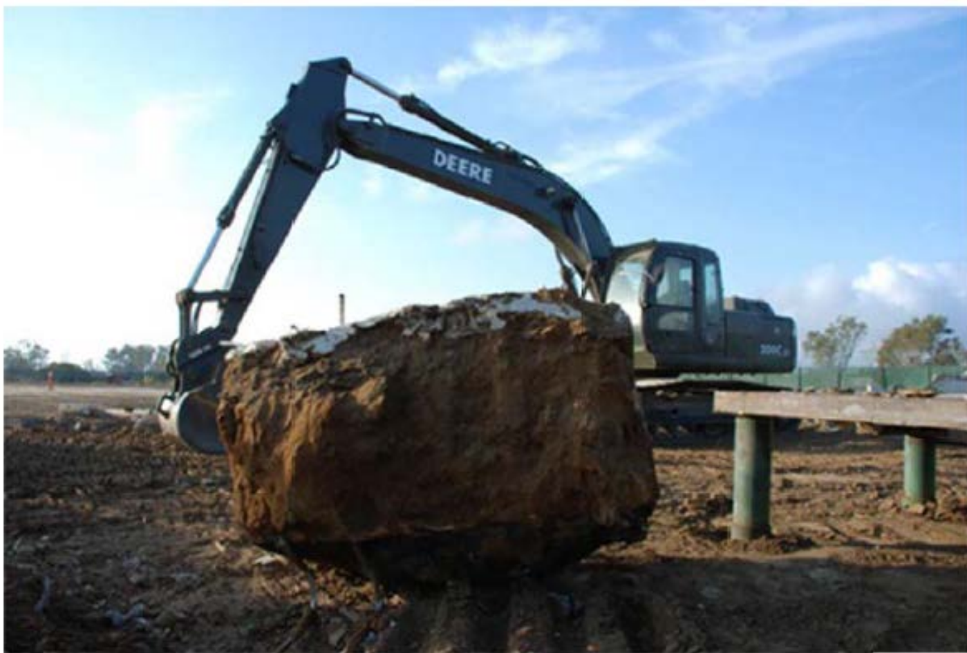
Intact Extraction of the Stabilized Crater Repair
