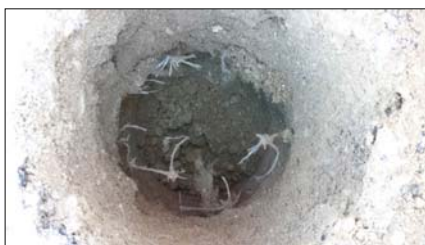
Drilled hole through geogrid reinforcement.
