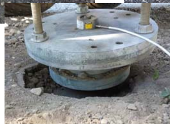
8 in. plate on gravel (after punching shear failure)
