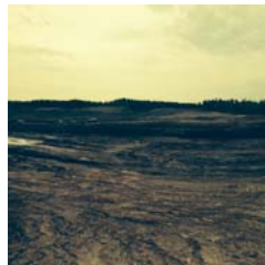
View of Phase 1 looking North
