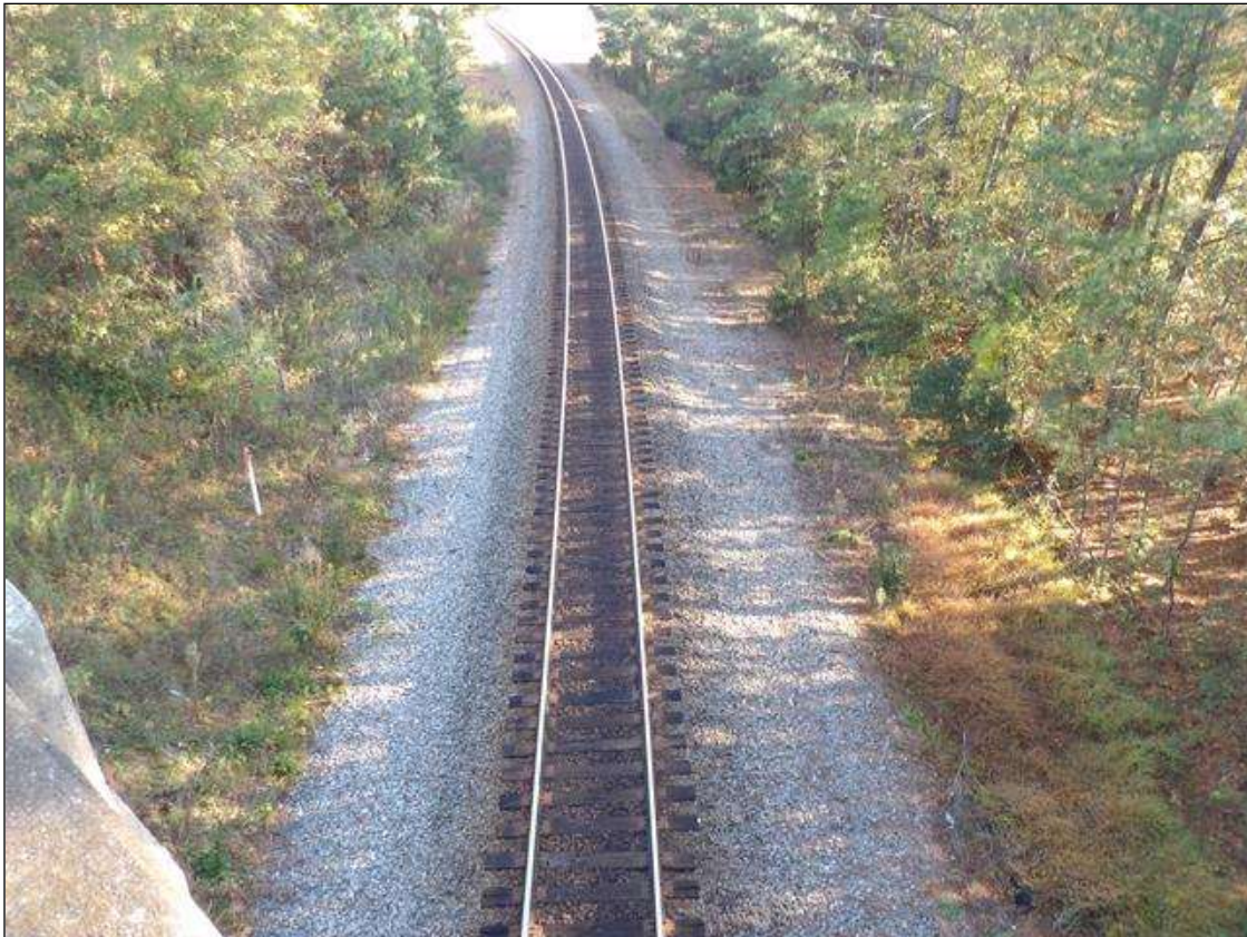
LOOKING EAST OVER SPAN 3
