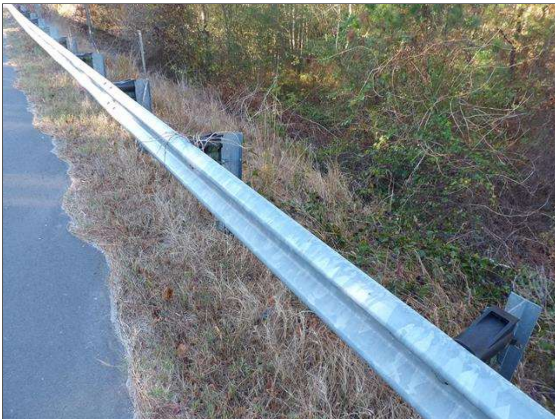
GUARDRAIL POST SPACING MIDWAY NORTHWEST SHOWN ALL OTHERS SIMILAR
