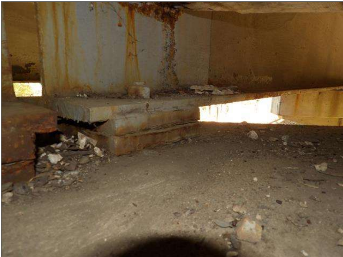
TYPICAL BEARING BEAM 2 AT PIER 1 SPAN 2 SHOWN
