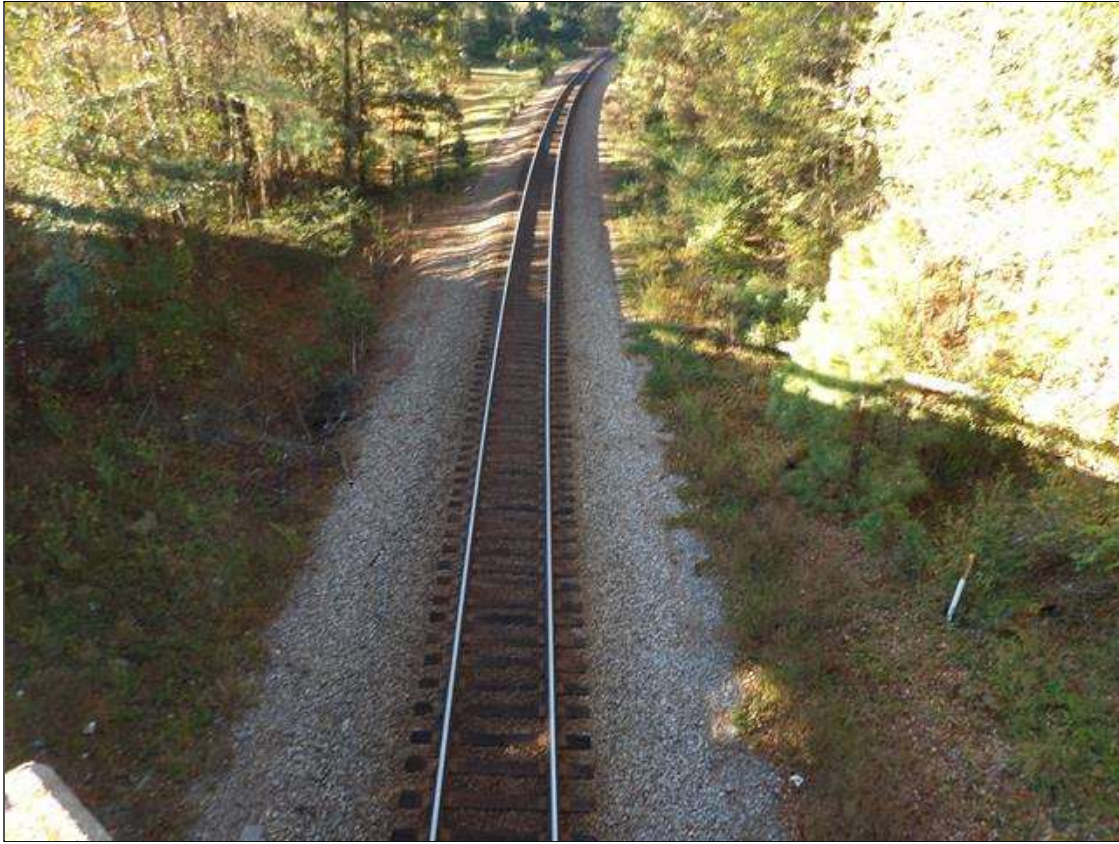
LOOKING WEST OVER SPAN 3
