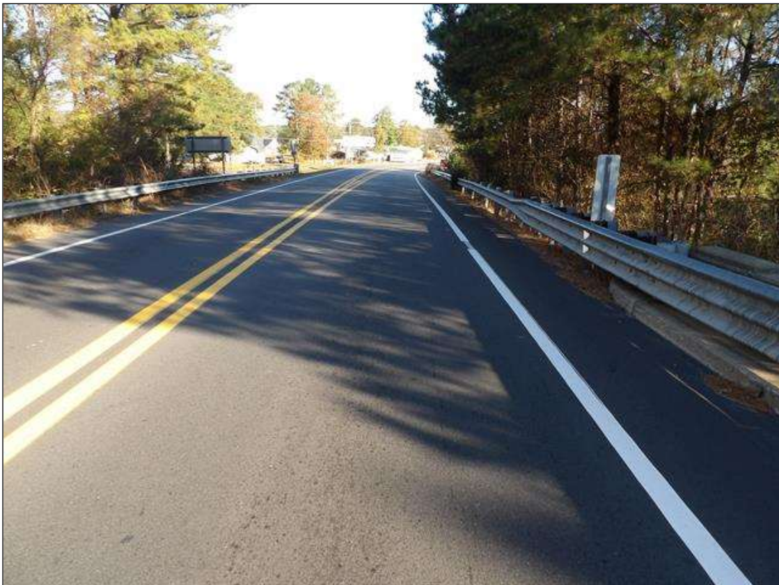
NORTH APPROACH LOOKING NORTH
