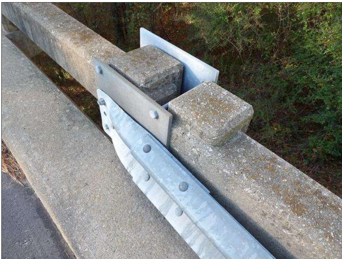
GUARDRAIL ATTACHMENT TO BRIDGE NORTHWEST SHOWN ALL OTHERS SIMILAR
