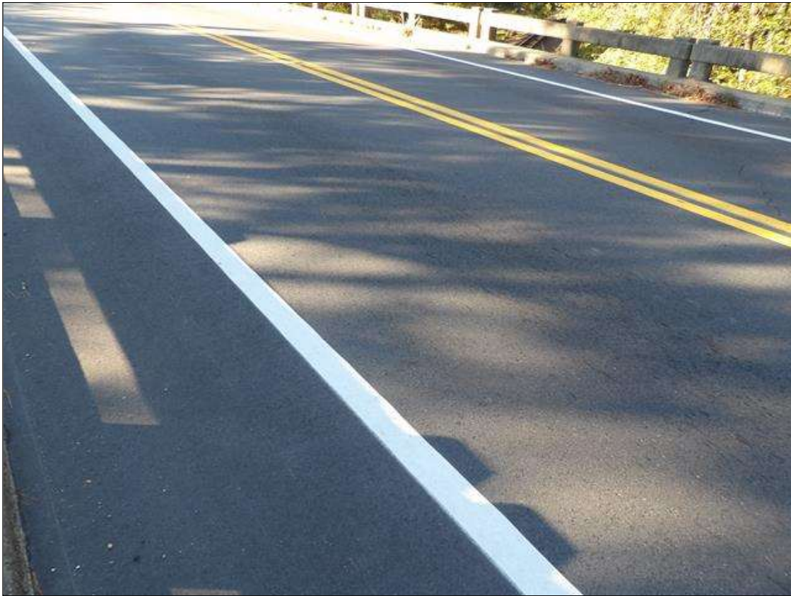
NEW ASPHALT WEARING SURFACE
