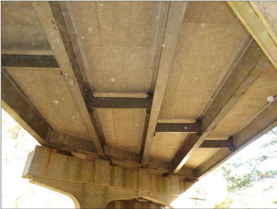
SUPERSTRUCTURE UNDERSIDE SPAN 2 SHOWN ALL OTHERS SIMILAR
