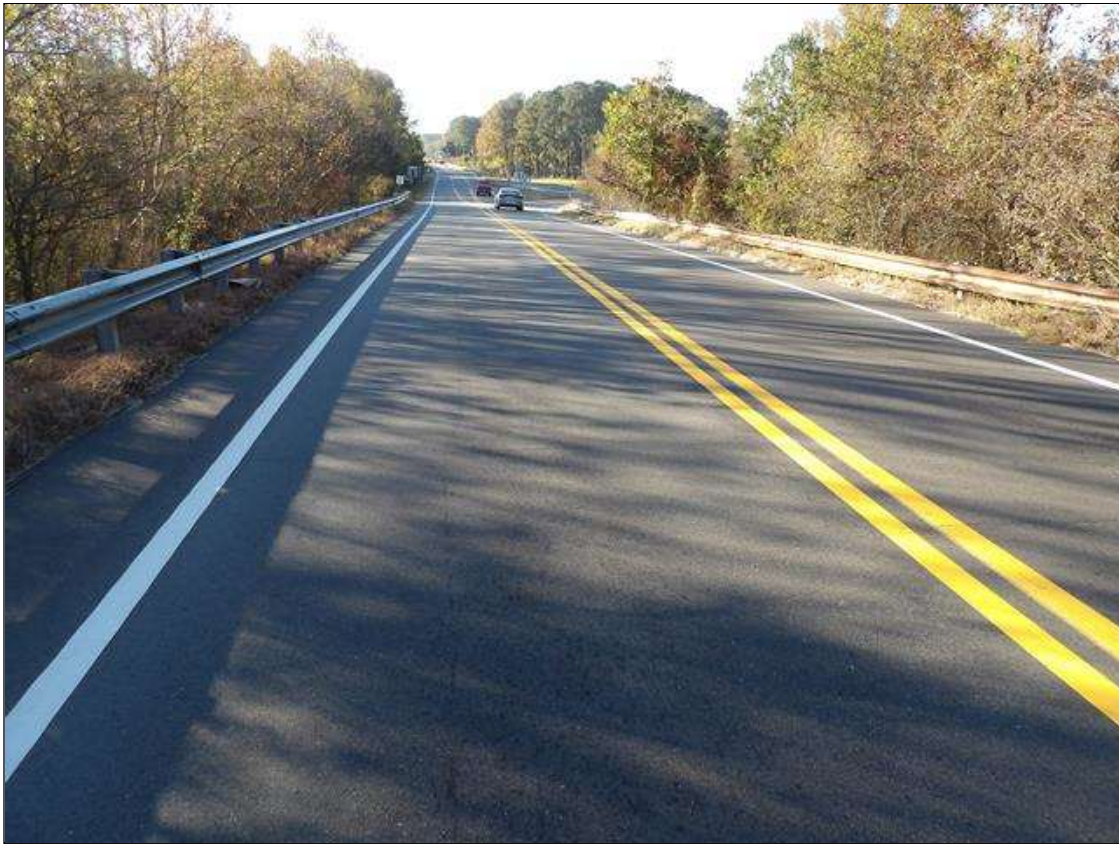
SOUTH APPROACH LOOKING SOUTH
