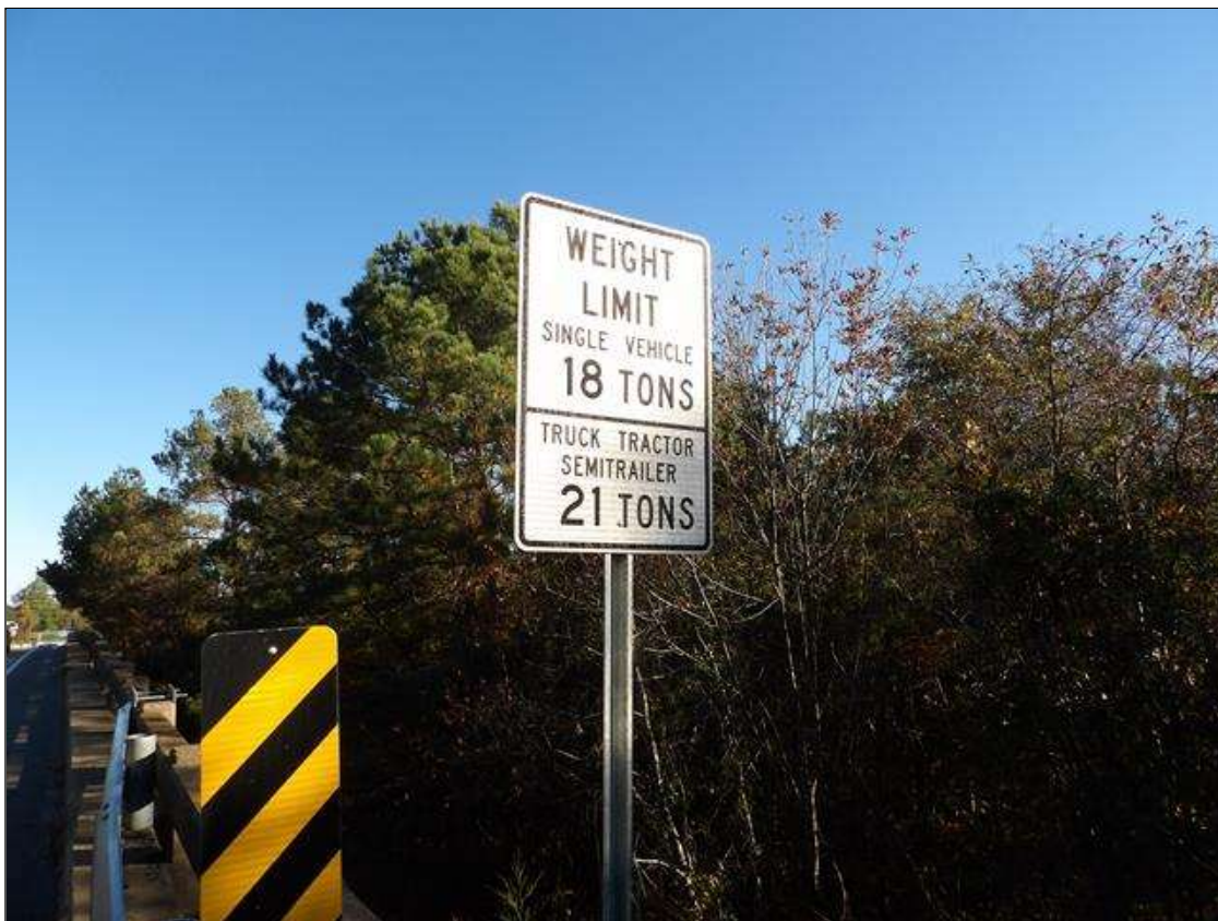
POSTING SIGN AT SOUTH APPROACH
