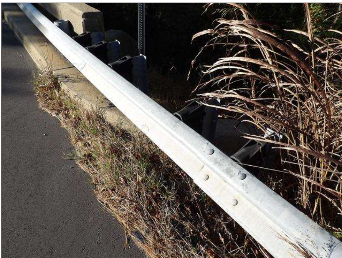
GUARDRAIL POST SPACING AT BRIDGE NORTHWEST SHOWN ALL OTHERS SIMILAR
