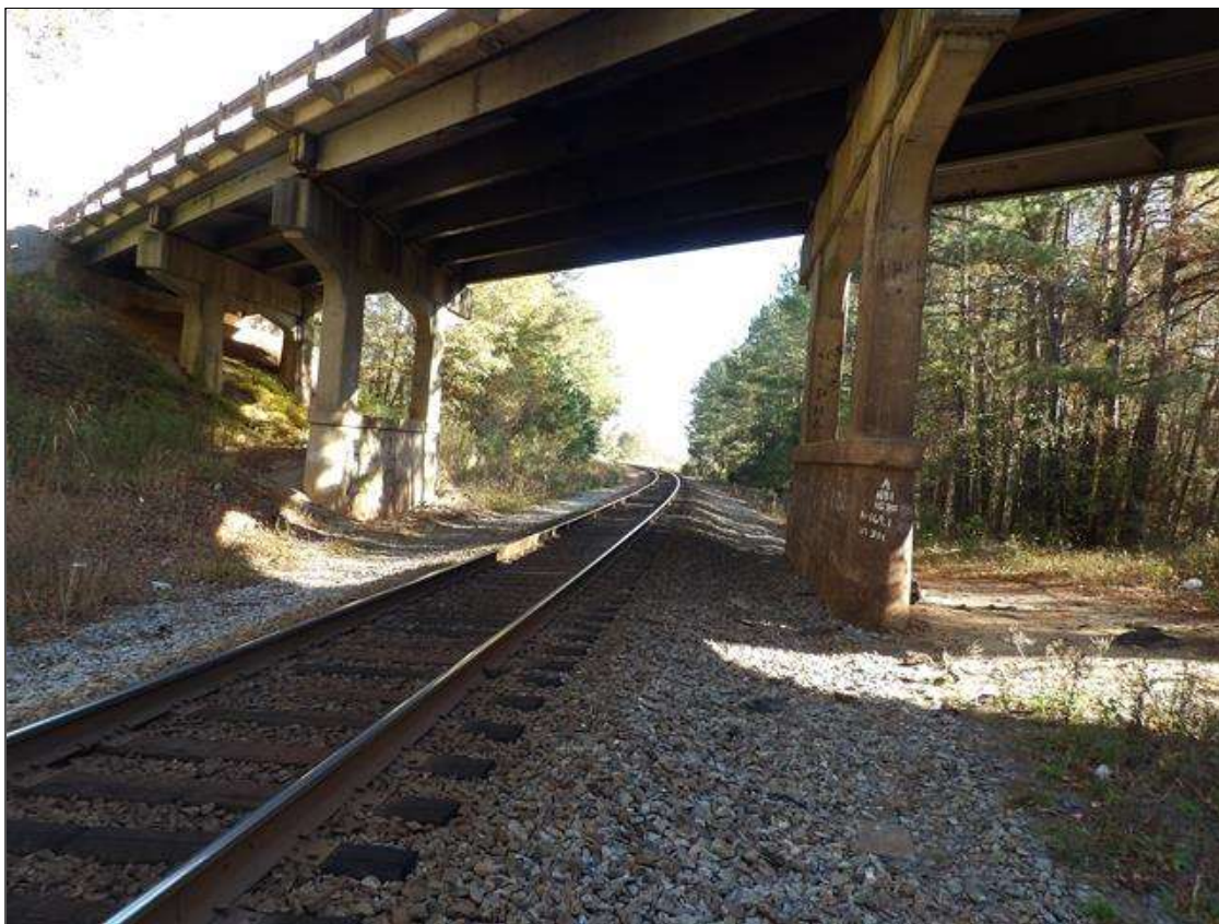
LOOKING EAST THROUGH SPAN 3
