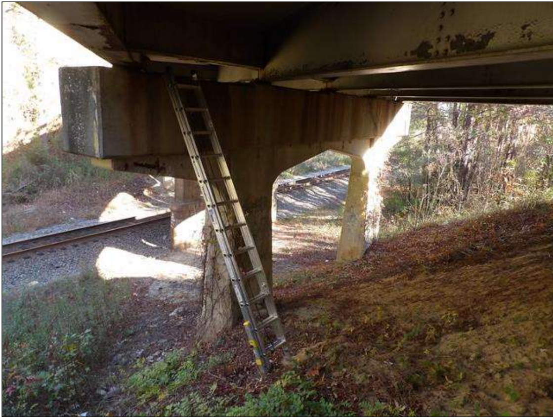
PIER 1, PIER 4 SIMILAR
