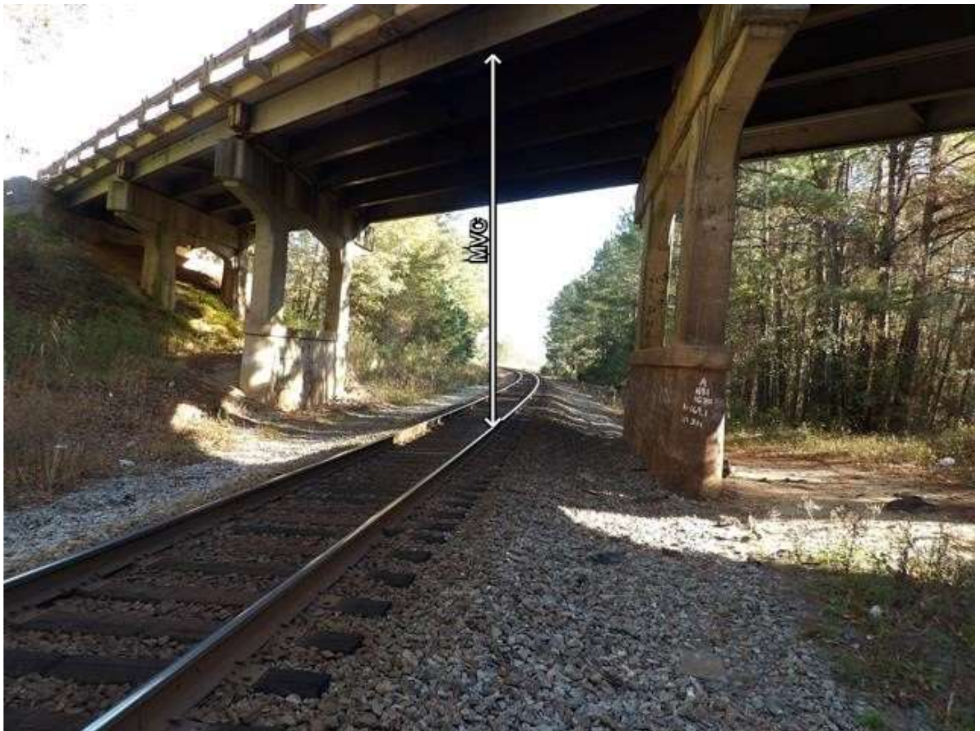
LOOKING EAST THROUGH SPAN 3
