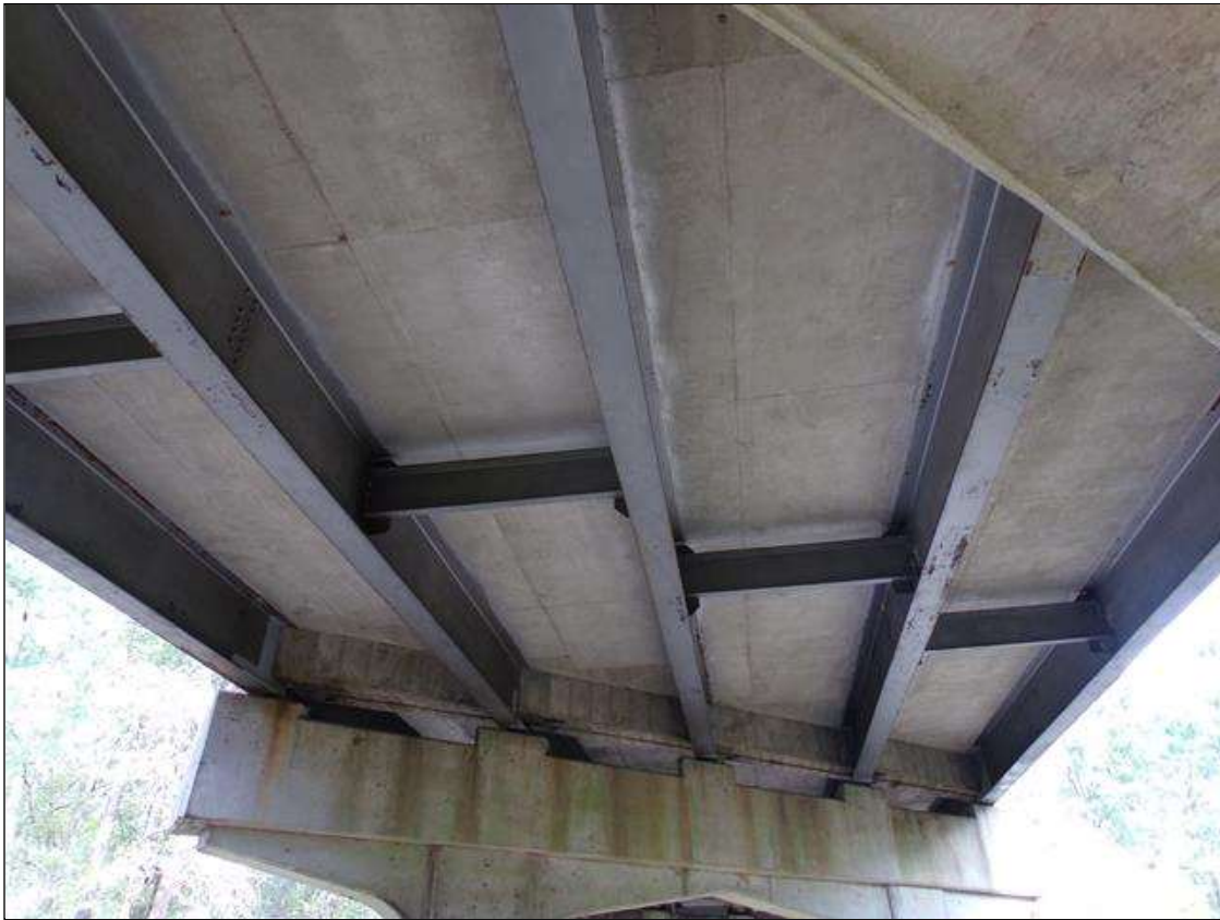
Superstructure underside span 2 shown, all others similar
