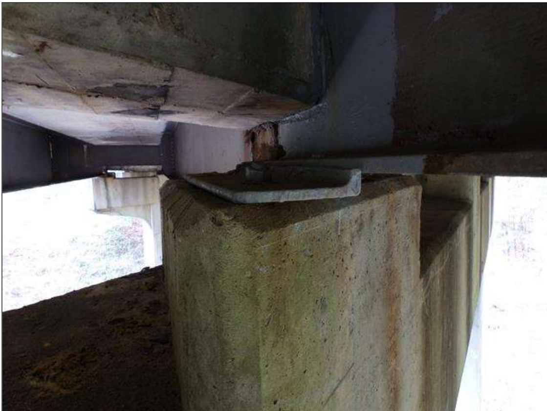
BEARING REPAIR AT BEAM 4 PIER 3 SPAN 4 EAST SIDE.
