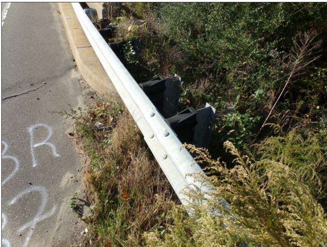
Guardrail post spacing at bridge northwest shown, northeast and southeast similar
