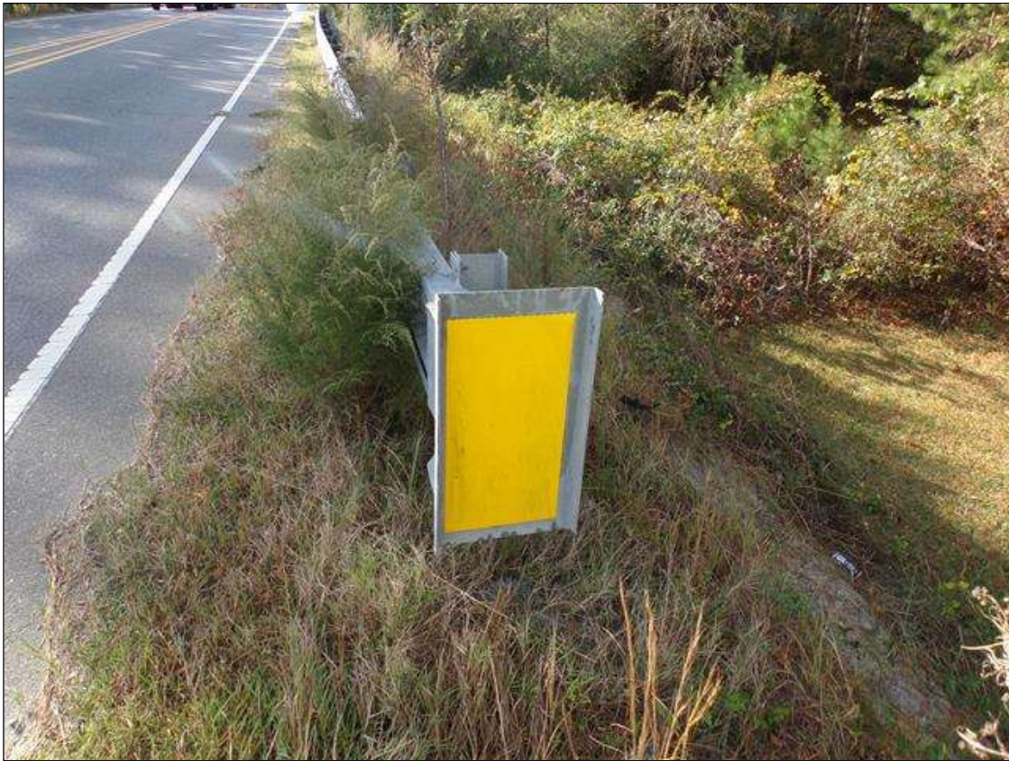
Guardrail terminal end northwest corner, northeast and southeast similar
