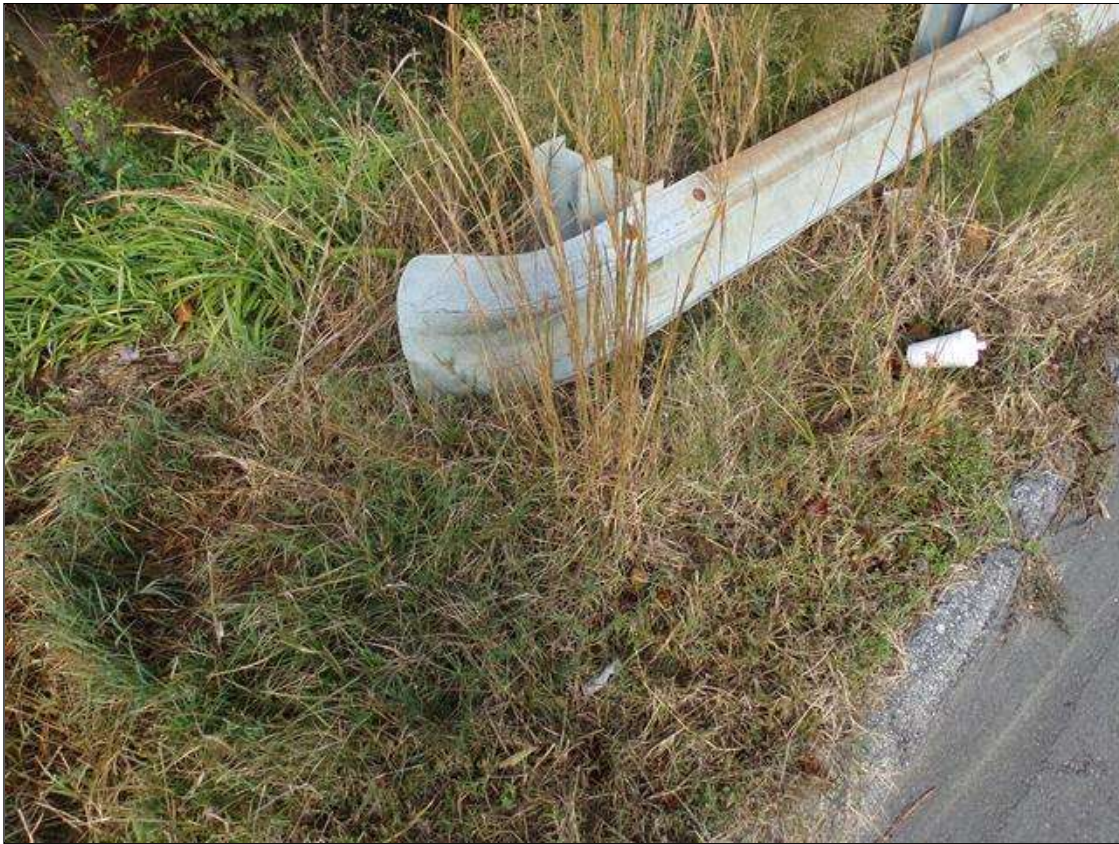
Guardrail terminal end southwest corne
