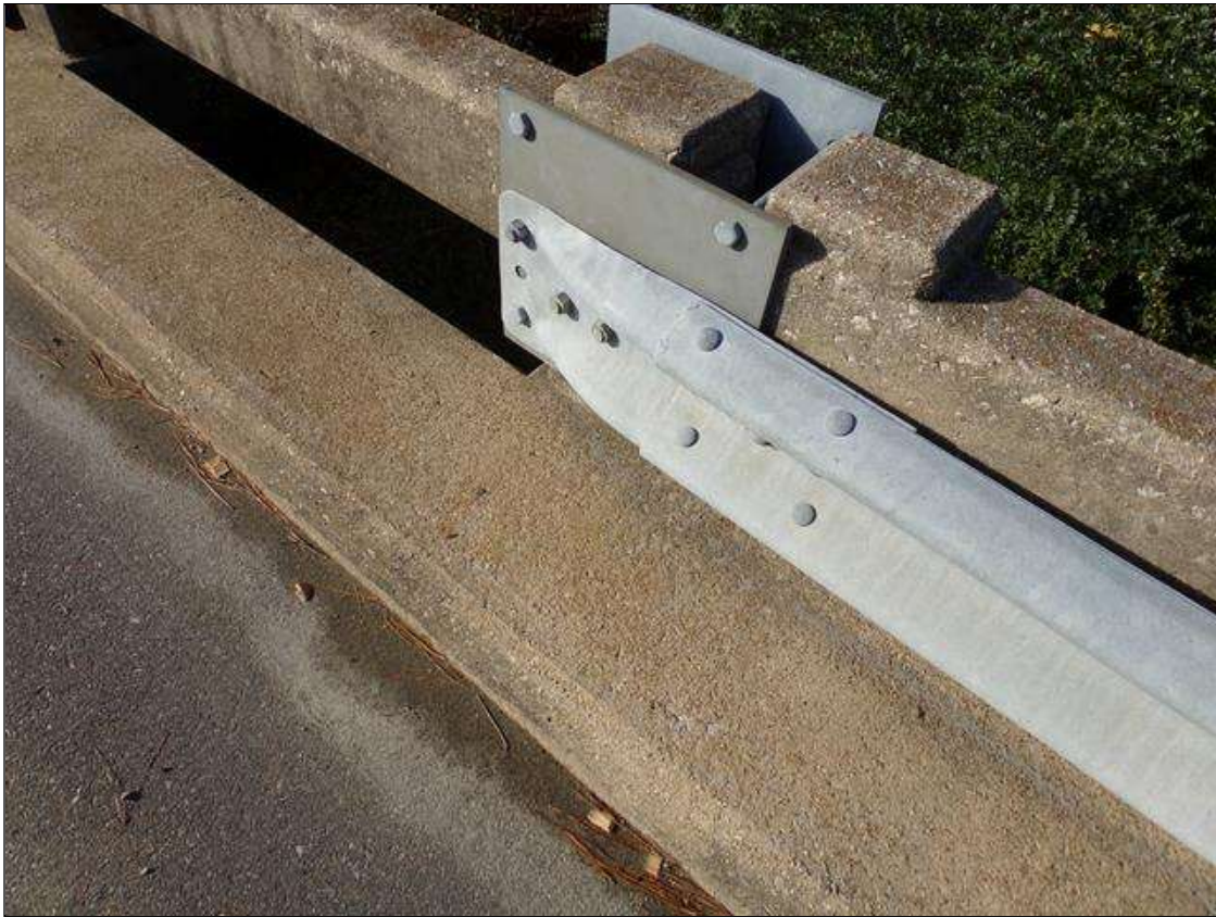
Guardrail attachment to bridge northwest shown
