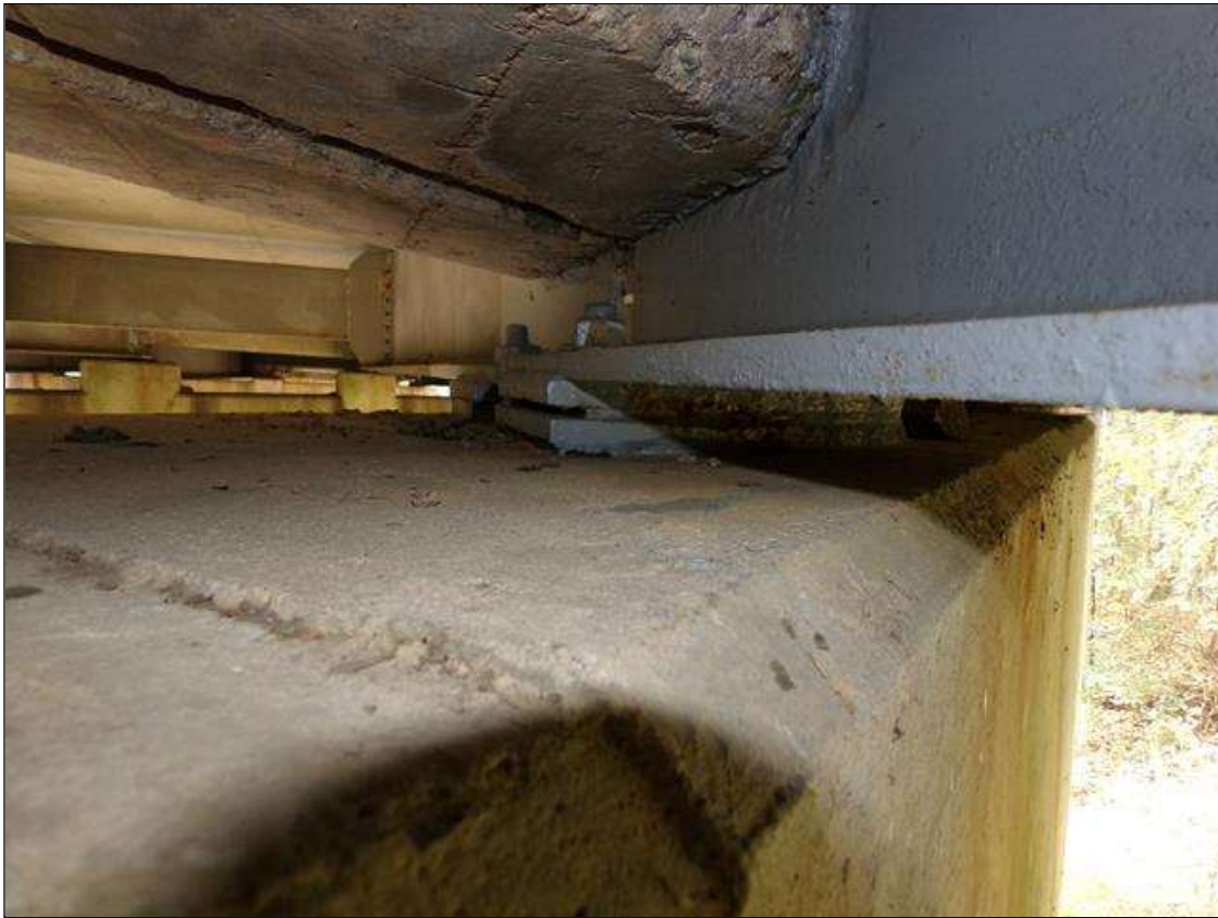
Typical bearing beam 2 at pier 4 span 5 shown
