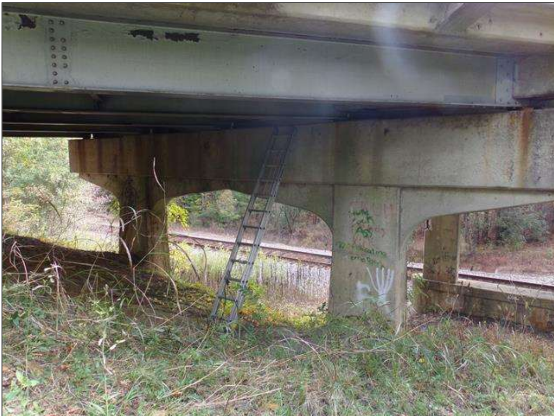
Pier 4, pier 1 similar
