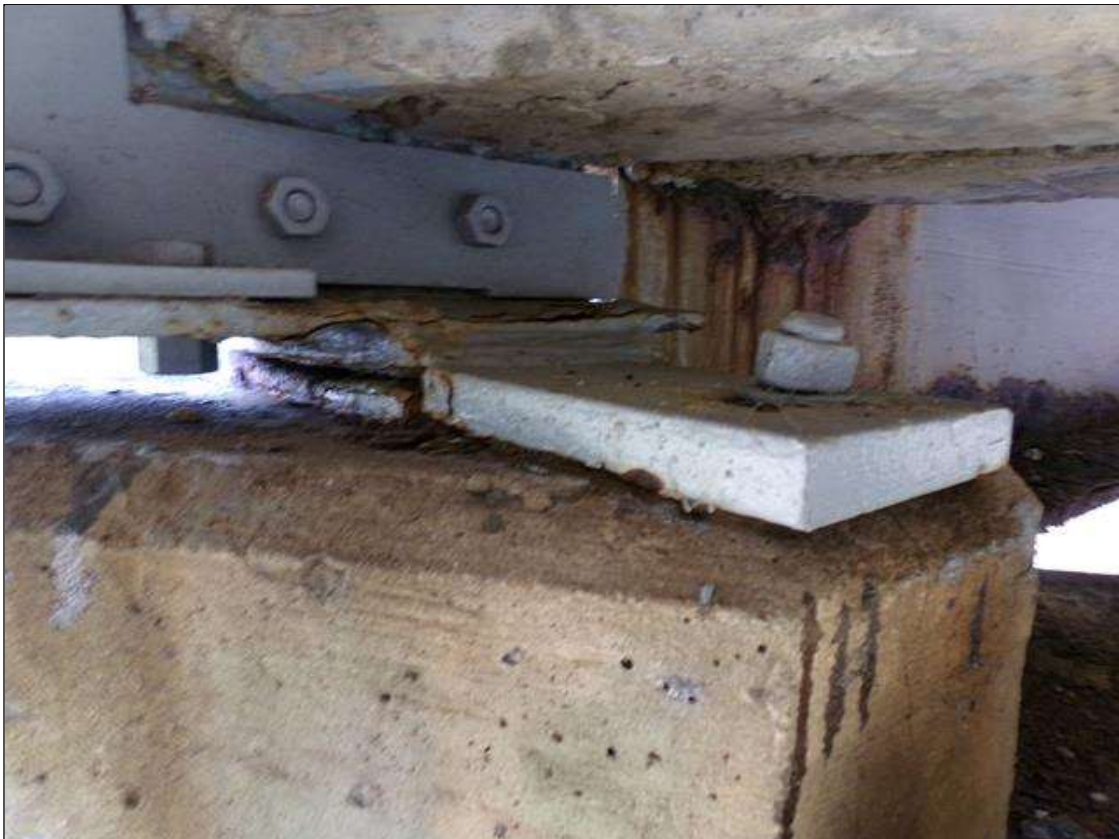
BEARING REPAIR AT BEAM 5 PIER 3 SPAN 4 WEST SIDE.
