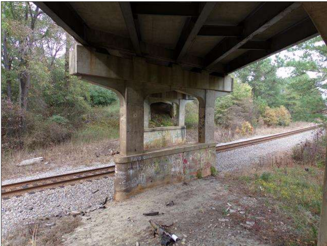
Pier 2, pier 3 similar
