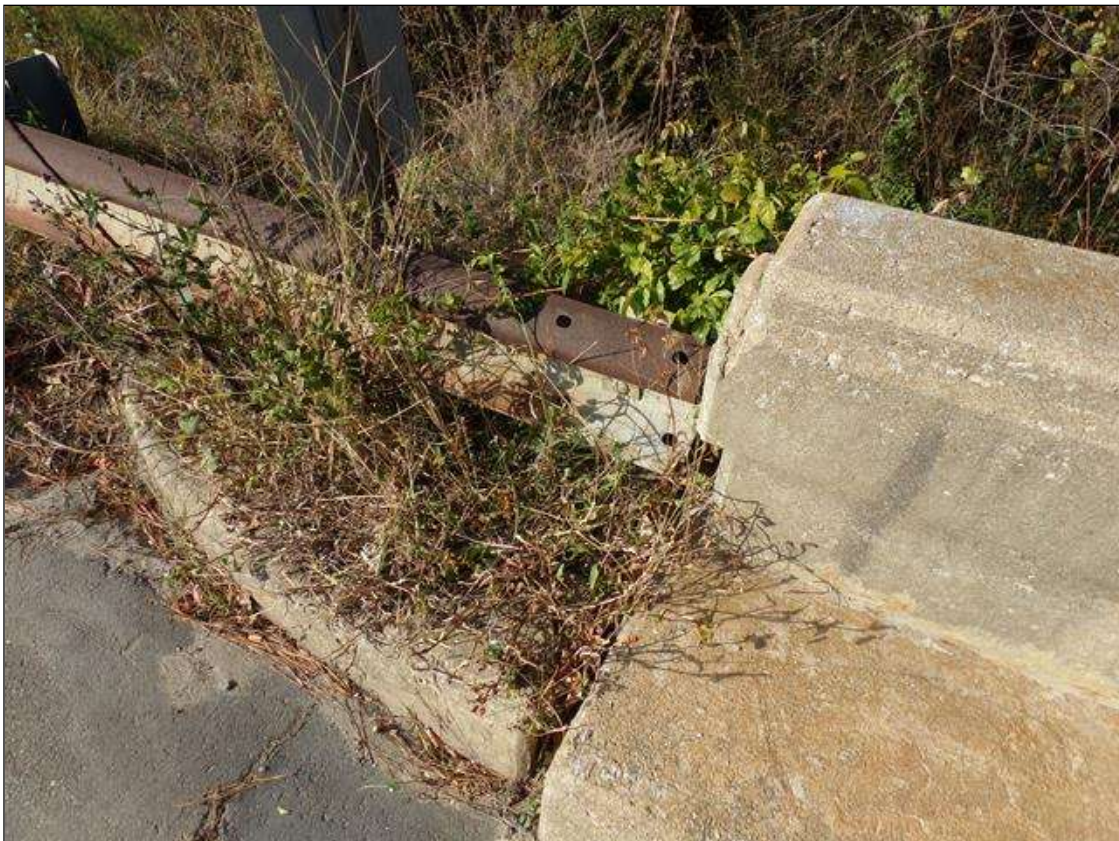
Guardrail transition at bridge southwest corner shown
