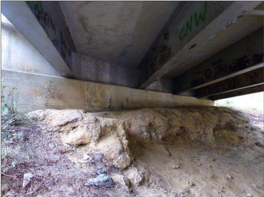
Abutment 1, abutment 2 similar
