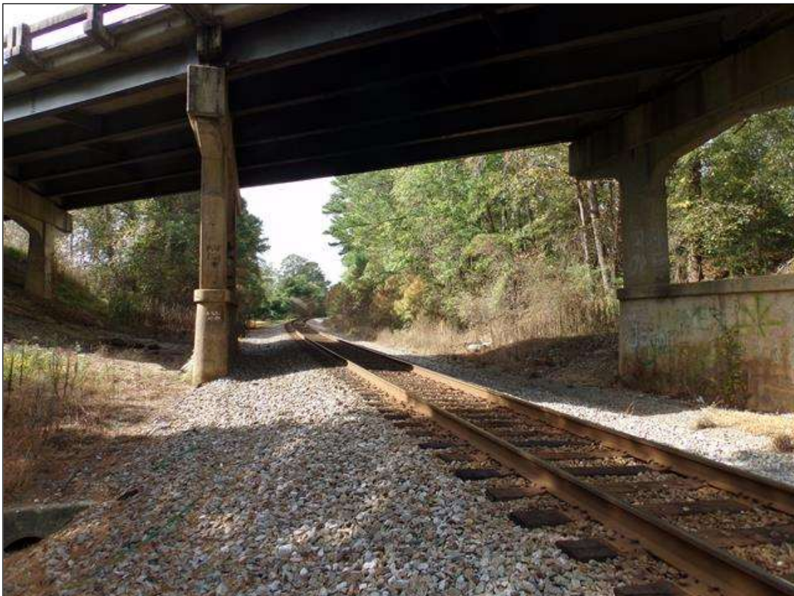
Looking west through span 3
