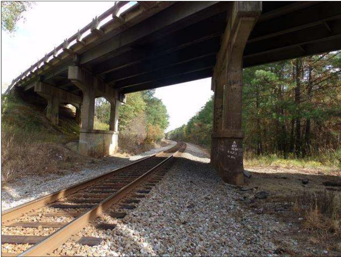
Looking east through span 3
