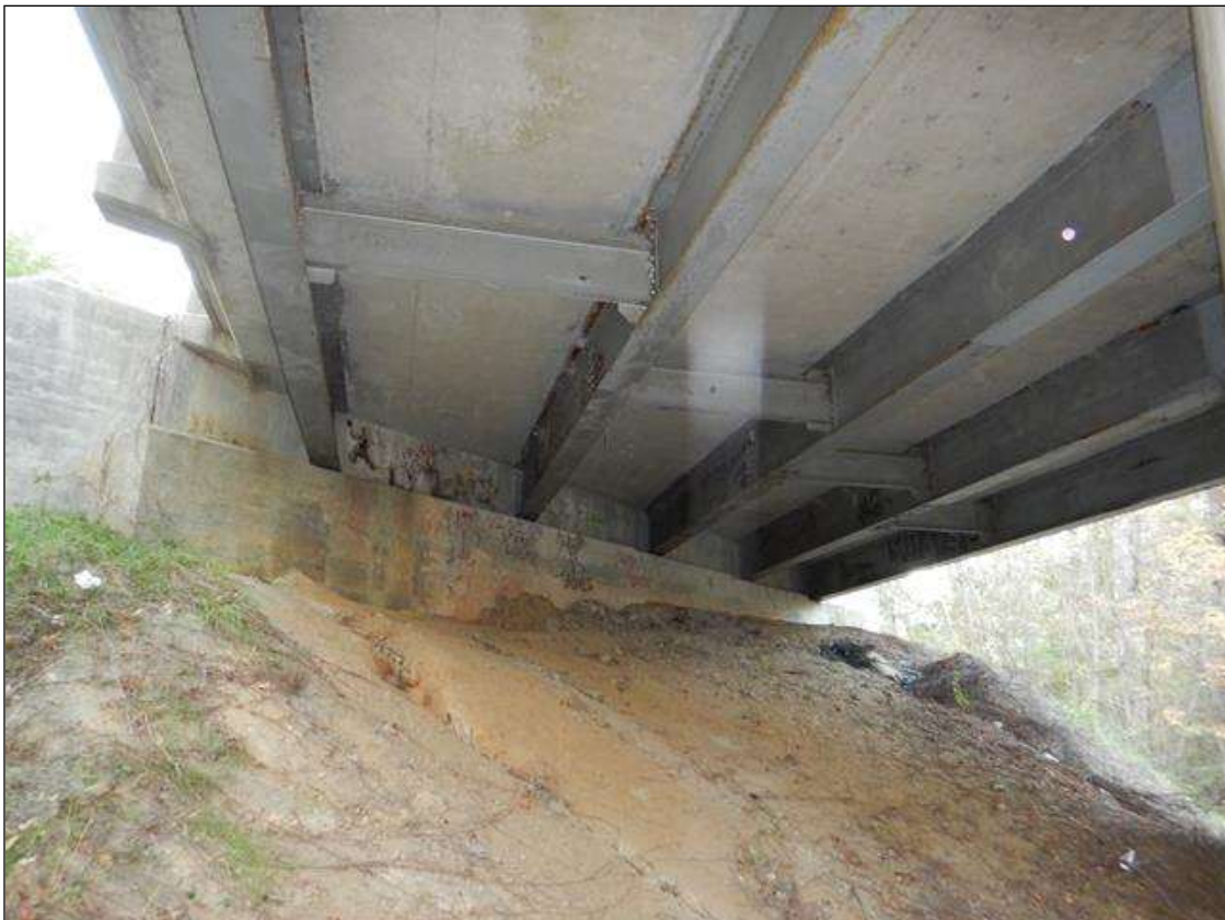
ABUTMENT 2, LOOKING NORTH
