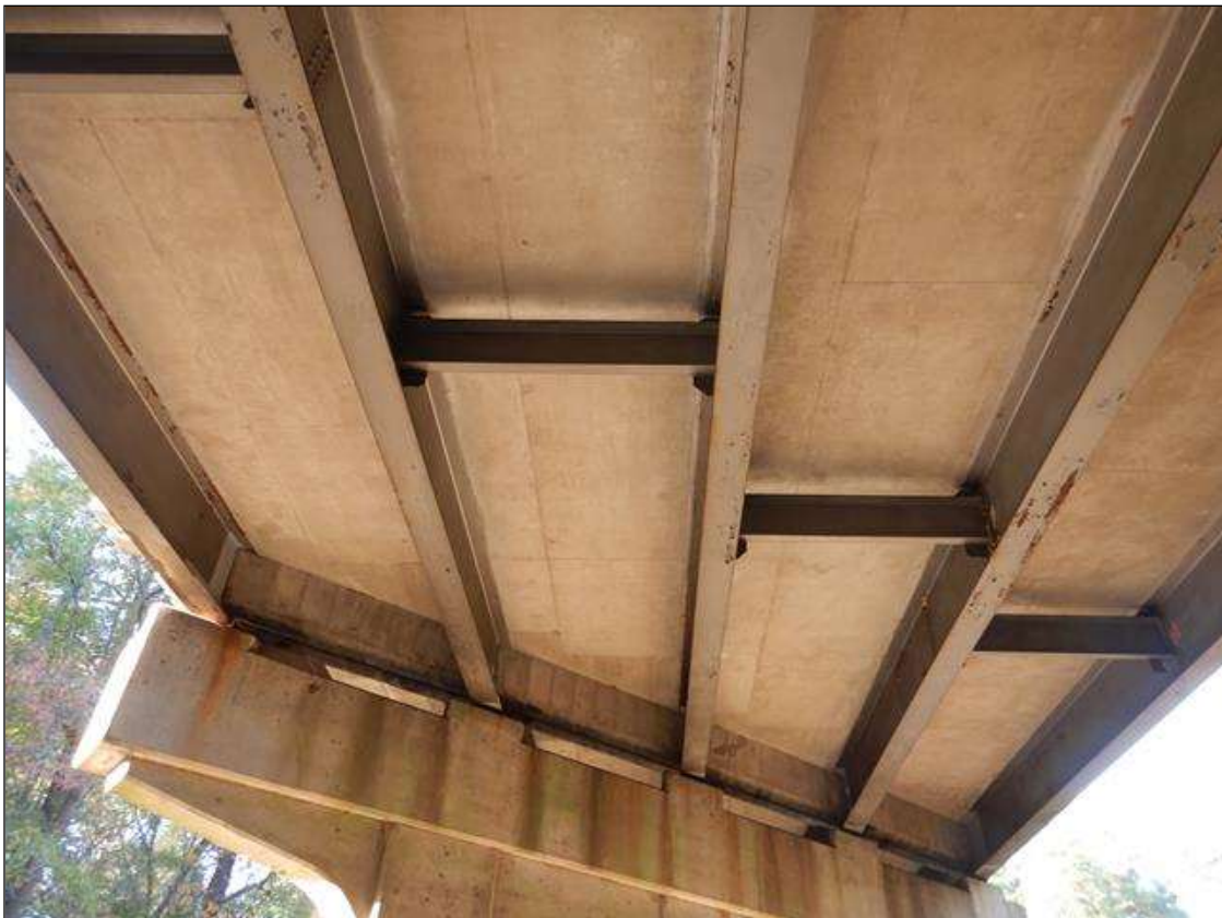
SPAN 2 SUPERSTRUCTURE, LOOKING NORTH [ALL SPANS SIMILAR]
