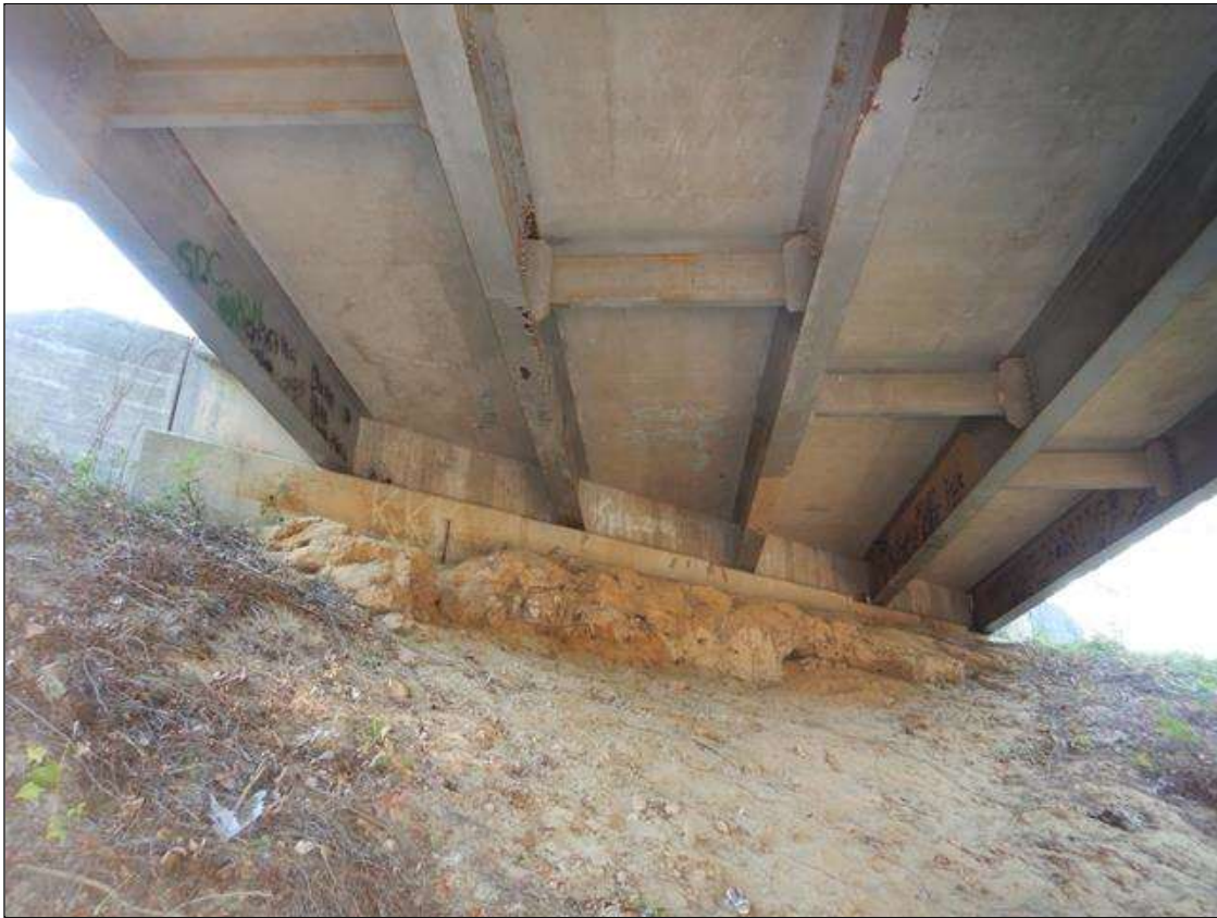
ABUTMENT 1, LOOKING SOUTH
