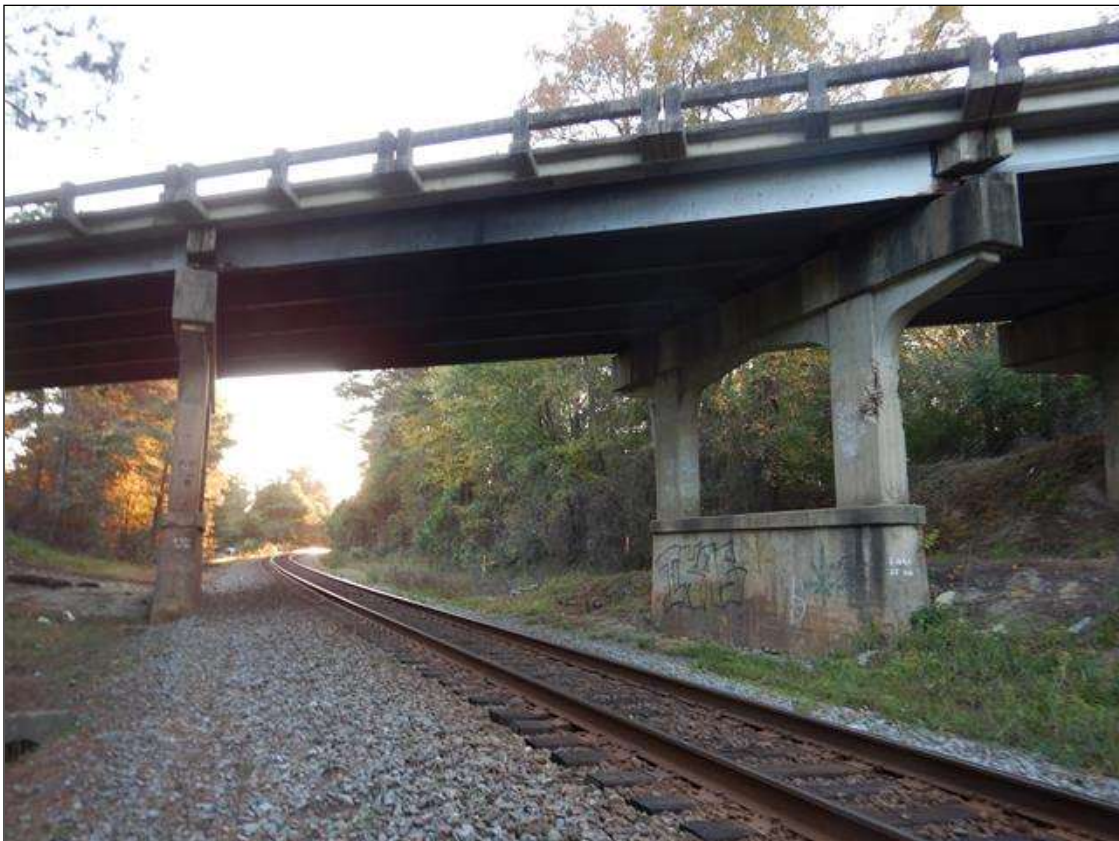
SPAN 3, LOOKING WEST AT THE RAIL LINE
