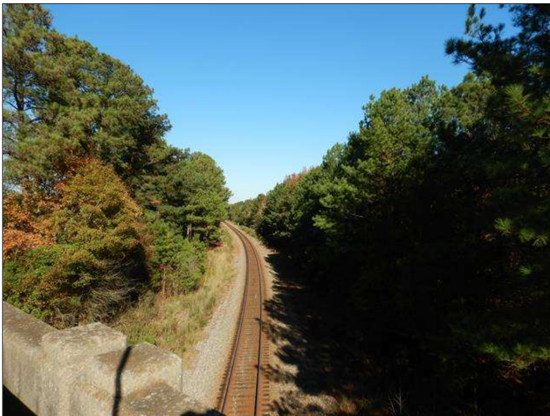
FROM THE DECK, LOOKING EAST AT THE RAIL LINE
