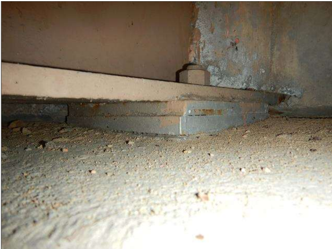
SPAN 1 GIRDER 3 NEAR BEARING [TYPICAL BEARING AT THE ABUTMENTS]
