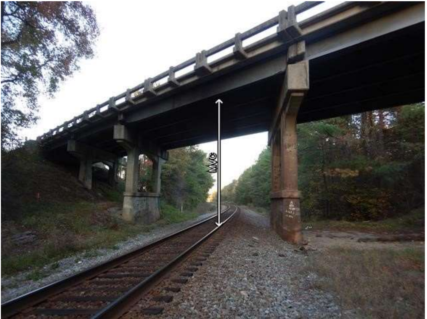
SPAN 3, LOOKING EAST AT THE RAIL LINE
