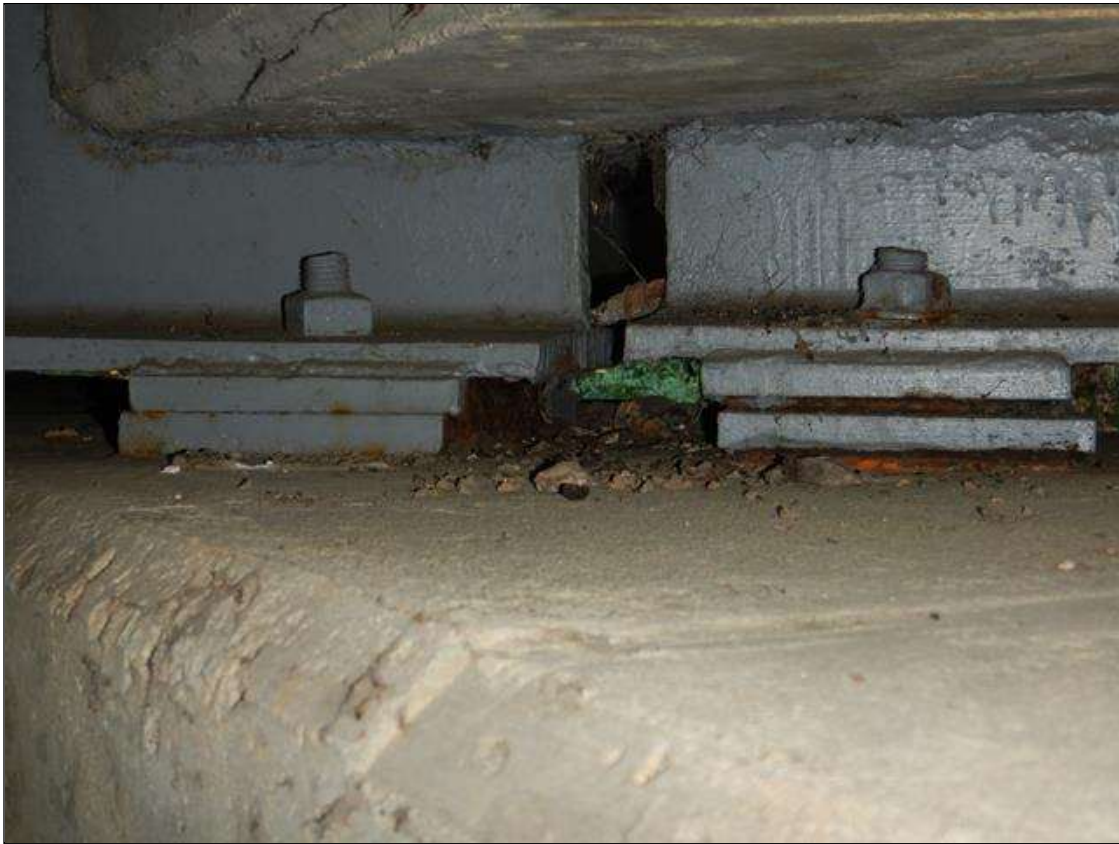
GIRDERS 2 BEARINGS AT BENT 4 [TYPICAL BEARINGS AT THE BENTS]
