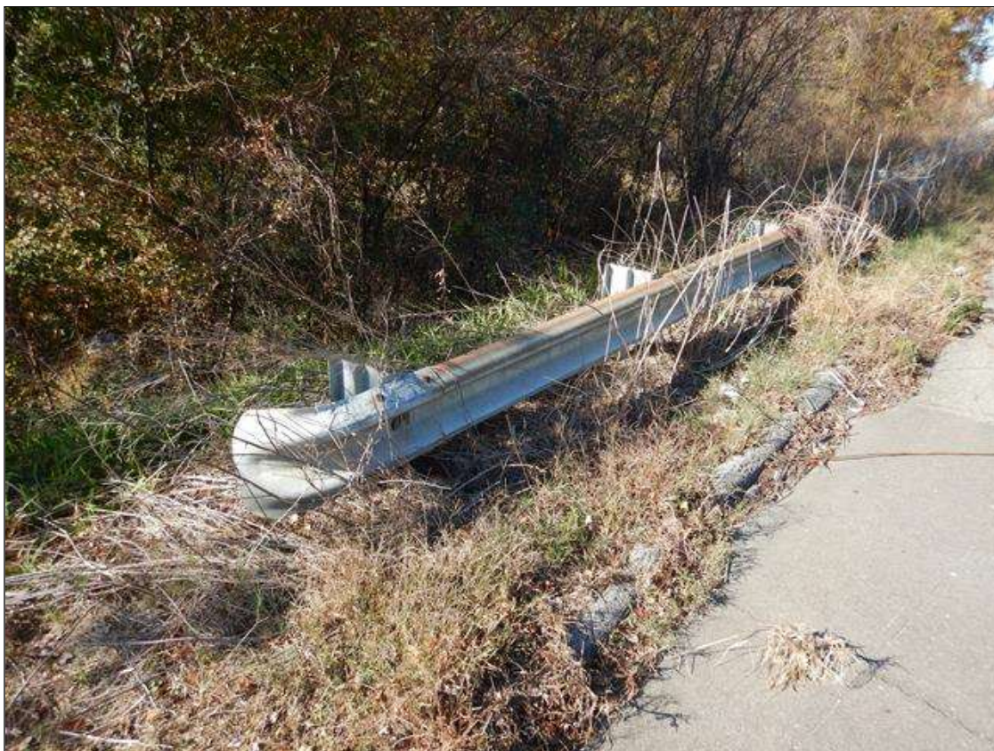
SOUTHWEST CORNER, GUARDRAIL END
