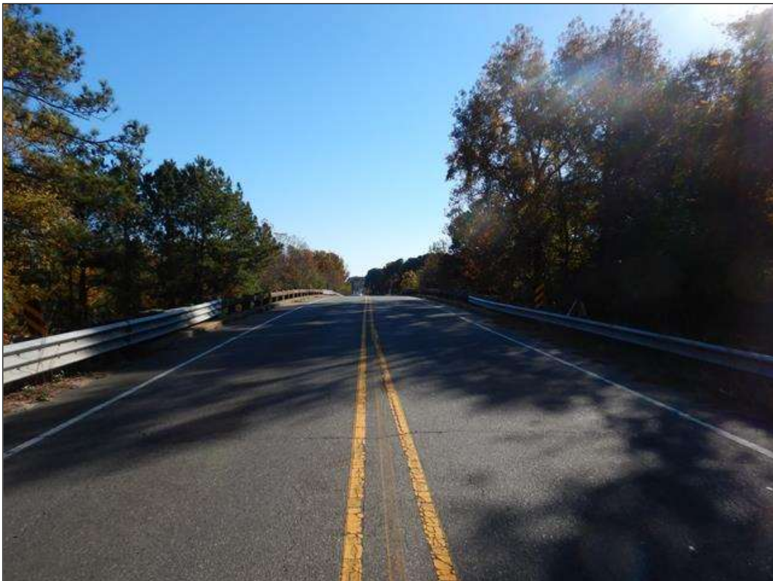
NORTH APPROACH LOOKING SOUTH
