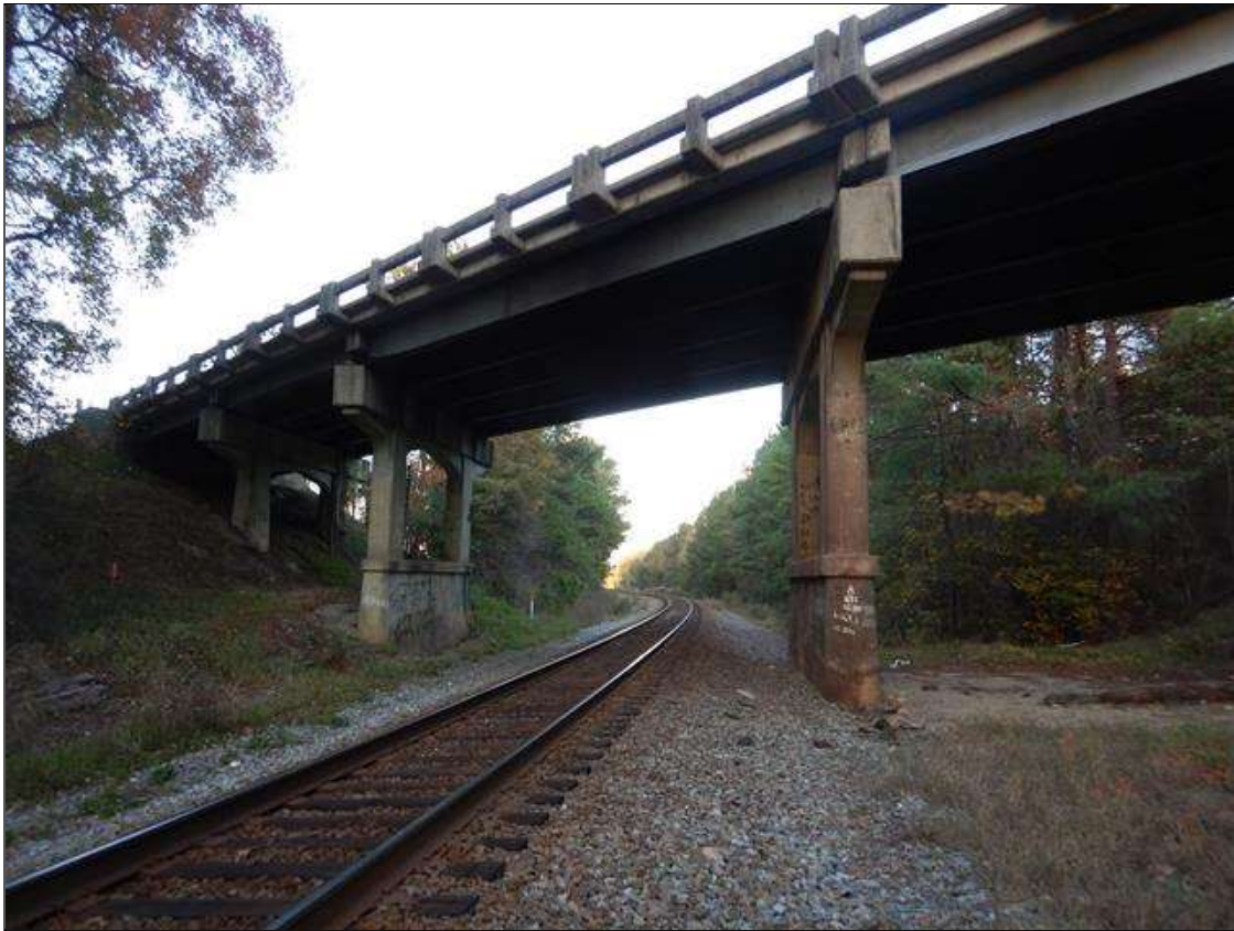
SPAN 3, LOOKING EAST AT THE RAIL LINE
