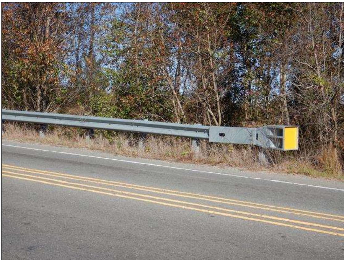
SOUTHEAST CORNER, GUARDRAIL END
