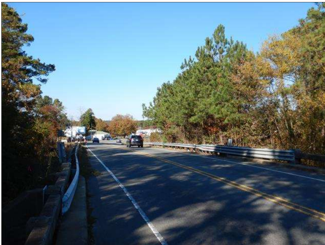
FROM THE DECK, LOOKING NORTH
