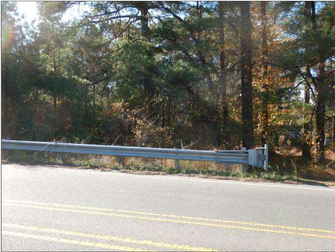
NORTHWEST CORNER, GUARDRAIL END
