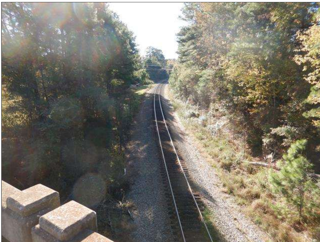
FROM THE DECK, LOOKING WEST AT THE RAIL LINE
