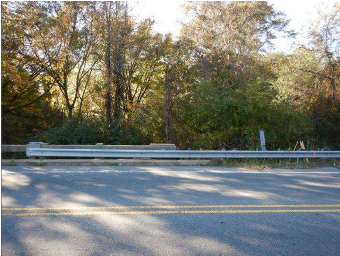
NORTHWEST CORNER, GUARDRAIL TRANSITION AND CONNECTION
