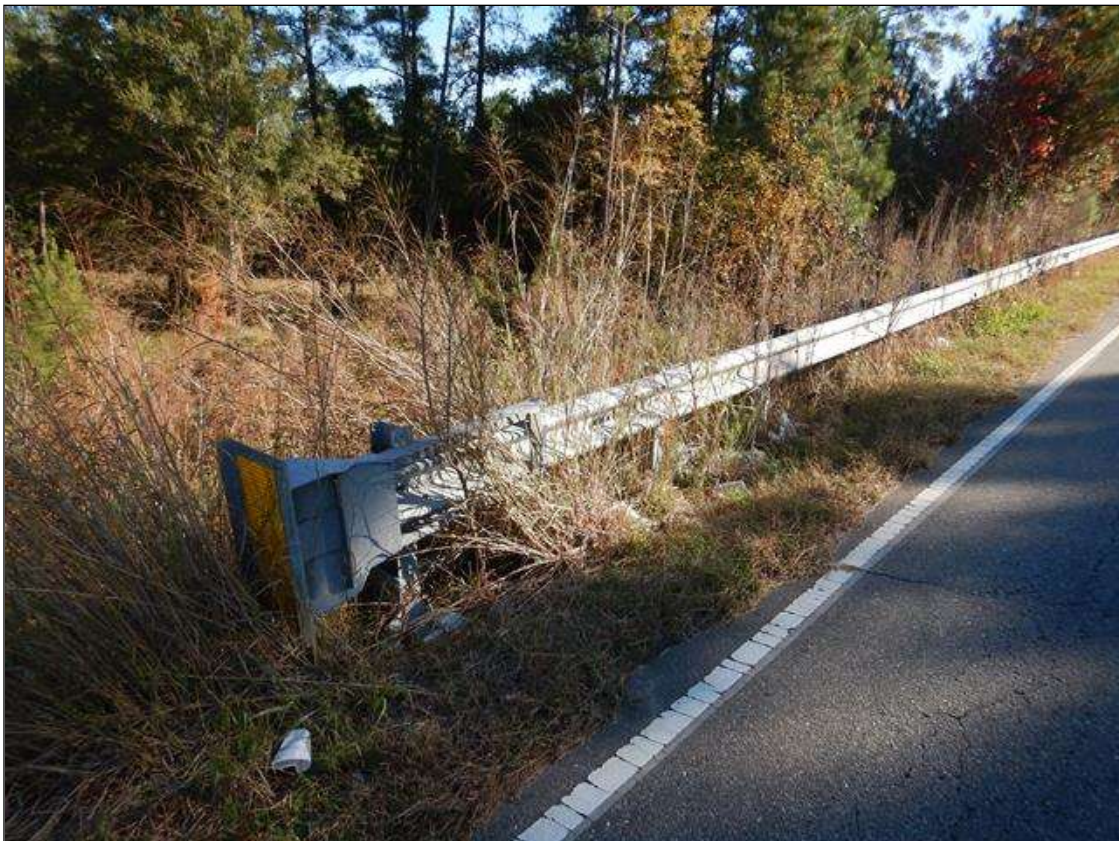
NORTHEAST CORNER, GUARDRAIL END
