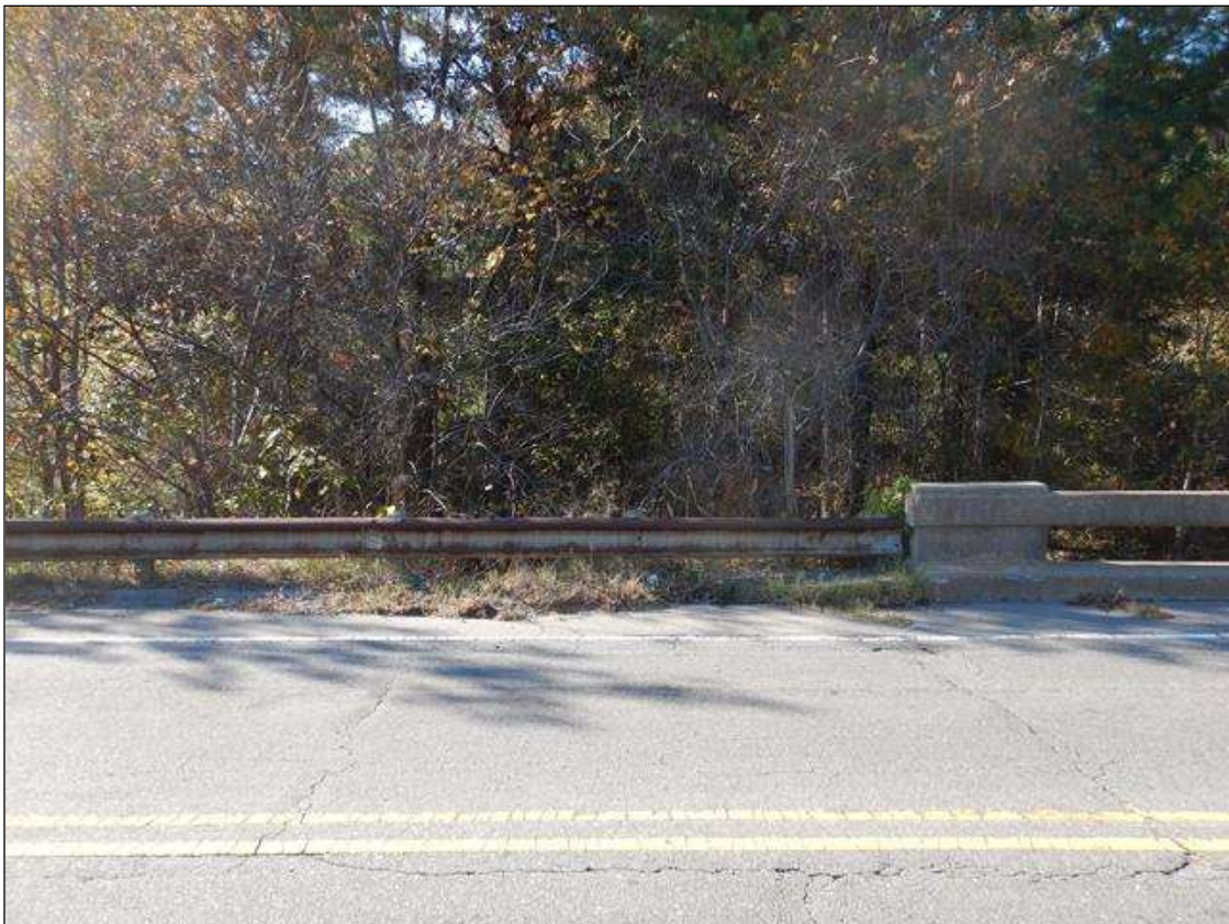
SOUTHWEST CORNER, GUARDRAIL TRANSITION
