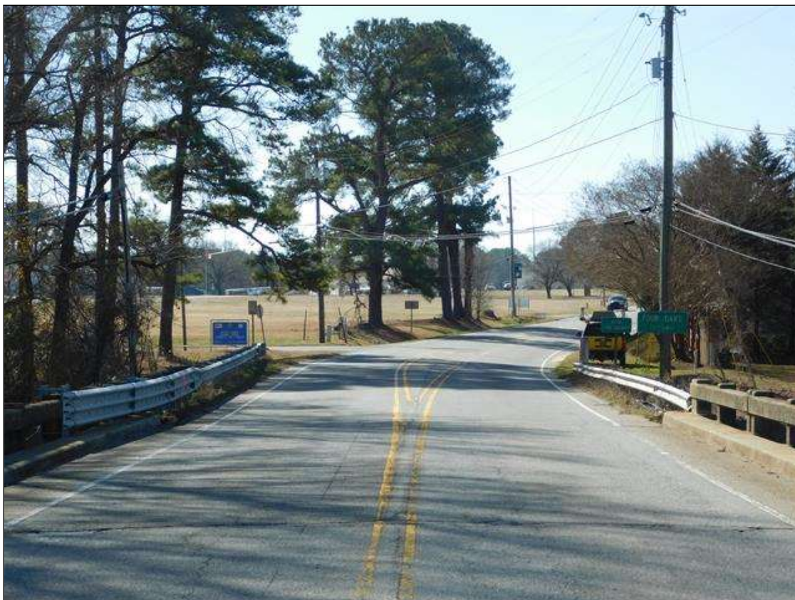
LOOKING AT SOUTH APPROACH
