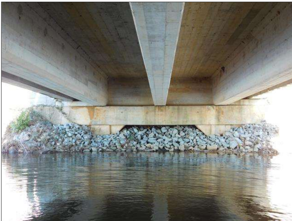
END BENT 2 OVERVIEW
