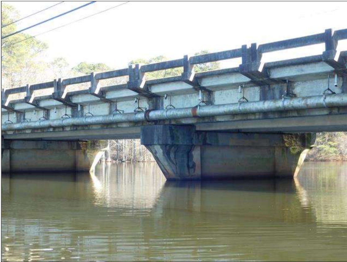
BENT 1 SPAN 1 SIDE
