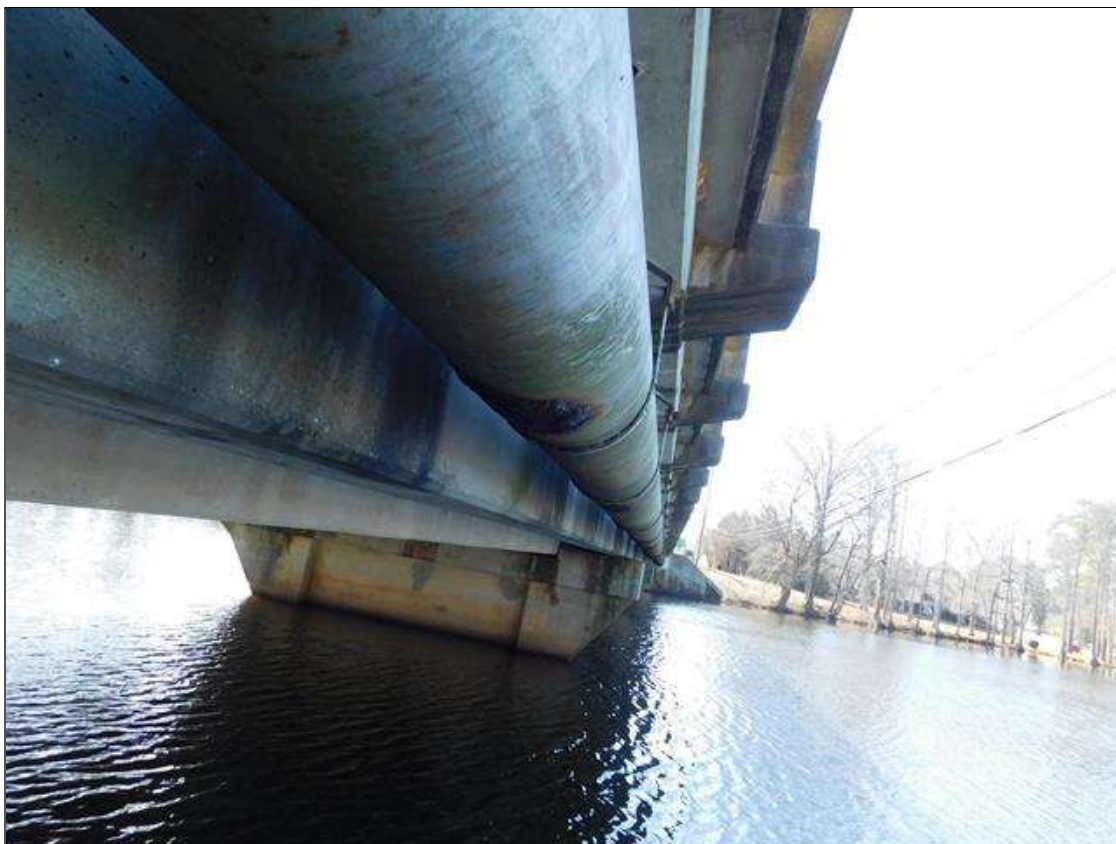
UTILITIES ALONG THE LEFT SIDE OVERHANG
