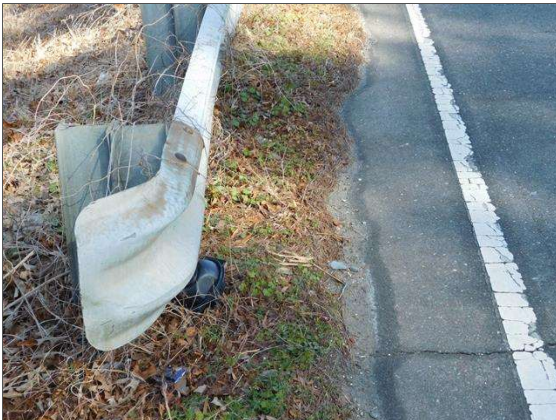
APPROACH GUARDRAIL TERMINAL END LEFT SIDE AT SOUTH END
