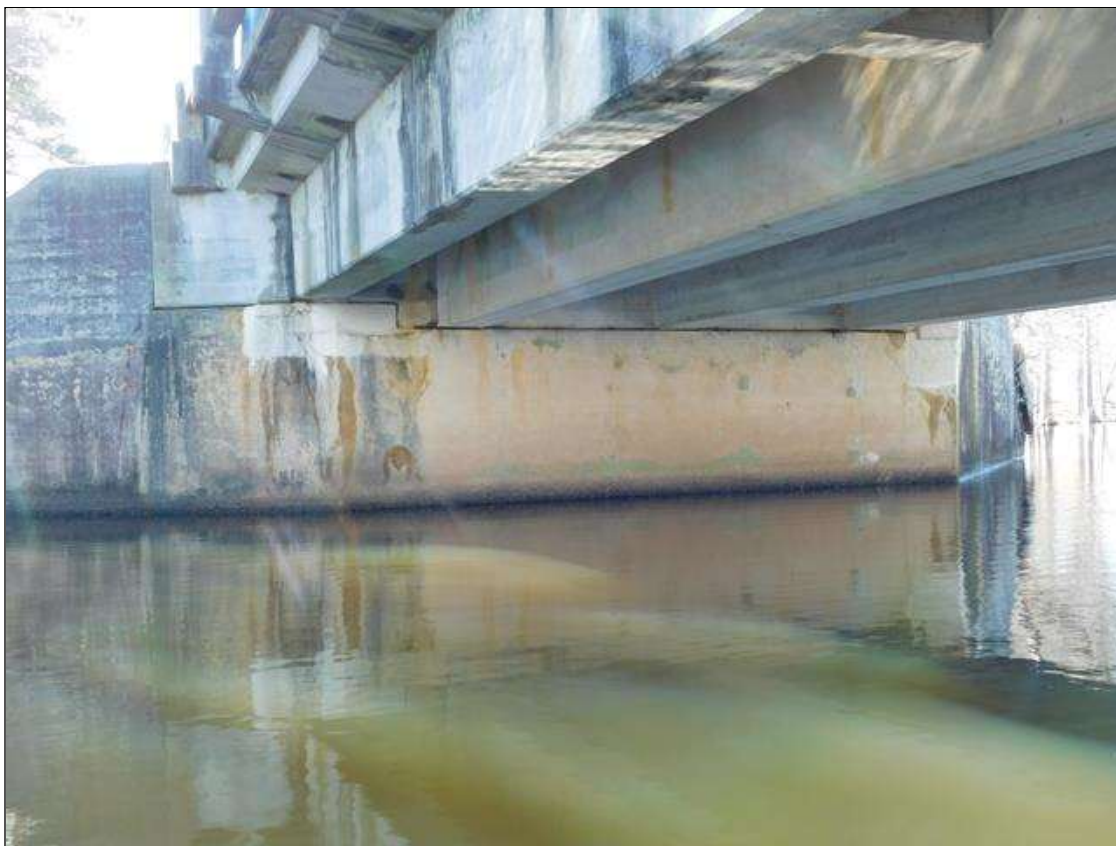
END BENT 1 OVERVIEW
