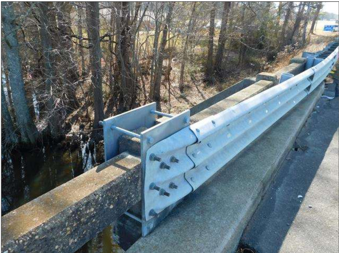
APPROACH GUARDRAIL CONNECTION
