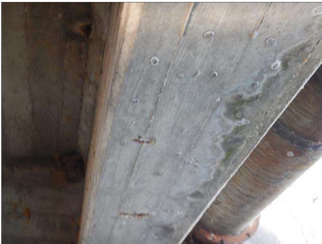
Span 1 Beam 1: SHALLOW SPALLS WITH EXPOSED REBAR IN BOTTOM OF GIRDER UP TO 6 FEET OUT FROM END BENT 1.
