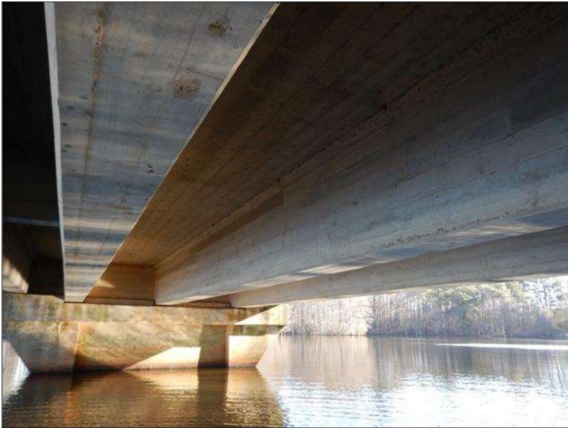
UNDERSIDE OF THE DECK, SPAN 1 SHOWN
