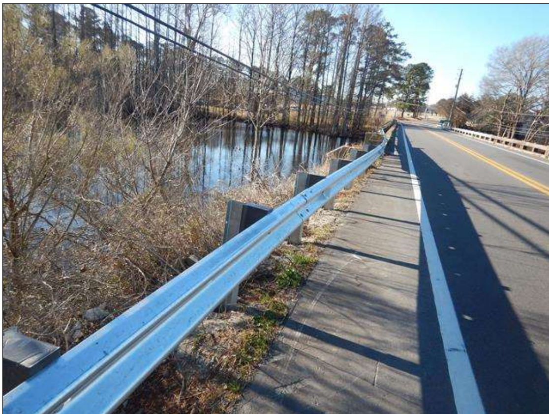
FAR RIGHT GUARDRAIL REPLACED
