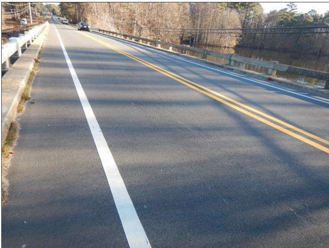
NEW 1/2 INCH ASPHALT WEARING ADDED TO THE DECK
