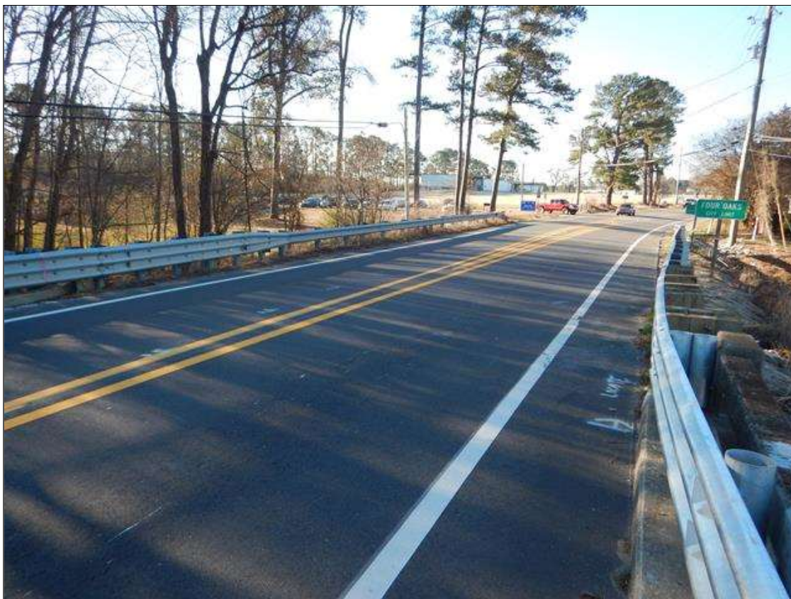
APPROACH ROADWAY RESURFACED, SOUTH APPROACH SHOWN
