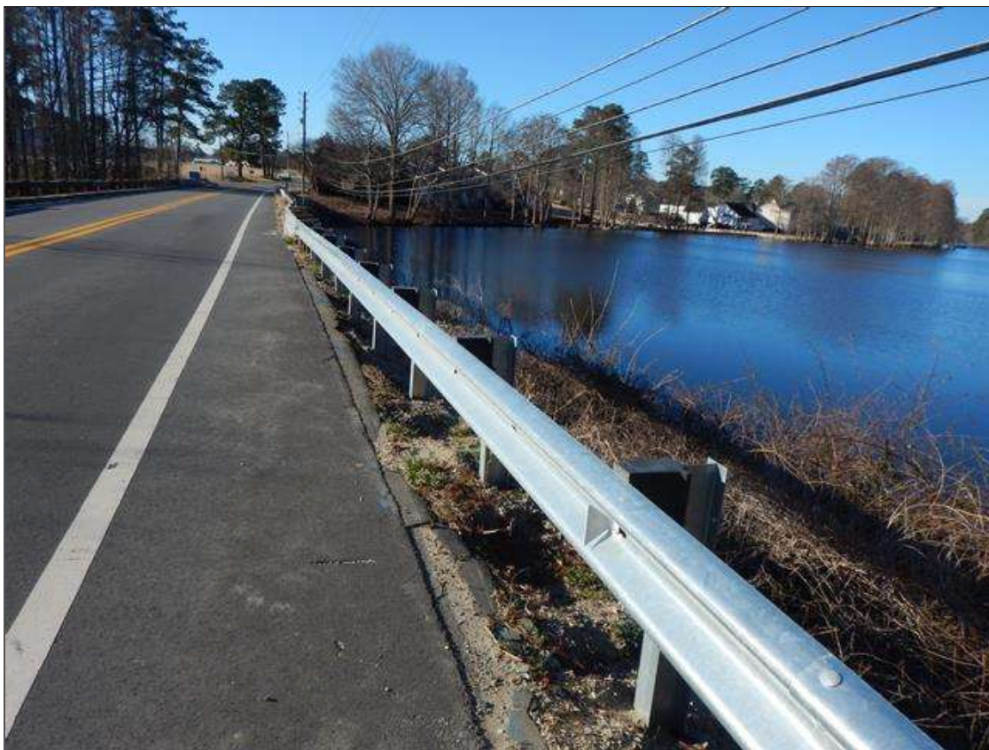
FAR LEFT GUARDRAIL REPLACED
