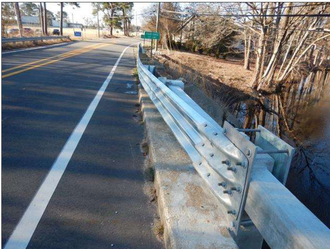
NEAR LEFT RAIL GUARDRAIL REPAIRED
