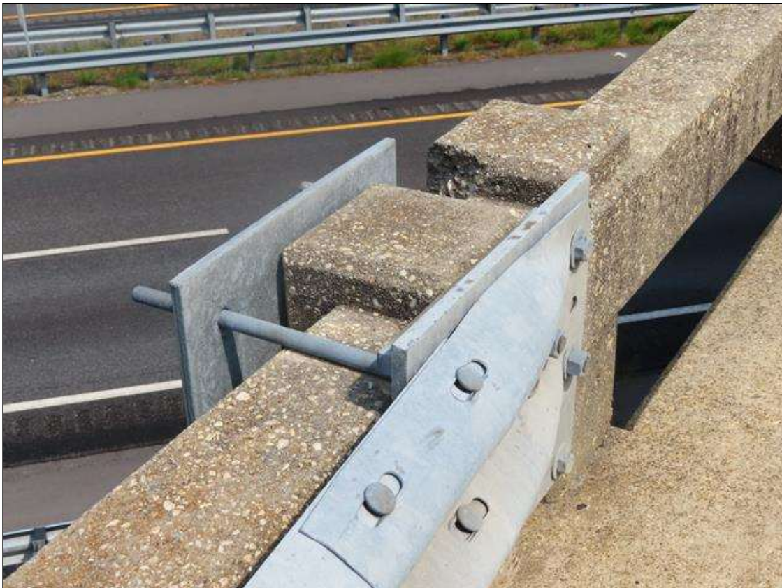
GUARDRAIL ATTACHMENT LEFT SIDE SOUTH END
