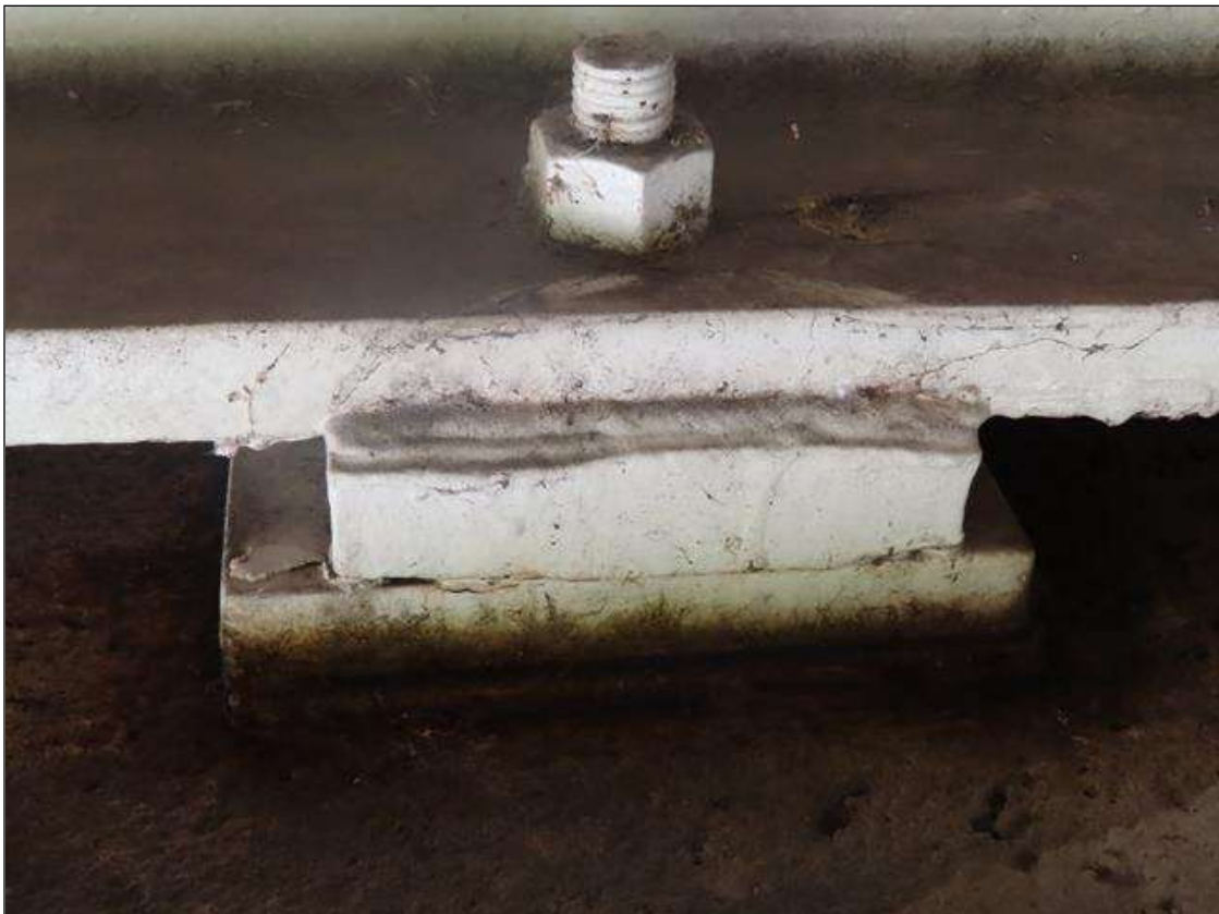
BEARING ASSEMBLY END BENT 1
