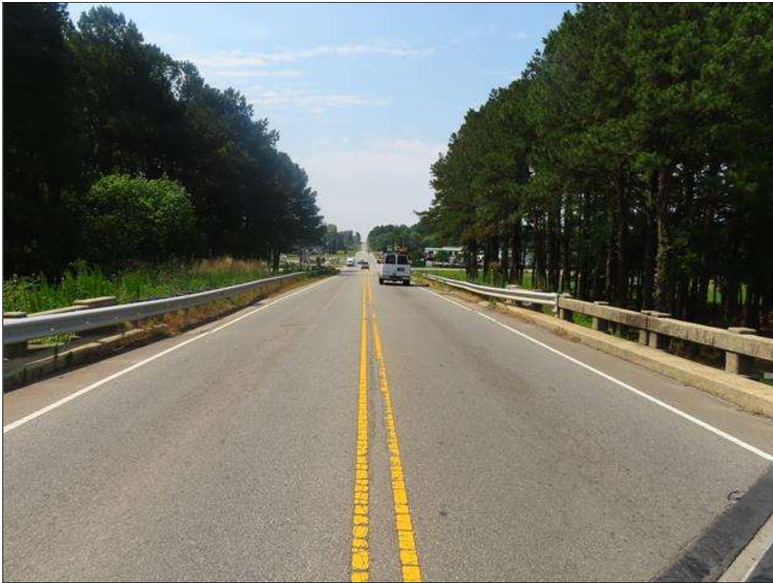
LOOKING SOUTH AT APPROACH ROADWAY SOUTH END
