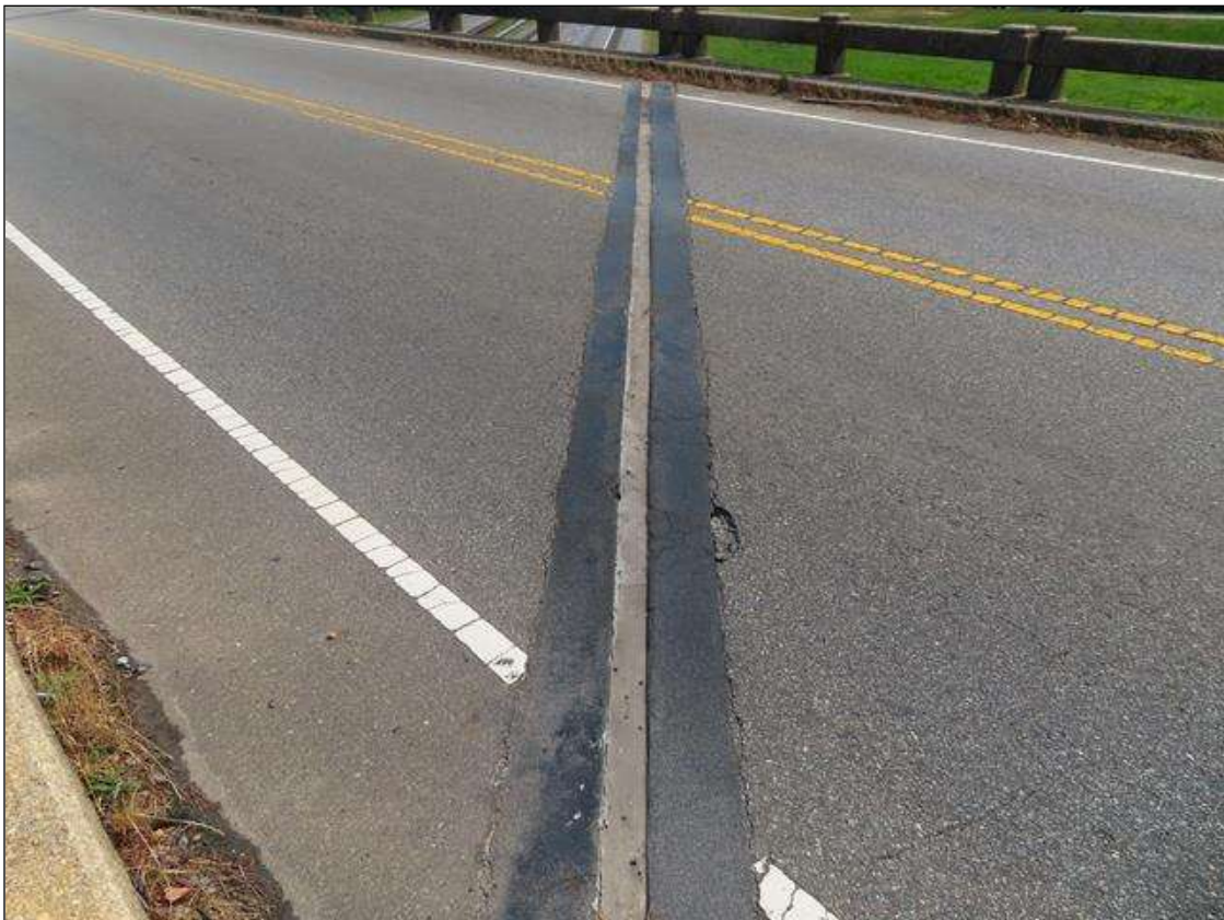
JOINT OVER BENT 1
