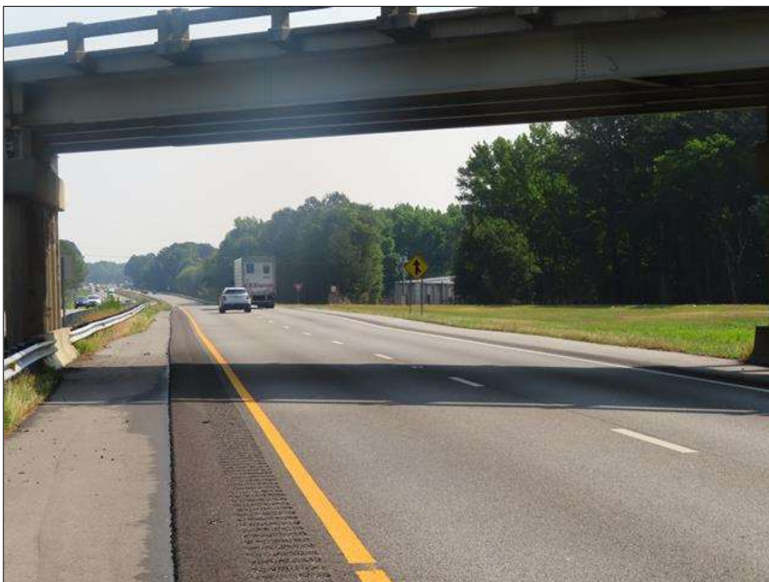
LOOKING NORTH THRU SPAN 2
