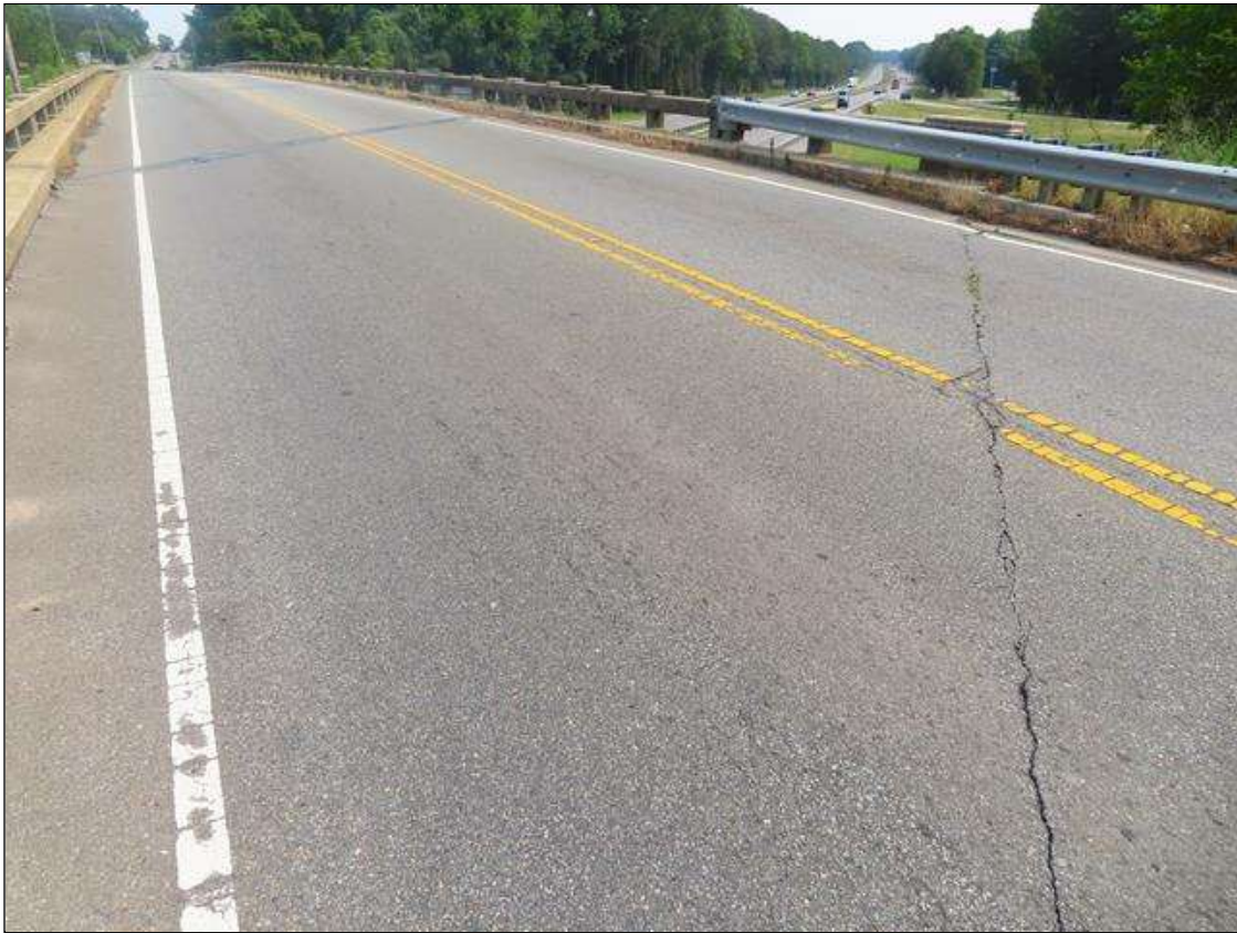
ASPHALT WEARING SURFACE OVERVIEW ALL OTHER SPANS SIMILAR
