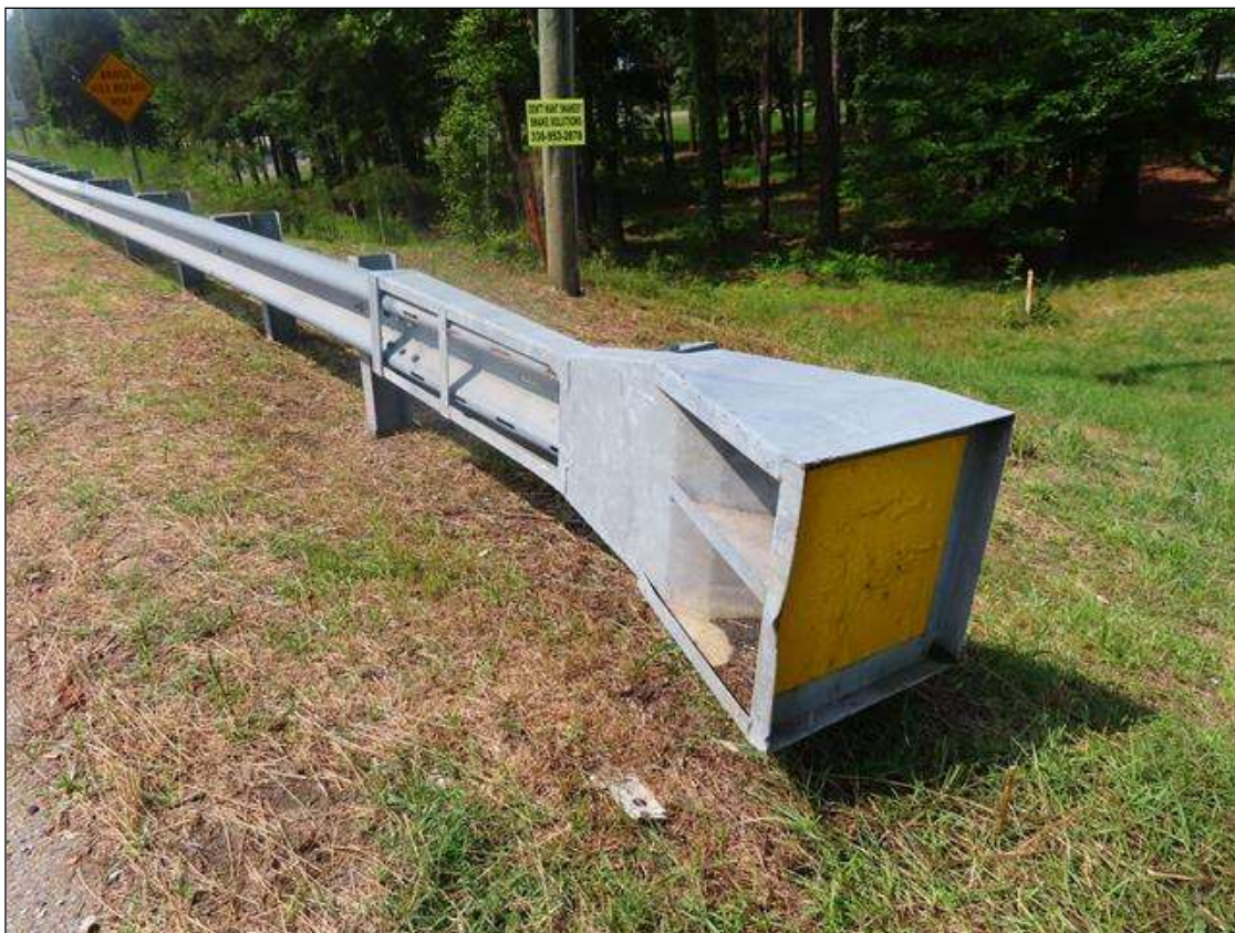
GUARDRAIL TERMINAL END LEFT SIDE NORTH END
