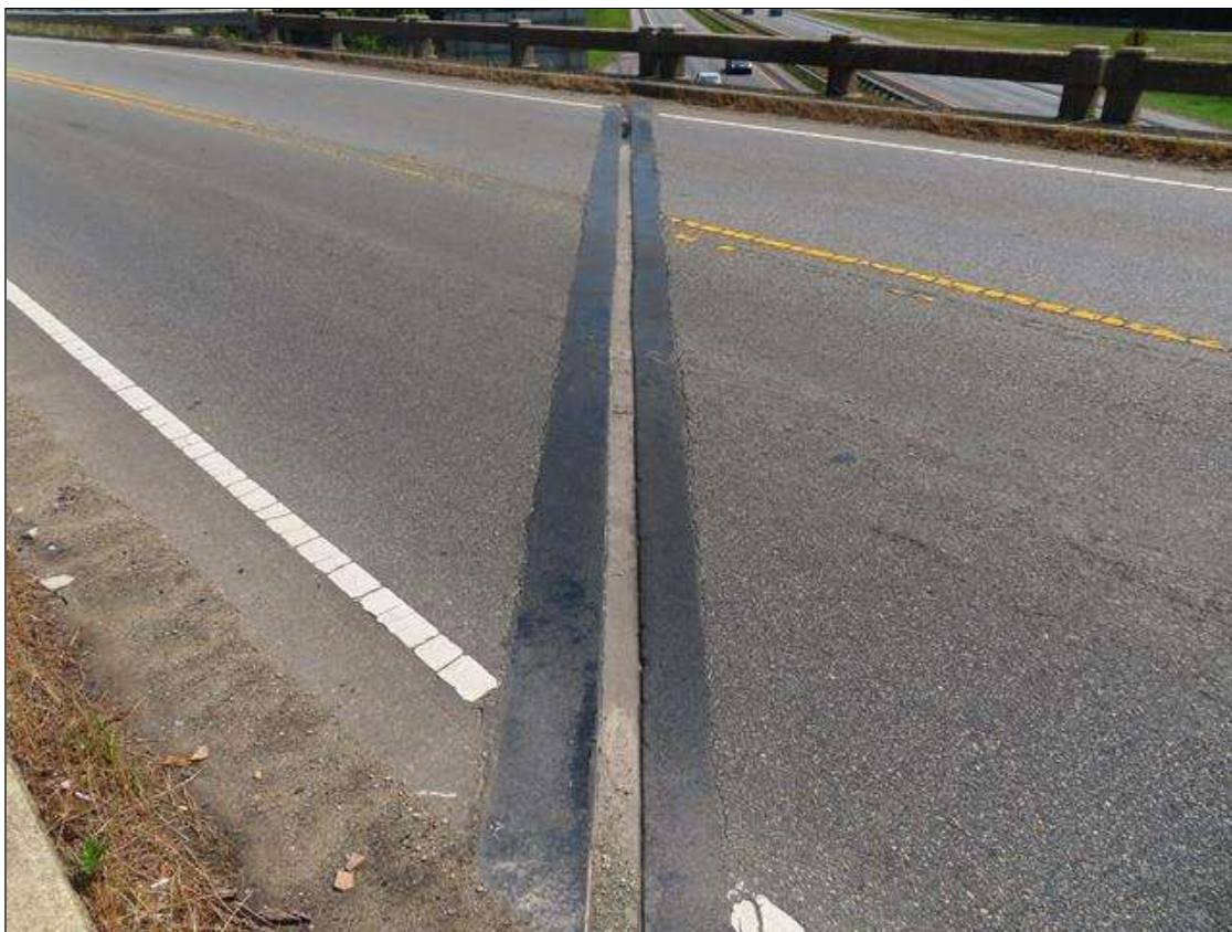
JOINT OVER BENT 3
