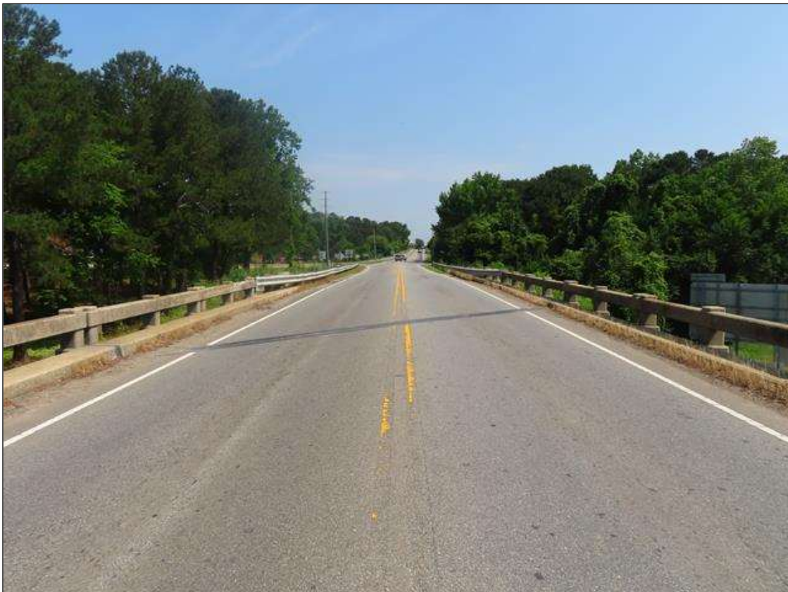
LOOKING NORTH AT APPROACH ROADWAY NORTH END
