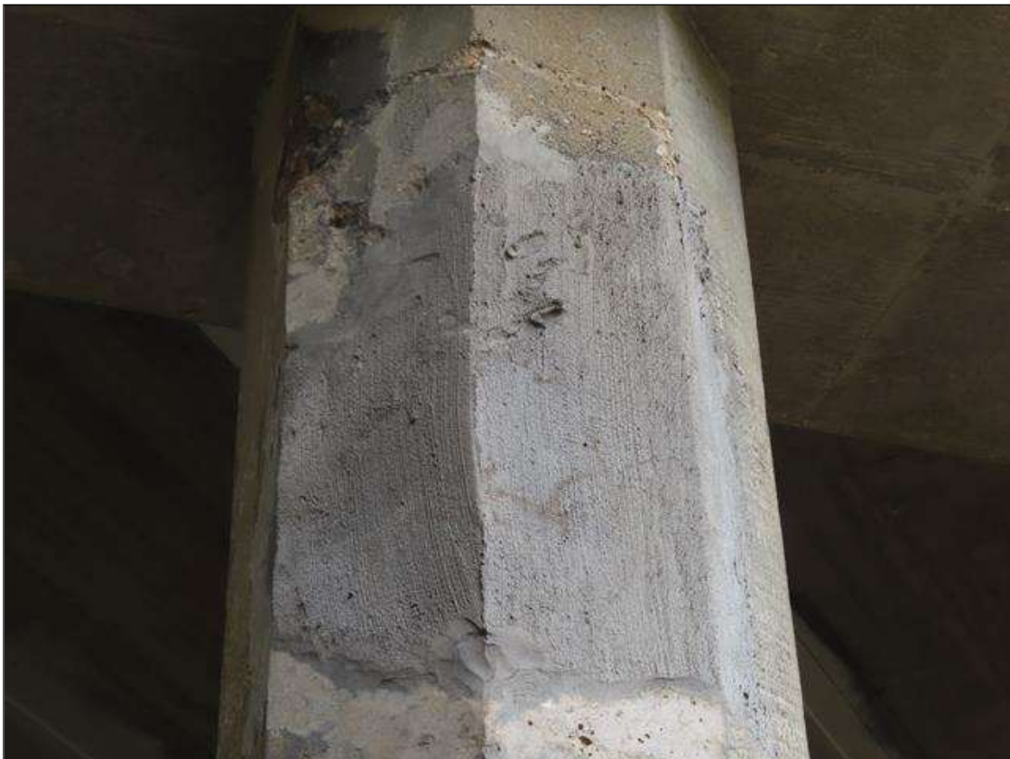
Bent 2 Pile 6: 2 FEET PATCHING
