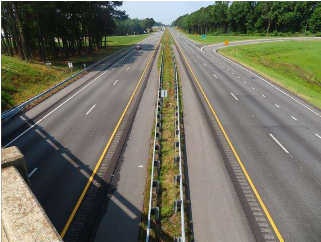
LOOKING SOUTH INTERSTATE 95
