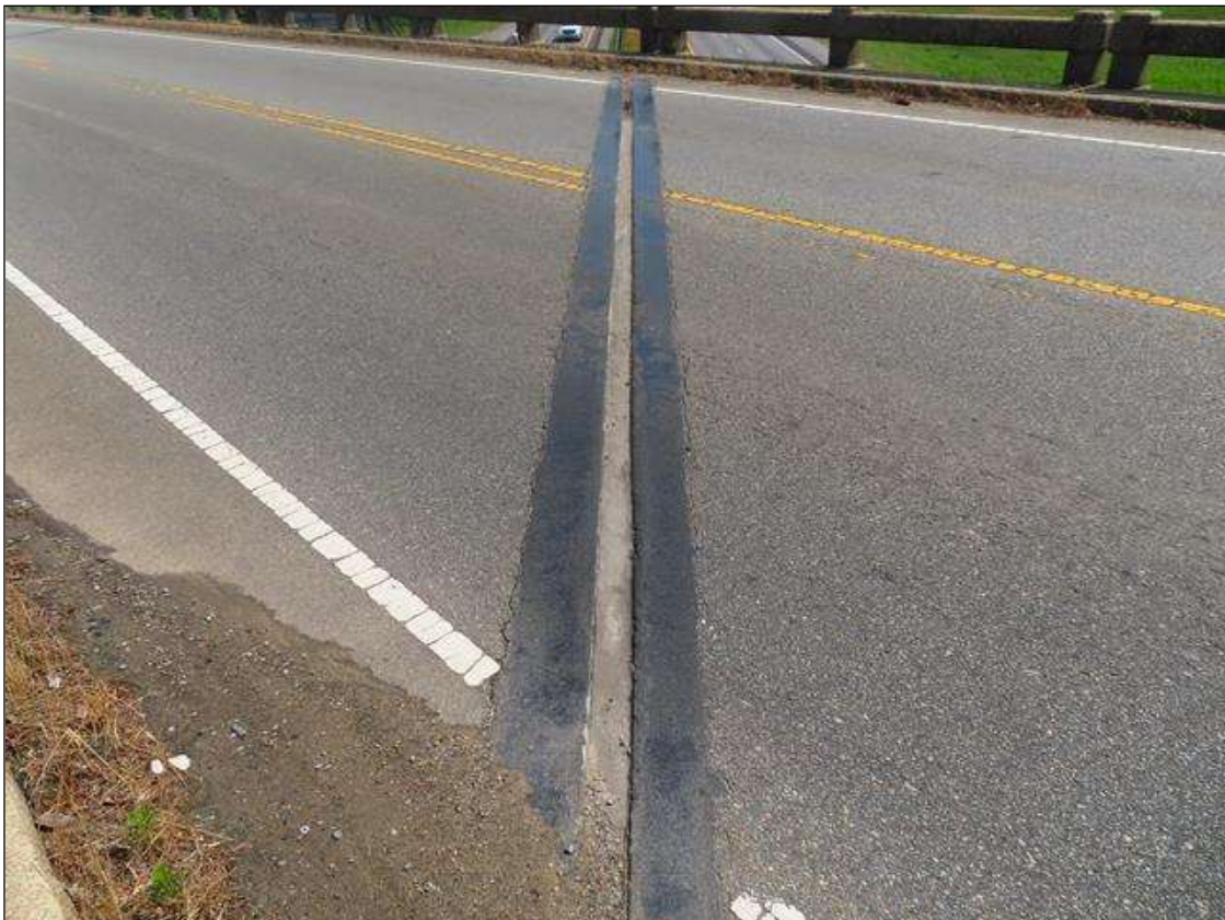
JOINT OVER BENT 2
