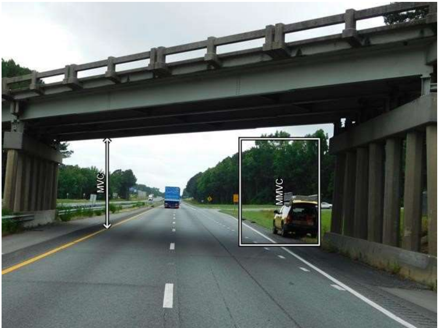
LOOKING SOUTH THROUGH SPAN 3
