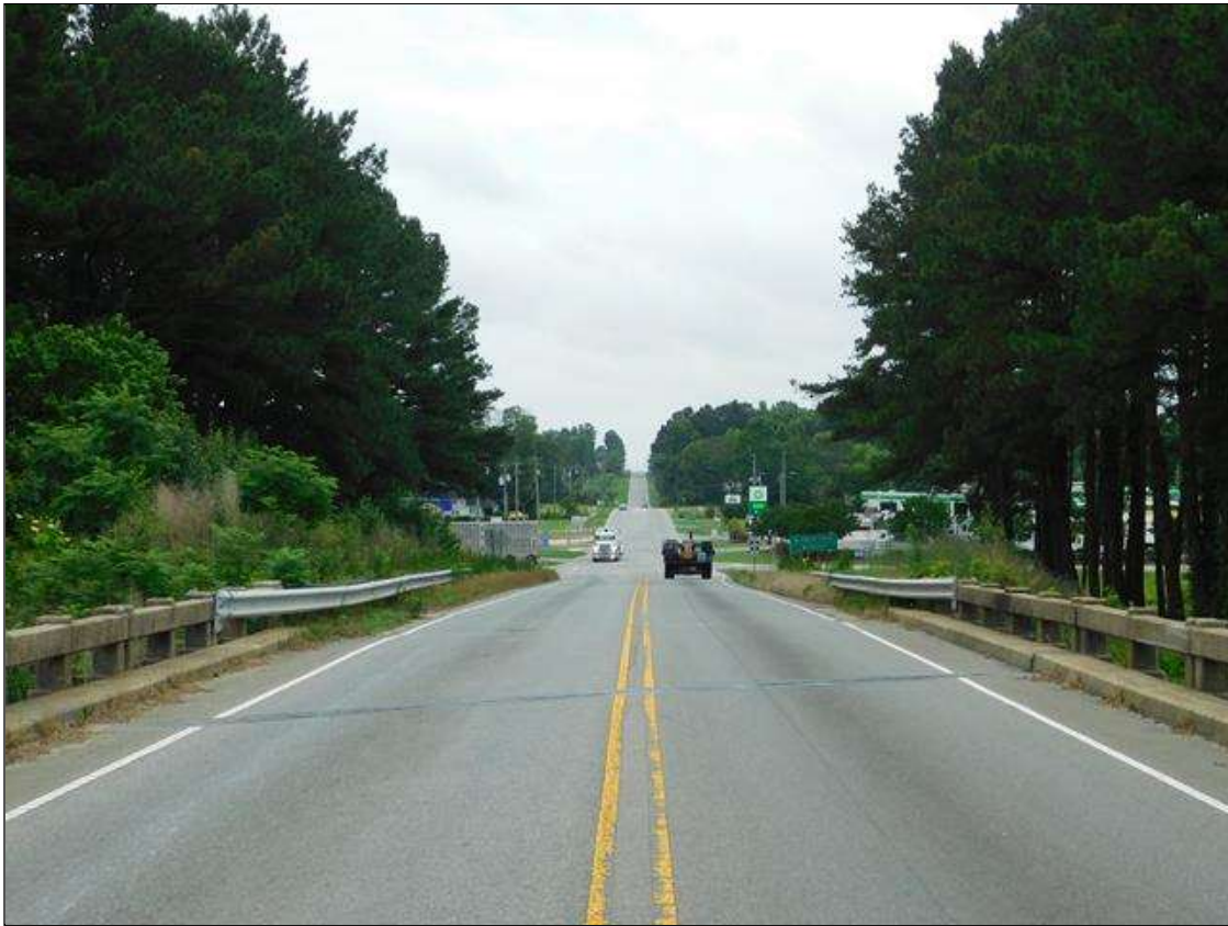
LOOKING AT SOUTH APPROACH
