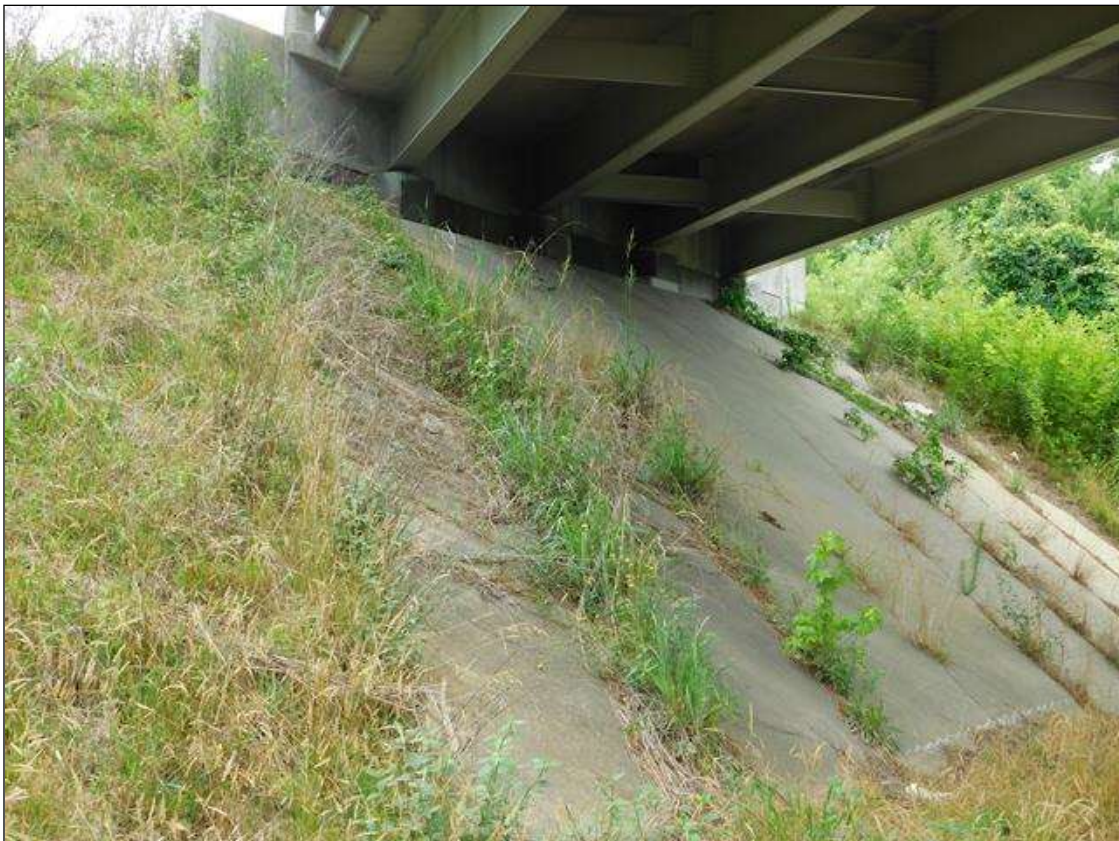
END BENT 2 AND SLOPE PROTECTION
