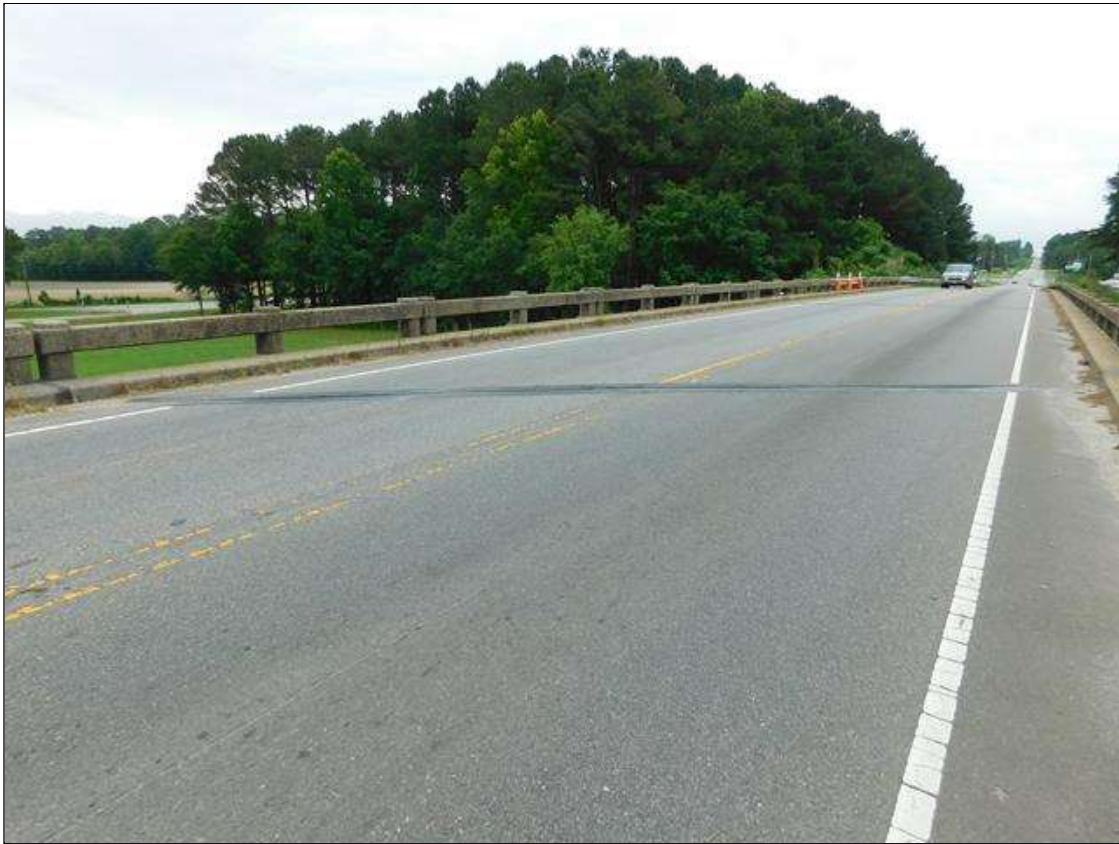
ASPHALT WEARING SURFACE OVERVIEW
