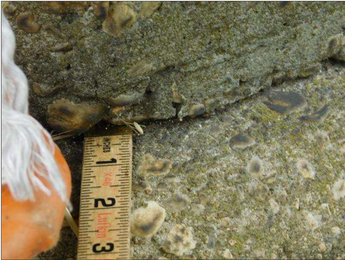
Span 2 Right Bridge Rail: IMPACT DAMAGE. THE 4TH GUARDRAIL POST FROM BENT 1 IS CRACKED, SPALLED AND LEANING OUT 1.5" AT TOP (REFERENCED FROM POST 3). HORIZONTAL RAILING FROM POST 4 TO POST 5 IS CRACKED AND PUSHED OUT. POSTS 5 & 6 HAVE WRAP-AROUND CRACKING AT BOTTOM OF POSTS BUT APPEAR TO BE PLUMB. TEMPORARY STEEL GUARDRAIL HAS BEEN ADDED FROM POST 3 TO POST 7. AFFECTED AREA IS OVER THE NORTHBOUND LANES OF I-95. PAR ISSUED.
