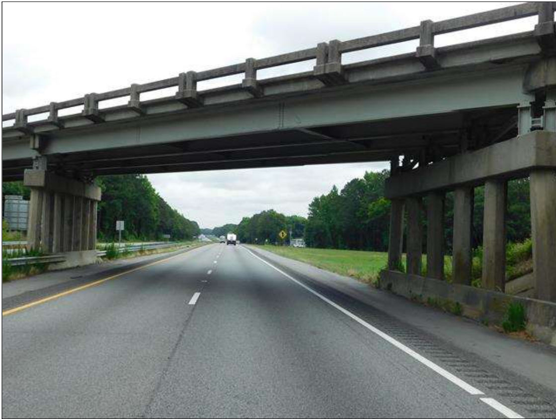
LOOKING NORTH THROUGH SPAN 2
