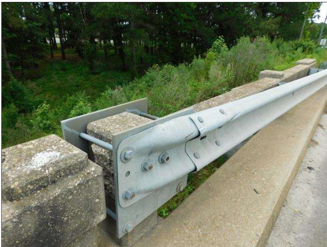
APPROACH GUARDRAIL CONNECTION
