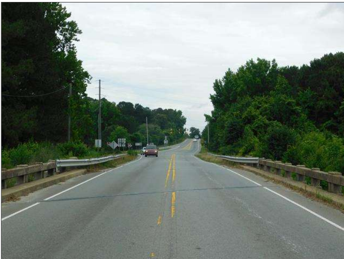
LOOKING AT NORTH APPROACH
