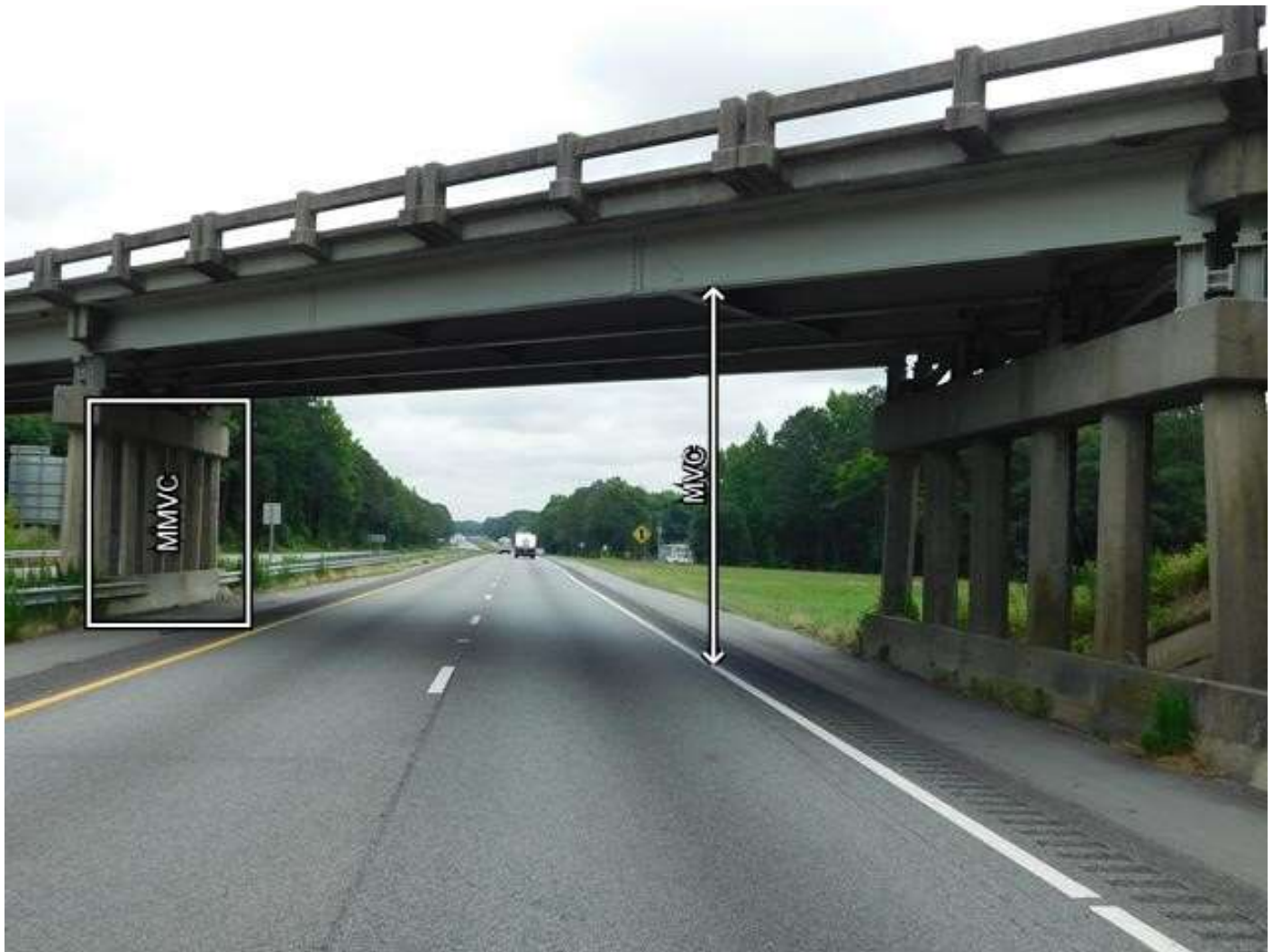
LOOKING NORTH THROUGH SPAN 2
