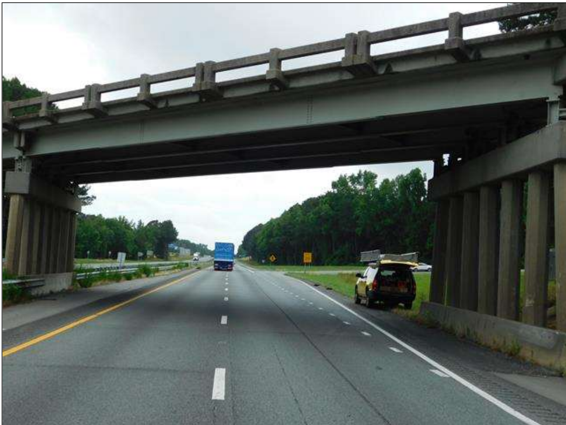
LOOKING SOUTH THROUGH SPAN 3
