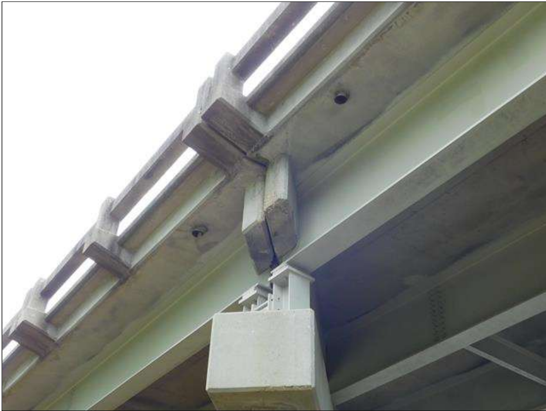
SUPERSTRUCTURE OVER END OF CAP
