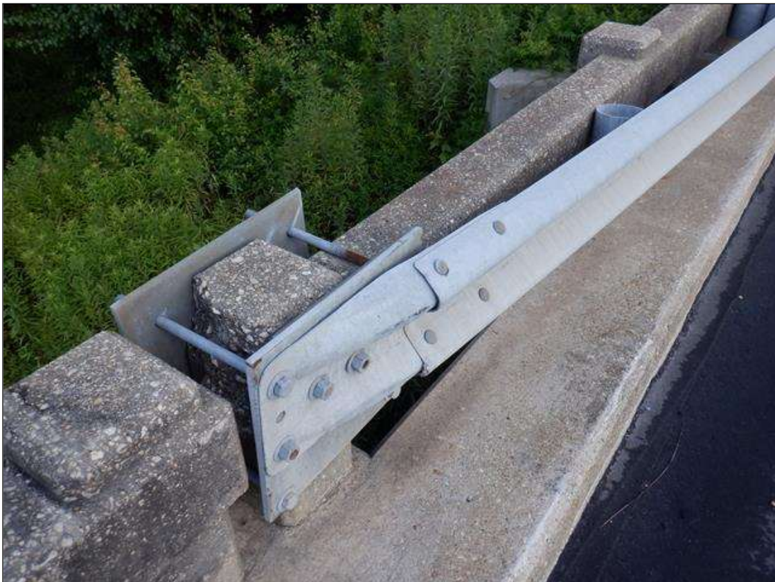
SOUTHEAST GUARDRAIL ATTACHMENT
