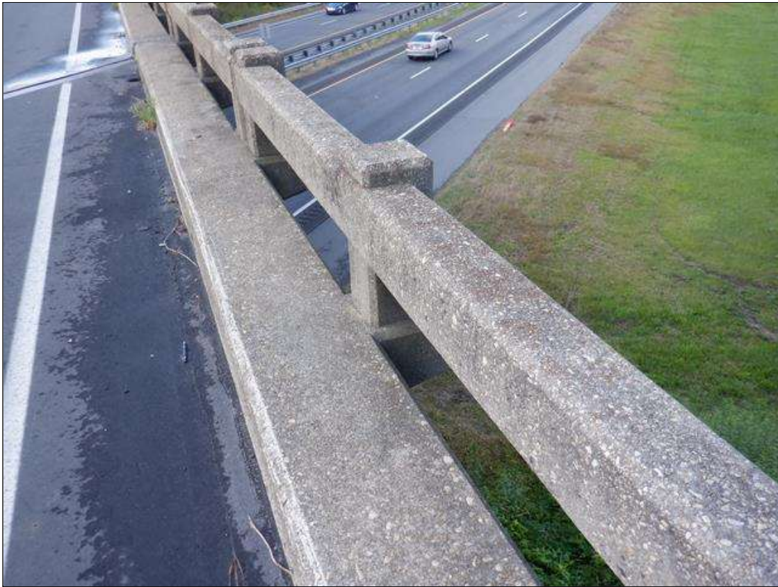
RIGHT BRIDGE RAIL
