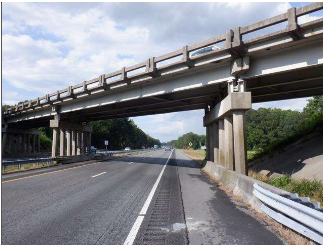
SPAN 2 VERTICAL CLEARANCE
