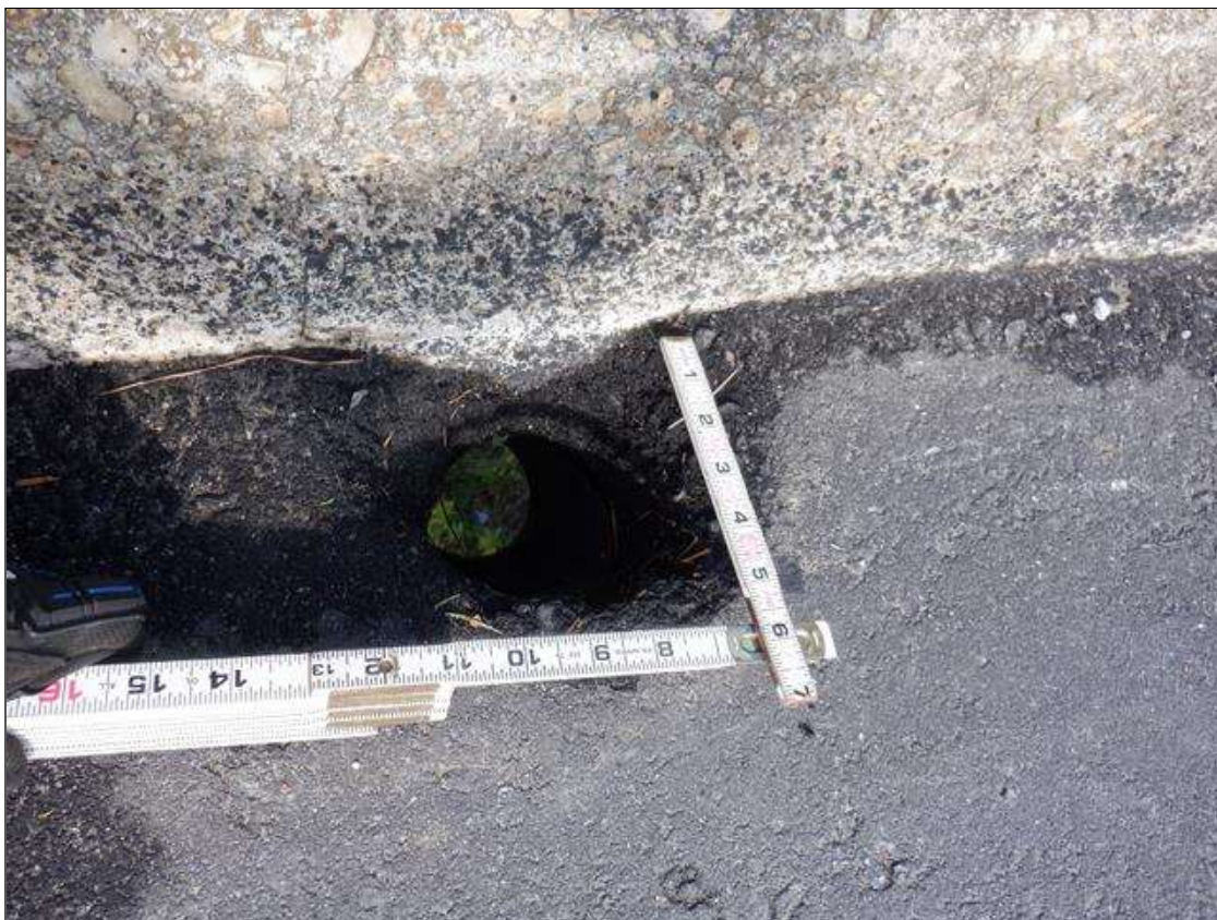
SPAN 1 ALONG RIGHT BRIDGE RAIL 4 INCH DIAMETER SCUPPER
