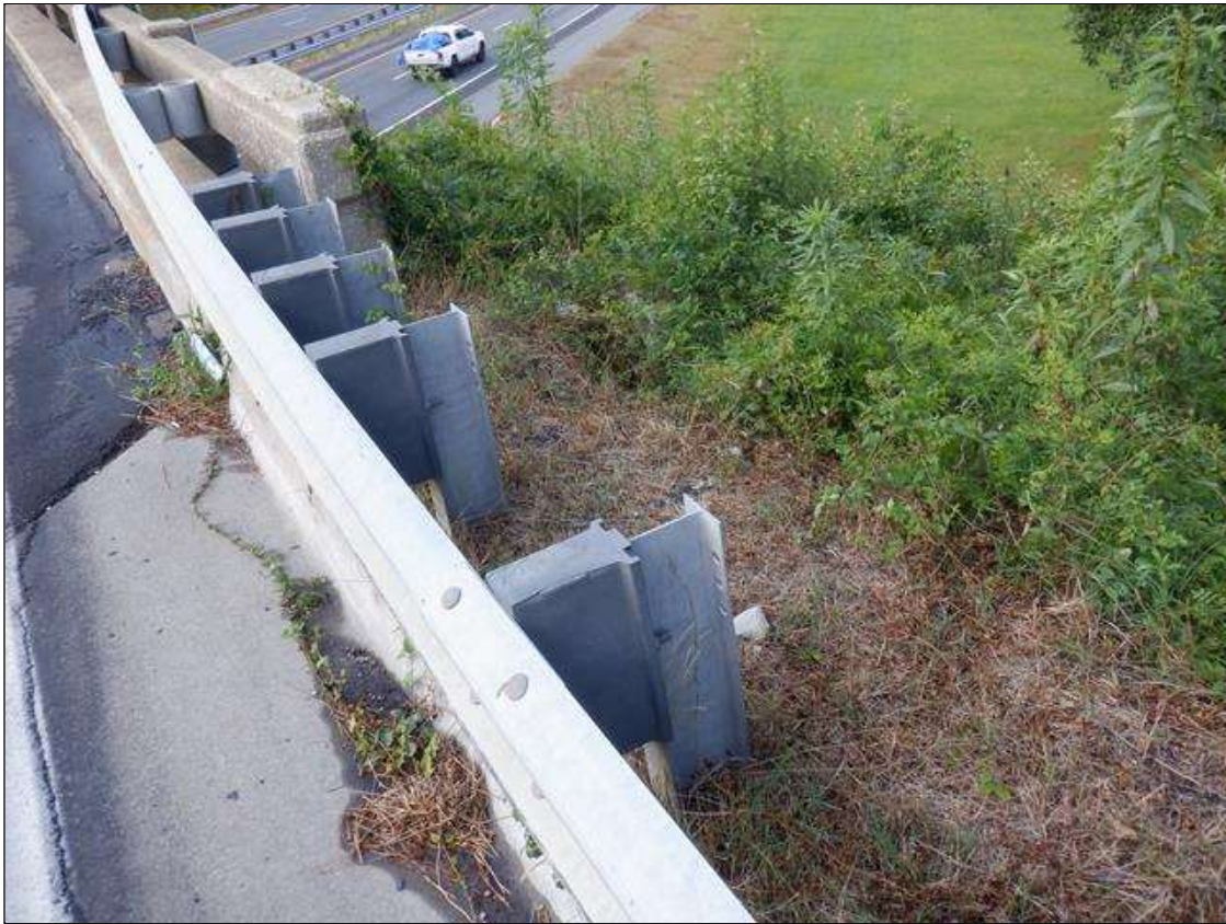
SOUTHEAST GUARDRAIL TRANSITION
