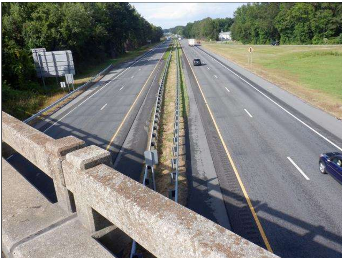
LOOKING EAST FROM BRIDGE
