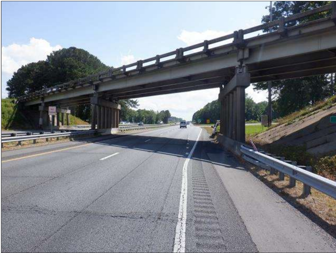
SPAN 3 VERTICAL CLEARANCE SOUTHBOUND LANES
