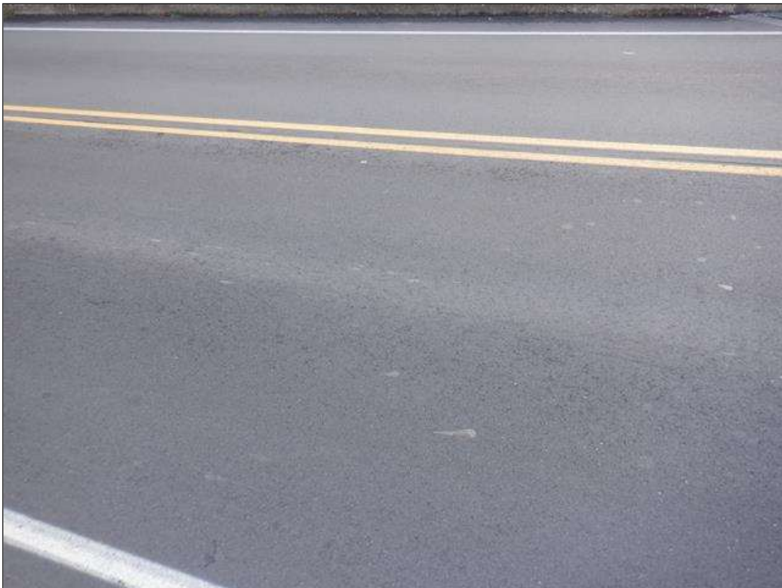
SPAN 1 WEARING SURFACE (REPLACED, BUT NO CHANGE IN THICKNESS)
