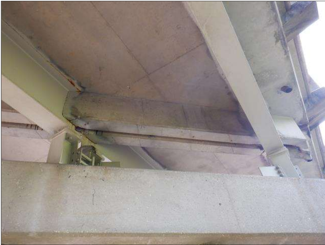
SPAN 1 BAY 3 FAR END DIAPHRAGM
