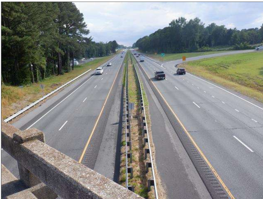
LOOKING WEST FROM BRIDGE
