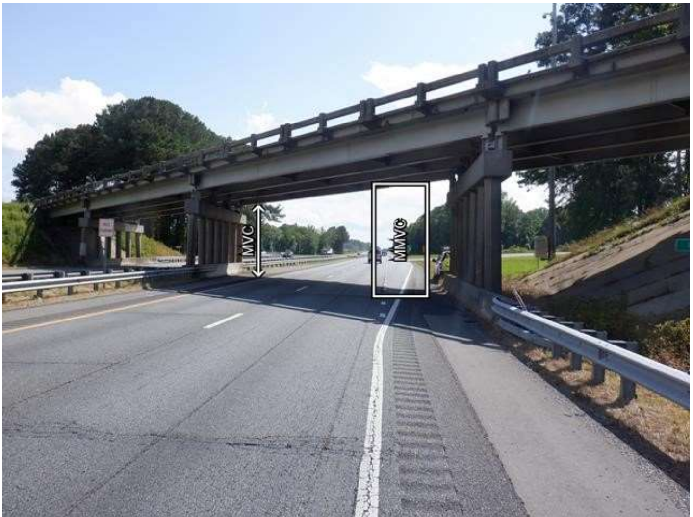
SPAN 3 VERTICAL CLEARANCE SOUTHBOUND LANES - MEASURED AT BEAM 1, REQUEST LIDAR
