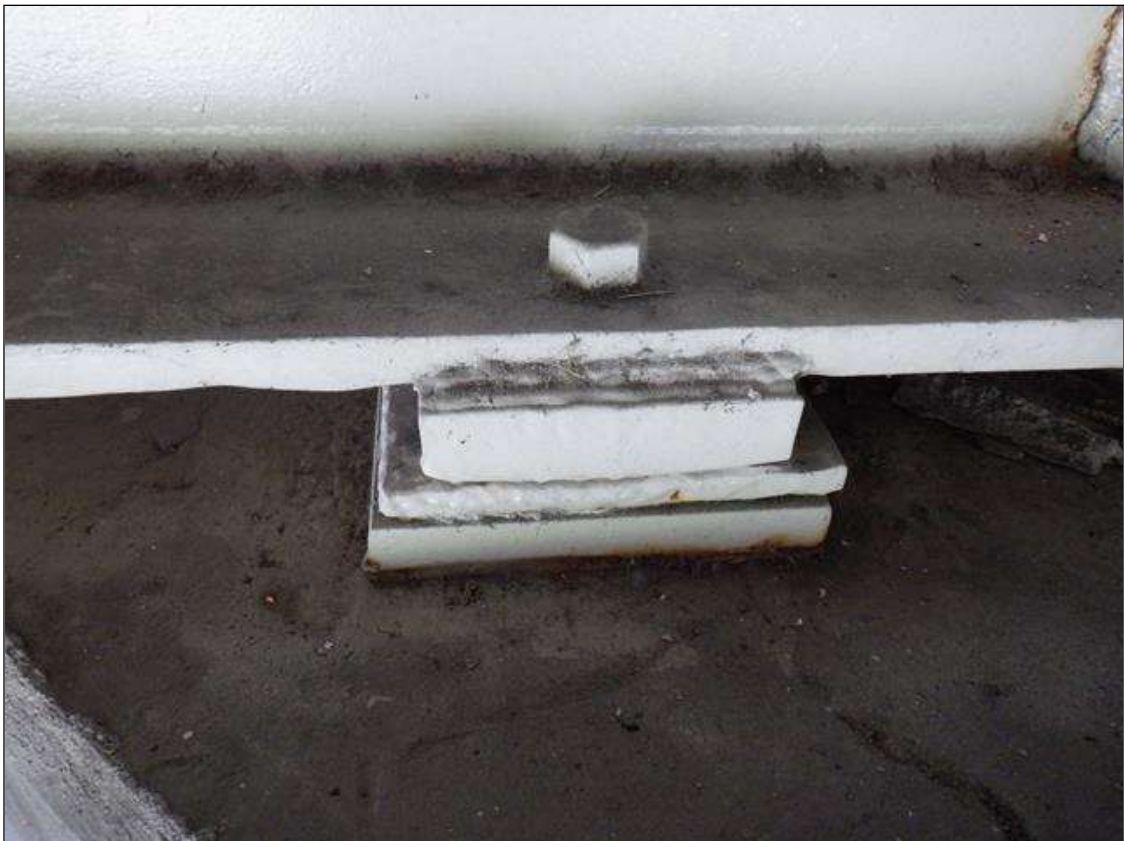
SPAN 4 BEAM 3 FAR BEARING
