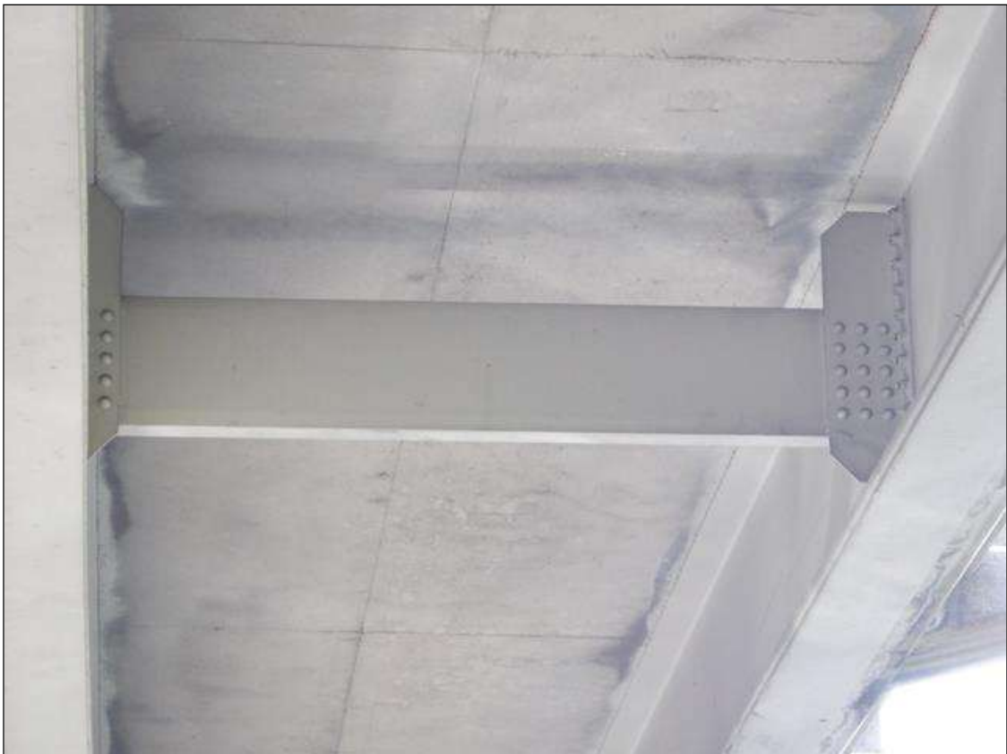
SPAN 2 BAY 3 INTERMEDIATE DIAPHRAGM
