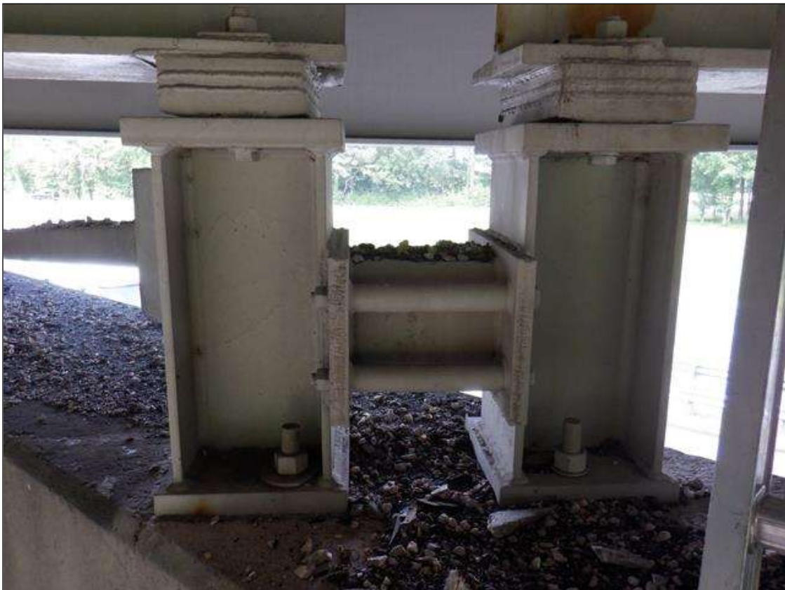
BEAM 3 BENT 3 BEARINGS
