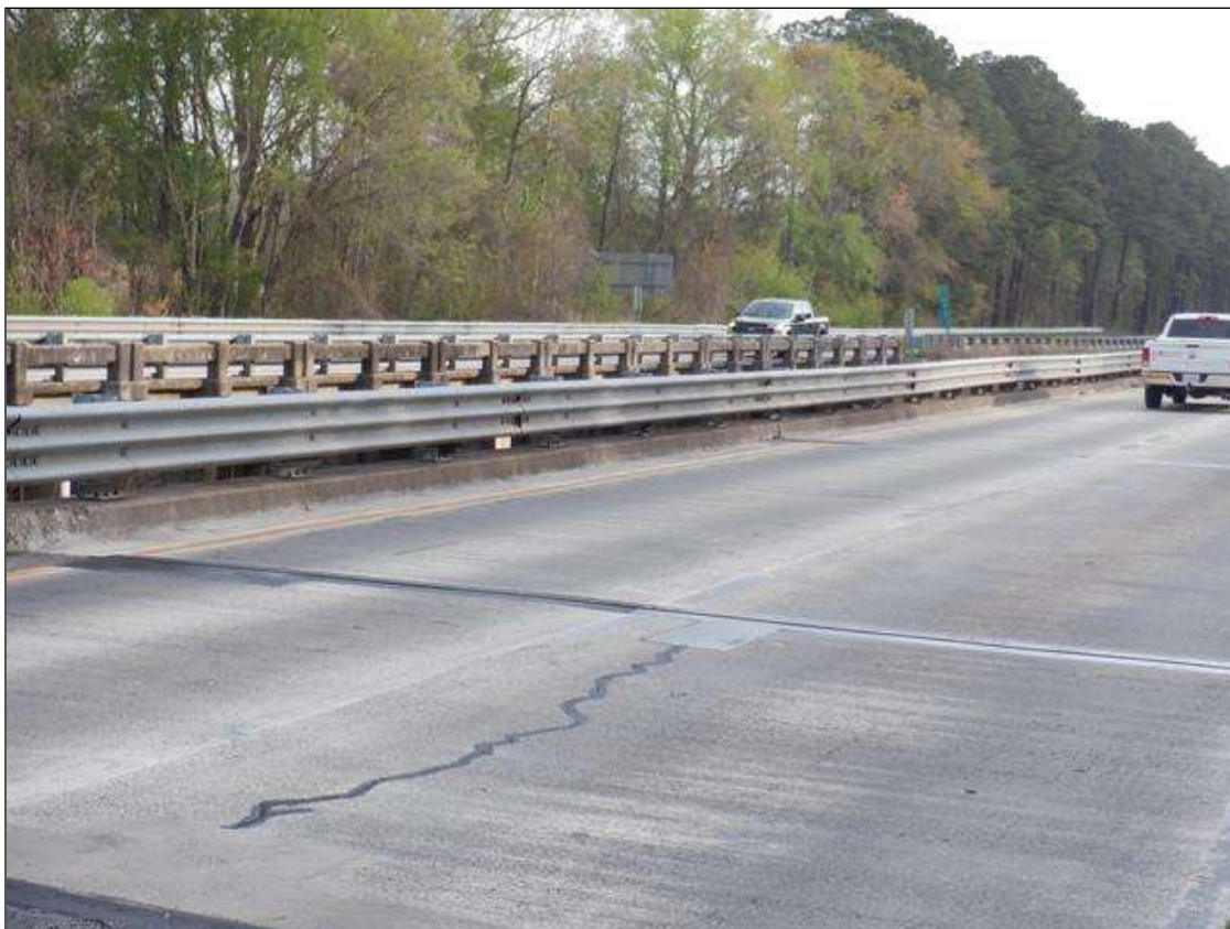
WEST BRIDGE RAIL
