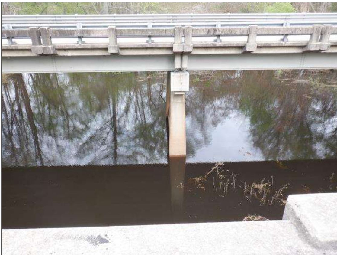
UPSTREAM VIEW FROM BRIDGE LOOKING WEST
