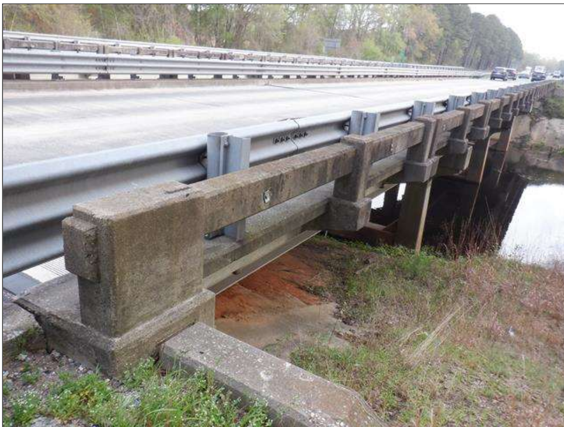
EAST BRIDGE RAIL
