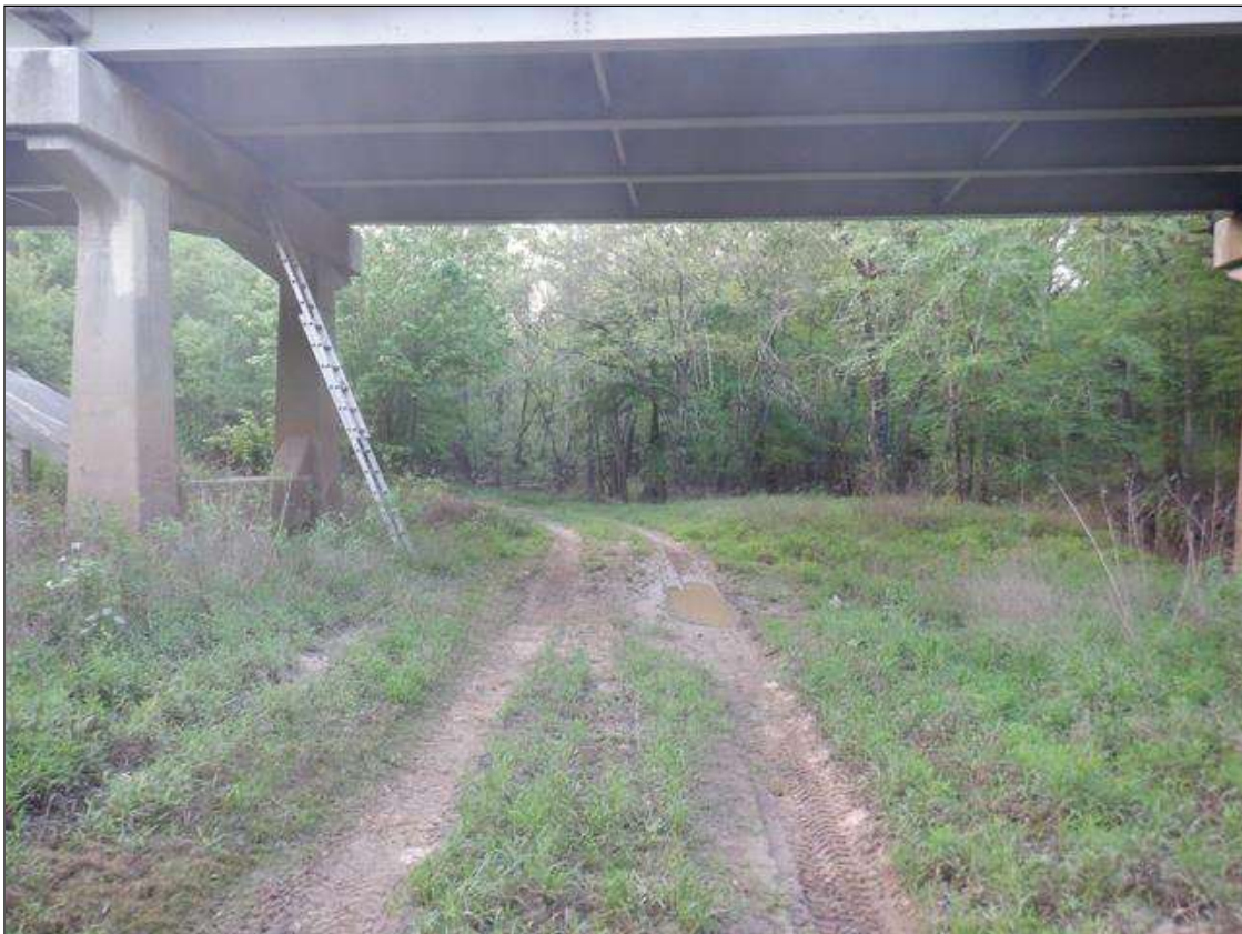
SPAN 3 CLEARANCE OPENING, GREENWAY, LOOKING EAST
