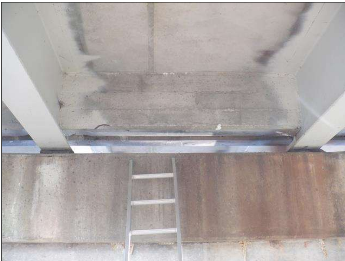
BENT 1 BAY 2 DIAPHRAGM LOOKING NORTH (OTHERS SIMILAR)
