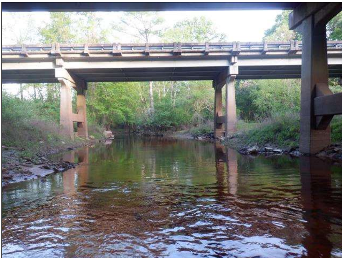
UPSTREAM VIEW LOOKING WEST
