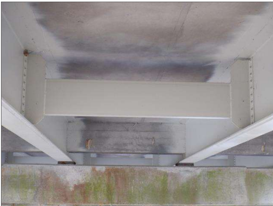
SPAN 4 BAY 2 INTERMEDIATE DIAPHRAGM LOOKING SOUTH (OTHERS SIMILAR)
