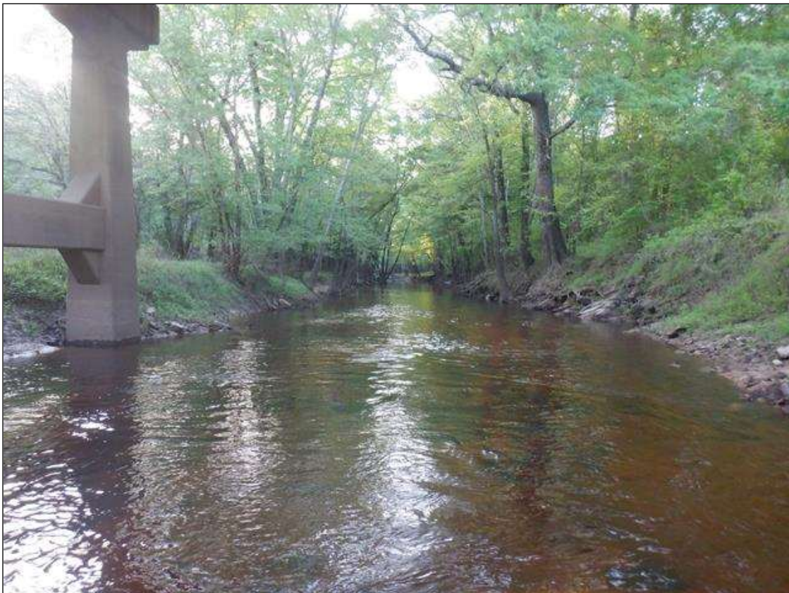
DOWNSTREAM VIEW LOOKING EAST
