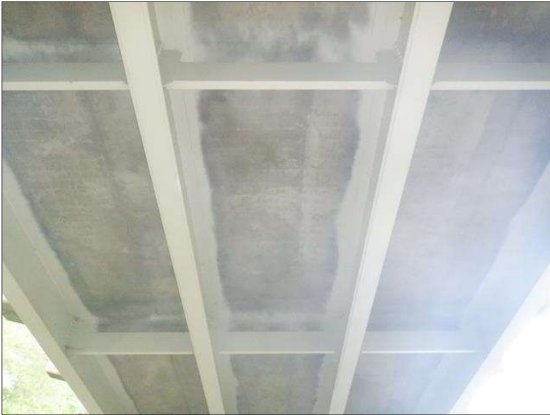
SPAN 3 SUPERSTRUCTURE UNDERSIDE LOOKING SOUTH
