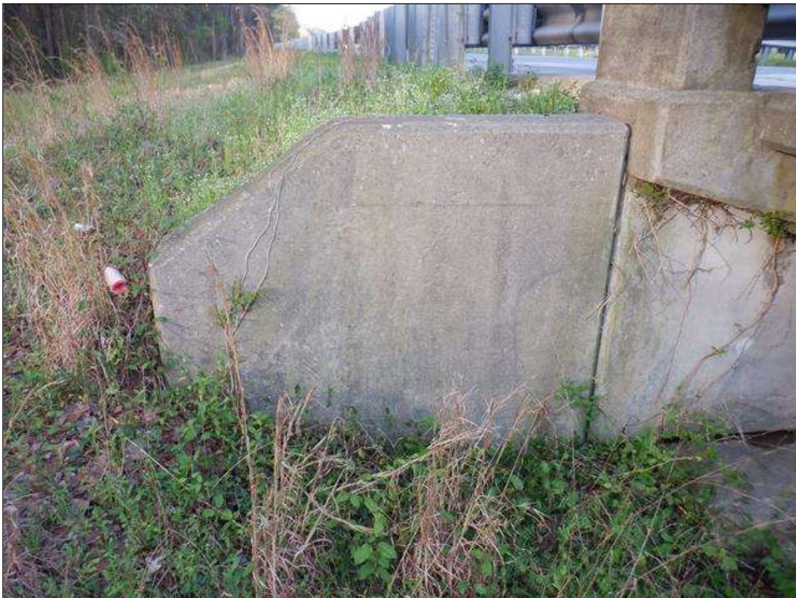
SOUTHEAST WINGWALL (OTHERS SIMILAR)
