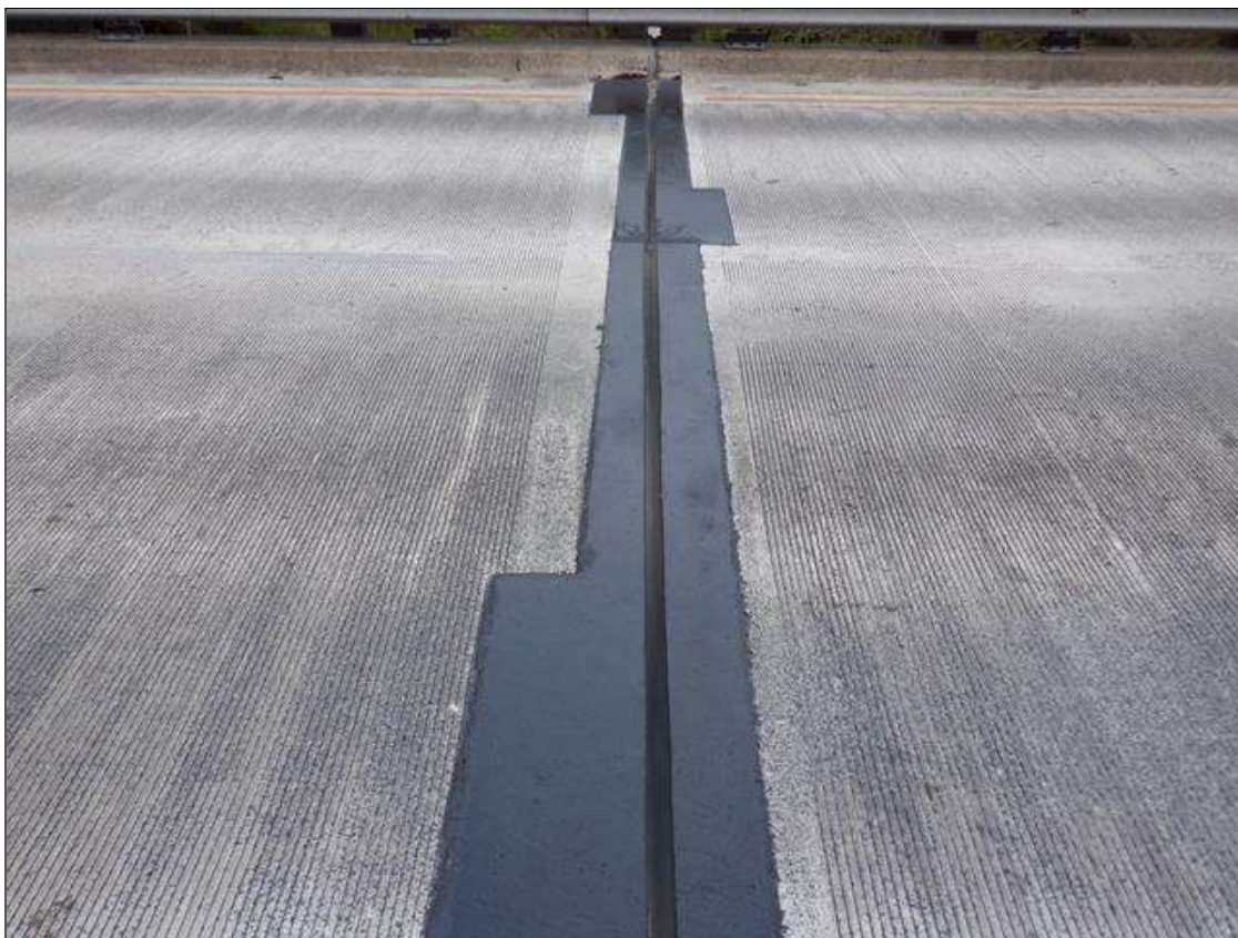
JOINT OVER BENT 1 LOOKING WEST
