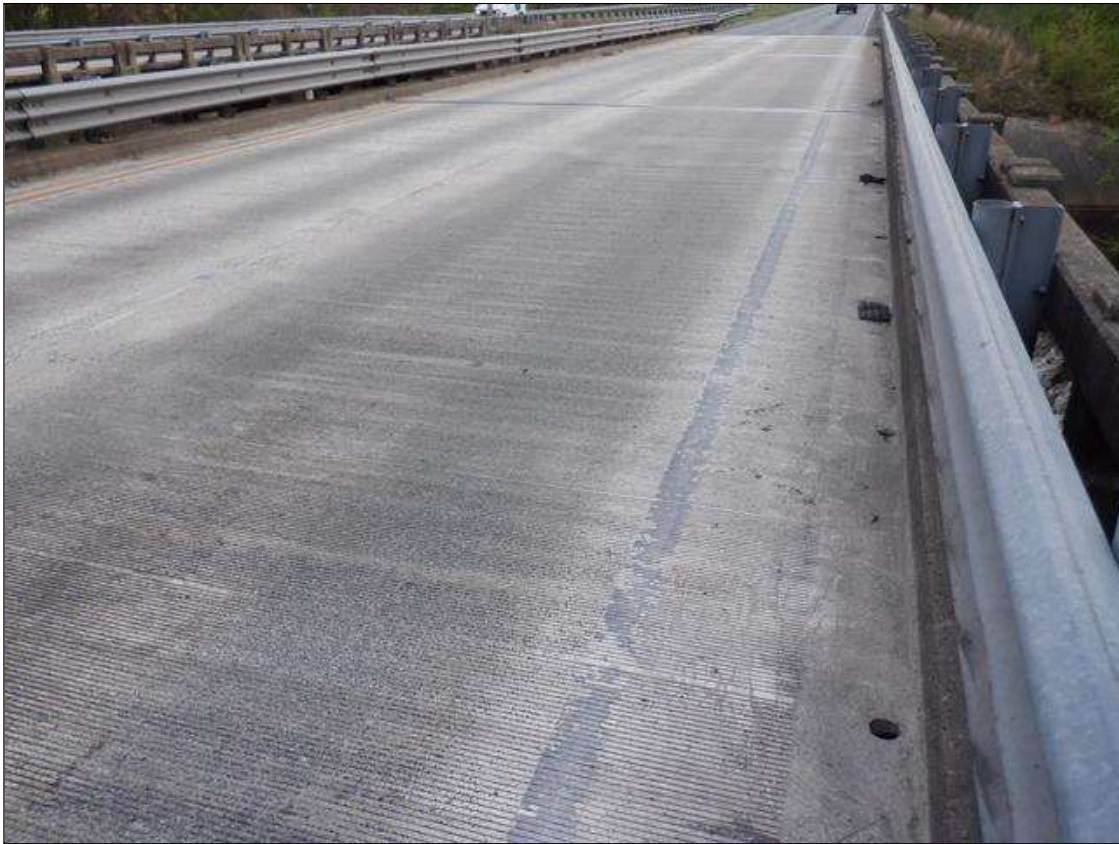
SPAN 2 CONCRETE WEARING SURFACE LOOKING NORTH
