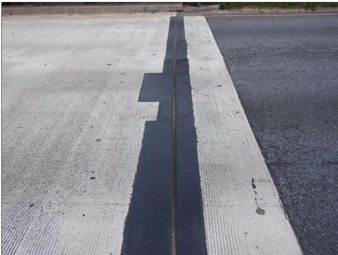
JOINT OVER END BENT 2 LOOKING WEST
