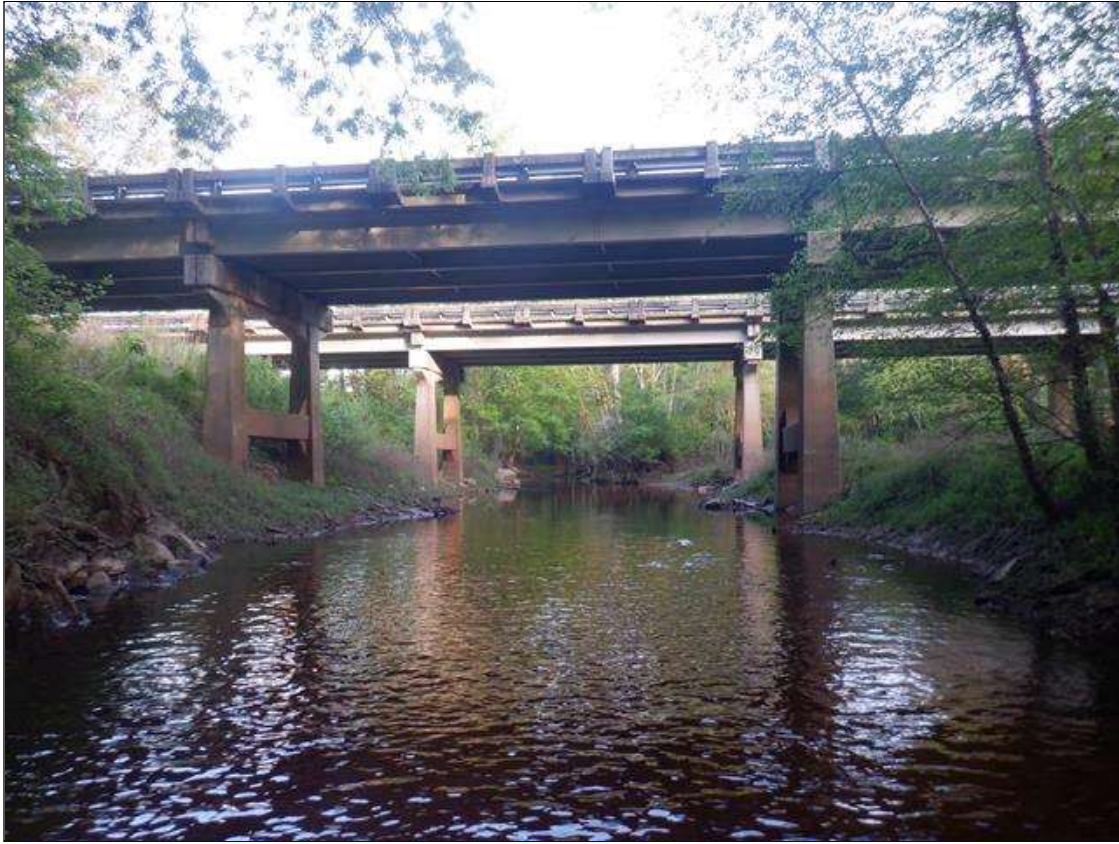
SPAN 2 WATERWAY OPENING LOOKING WEST
