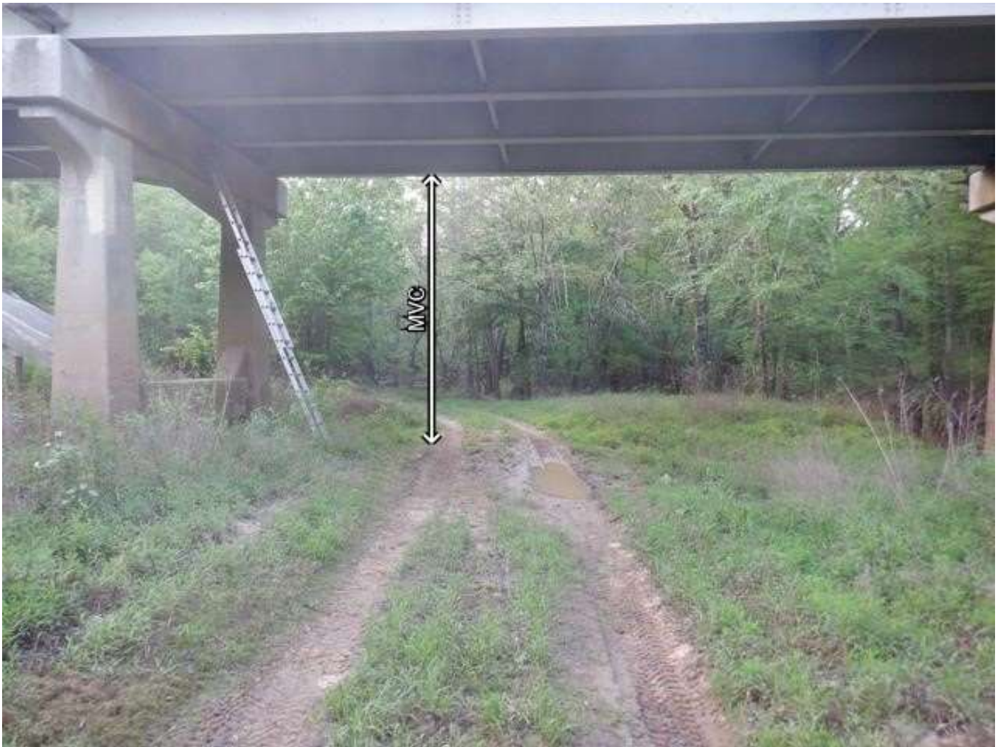
SPAN 3 CLEARANCE OPENING, GREENWAY, LOOKING EAST
