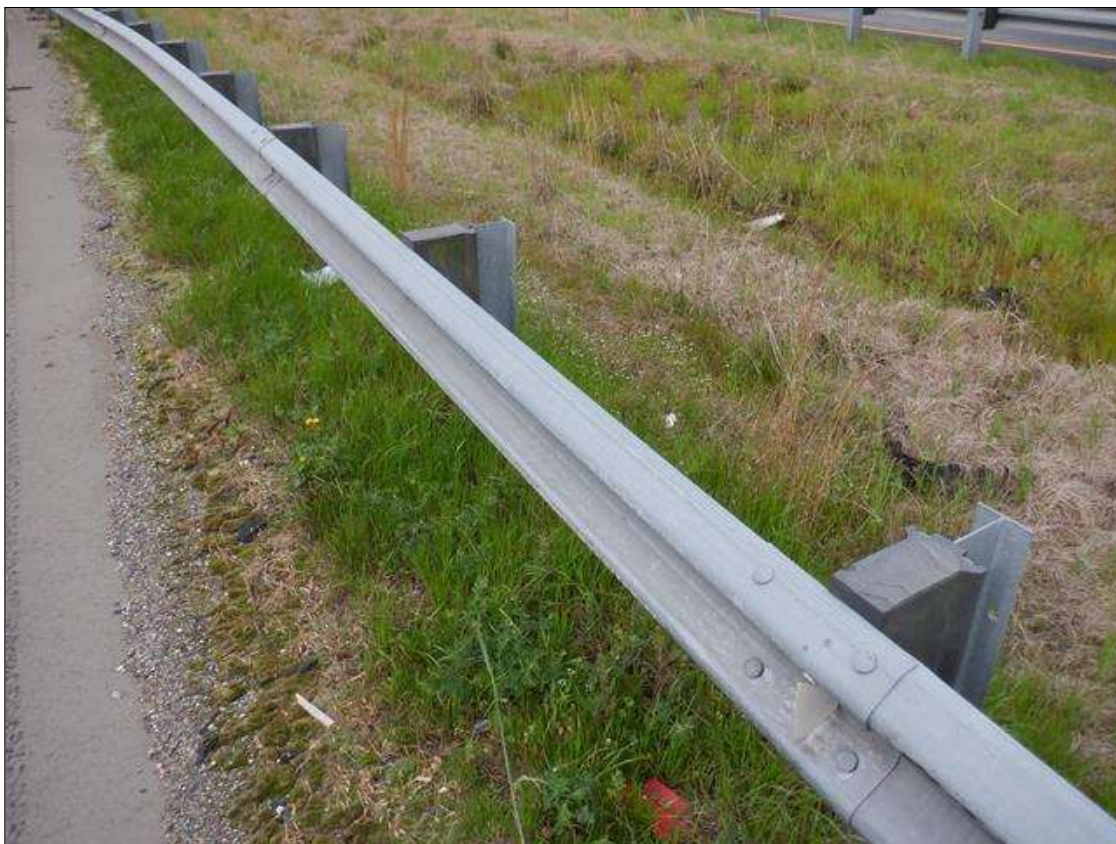
NORTHWEST TYPICAL GUARDRAIL POST SPACING 75 INCHES (OTHERS SIMILAR)
