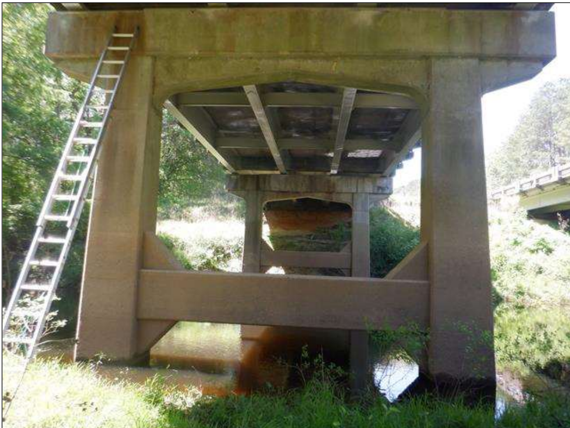
BENT 2 ELEVATION LOOKING SOUTH
