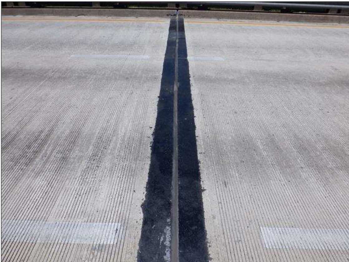
JOINT OVER BENT 3, LOOKING WEST
