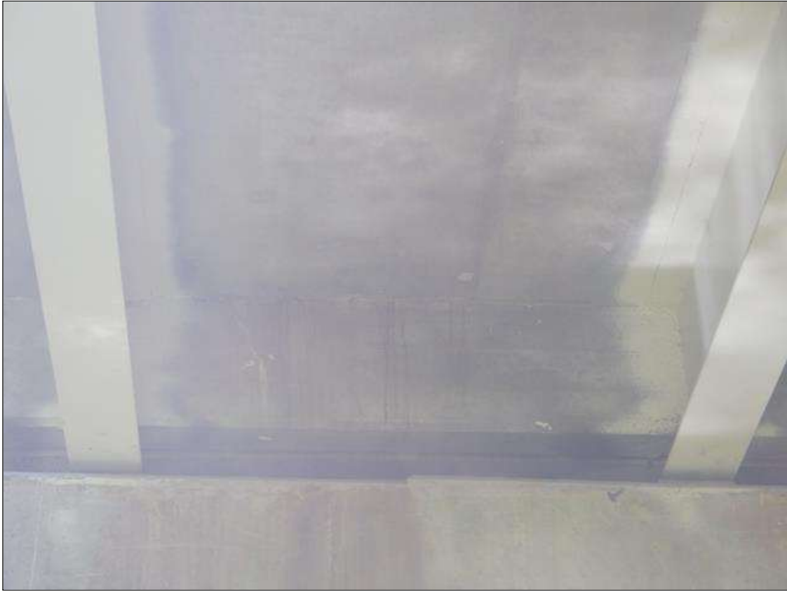
BENT 3 DIAPHRAGM SPAN 3 BAY 3 LOOKING SOUTH (OTHERS SIMILAR)
