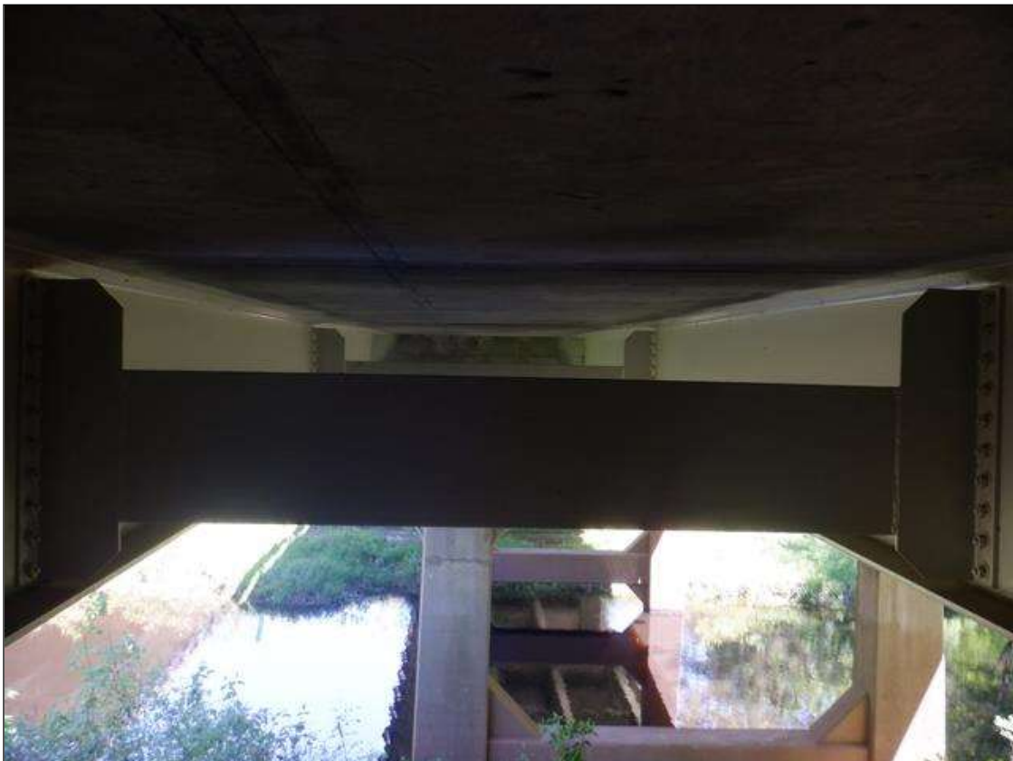
INTERMEDIATE DIAPHRAGM SPAN 1 BAY 1 LOOKING NORTH
