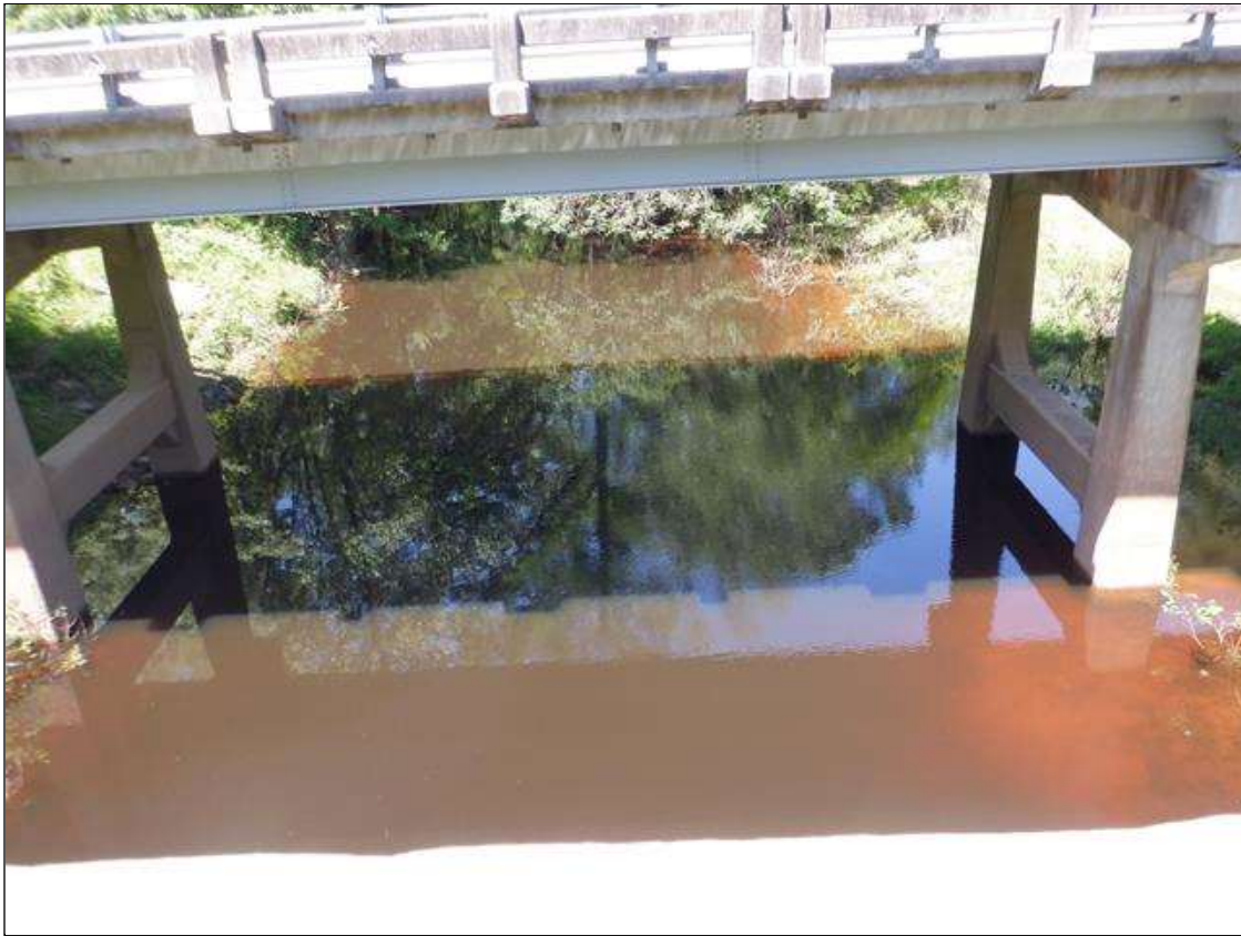
UPSTREAM VIEW FROM BRIDGE, LOOKING WEST
