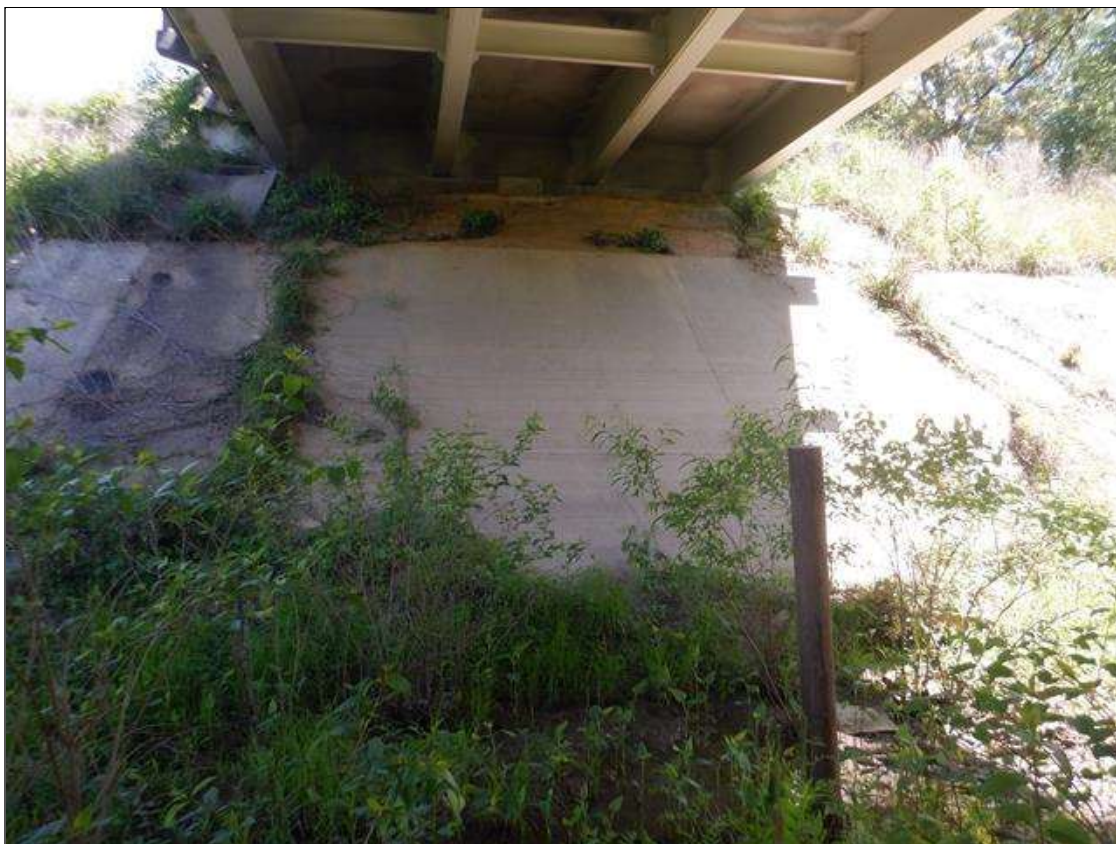
END BENT 2 SLOPE PROTECTION
