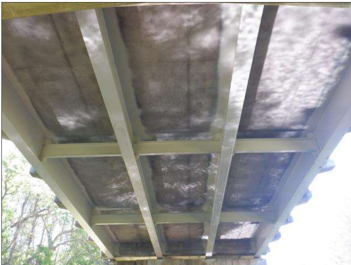
SUPERSTRUCTURE UNDERSIDE SPAN 2 LOOKING SOUTH
