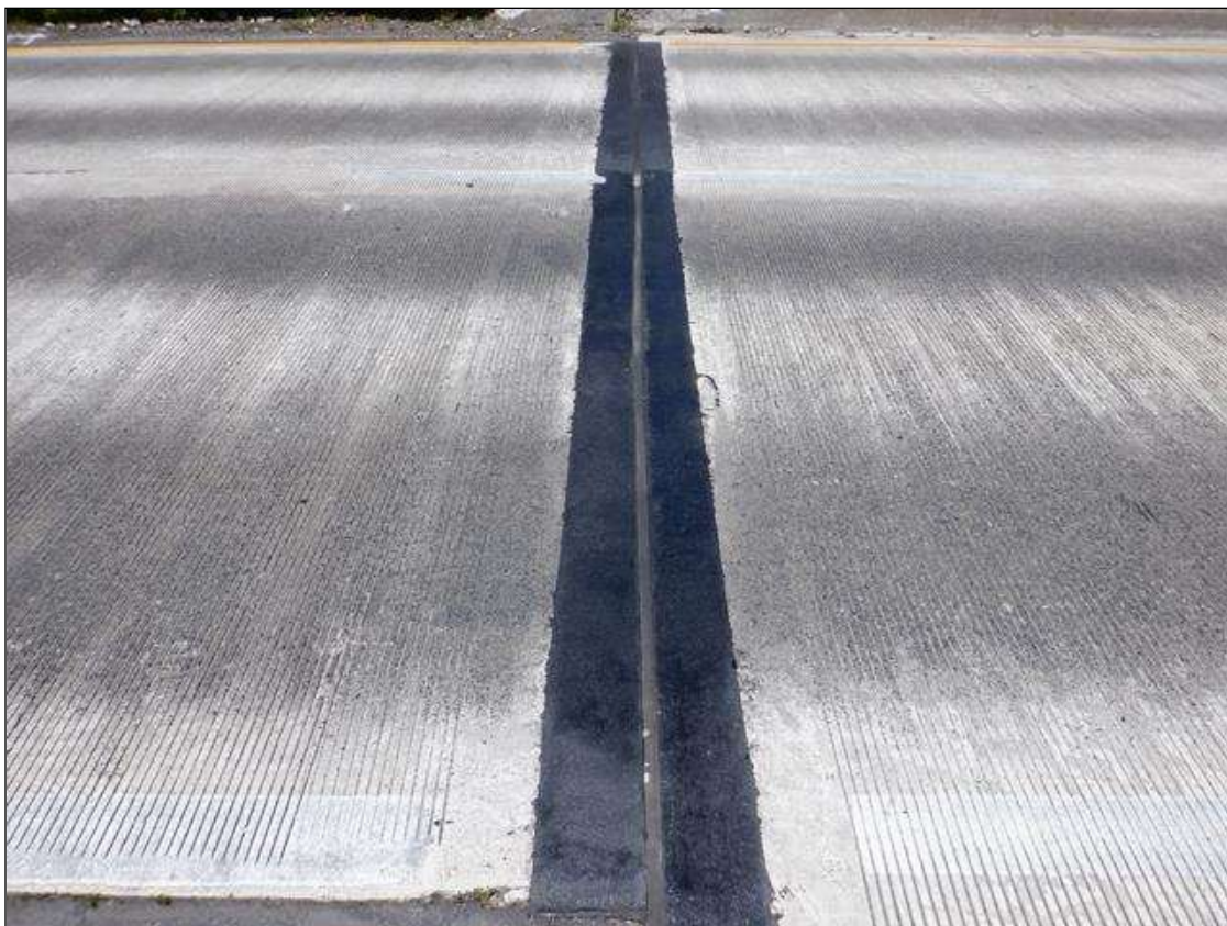
JOINT OVER END BENT 1, LOOKING WEST
