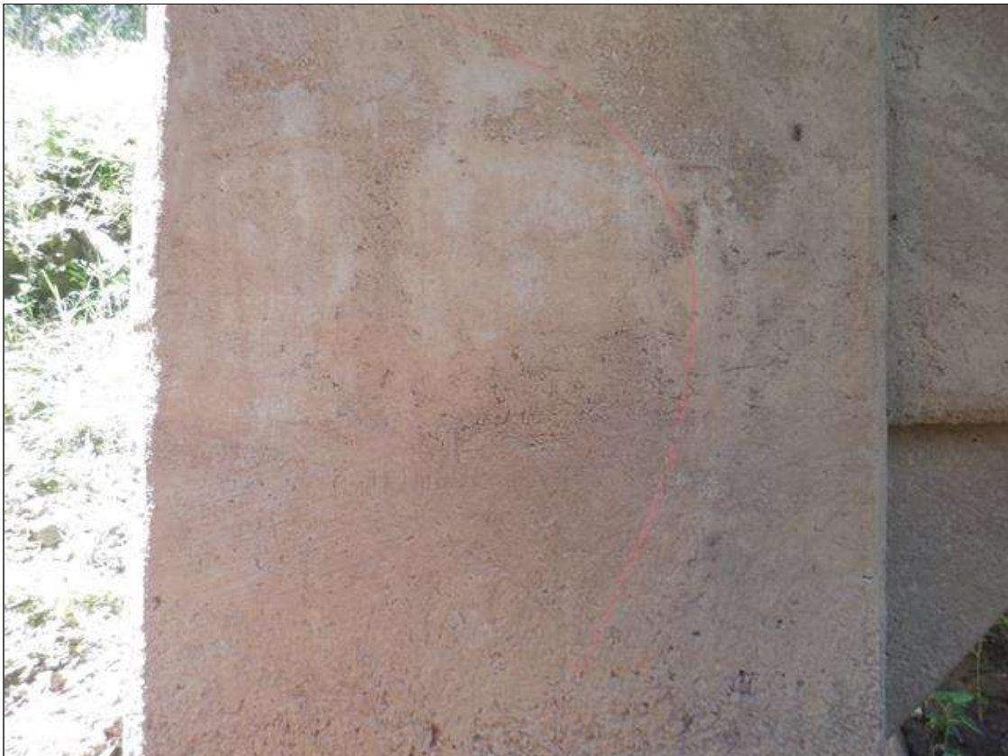
Bent 1 Pile 2: 2' diameter area of sound patch on Span 2 face, 12' from bottom of cap.
