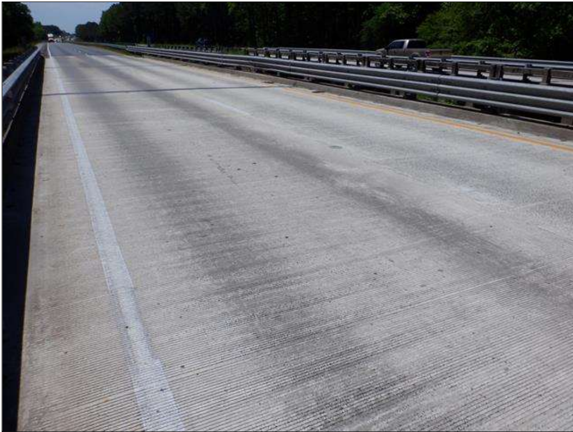
SPAN 3 CONCRETE WEARING SURFACE LOOKING SOUTH
