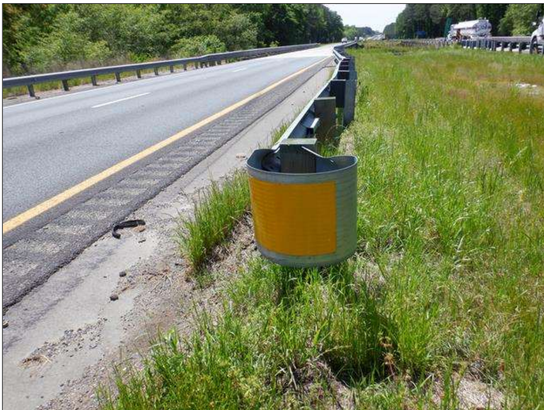
NORTHWEST GUARDRAIL TERMINAL (NORTHEAST SIMILAR)
