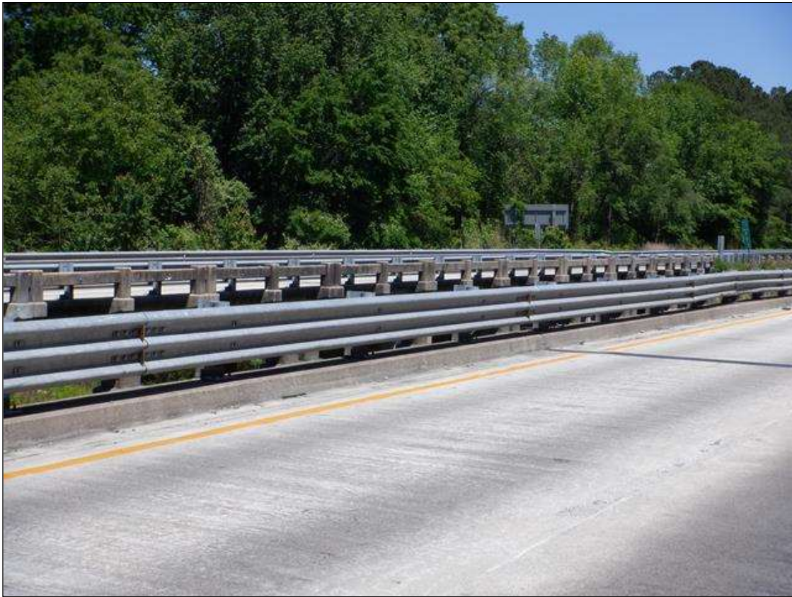
WEST BRIDGE RAIL (EAST SIMILAR)
