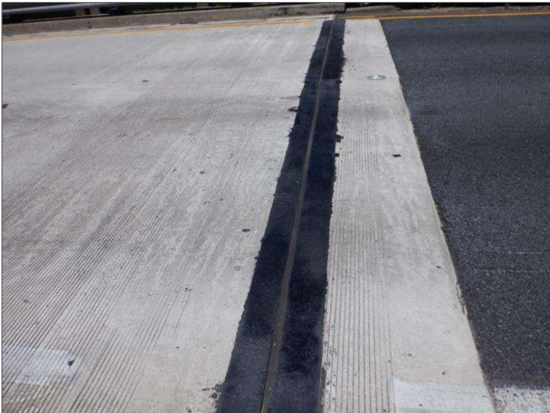
JOINT OVER END BENT 2, LOOKING WEST
