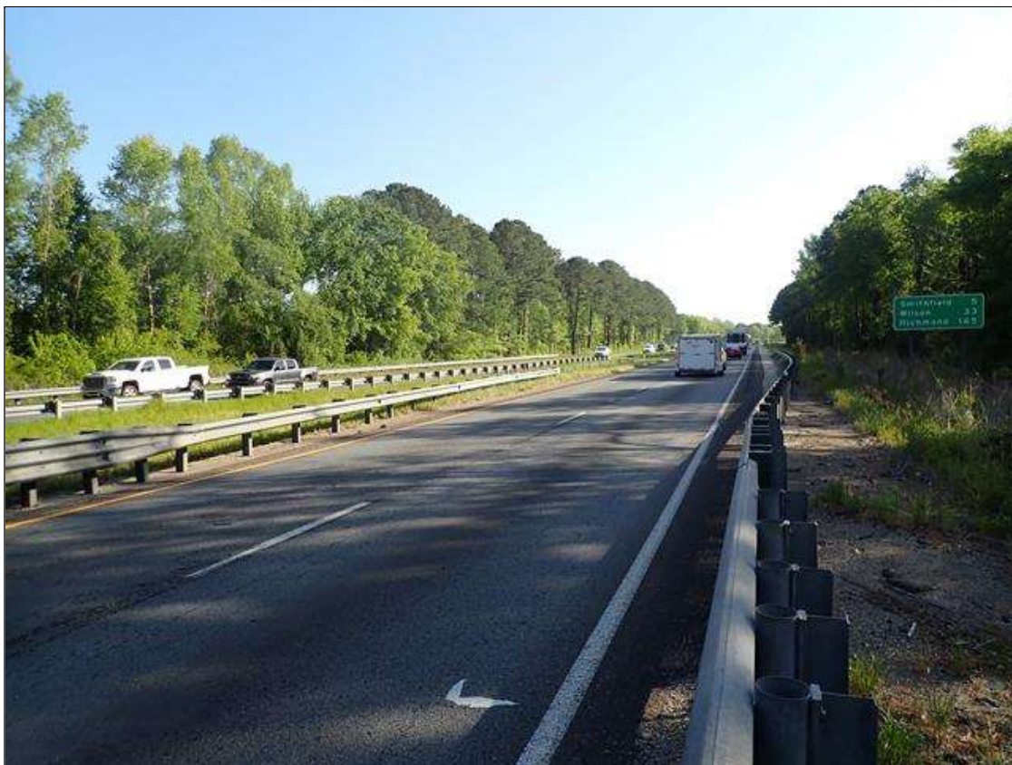
NORTH APPROACH LOOKING NORTH
