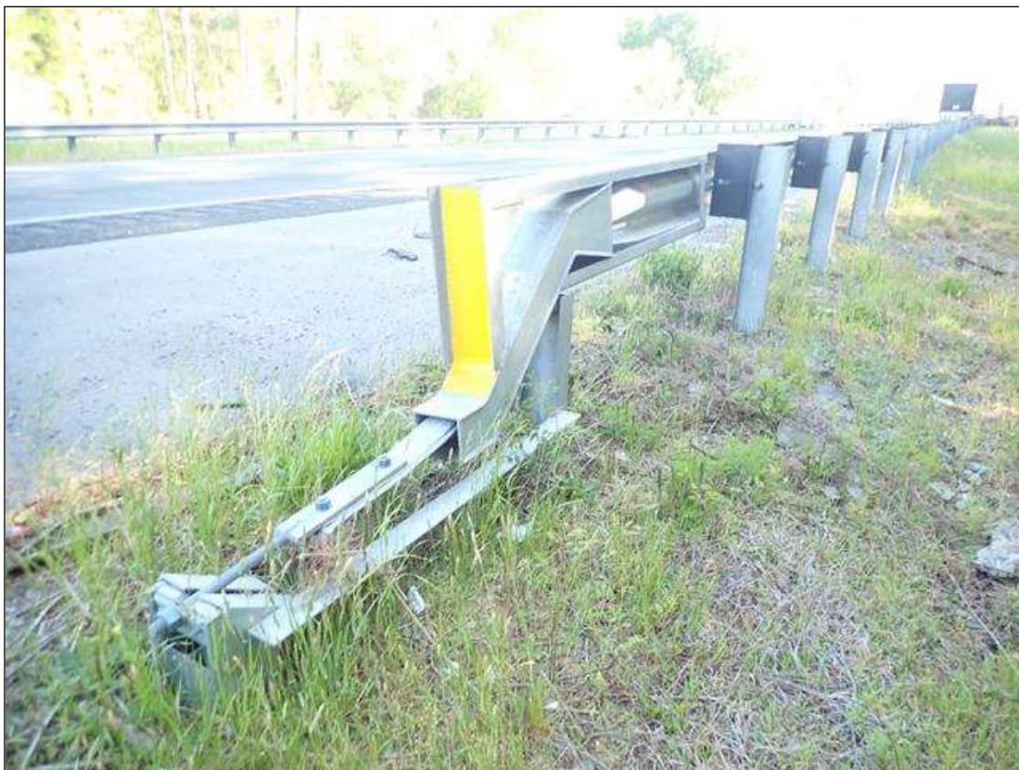
GUARDRAIL TERMINATION (SOUTHEAST CORNER SHOWN)
