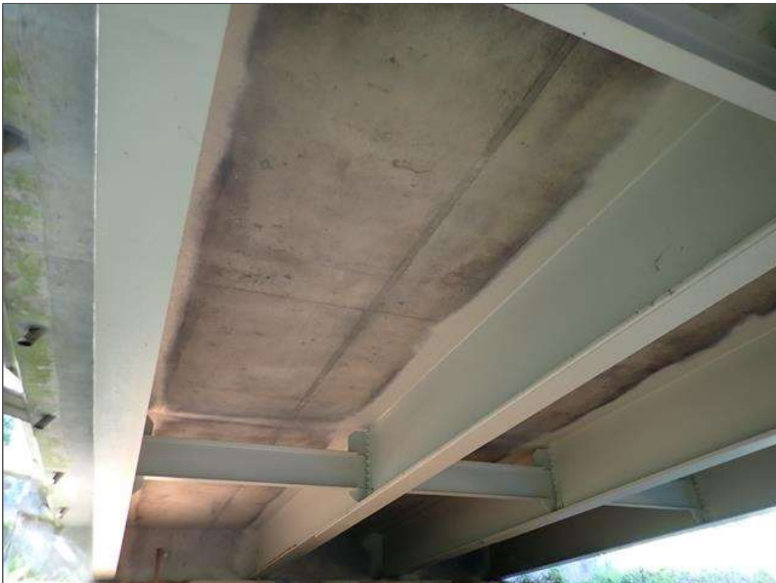
UNDERSIDE OF SUPERSTRUCTURE (SPAN 1, OTHERS SIMILAR)
