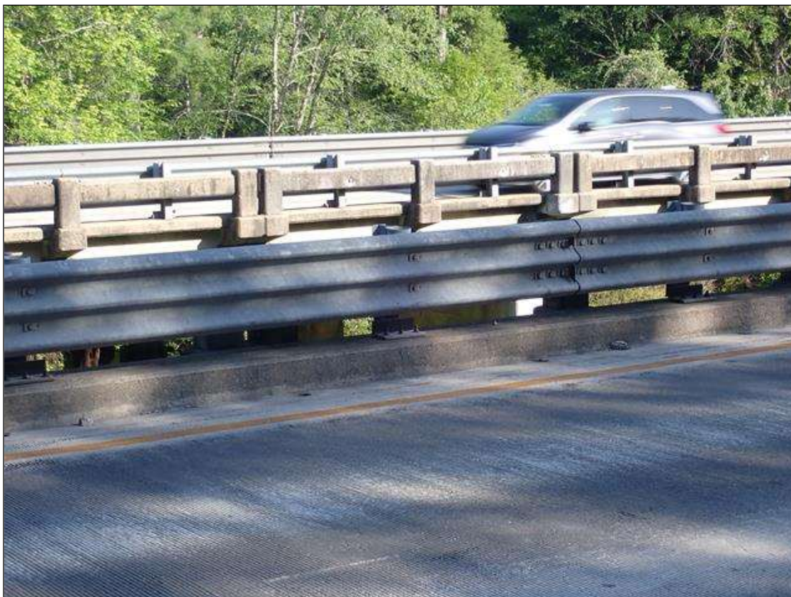
LEFT BARRIER RAIL (RIGHT BARRIER RAIL SIMILAR)
