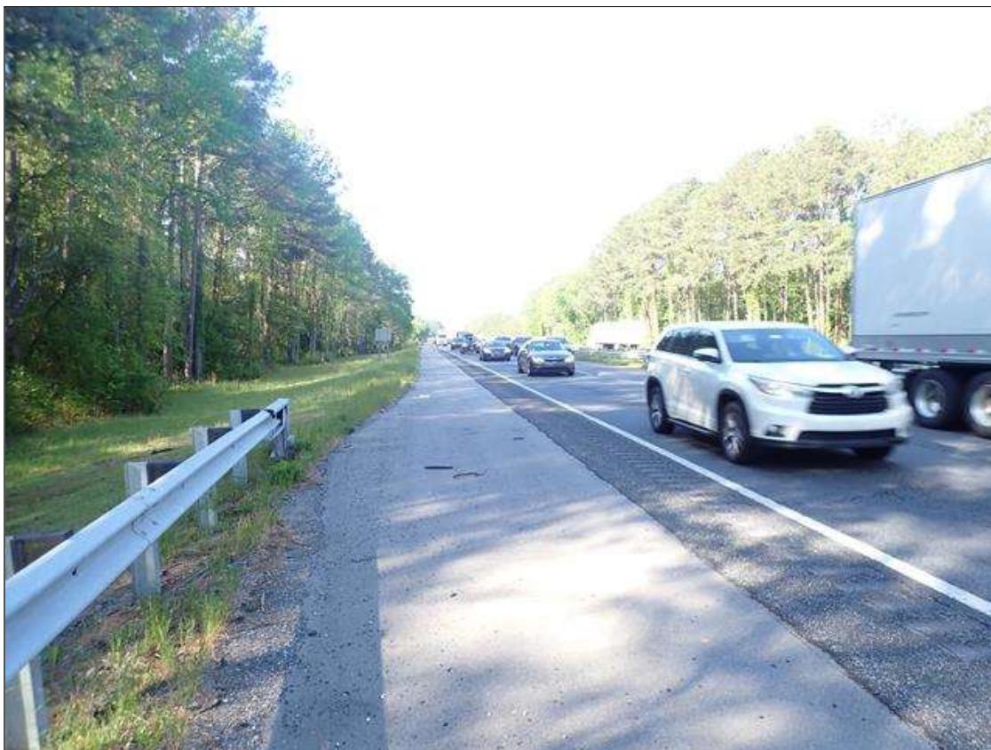
SOUTH APPROACH LOOKING SOUTH
