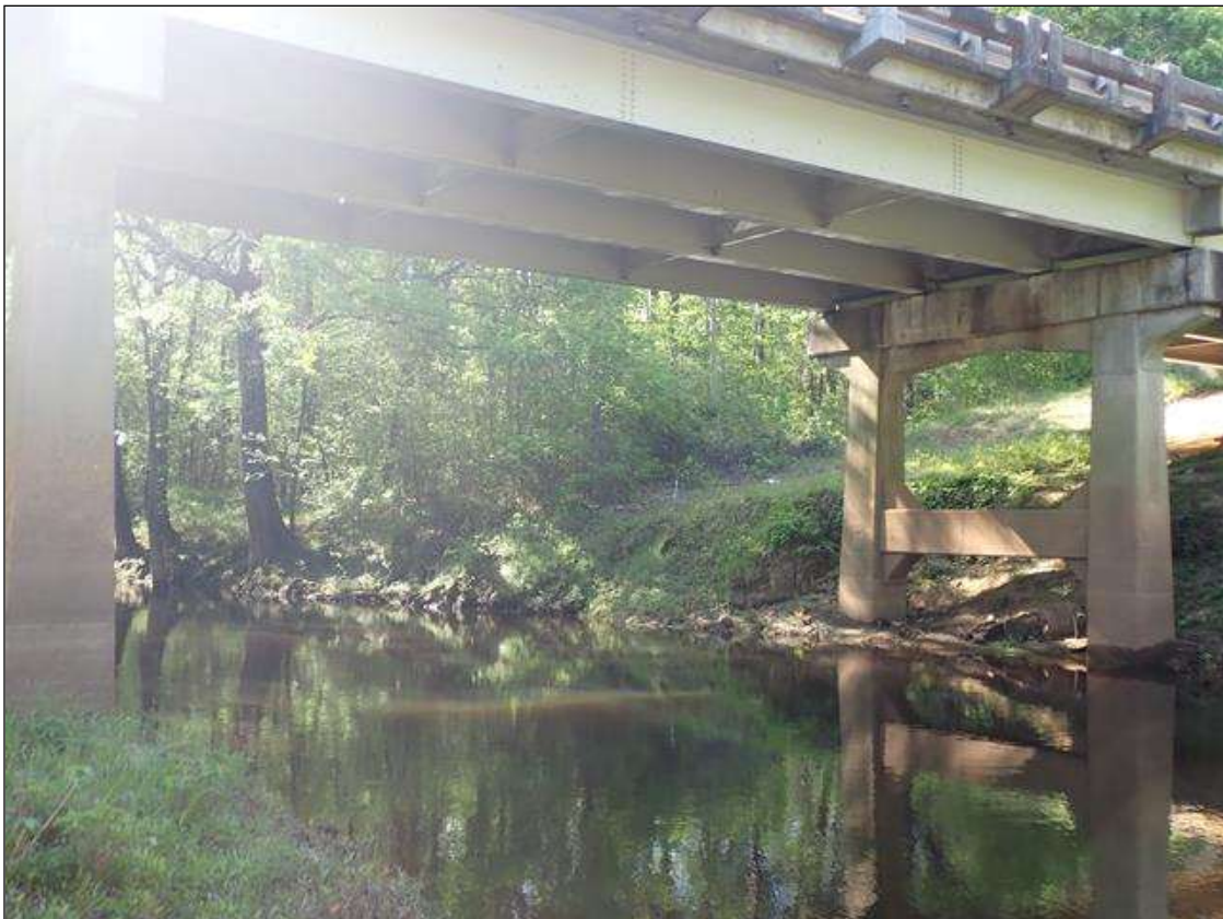
WATERWAY OPENING LOOKING DOWNSTREAM (SPAN 2)
