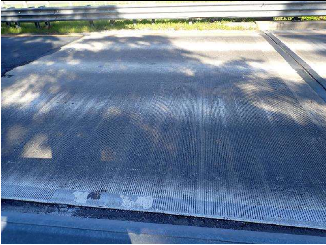
SOUTH APPROACH SLAB
