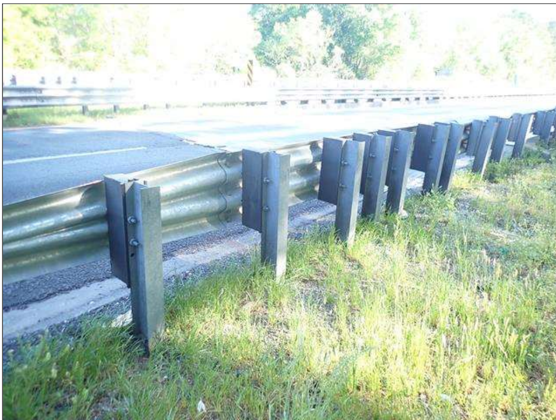
GUARDRAIL TRANSITION (SOUTHEAST CORNER SHOWN)
