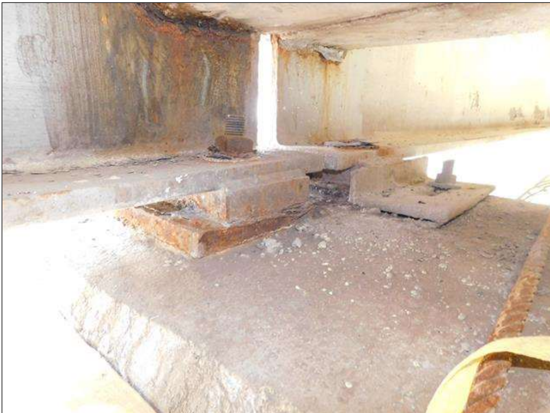
Bent bearing (Beam 4, Bent 3 shown)
