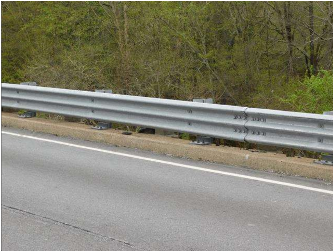
West bridge rail (East bridge rail similar)
