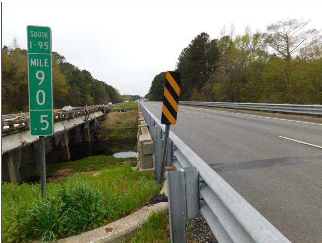
Northeast delineator (Northwest similar)
