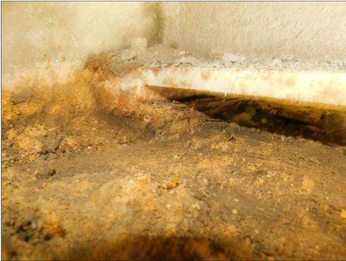
End Bent bearing (Beam 2, End Bent 2 shown)
