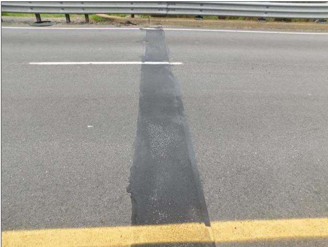
End Bent 1 joint (End Bent 2 joint similar)
