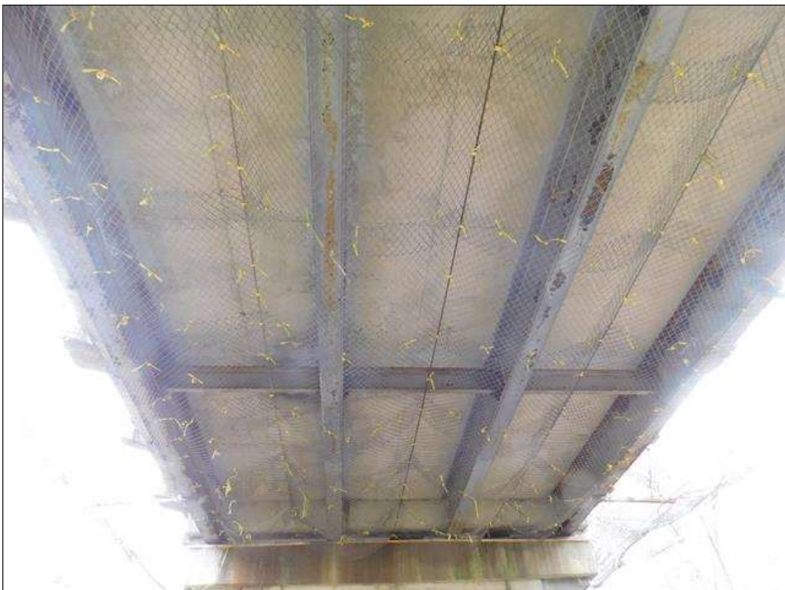
Underside of superstructure (Span 3 shown)
