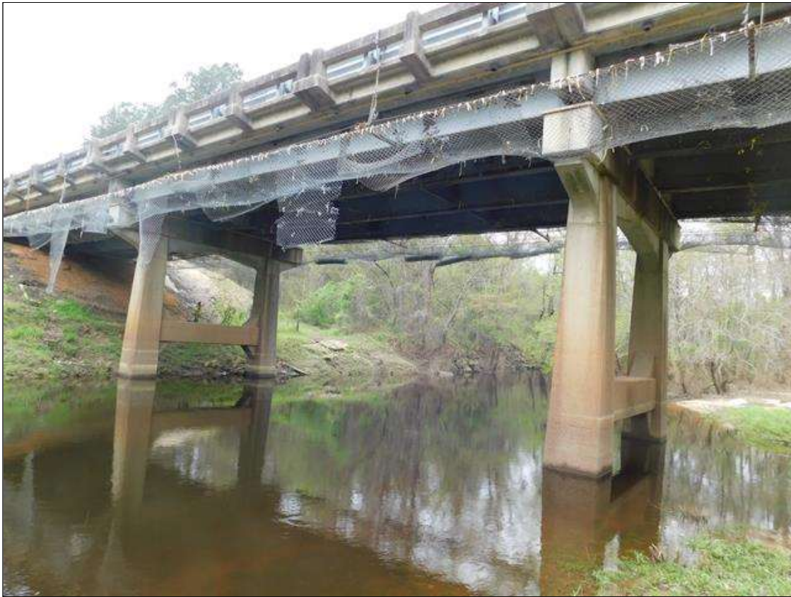
Downstream profile, looking West
