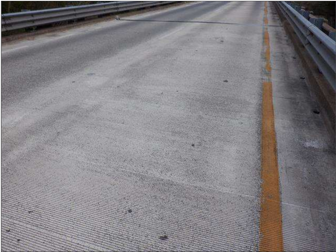
SPAN 1 CONCRETE WEARING SURFACE LOOKING NORTH
