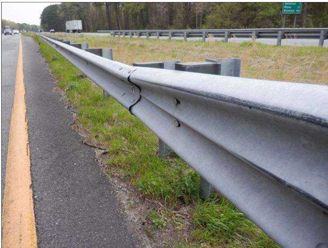
NORTHEAST GUARDRAIL TO BRIDGE RAIL TRANSITION (OTHERS SIMILAR)
