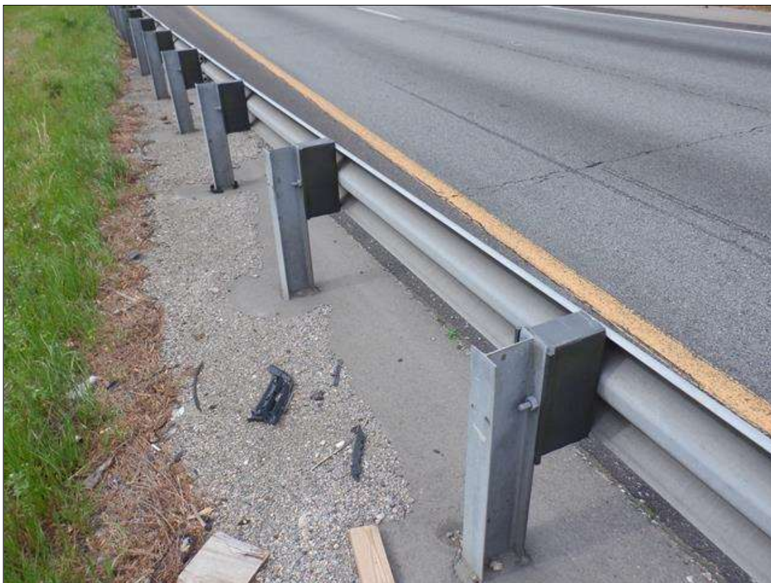
SOUTHEAST TYPICAL GUARDRAIL POST SPACING 75 INCHES (OTHERS SIMILAR)
