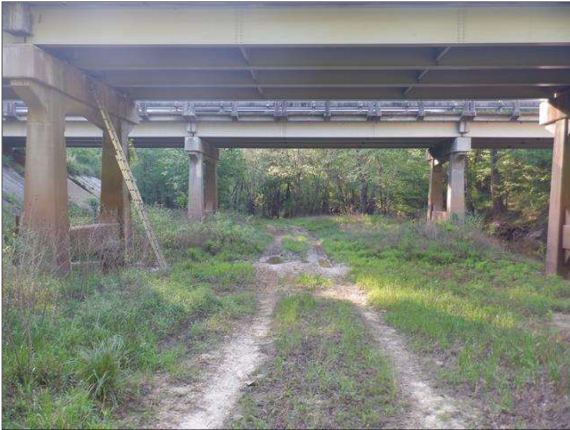
SPAN 3 CLEARANCE OPENING, GREENWAY, LOOKING EAST
