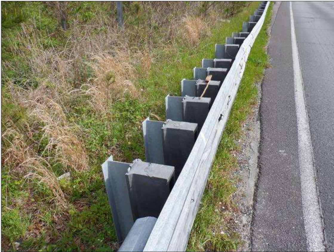
NORTHWEST GUARDRAIL POST SPACING AT BRIDGE 18 INCHES (OTHERS SIMILAR)
