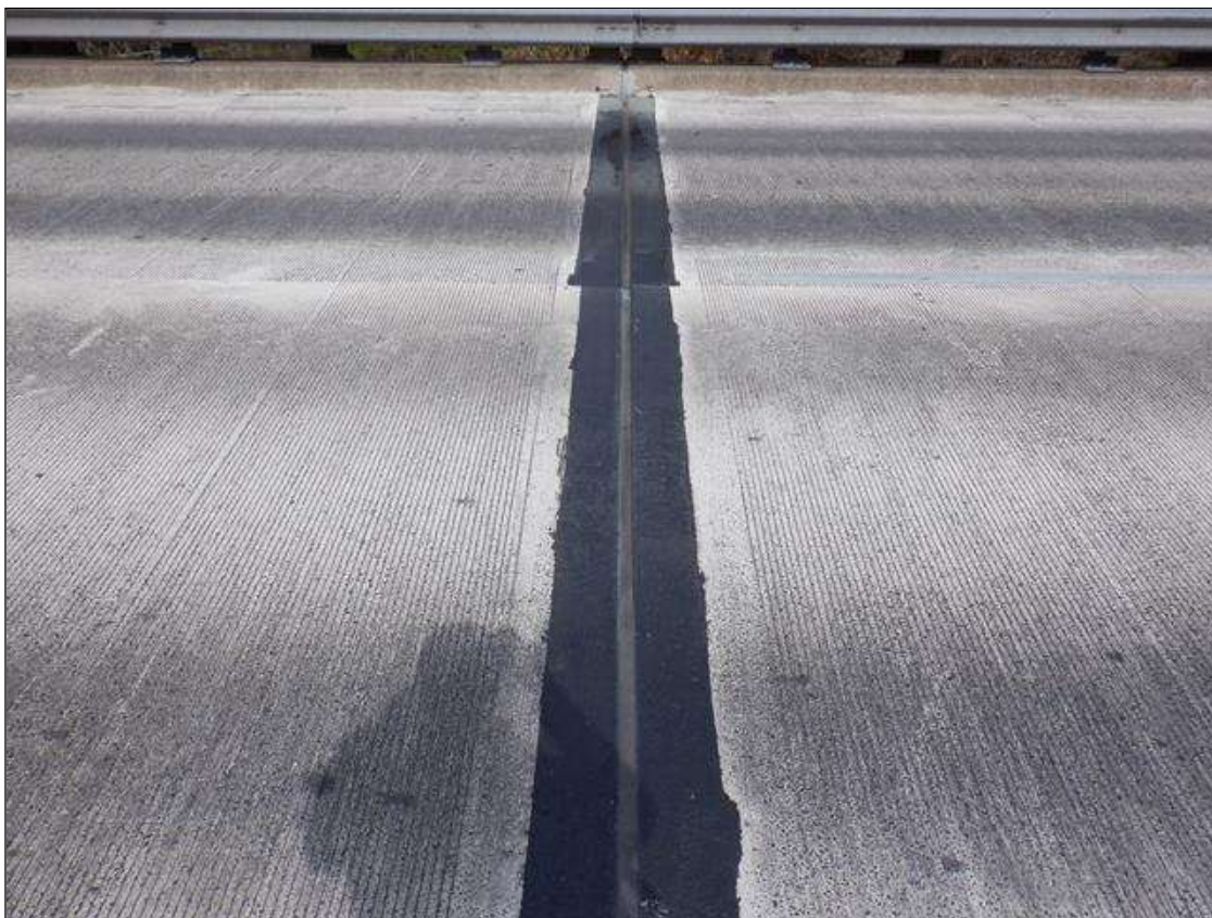
JOINT OVER BENT 3 LOOKING WEST
