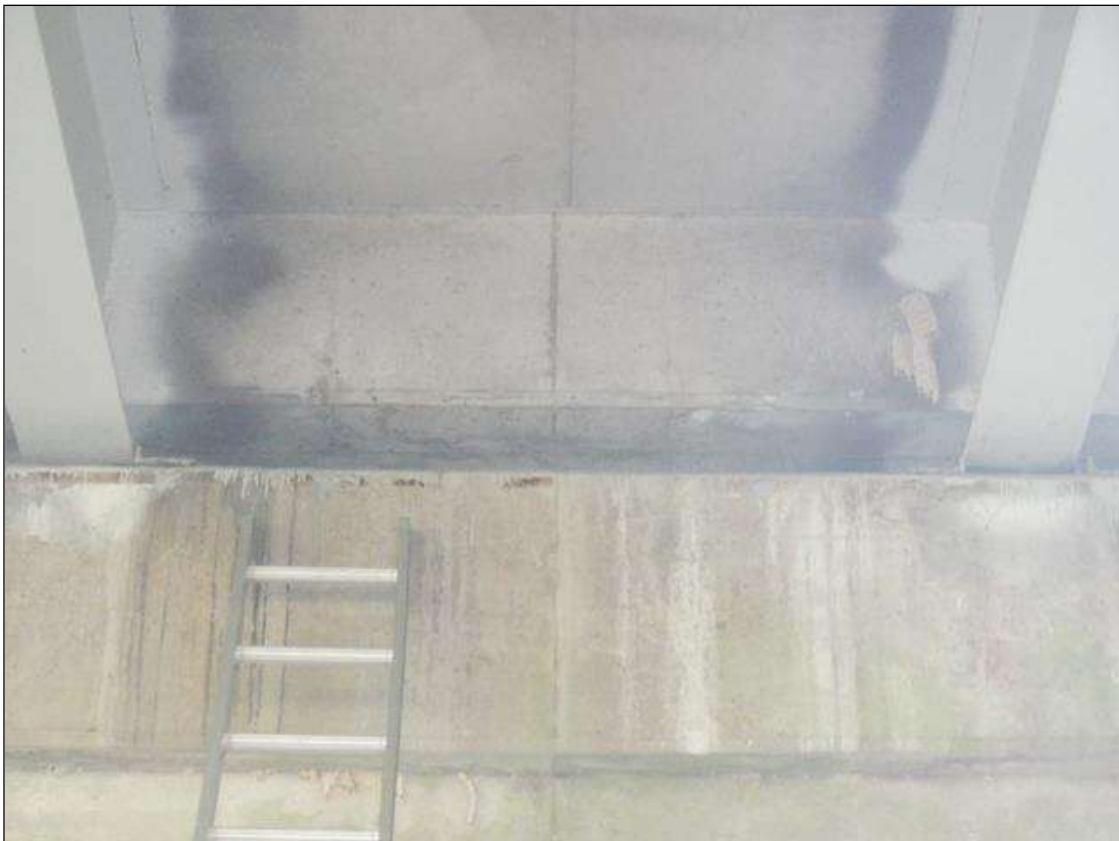
BENT 3 BAY 2 DIAPHRAGM LOOKING NORTH (OTHERS SIMILAR)
