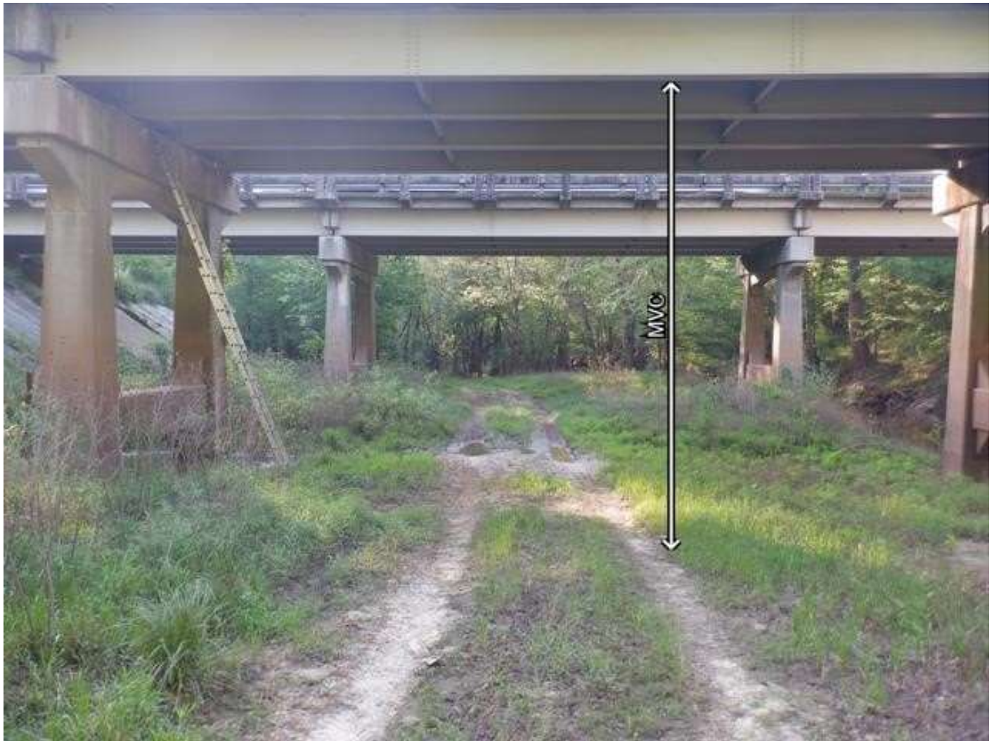
SPAN 3 CLEARANCE OPENING, GREENWAY, LOOKING EAST
