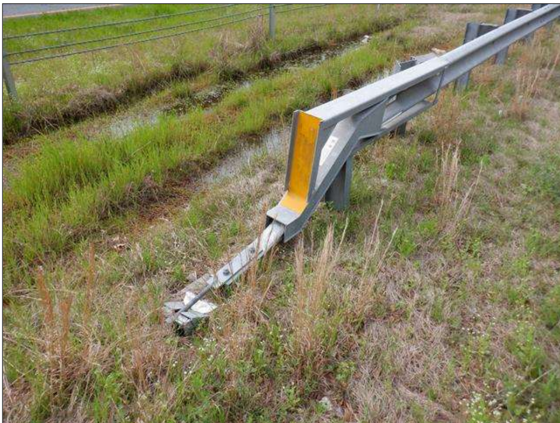
NORTHEAST GUARDRAIL TERMINAL (NORTHWEST SIMILAR)
