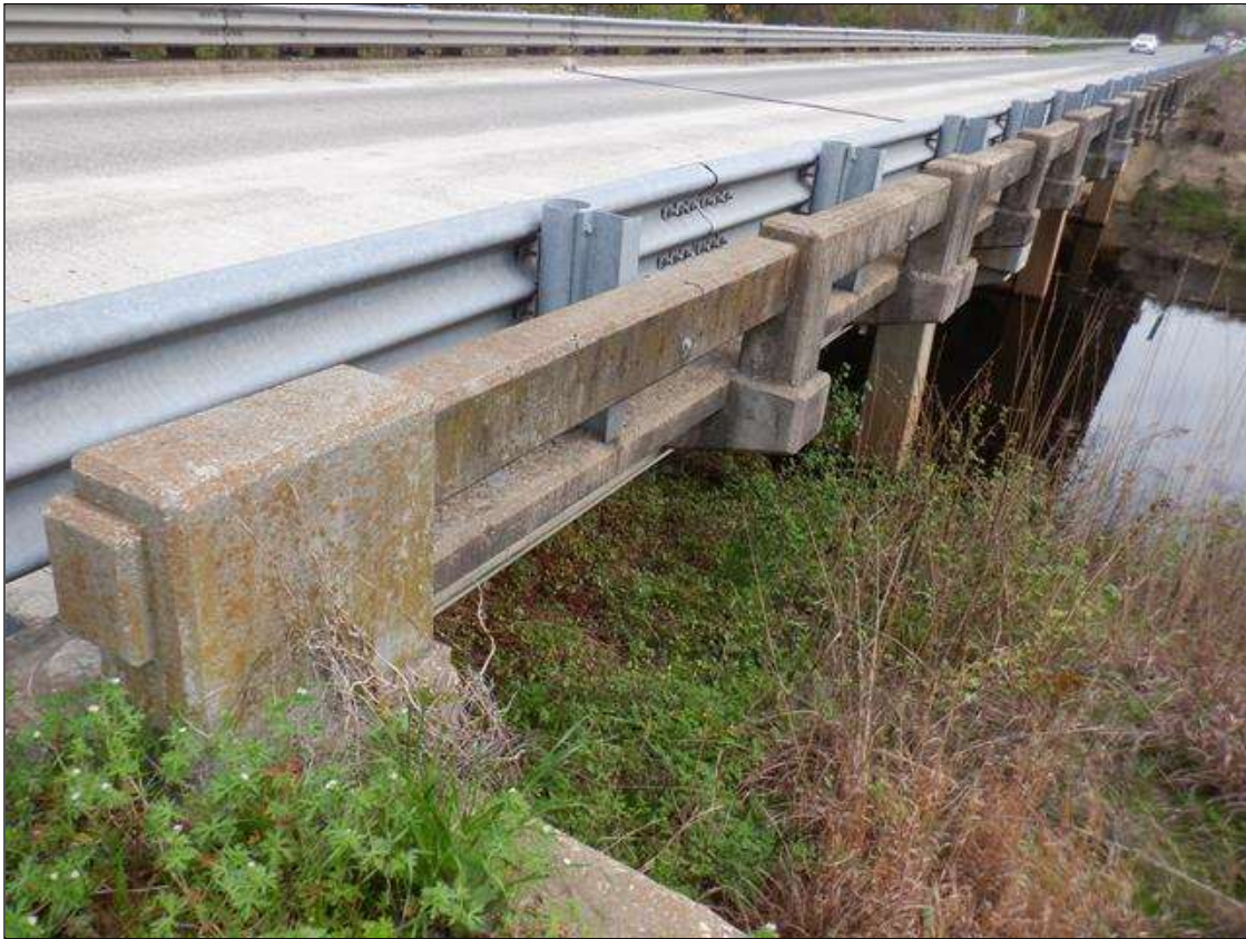
EAST BRIDGE RAIL
