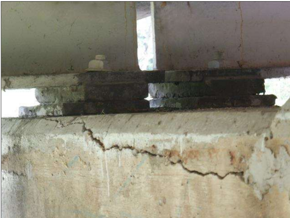
BEAM 1 BEARING ASSEMBLIES OVER BENT 1 (OTHERS SIMILAR)
