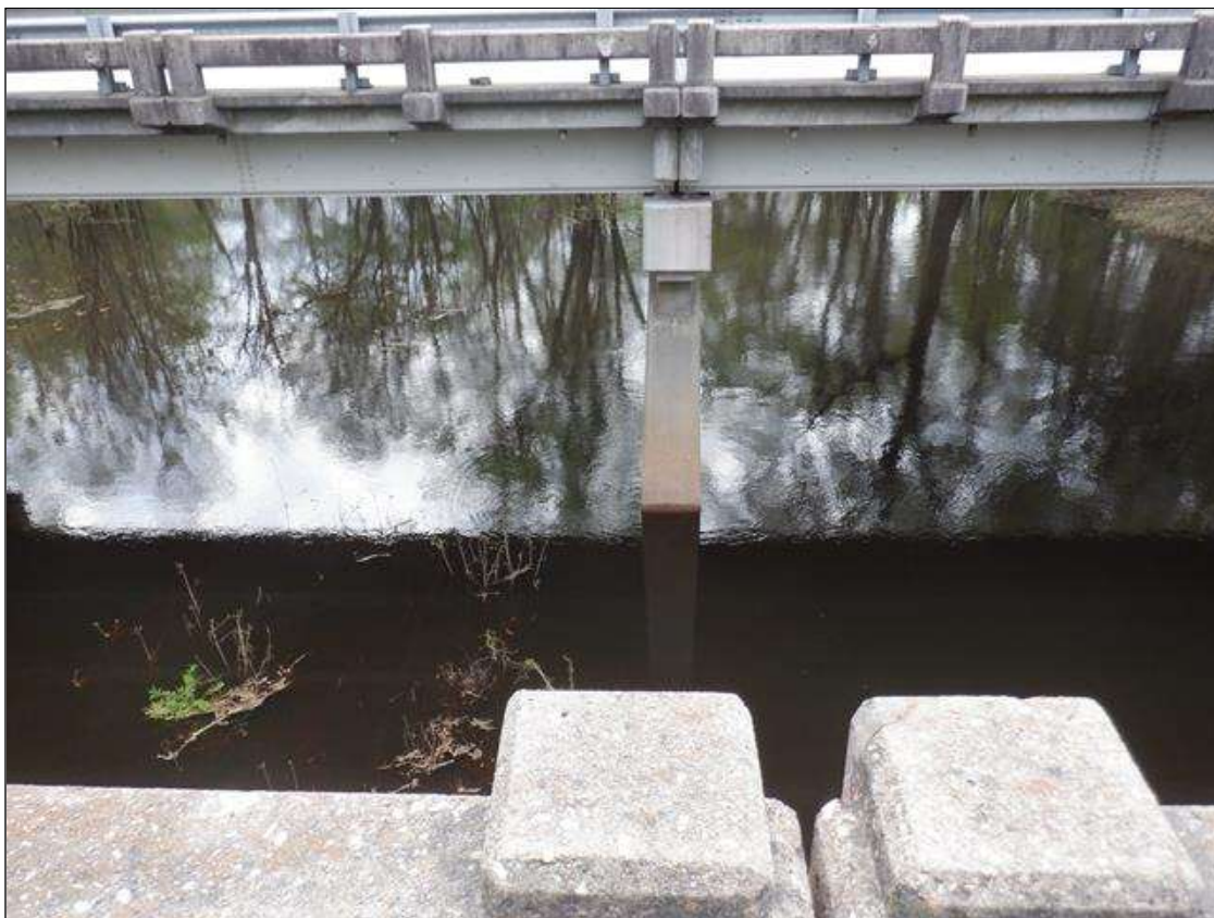
DOWNSTREAM VIEW FROM BRIDGE LOOKING EAST
