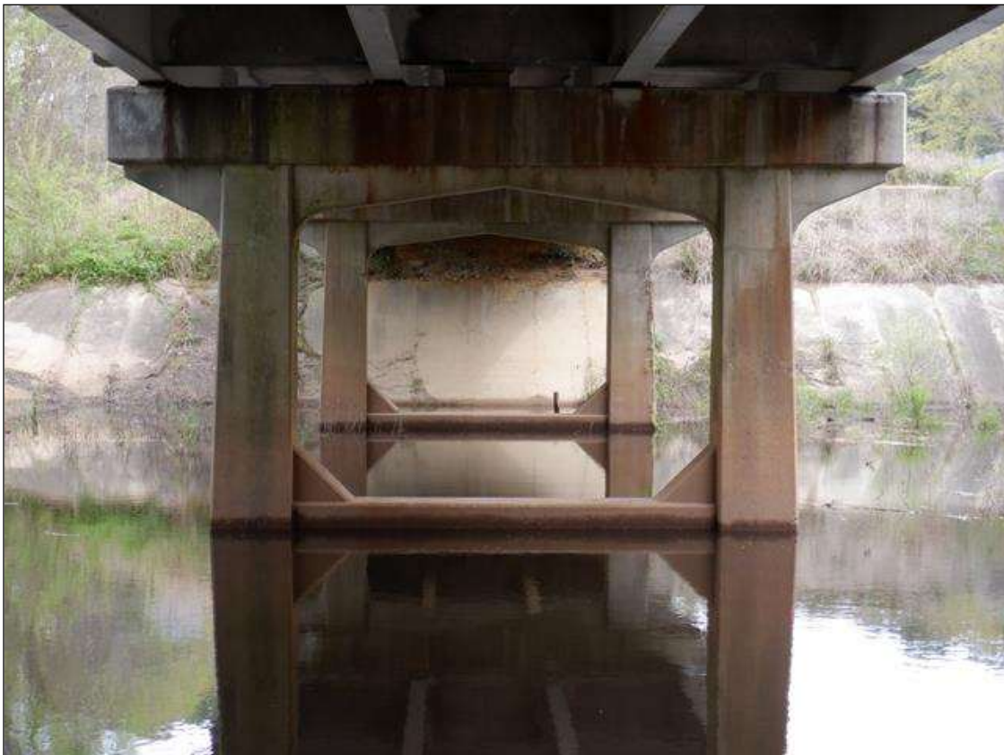
BENT 2 ELEVATION LOOKING NORTH
