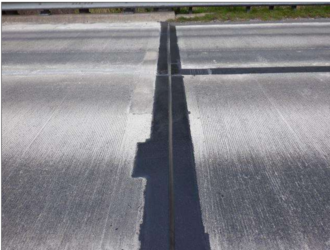
JOINT OVER END BENT 2 LOOKING WEST
