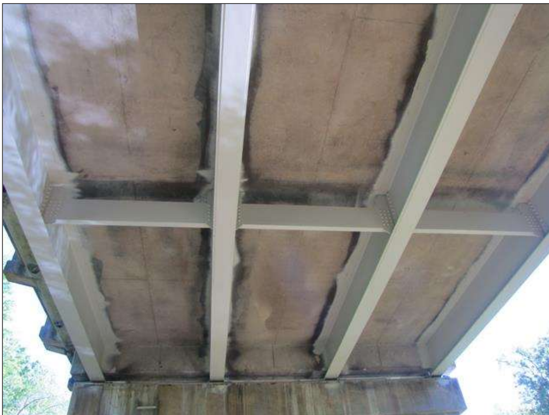
SUPERSTRUCTURE UNDERSIDE SPAN 3 LOOKING NORTH
