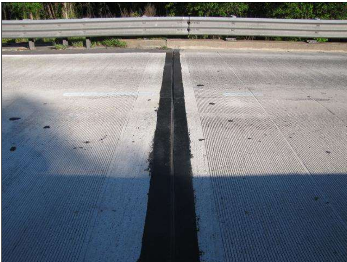
JOINT OVER END BENT 1 LOOKING WEST
