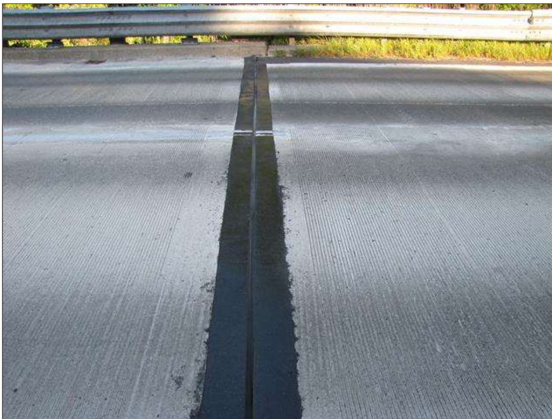
JOINT OVER END BENT 2 LOOKING WEST
