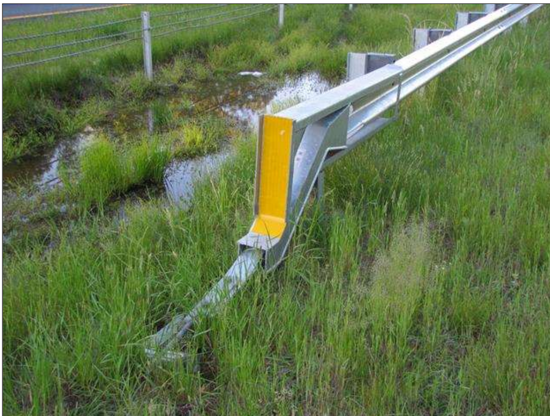
NORTHEAST GUARDRAIL TERMINAL (NORTHWEST SIMILAR)
