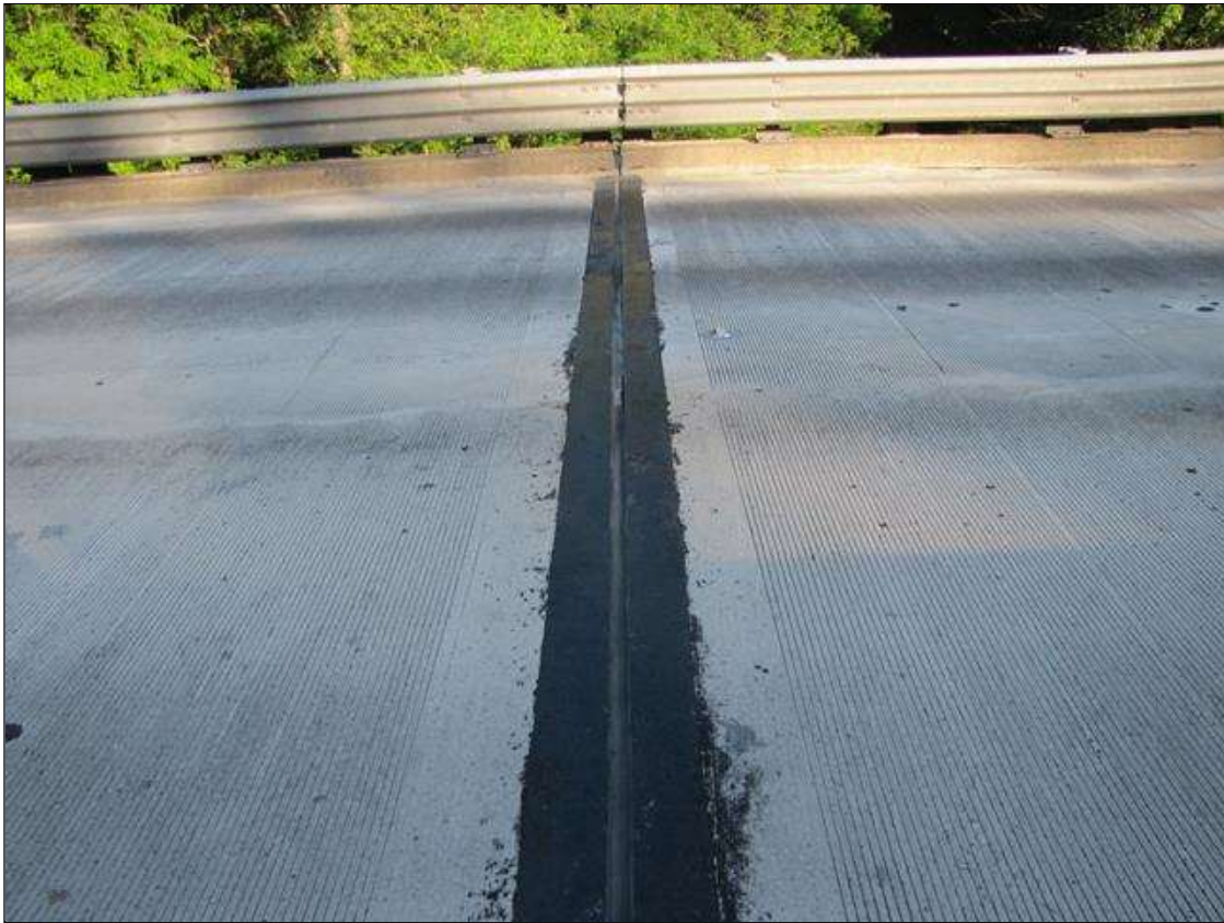
JOINT OVER BENT 2 LOOKING WEST
