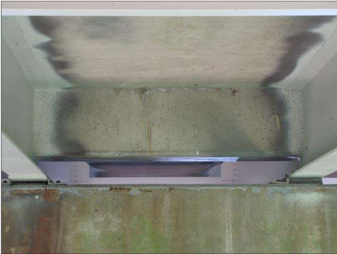
BENT 1 DIAPHRAGM SPAN 1 BAY 2 (OTHERS SIMILAR)
