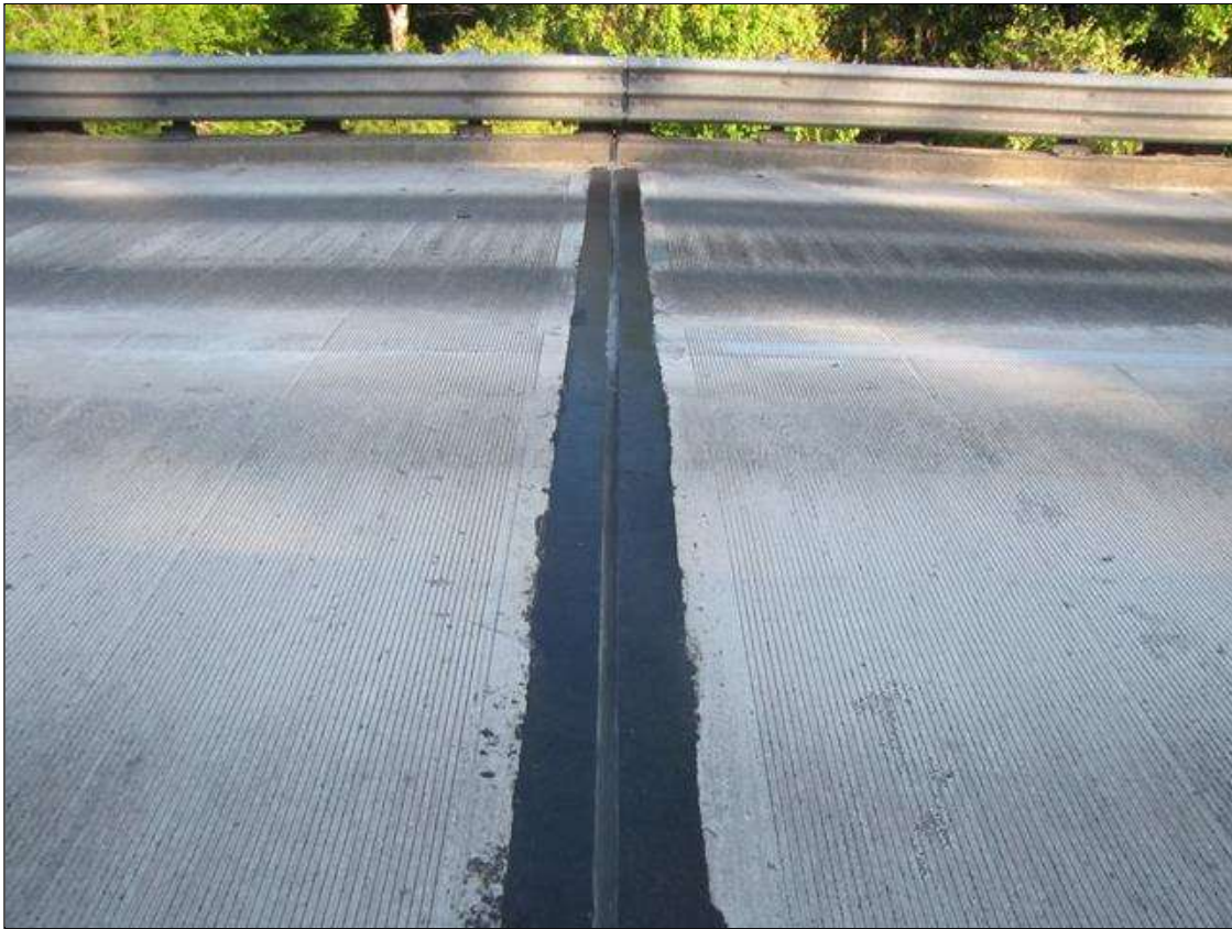
JOINT OVER BENT 3 LOOKING WEST
