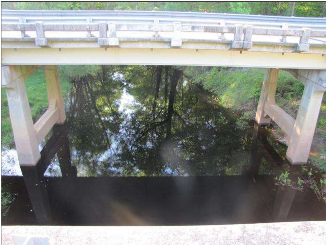
DOWNSTREAM VIEW FROM BRIDGE LOOKING EAST
