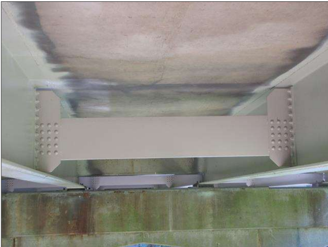
INTERMEDIATE DIAPHRAGM SPAN 1 BAY 2 LOOKING NORTH
