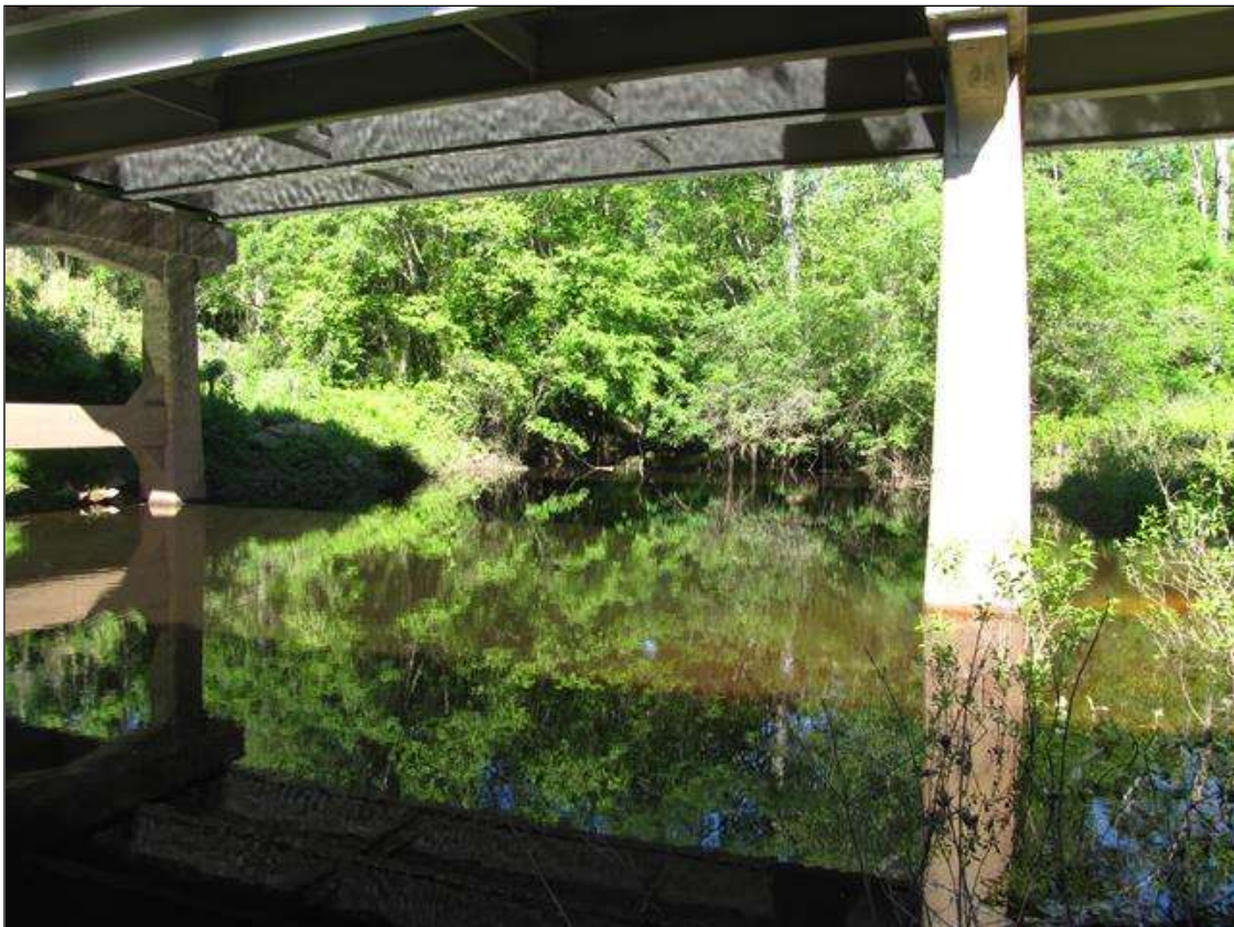
UPSTREAM VIEW FROM BANK UNDER SPAN 2
