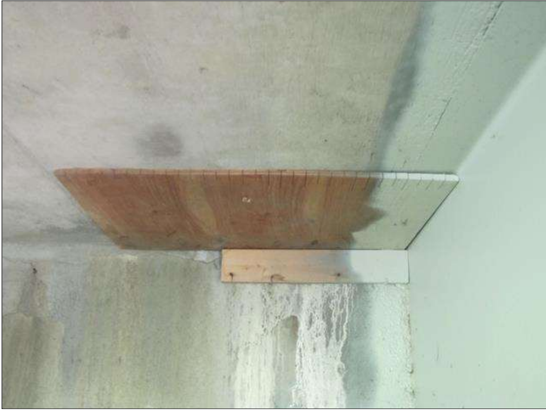
Span 4 Deck: 4' x 2.5' TIMBER STAY IN PLACE FORM WORK IN BAY 1 AT END BENT 2.( 1' X 1' SIMILAR IN BAY 3)
