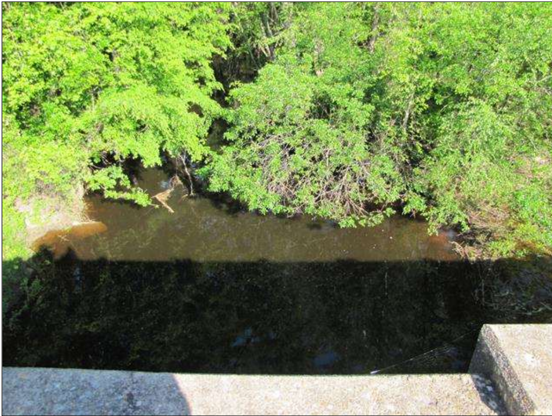
UPSTREAM VIEW FROM BRIDGE LOOKING WEST
