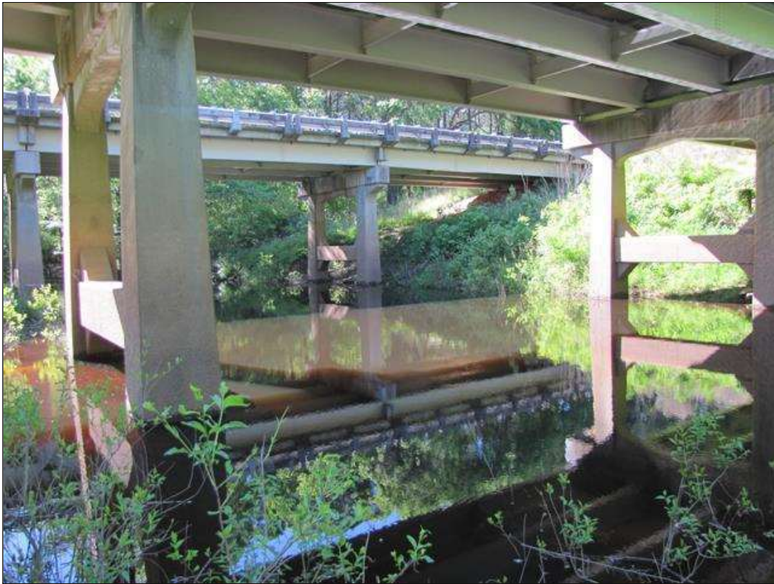
DOWNSTREAM VIEW FROM BANK UNDER SPAN 2
