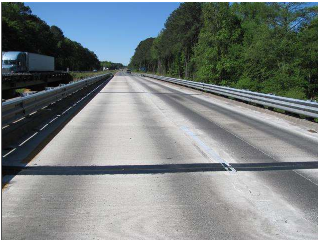
CONCRETE WEARING SURFACE SPAN 4 LOOKING SOUTH
