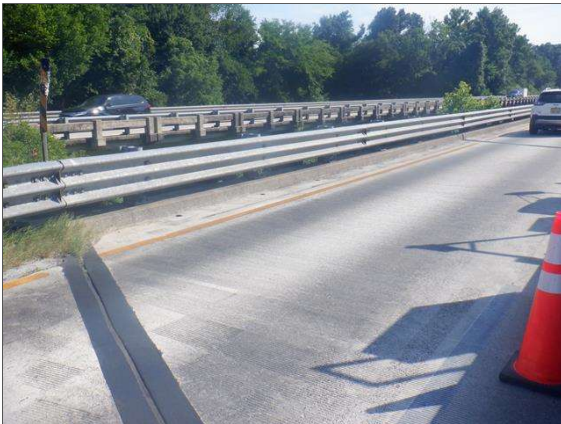
TYPICAL LEFT BRIDGE RAIL IN SPAN 1
