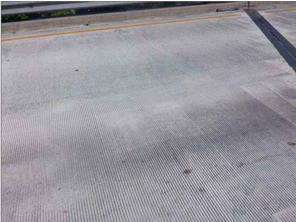
TOP OF DECK
