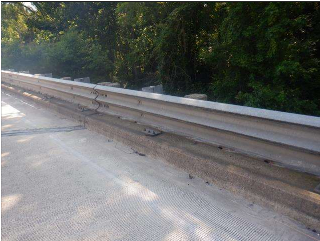
TYPICAL RIGHT BRIDGE RAIL IN SPAN 7
