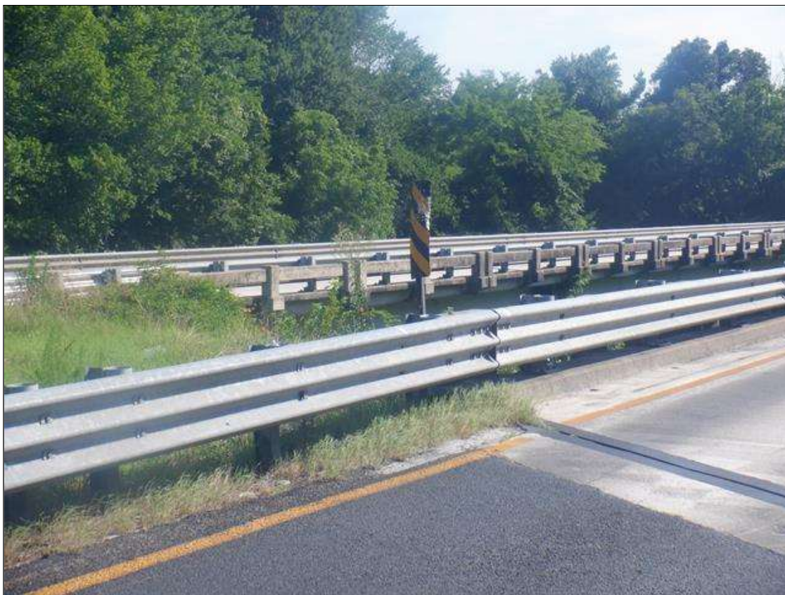
DELINEATOR AT SOUTHWEST CORNER
