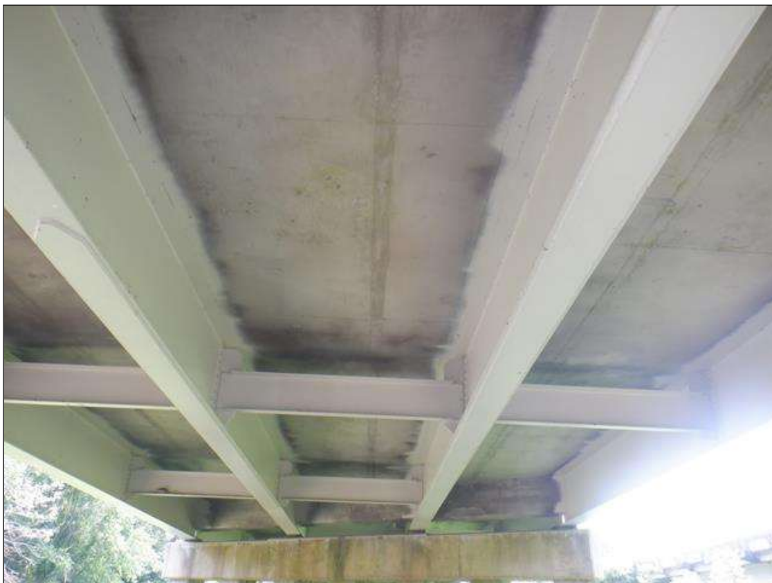
TYPICAL SUPERSTRUCTURE UNDERSIDE SPAN 3
