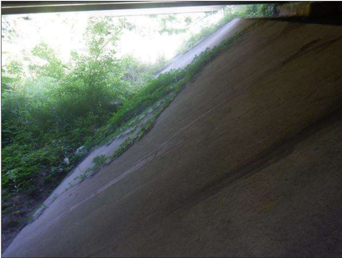
SLOPE PROTECTION AT END BENT 2
