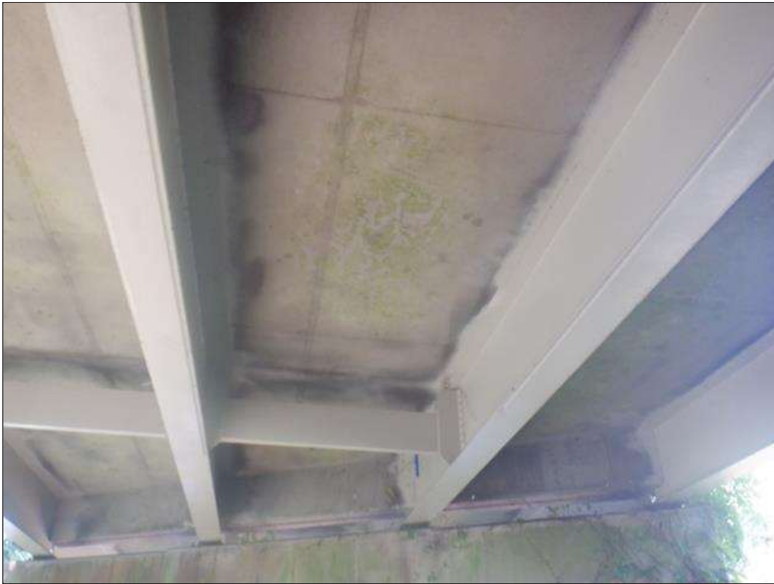
SUPERSTRUCTURE UNDERSIDE SPAN 8
