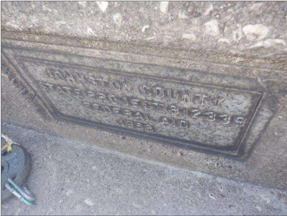
BRIDGE IDENTIFICATION AT SOUTHEAST CORNER
