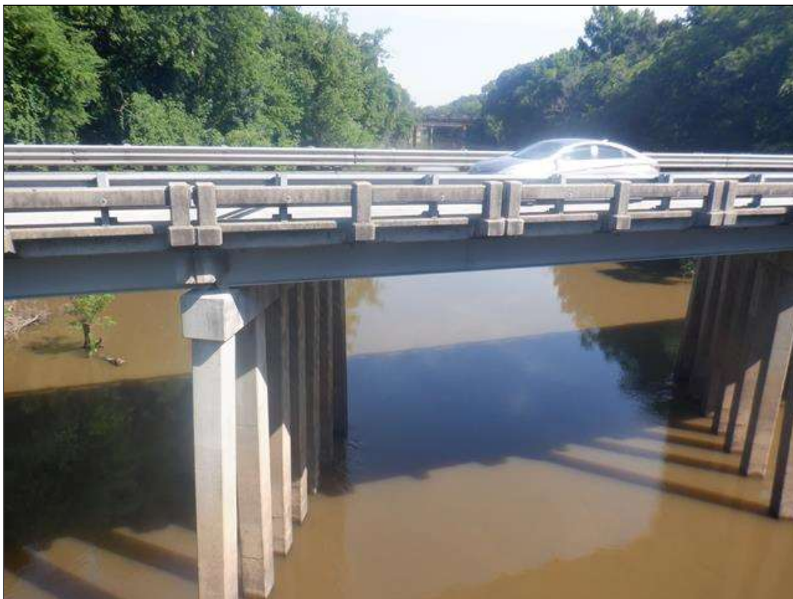
LOOKING UPSTREAM FROM TOP OF BRIDGE
