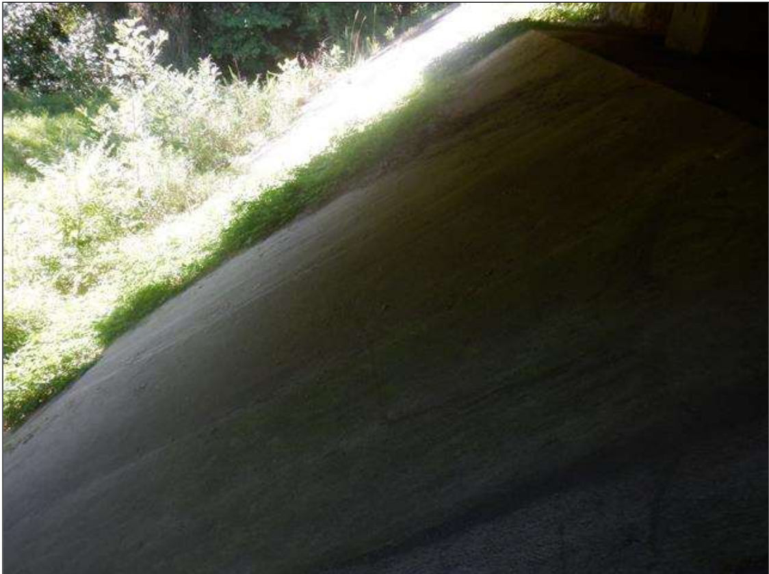
SLOPE PROTECTION AT END BENT 1
