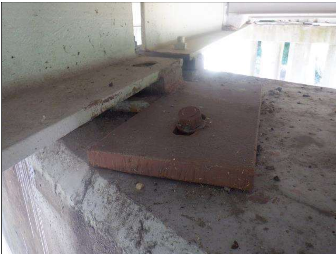
Span 4 Far Bearing: WELDED REPAIR WITH NEW ANCHOR BOLT.
