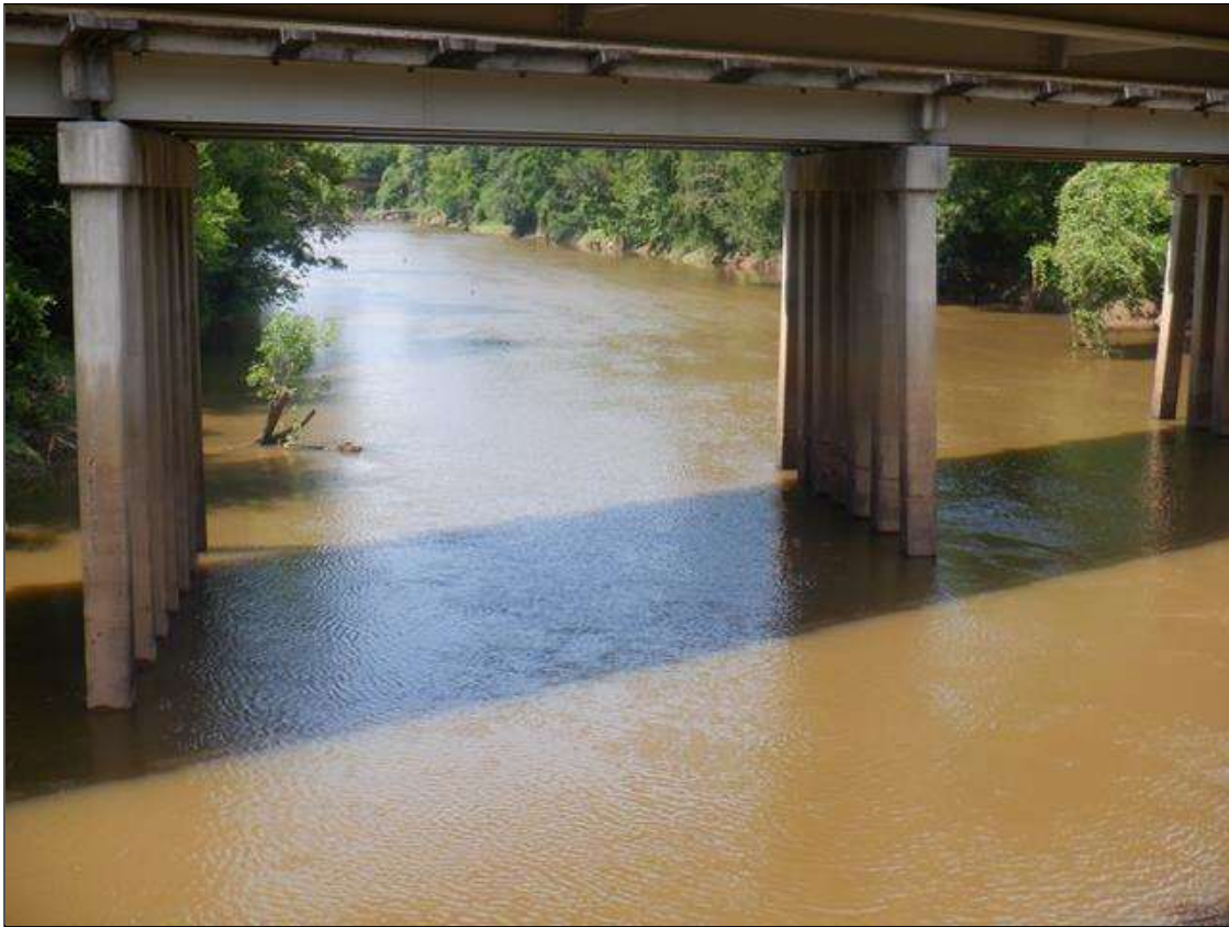
LOOKING UPSTREAM FROM UNDER THE BRIDGE
