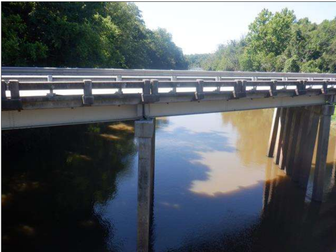
LOOKING DOWNSTREAM FROM TOP OF SPAN 5
