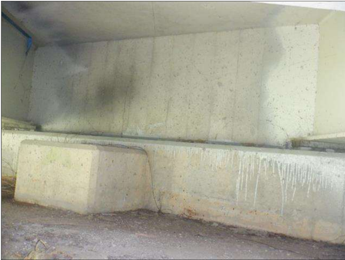
TYPICAL BACKWALL AND CAP AT END BENT 1
