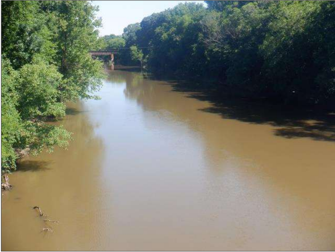
LOOKING UPSTREAM FROM TOP OF SPAN 4
