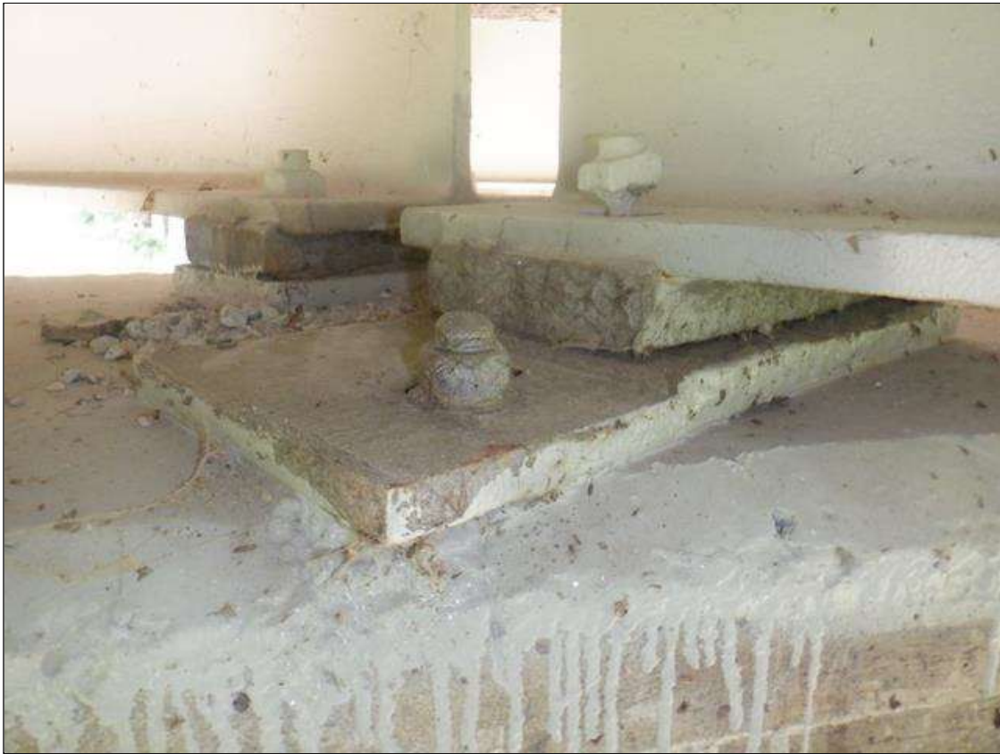
Span 3 Far Bearing: WELDED REPAIR WITH NEW ANCHOR BOLT.
