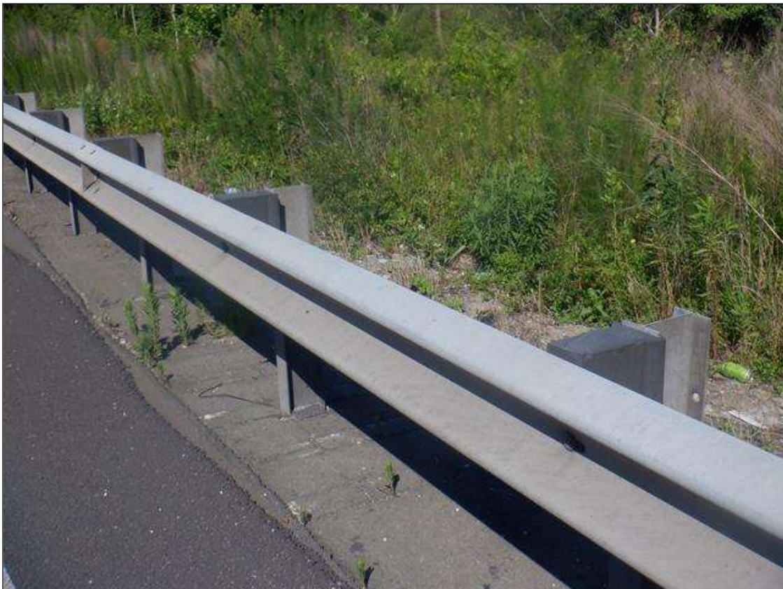
TYPICAL POST SPACING AT MID-LENGTH AT SOUTHWEST CORNER
