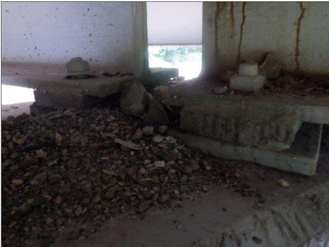
TYPICAL BEARINGS AT BENT
