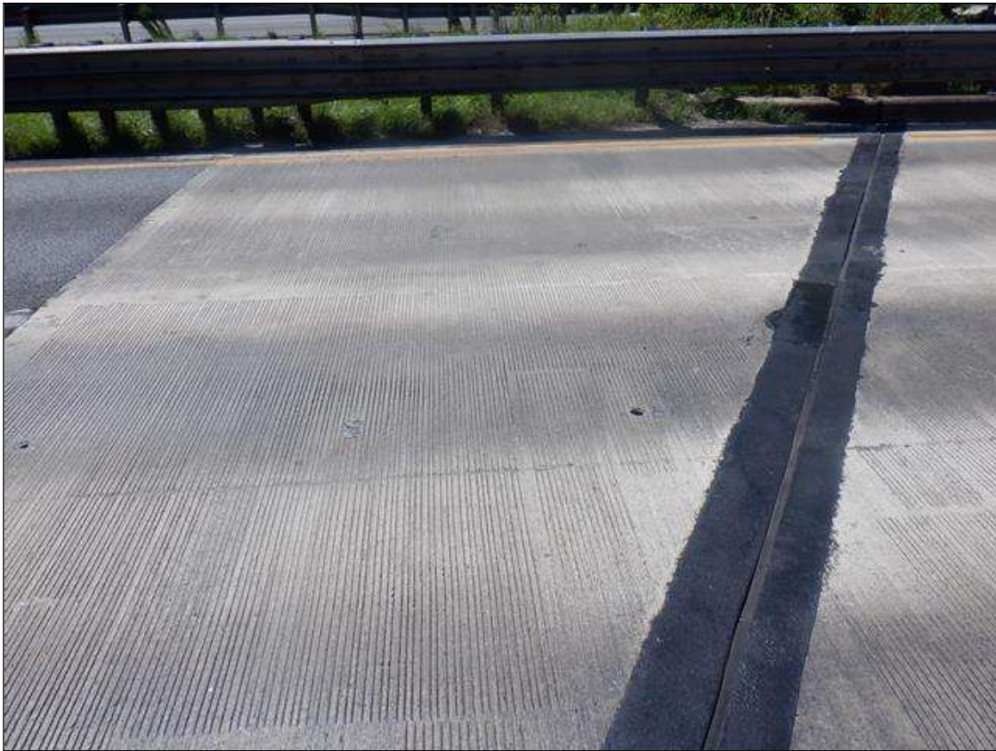
NORTH APPROACH SLAB
