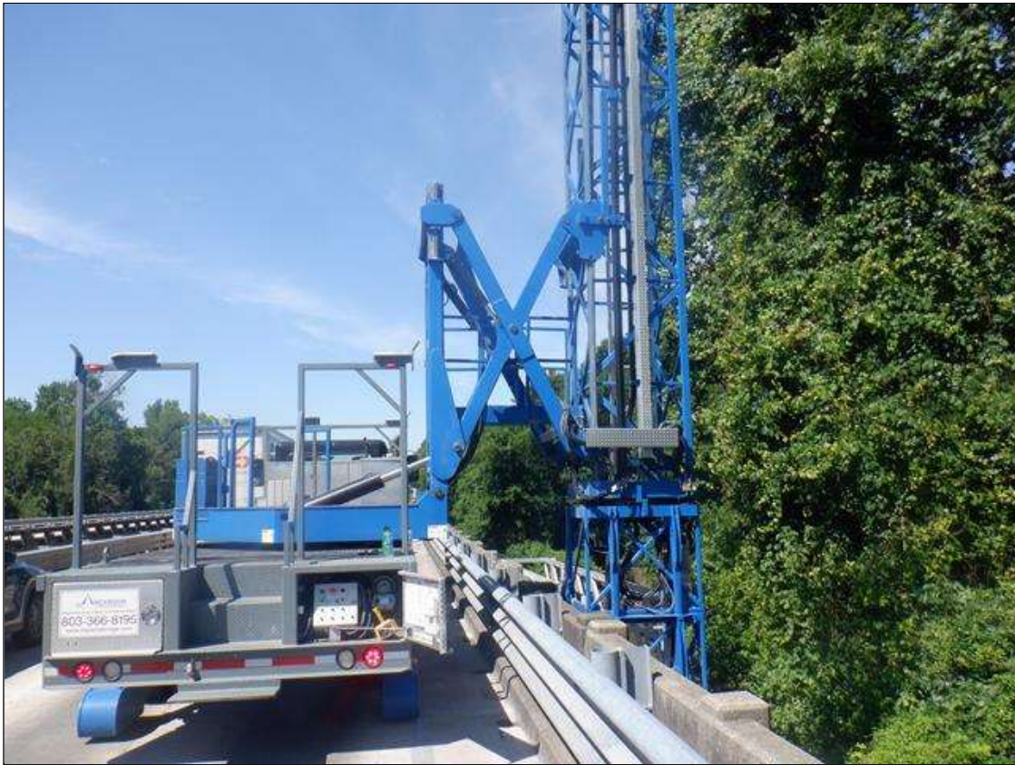
HYDRA PLATFORM USED
