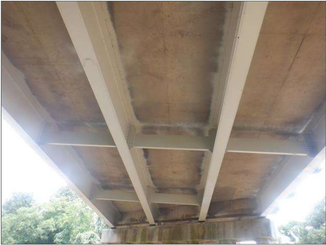
TYPICAL SUPERSTRUCTURE UNDERSIDE SPAN 4
