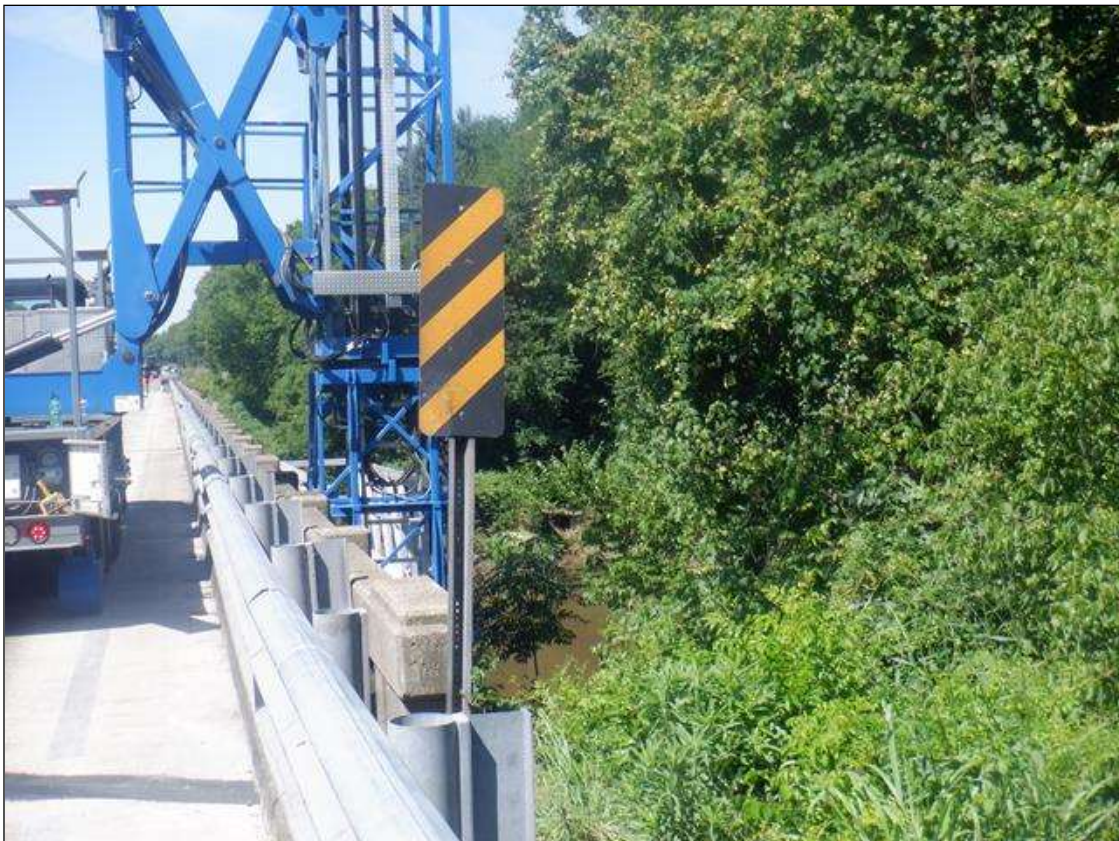
DELINEATOR AT NORTHWEST CORNER
