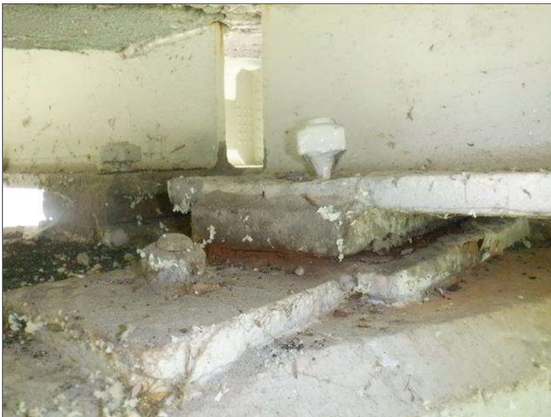
Span 2 Beam 2 - Far Bearing: WELDED BEARING REPAIR WITH ANCHOR ROD.
