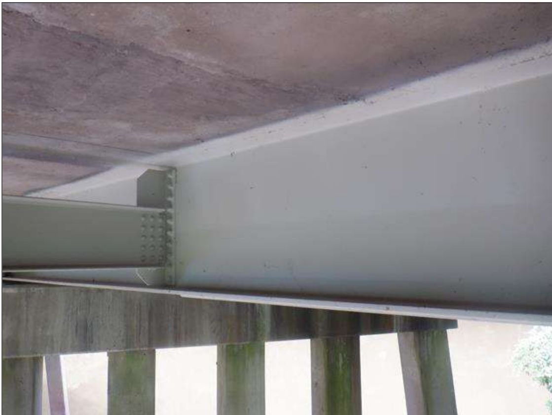
TYPICAL BEAMS AND INTERMEDIATE DIAPHRAGM PAINTED OVER IN ALL SPANS
