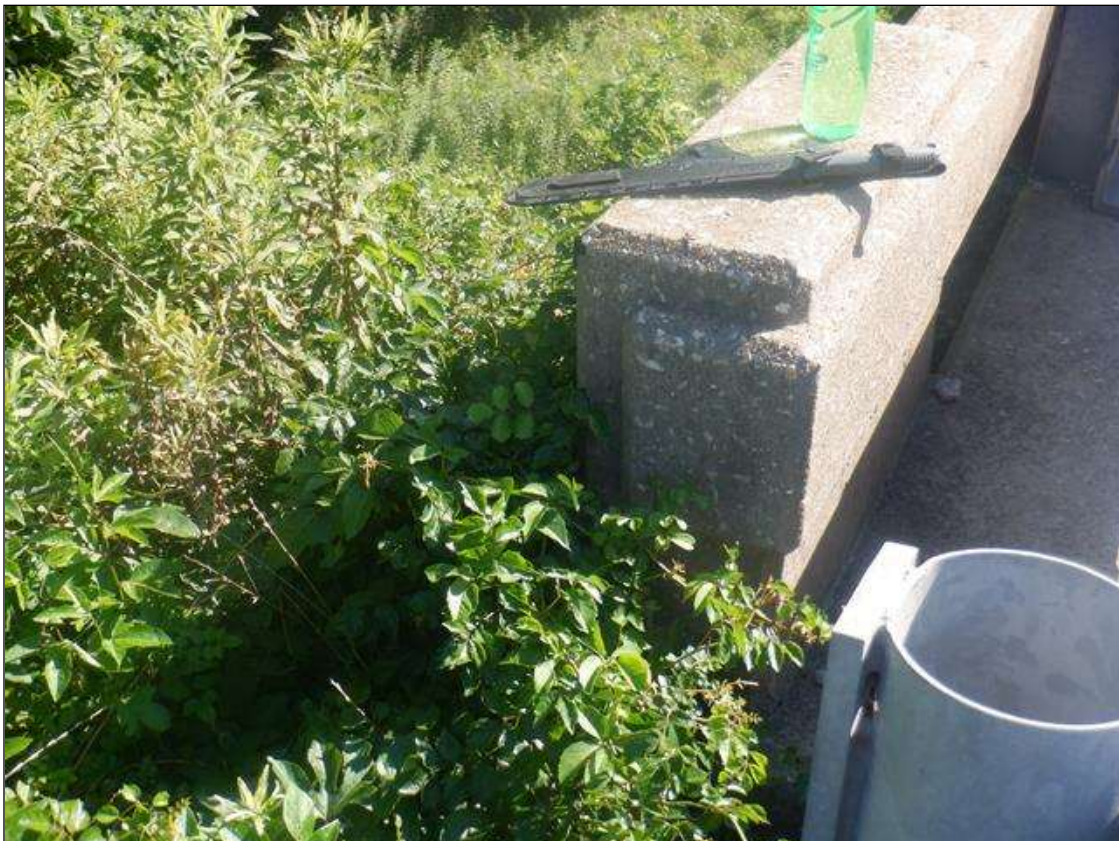
TYPICAL ENDS OF BRIDGE RAIL AT SOUTHWEST CORNER
