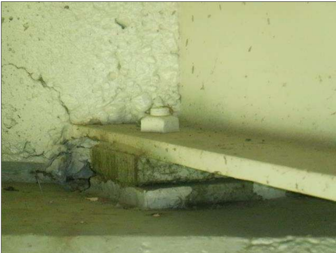
TYPICAL BEARINGS AT END BENT
