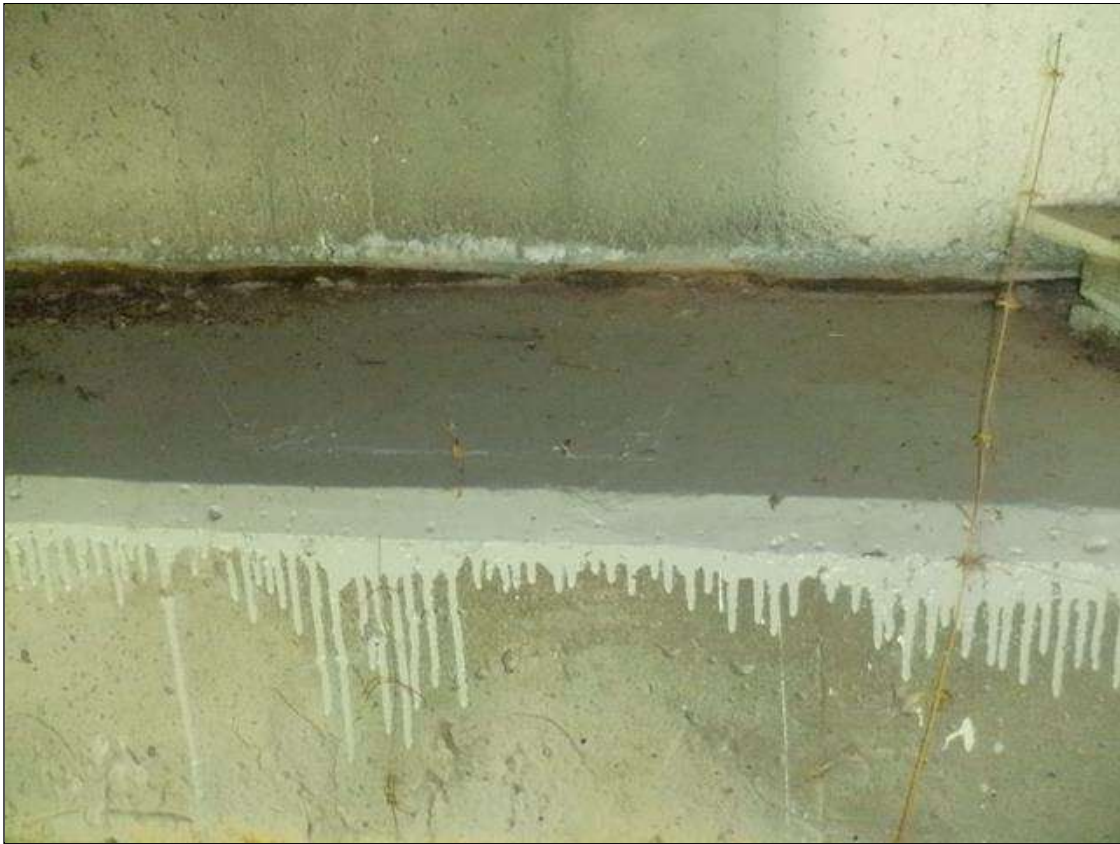
TYPICAL PAINT OVER TOP OF CAP AT END BENT
