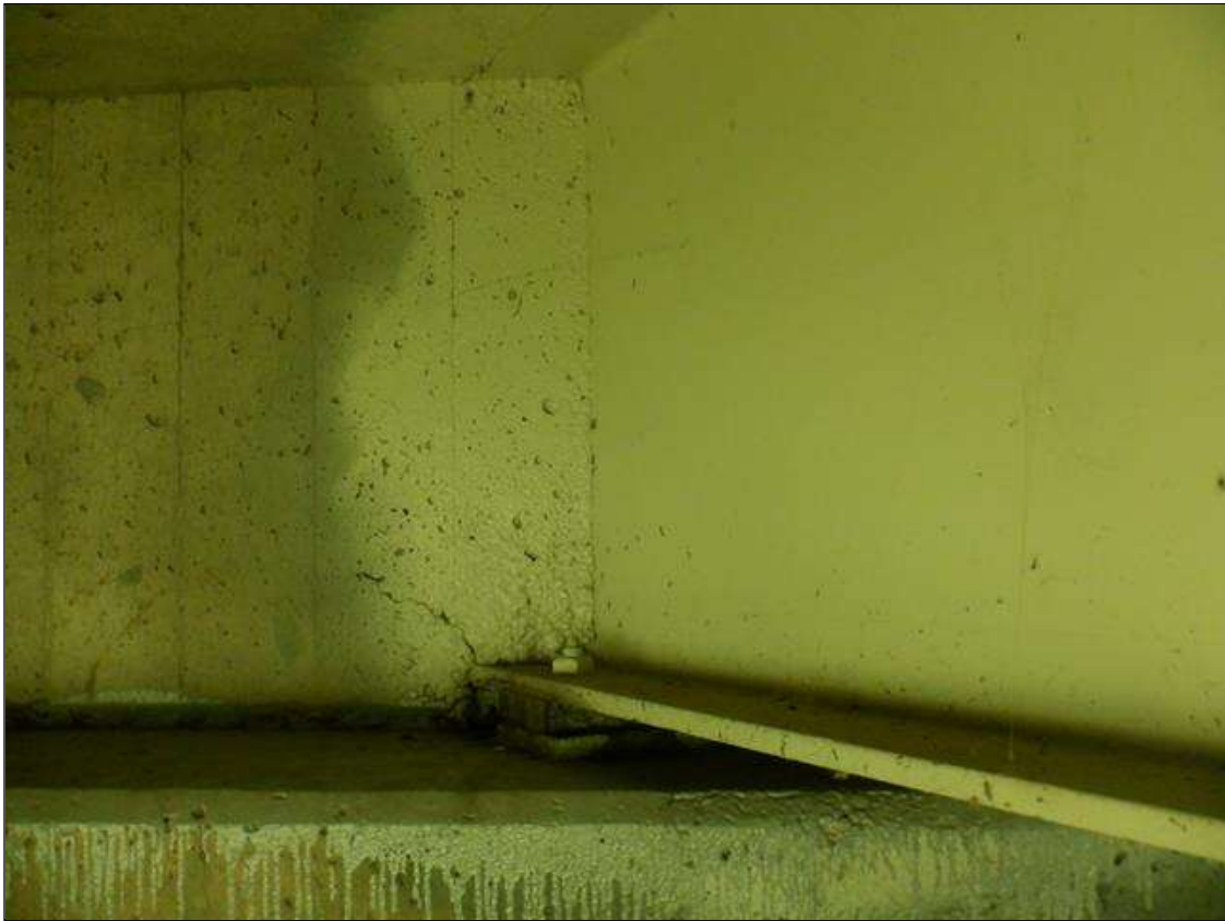
TYPICAL BEAM ENDS AT END BENT
