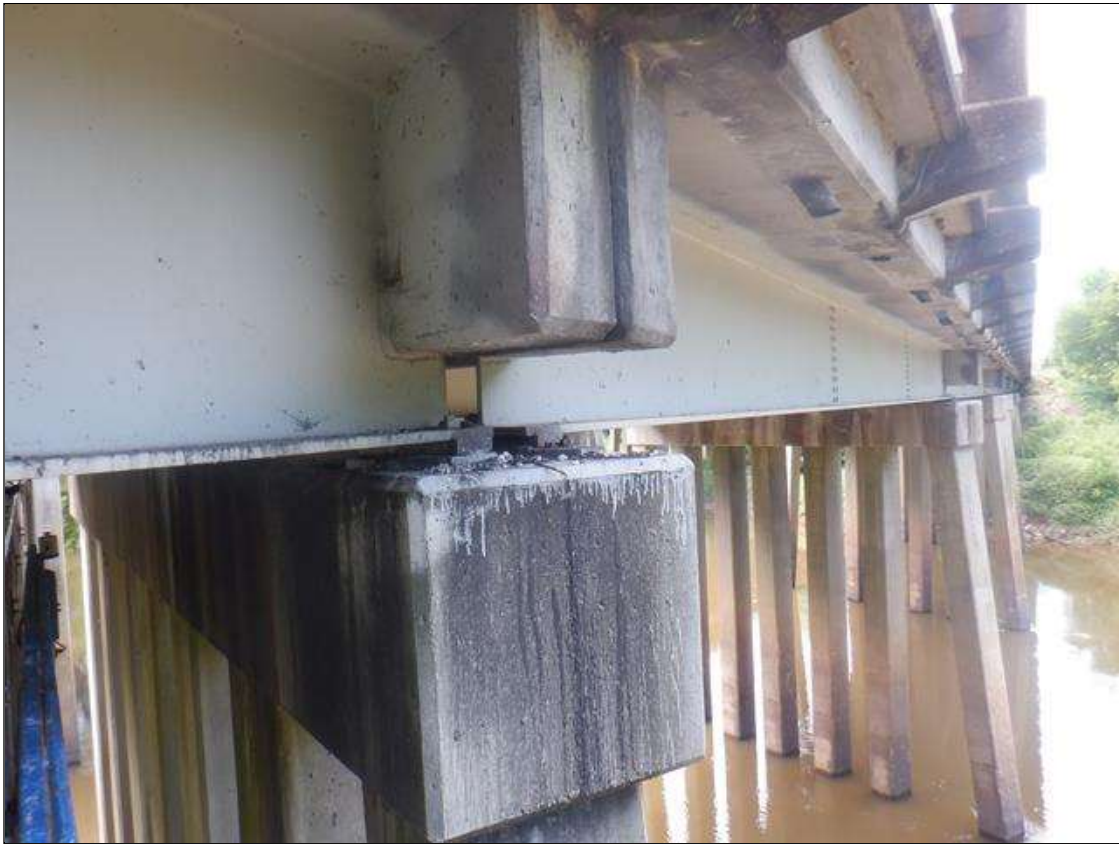
TYPICAL BEAM AND CAP ENDS
