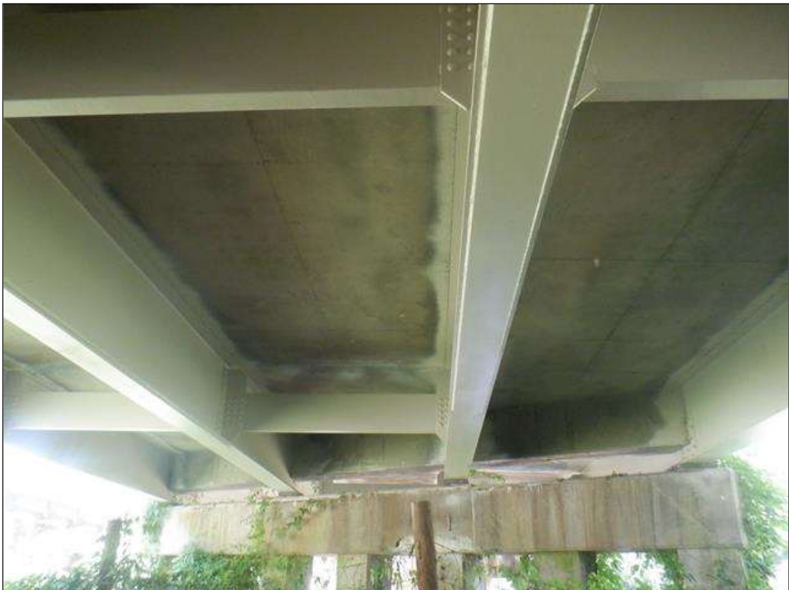
TYPICAL SUPERSTRUCTURE UNDERSIDE, SPAN 8
