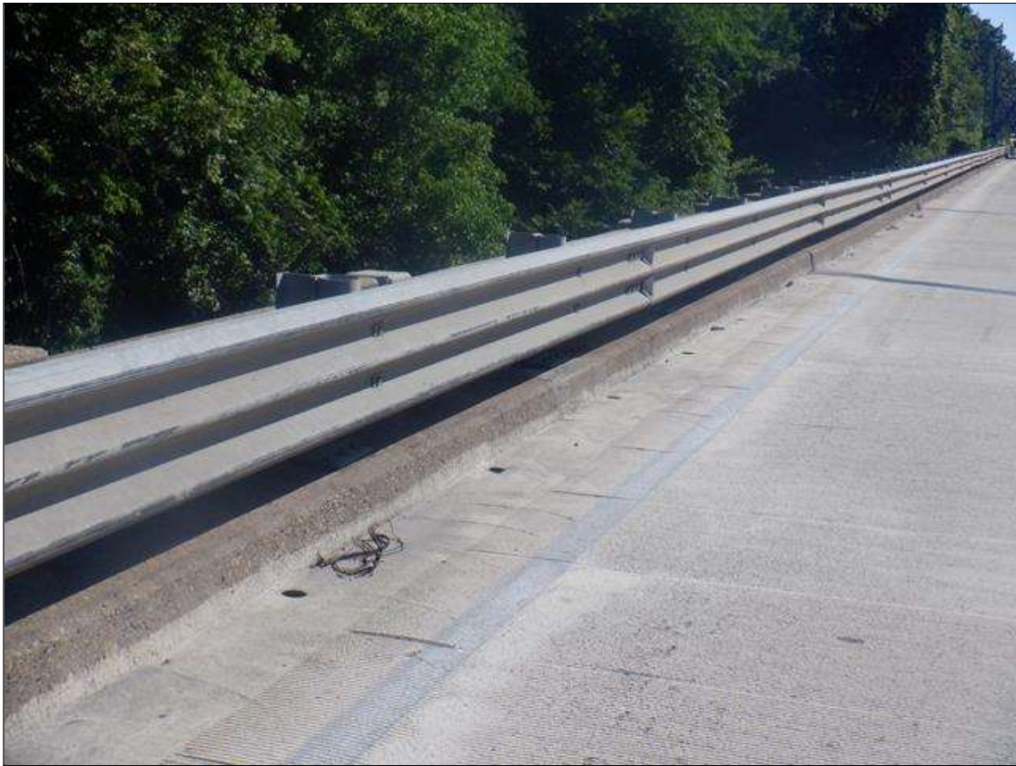
LEFT BRIDGE RAIL
