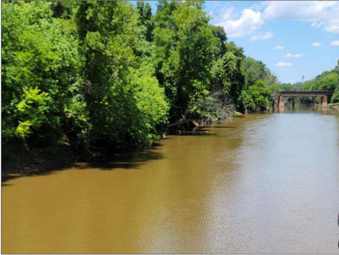
LOOKING UPSTREAM FROM UNDER THE BRIDGE
