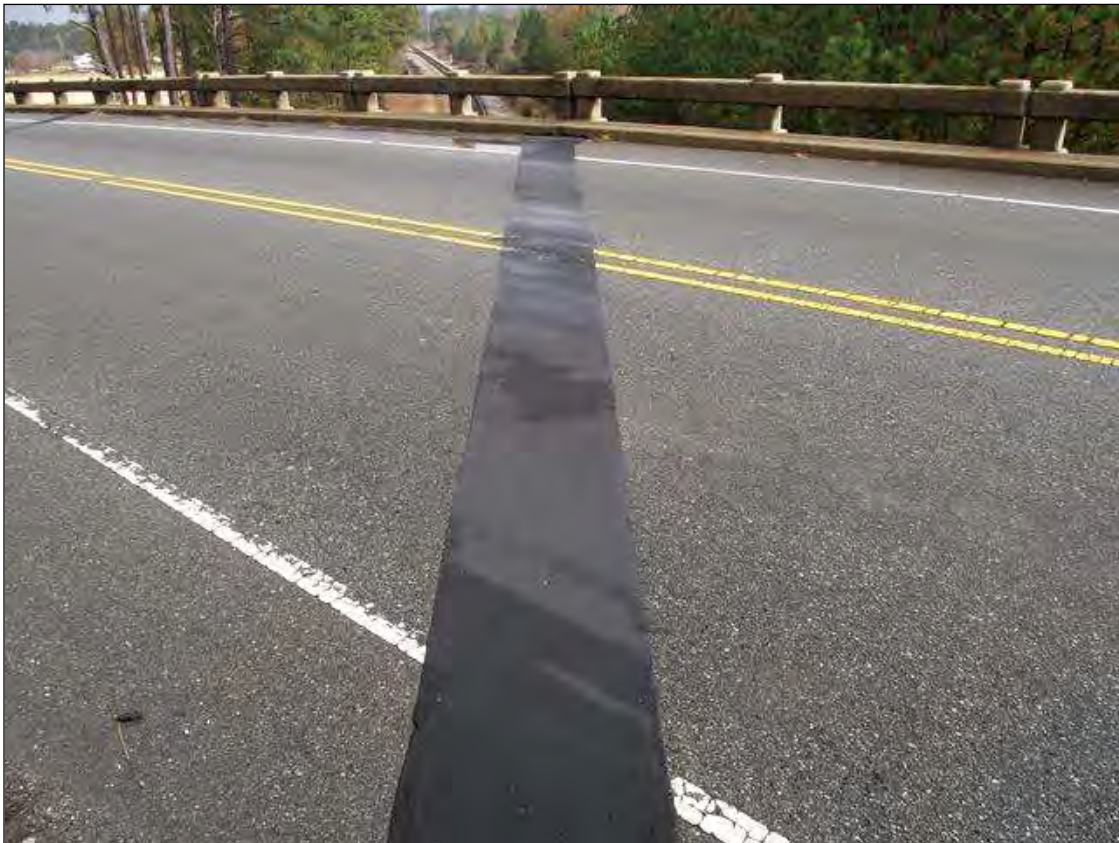
JOINT AT BENT 2
