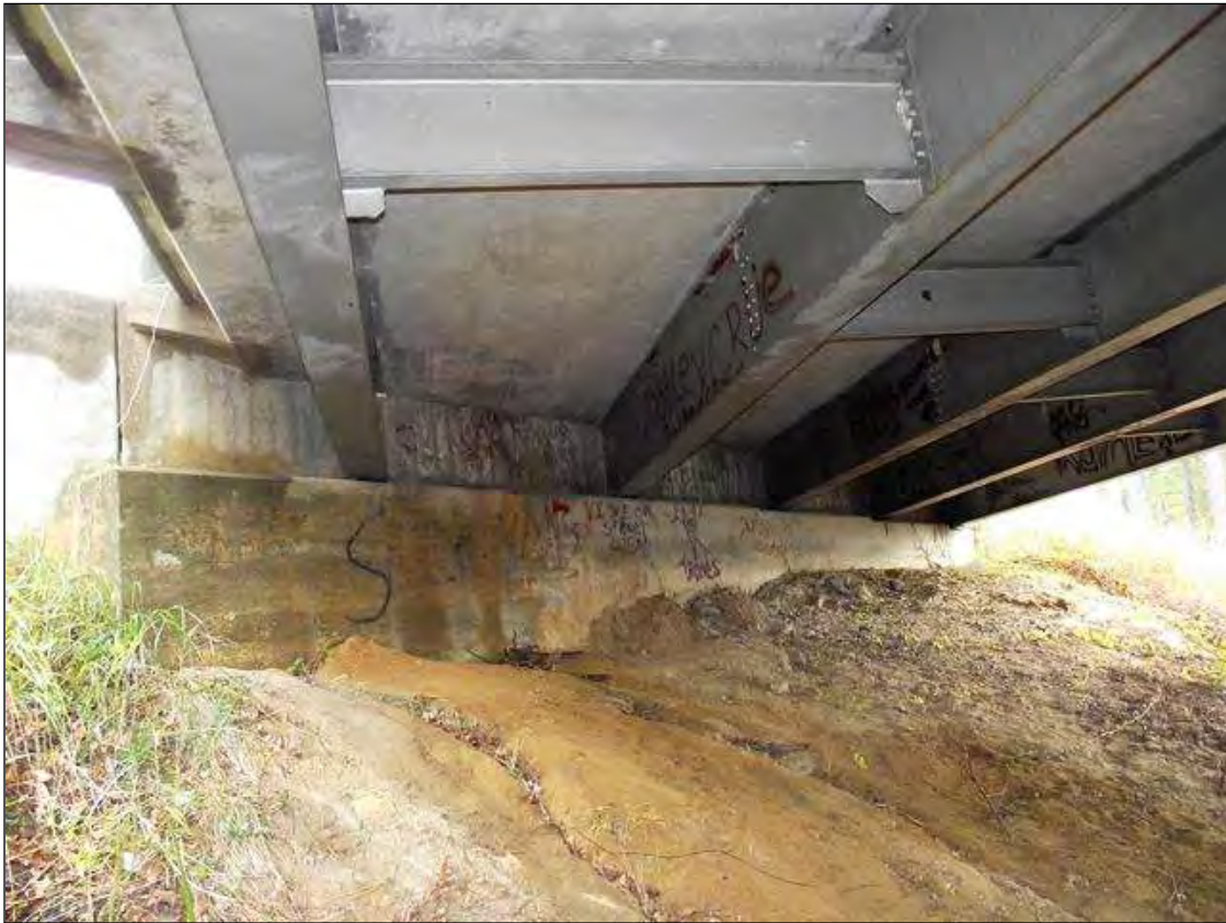
END BENT 2 OVERVIEW
