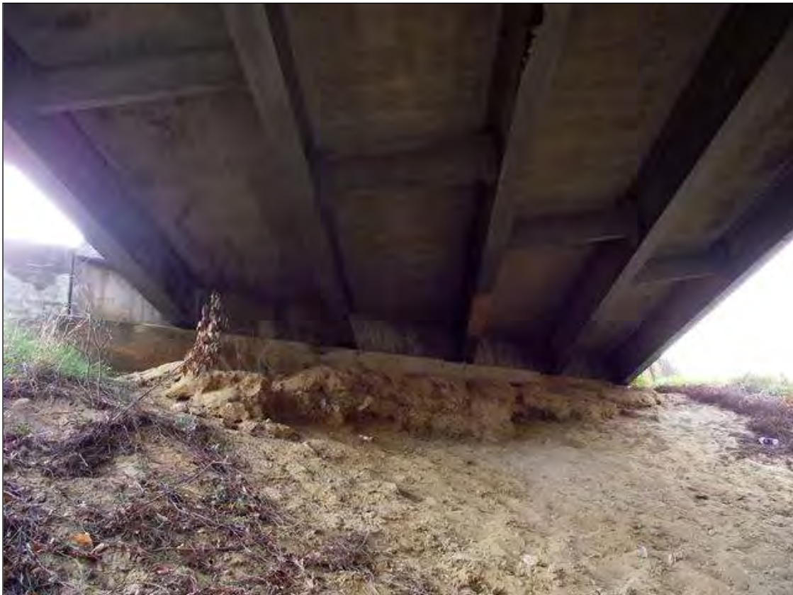
END BENT 1 OVERVIEW
