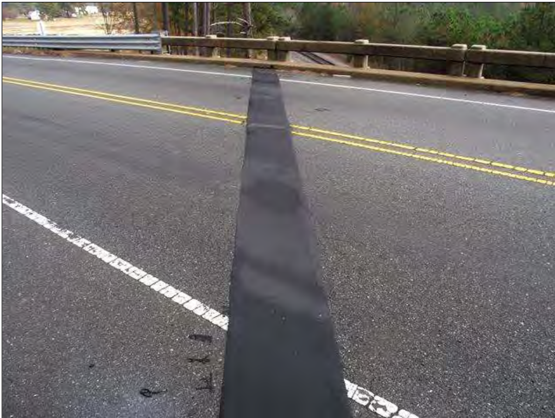
JOINT AT BENT 4
