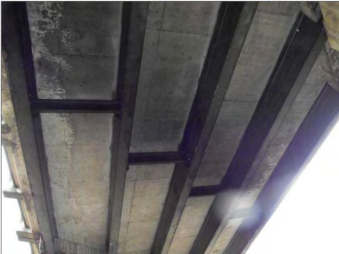
SUPERSTRUCTURE OVERVIEW - ALL SPANS SIMILAR
