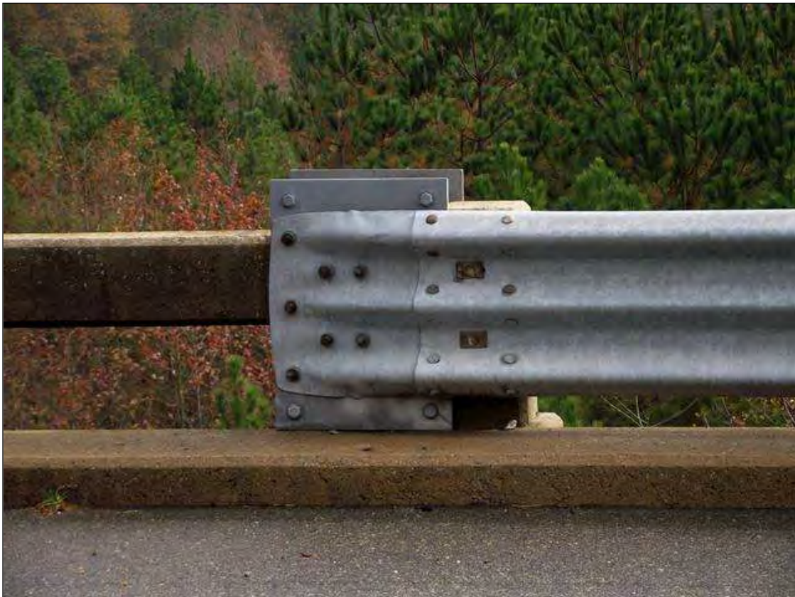
RIGHT SIDE GUARDRAIL CONNECTION IN SPAN 1
