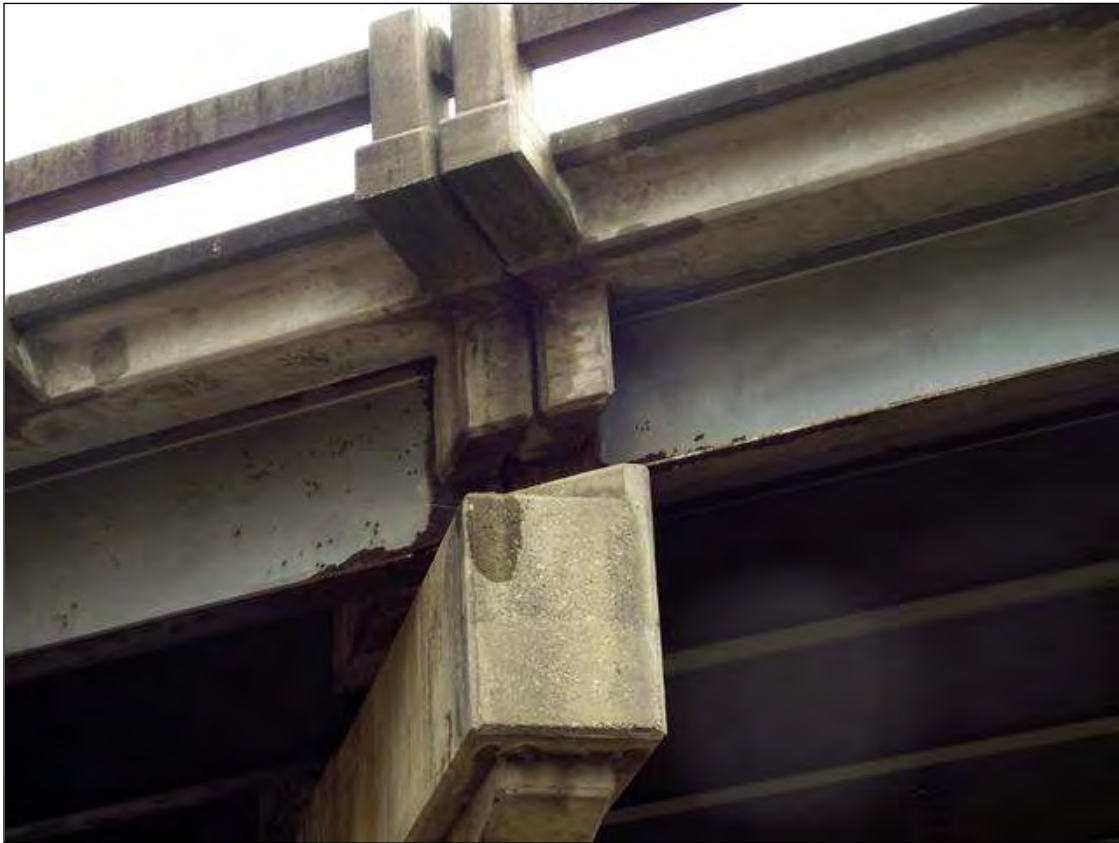
SUPERSTRUCTURE OVER END OF CAP AT BENT 2 - OTHER BENTS SIMILAR
