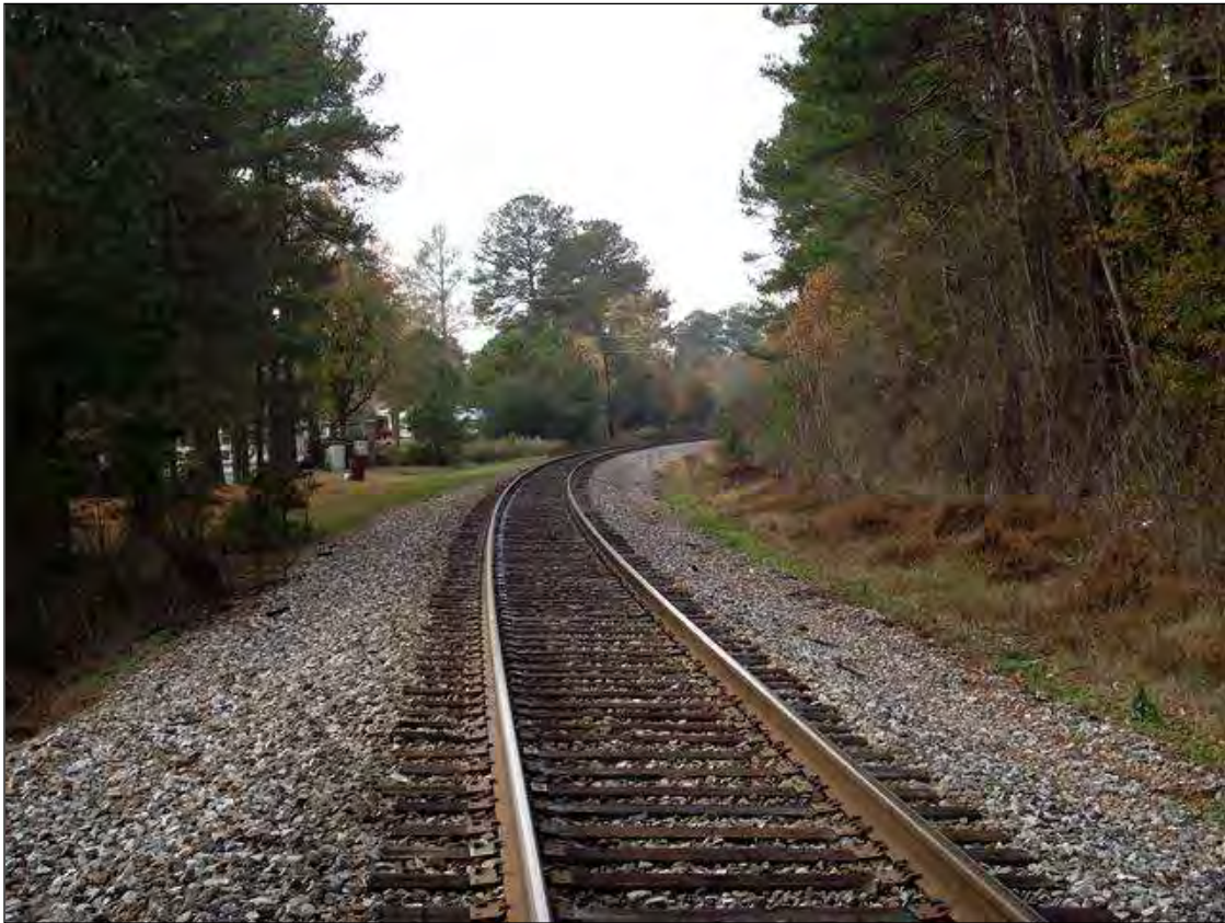
LOOKING WEST ALONG RAILROAD
