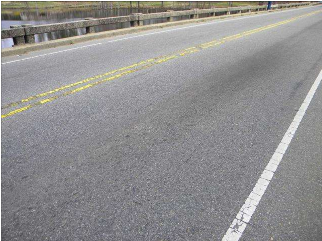
SPAN 1 OVERVIEW, OTHER SPANS SIMILAR
