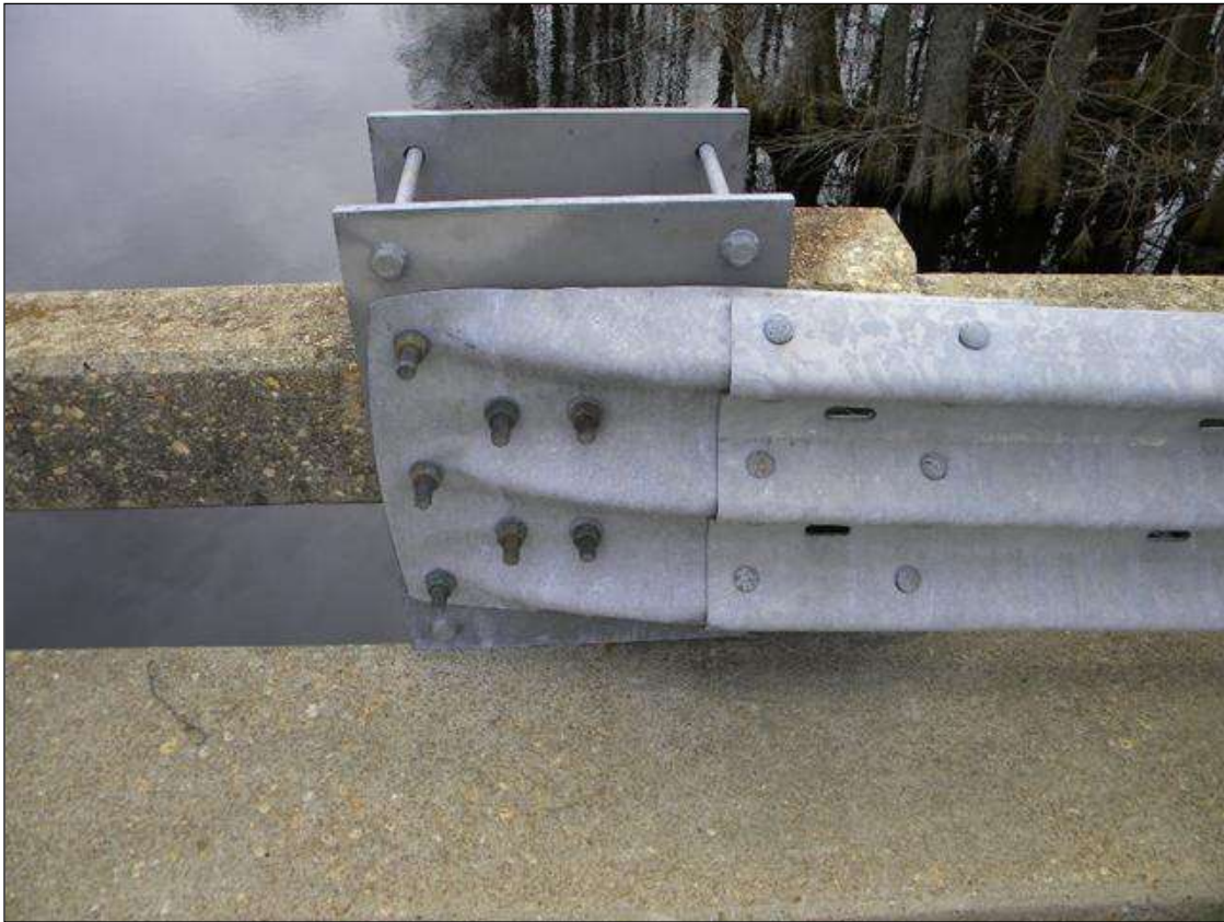
RIGHT SIDE GUARDRAIL CONNECTION IN SPAN 1
