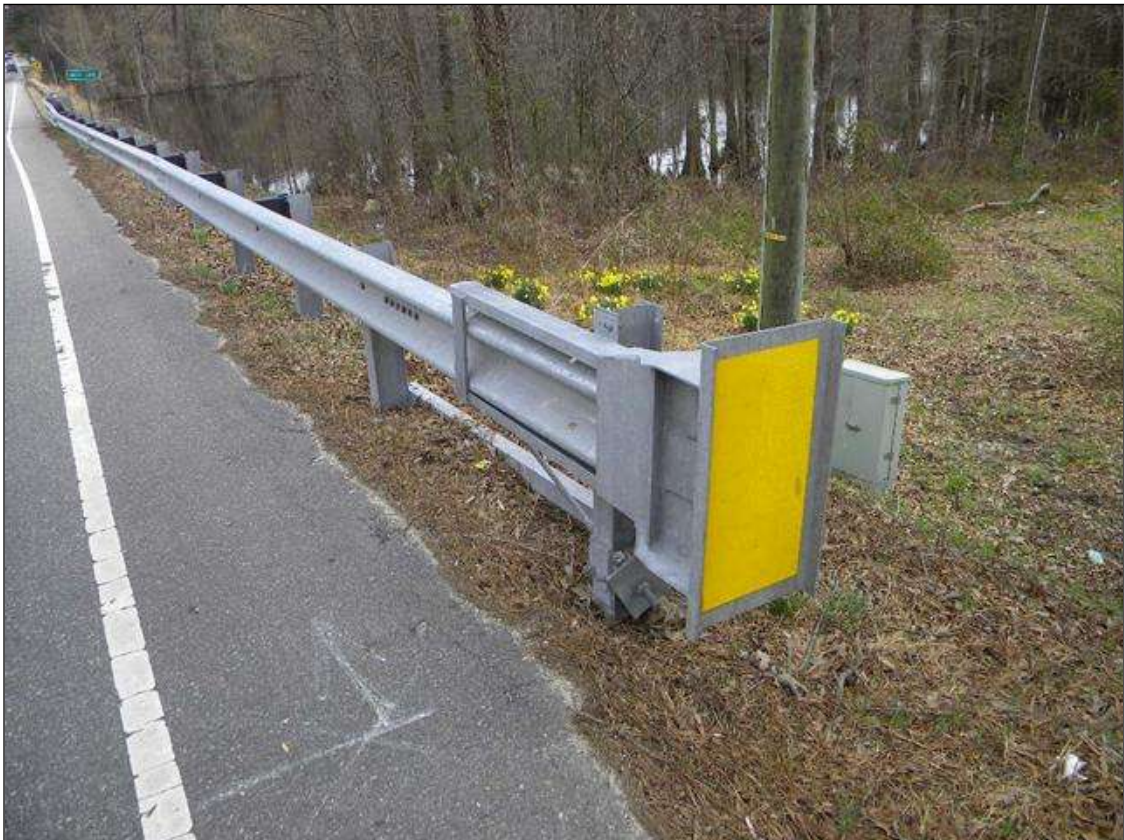
RIGHT SIDE GUARDRAIL TERMINAL END IN APPROACH 1, OTHERS SIMILAR
