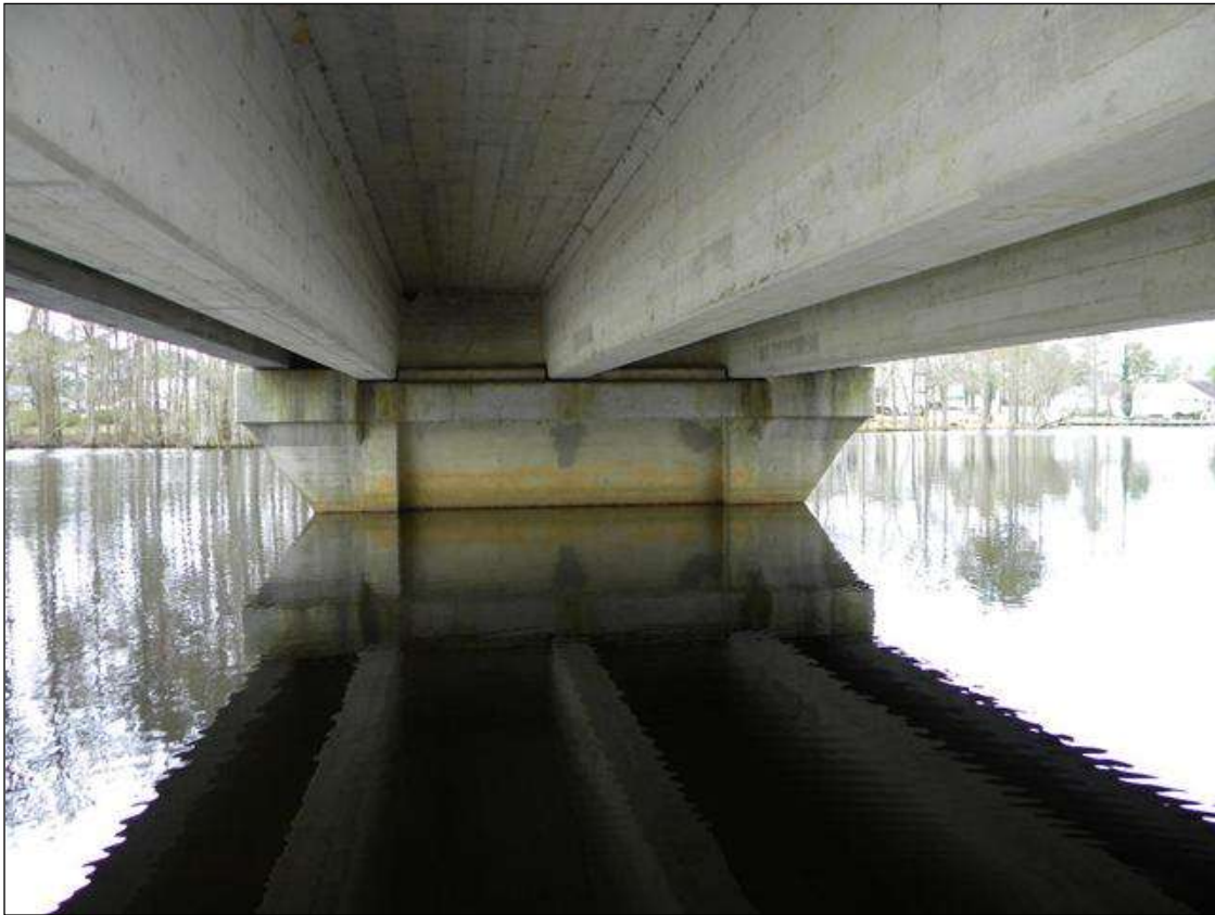
BENT 3 SPAN 4 SIDE
