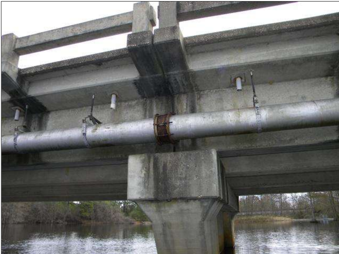
SUPERSTRUCTURE OVER END OF CAP
