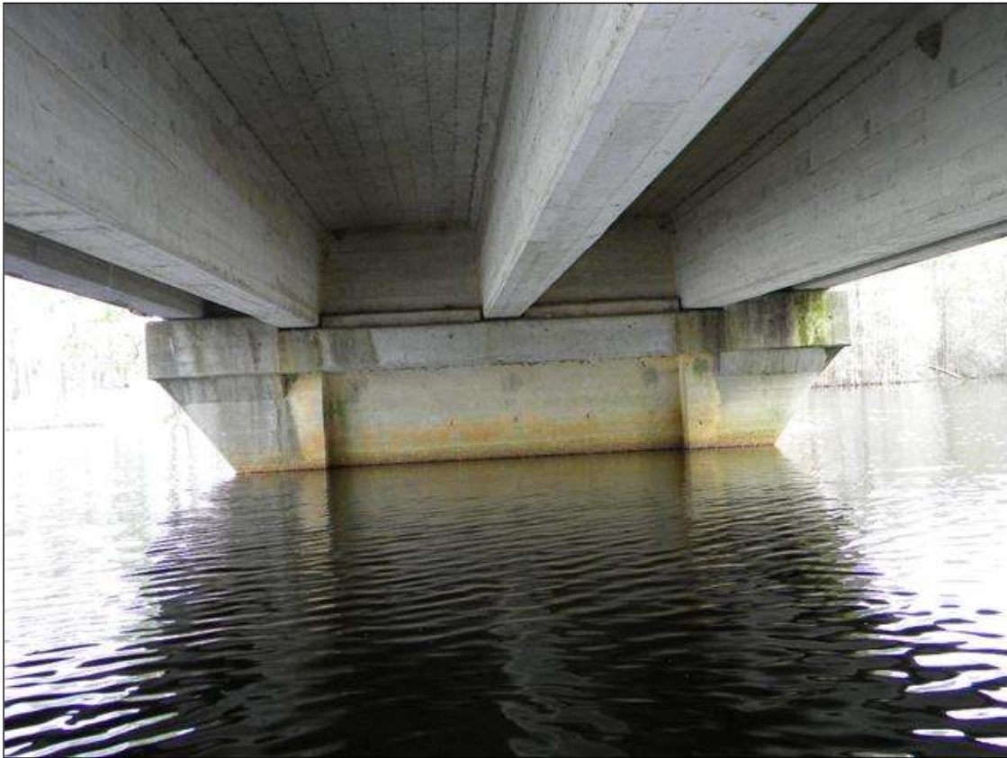
BENT 1 SPAN 1 SIDE
