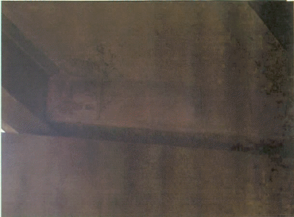
BT-1, SP-2; DIAPH IN BAY-4 HAS HORIZ CRK TO 1/16" ALONG LOWER EDGE
