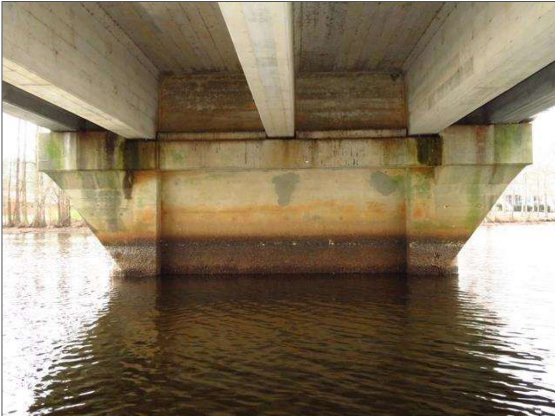
BENT 3 SPAN 4 SIDE
