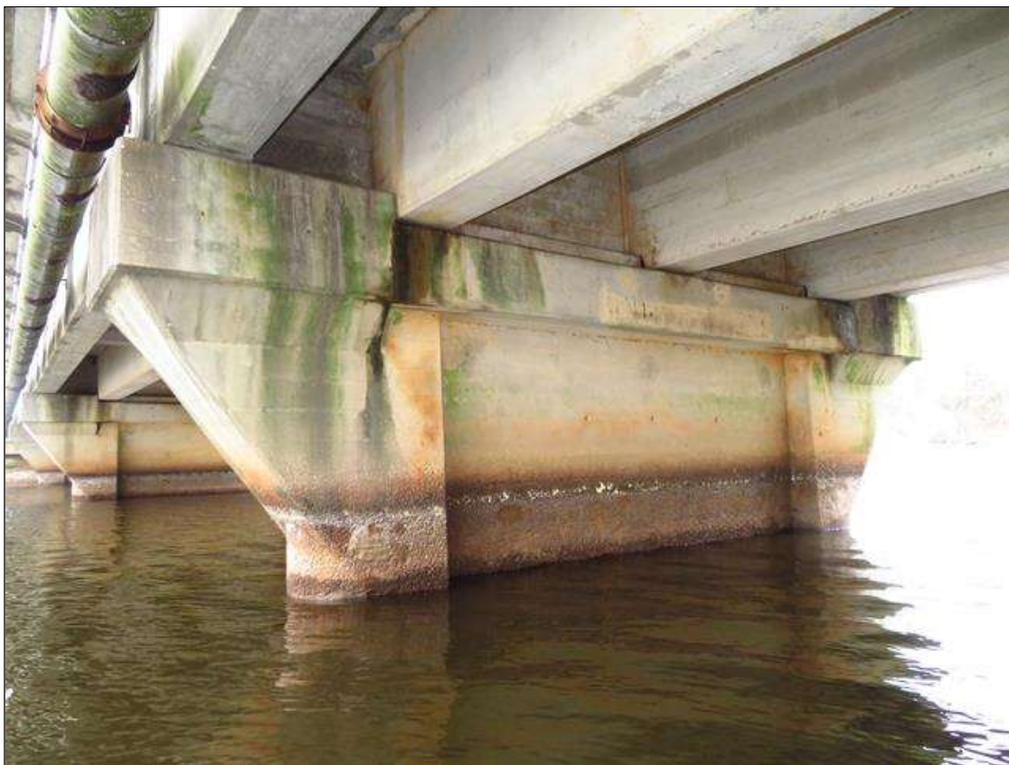
BENT 1 SPAN 1 SIDE
