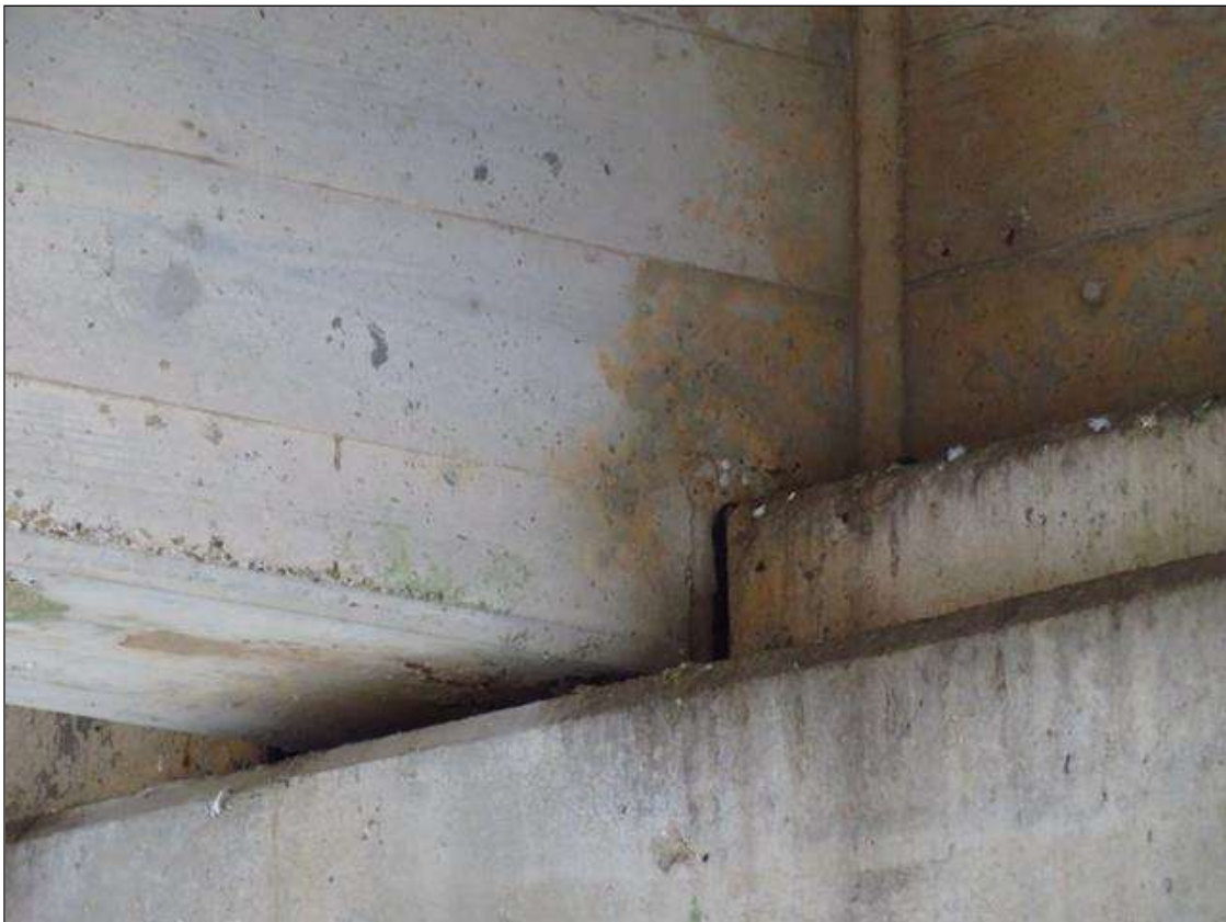
TYPICAL GIRDER SEAT/BEARING AREA AT THE INTERIOR BENT
