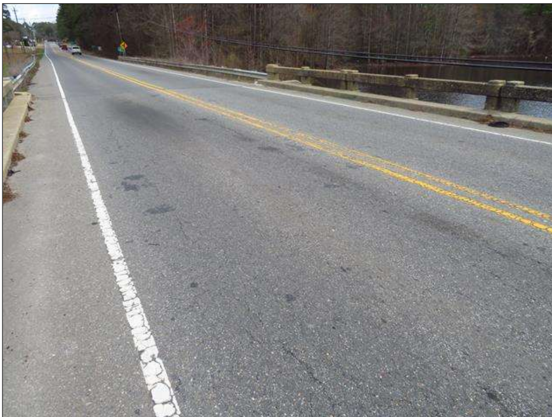
SPAN 4 WEARING SURFACE OVERVIEW
