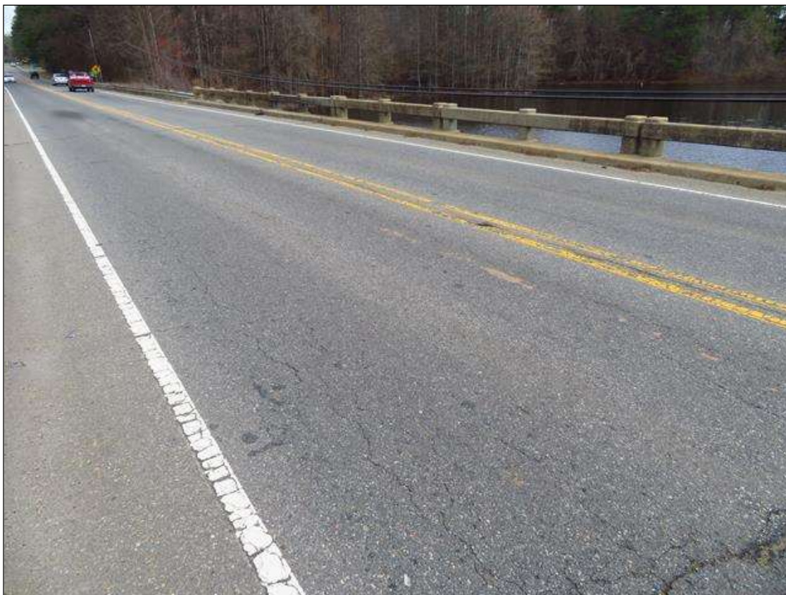
SPAN 3 WEARING SURFACE OVERVIEW
