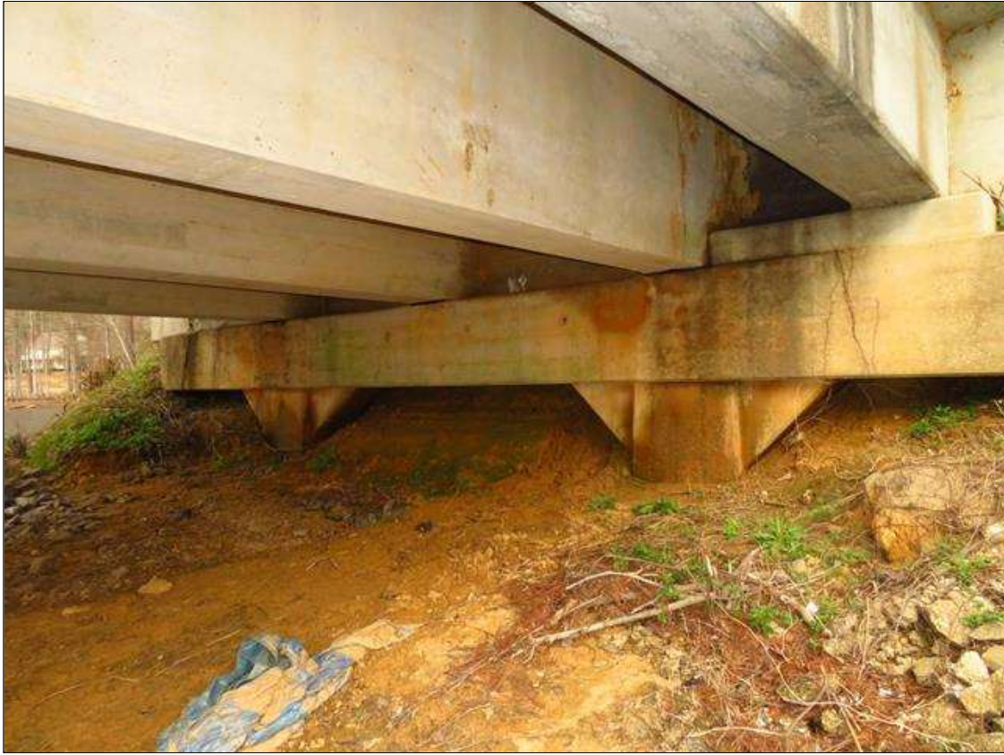
END BENT 2 OVERVIEW
