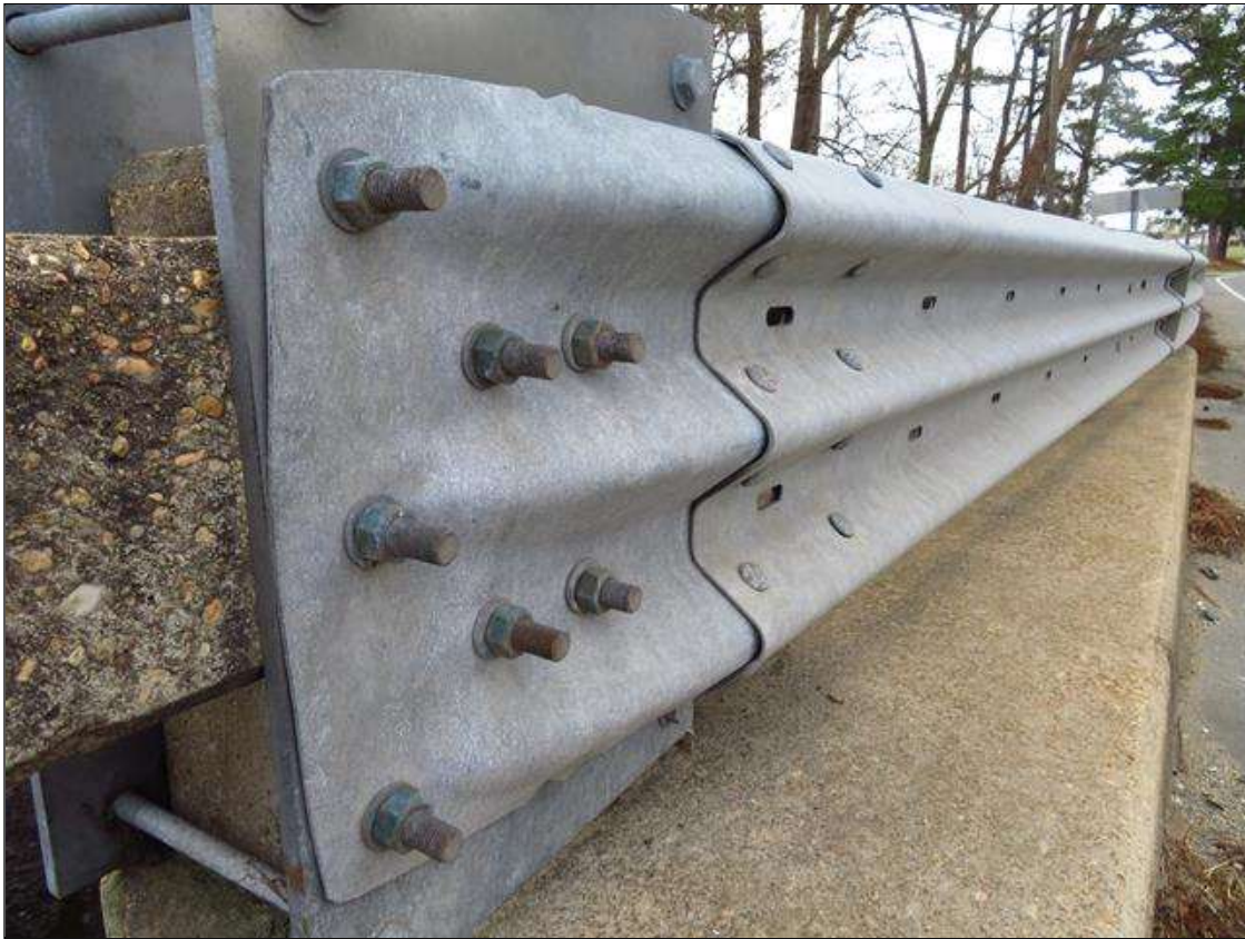
APPROACH GUARDRAIL CONNECTION
