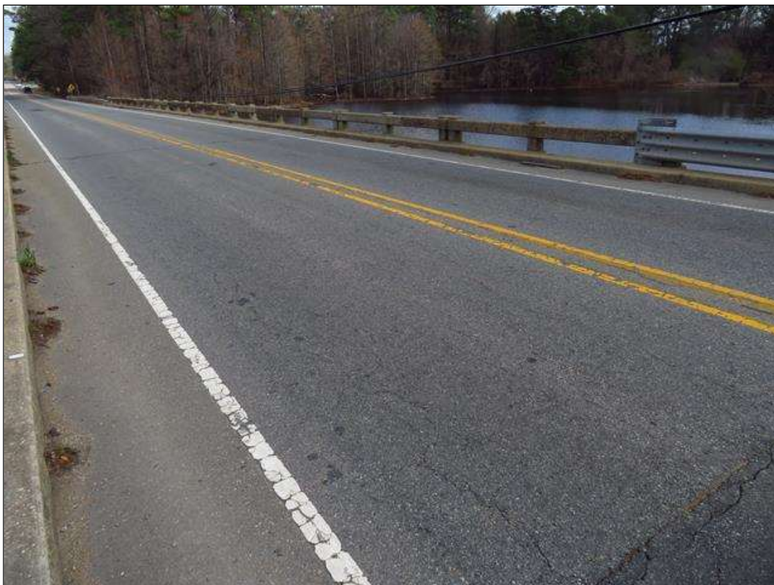
SPAN 1 WEARING SURFACE OVERVIEW
