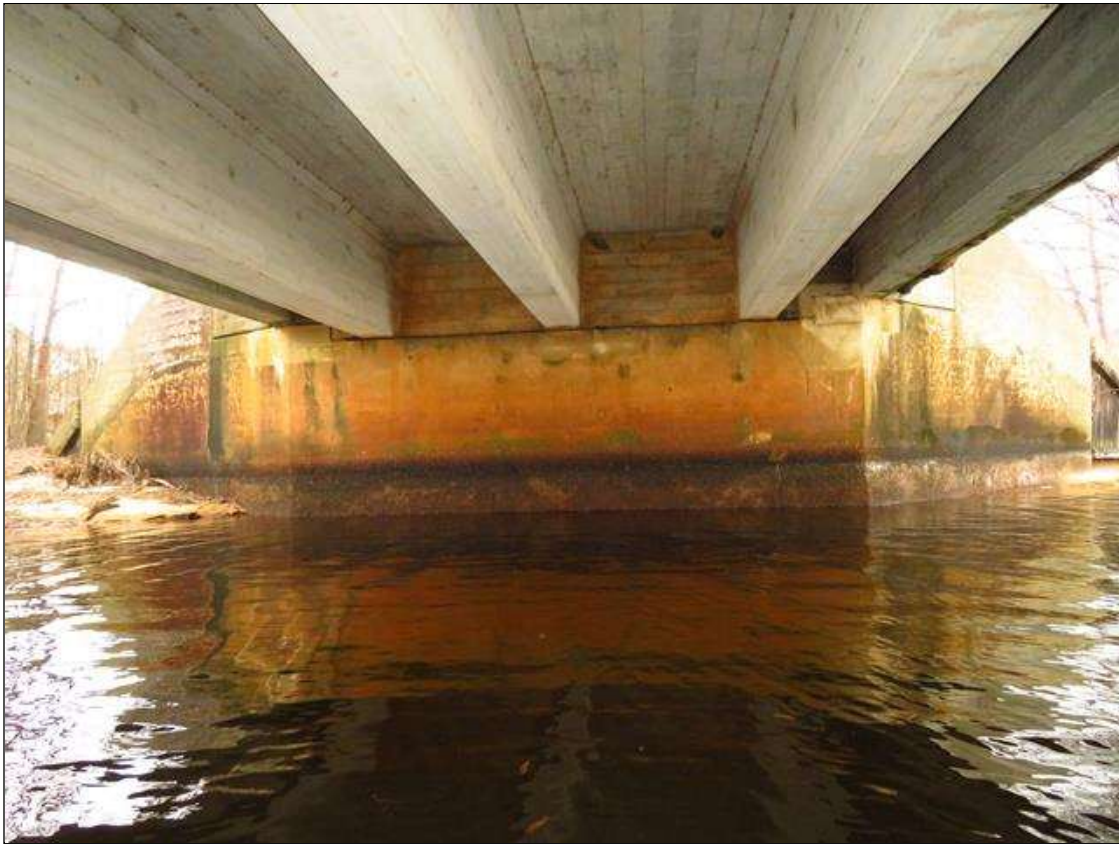
END BENT 1 OVERVIEW
