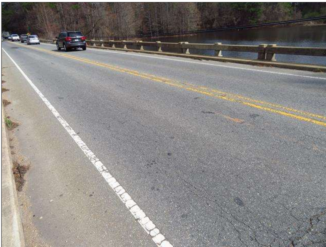
SPAN 2 WEARING SURFACE OVERVIEW
