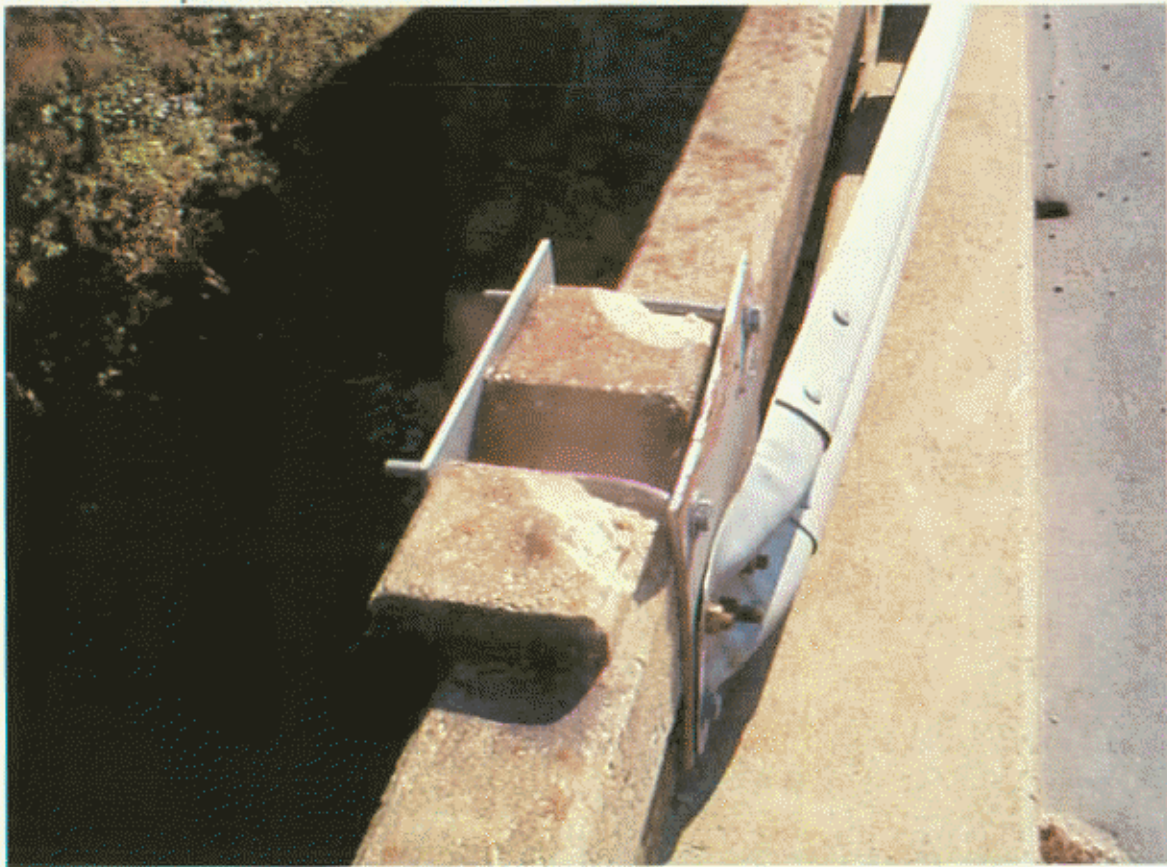
N.W. APPROACH RAIL
