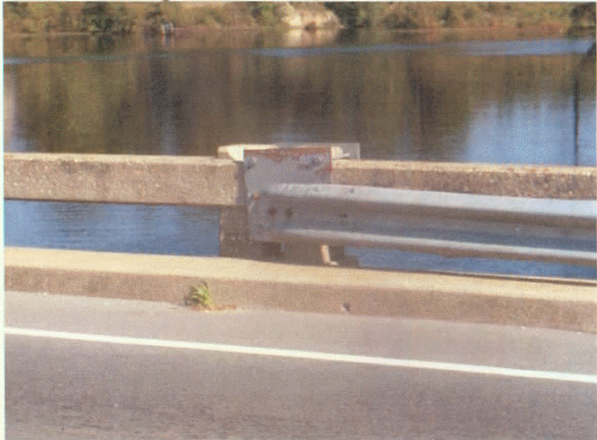
WEST SIDE DRAINAGE
