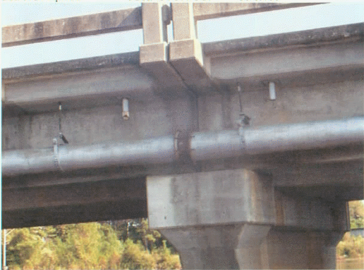
WEST END OF BENT 3
