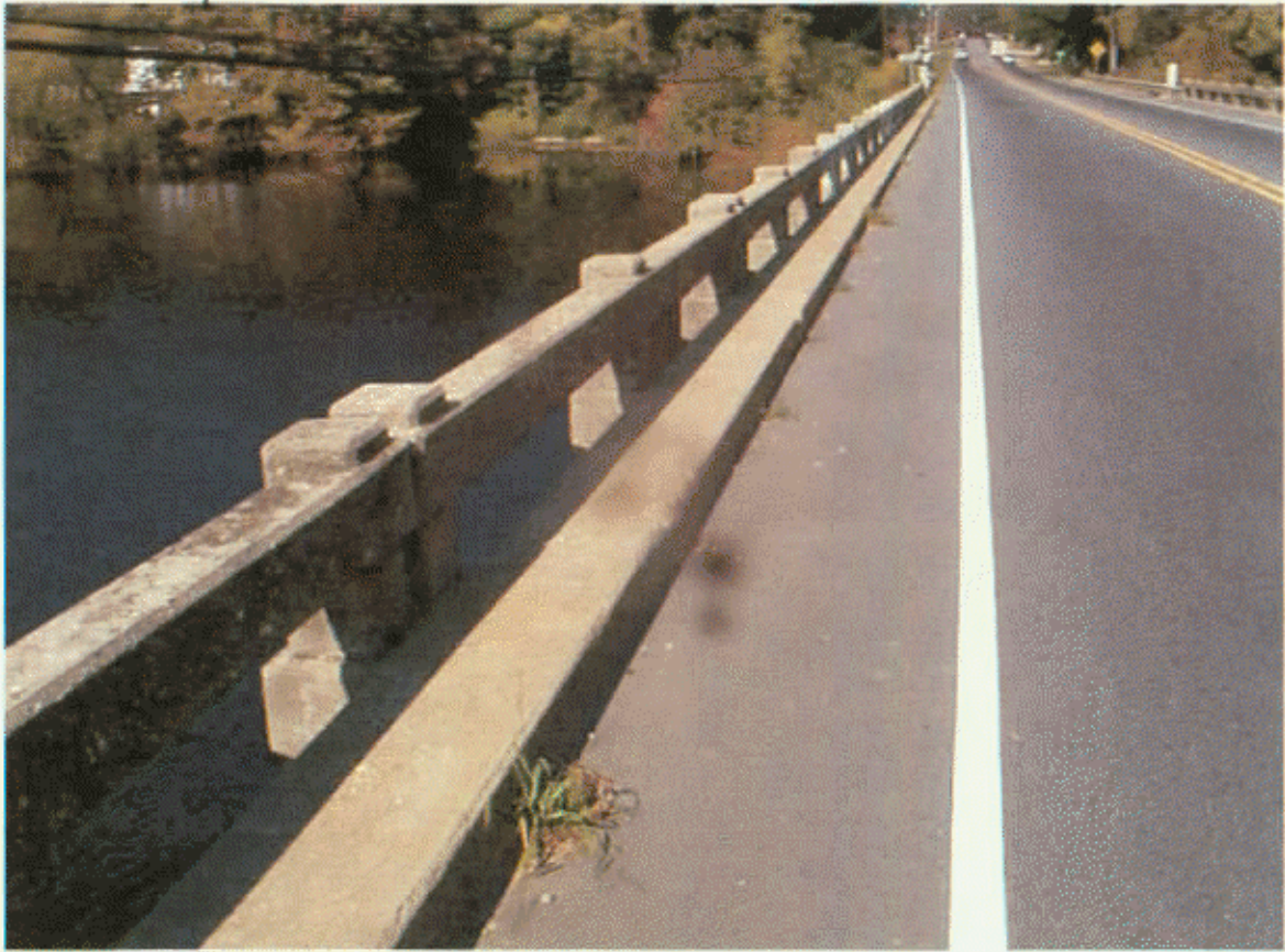
DRAINAGE ALONG WEST CURB
