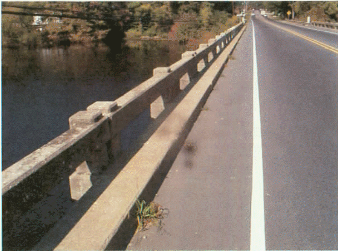
DRAINAGE ALONG WEST CURB
