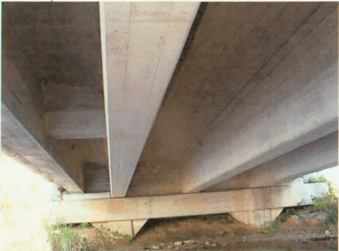
SPAN 2 UNDERSIDE (ALL SPANS SIMILAR)
