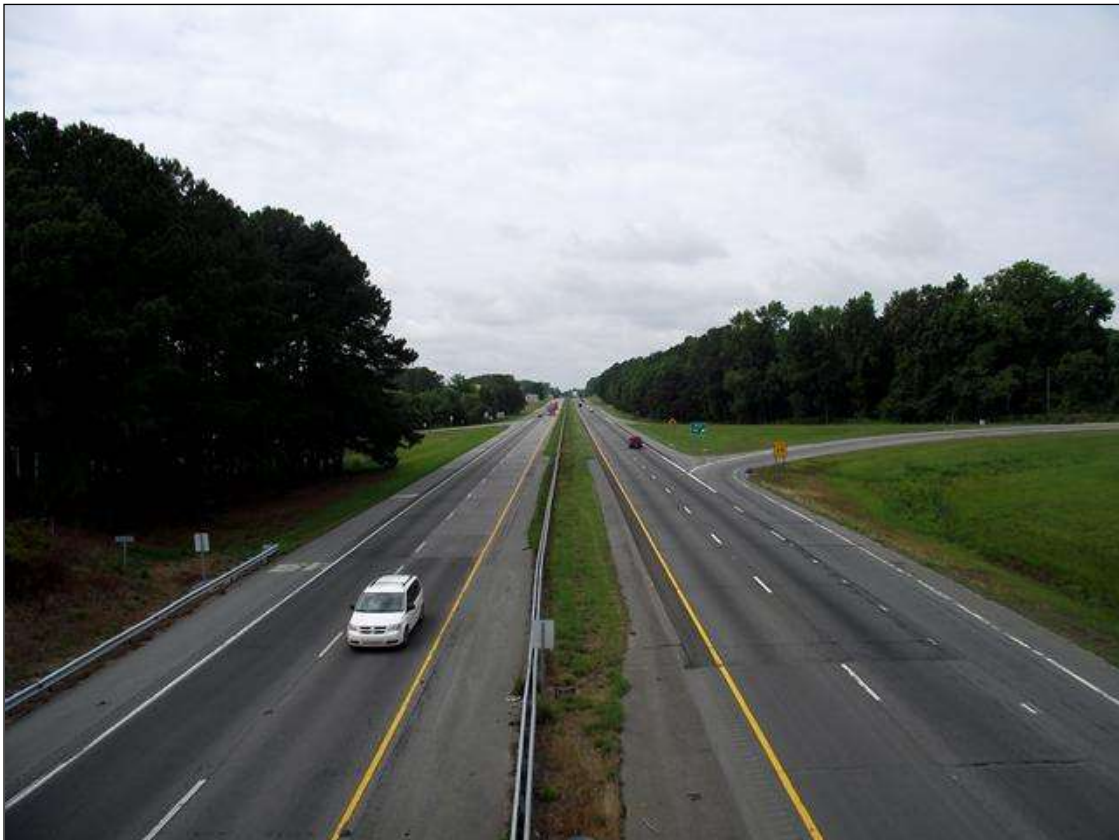
LOOKING SOUTH ALONG I-95
