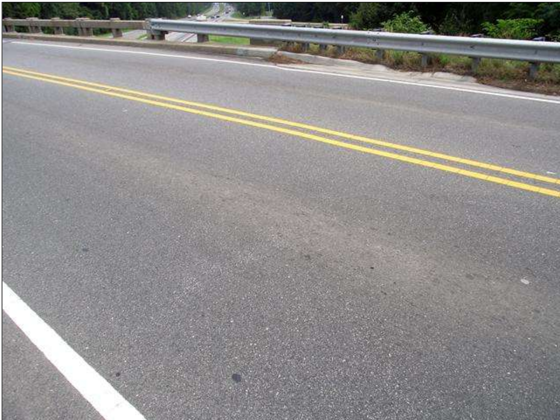
WEARING SURFACE OVER END BENT 1
