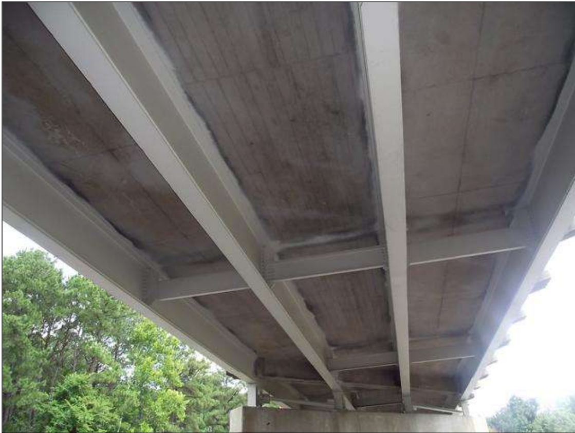
SUPERSTRUCTURE OVERVIEW - ALL SPANS SIMILAR
