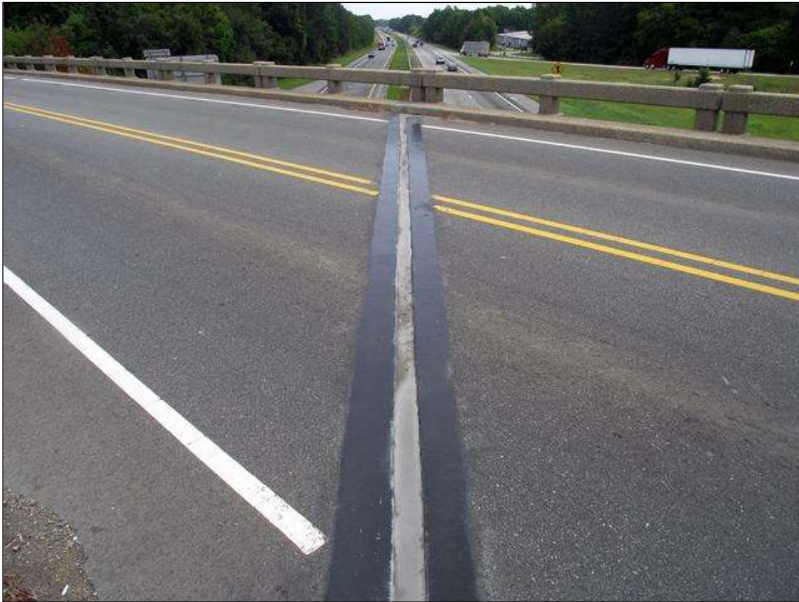
JOINT AT BENT 2
