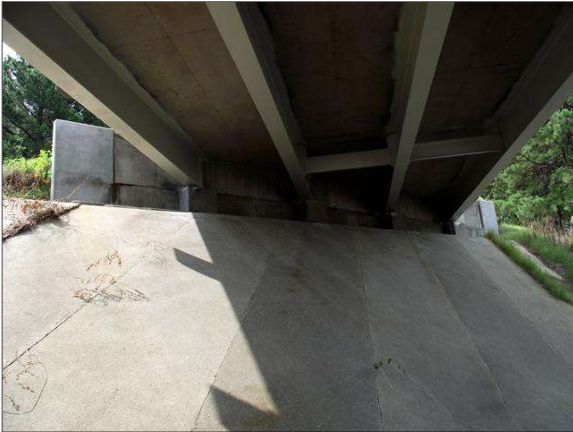
END BENT 1 OVERVIEW
