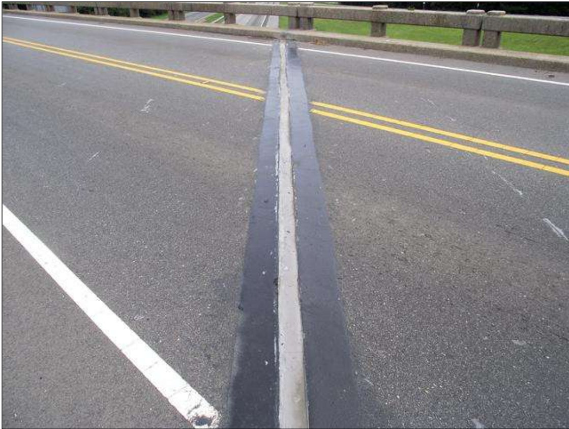
JOINT AT BENT 1
