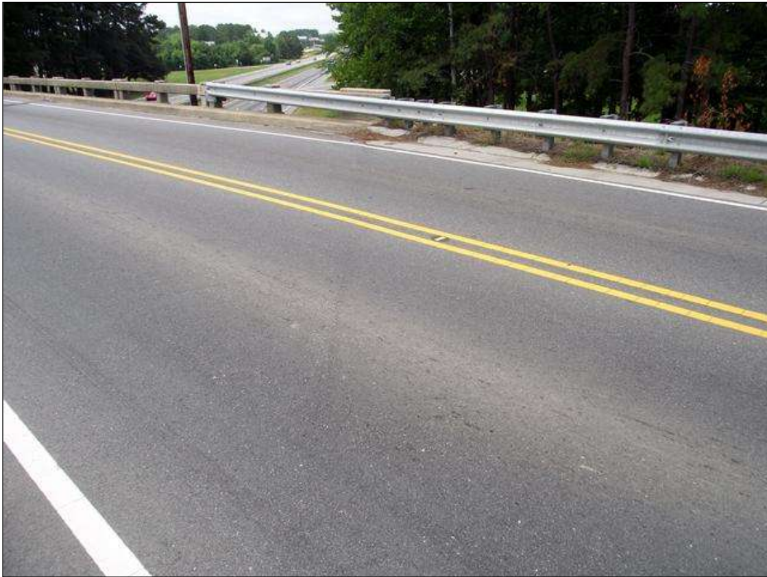
WEARING SURFACE OVER END BENT 2
