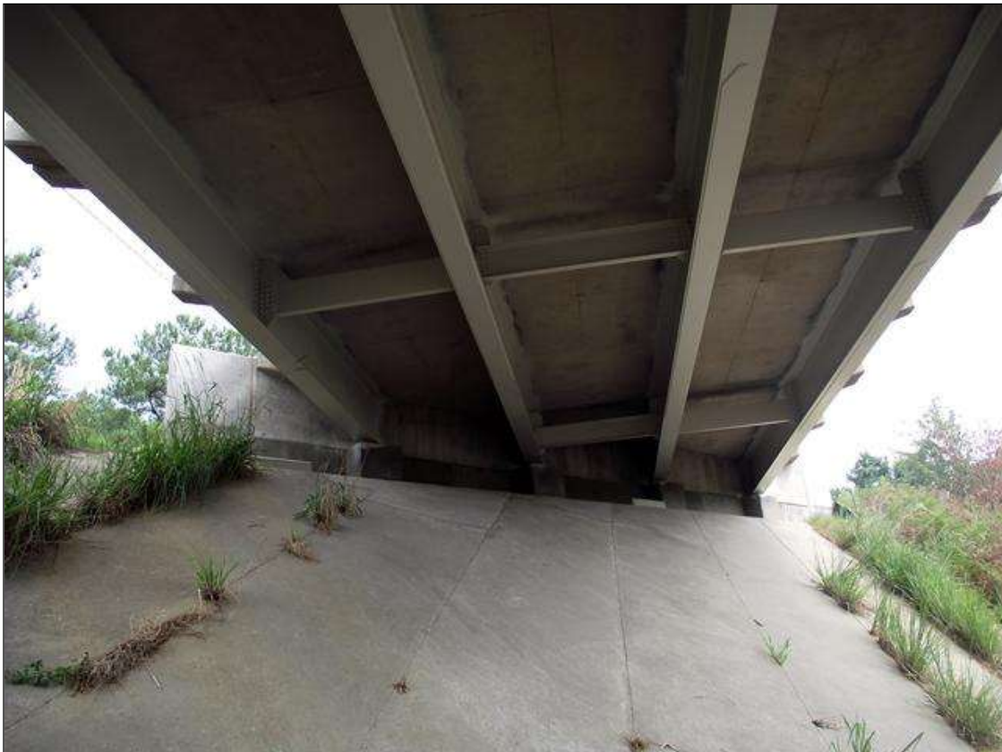
END BENT 2 OVERVIEW
