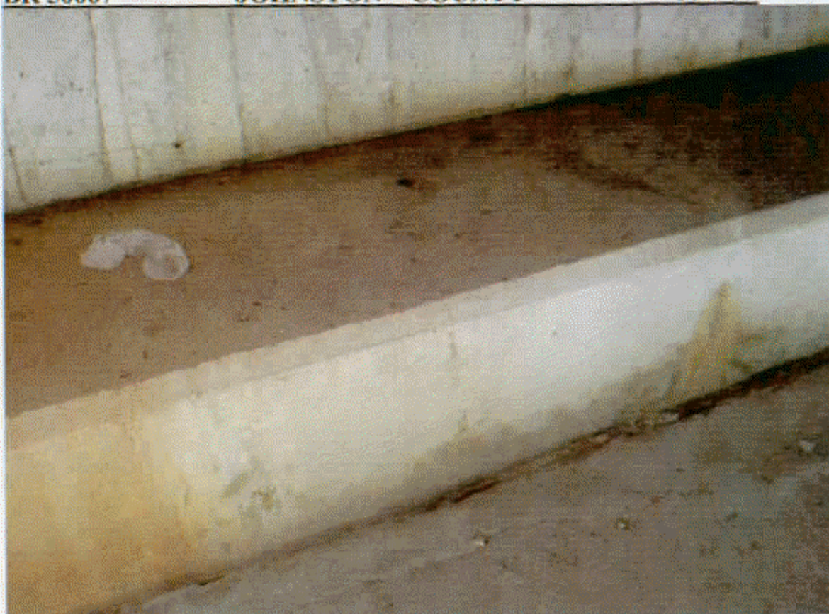
EB 1, BAY 3, CAP HAS H/L CRS ACROSS TOP AND DOWN FACE
