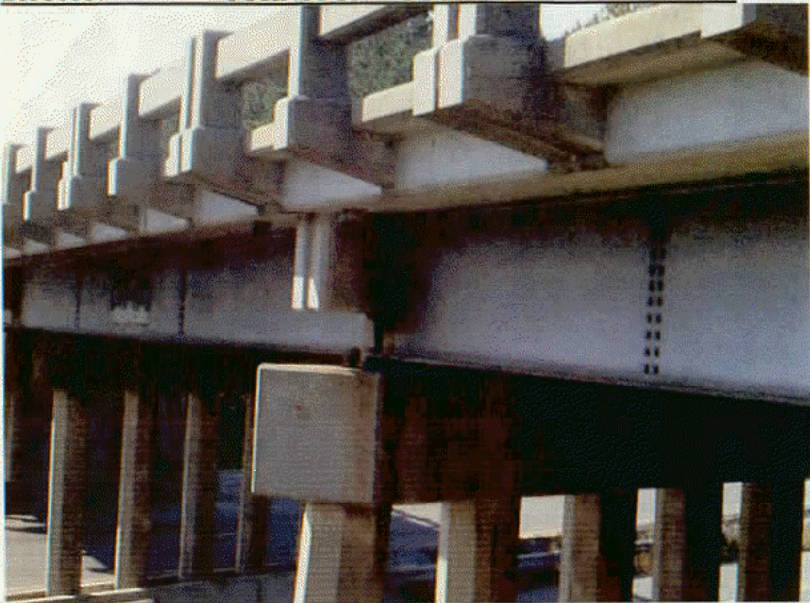
BT 1, RT END OF CAP HAS FEW VERT H/L CRS
