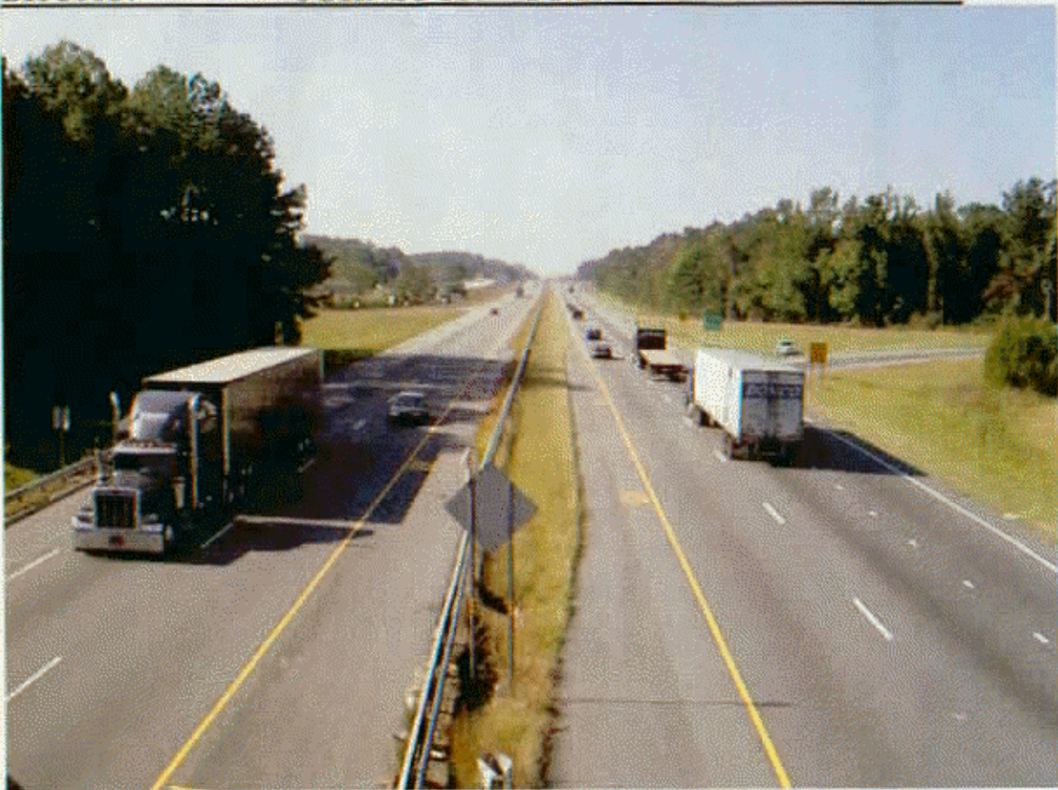
LOOKING WEST AT RAMPS
