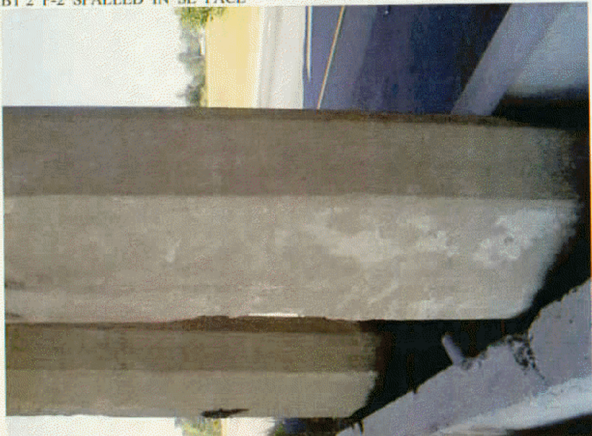
BT 2, P-2 HAS HORIZ. H/L CRS IN EAST FACE
