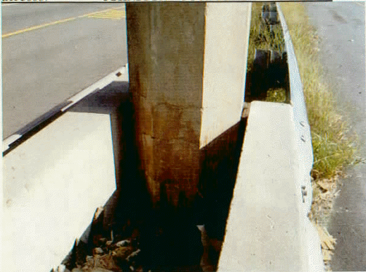
BT 2 P-7 HAS HORIZ CRS IN W FACE
