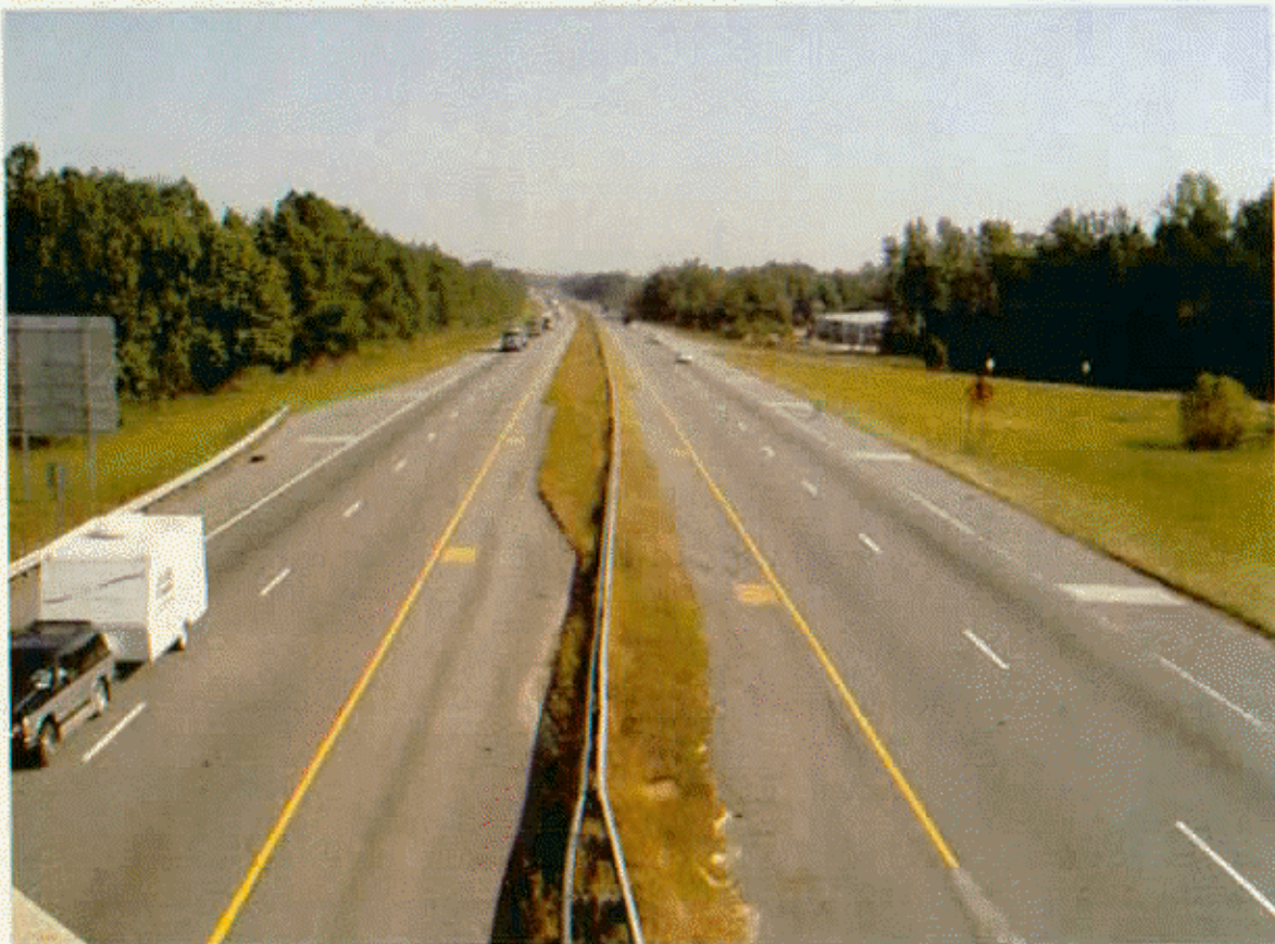
LOOKING EAST AT RAMPS
