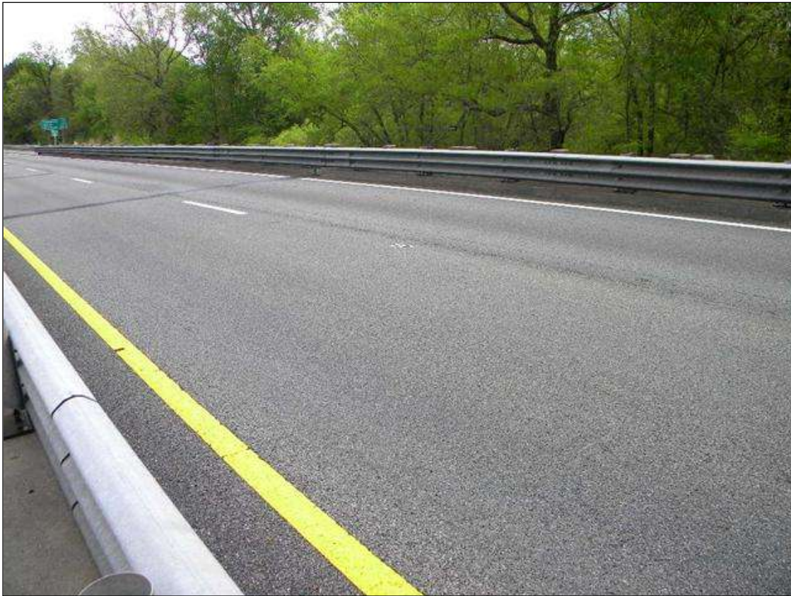
SPAN 1 OVERVIEW, OTHER SPANS SIMILAR
