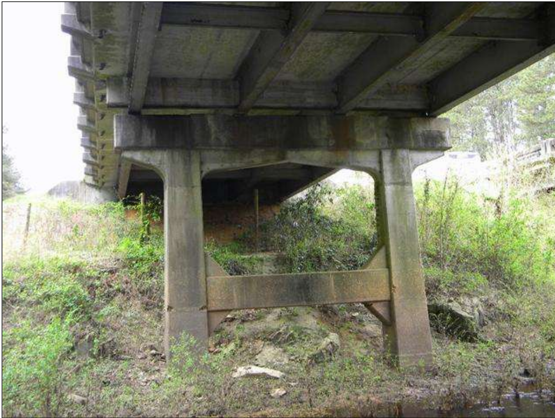
BENT 1 SPAN 2 SIDE
