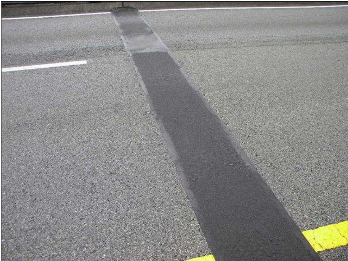
JOINT AT BENT 3
