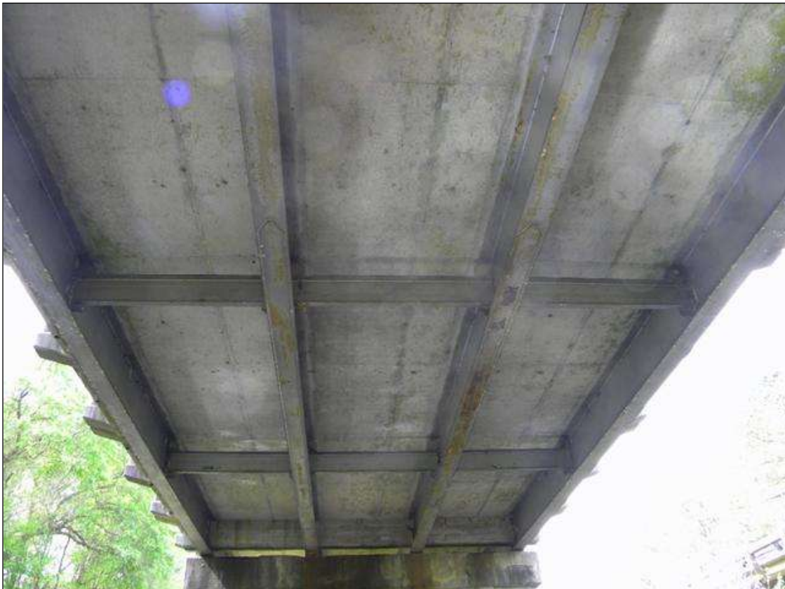
SUPERSTRUCTURE OVERVIEW, ALL SPANS SIMILAR
