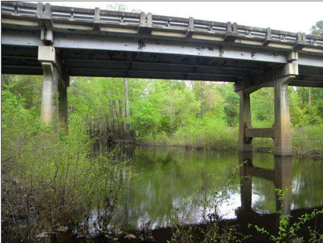
LOOKING WEST UPSTREAM UNDER THE SOUTHBOUND STRUCTURE
