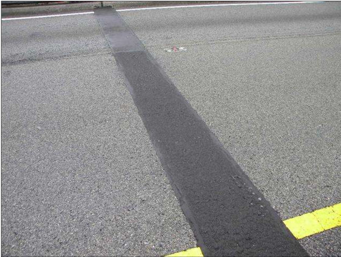
JOINT AT BENT 2
