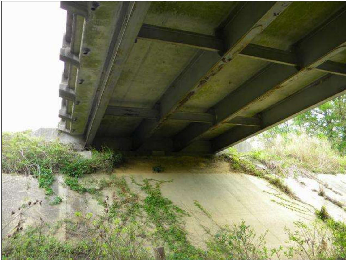
END BENT 2 OVERVIEW
