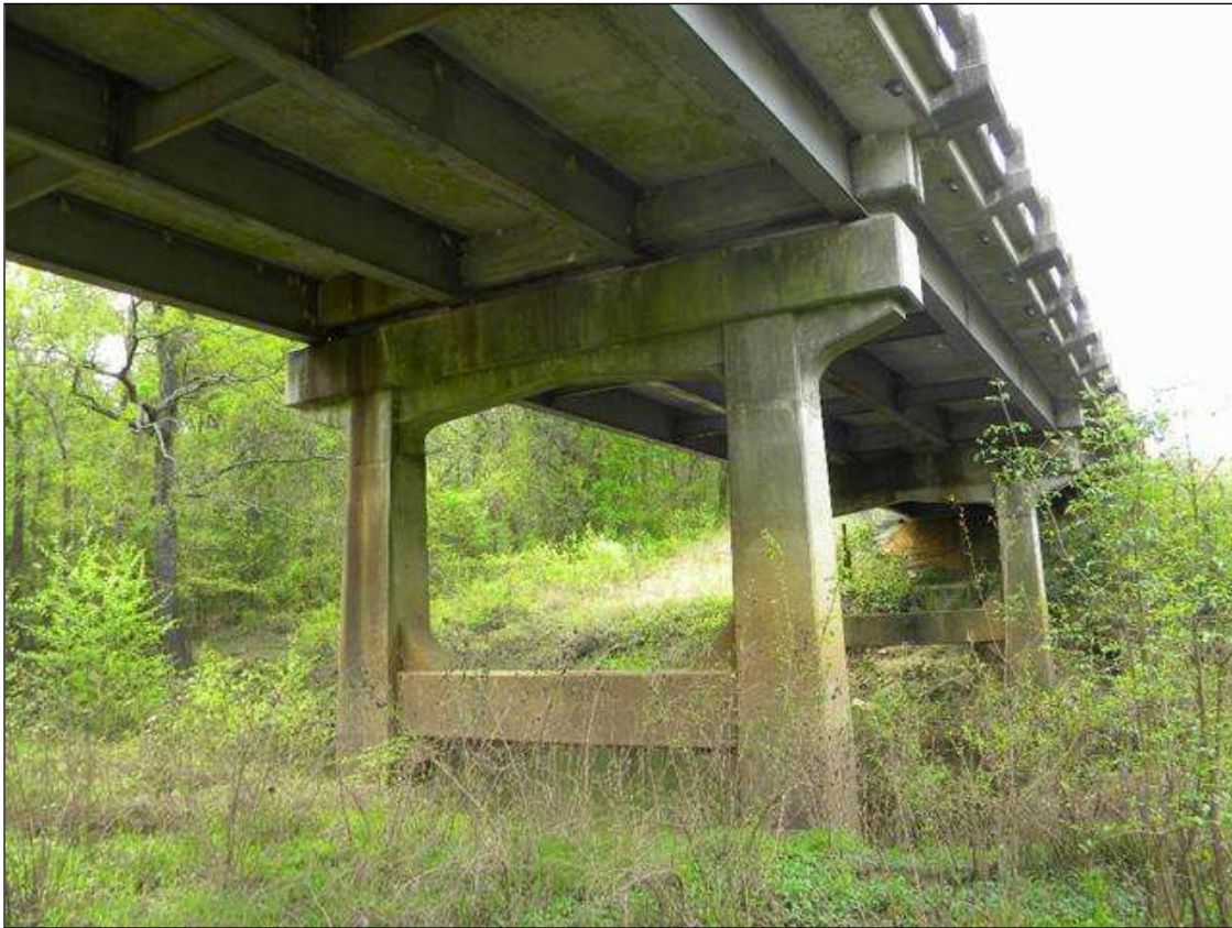
BENT 2 SPAN 3 SIDE
