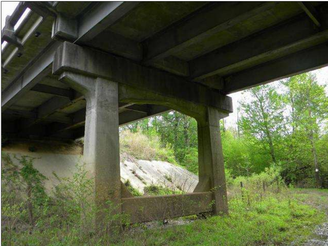
BENT 3 SPAN 3 SIDE
