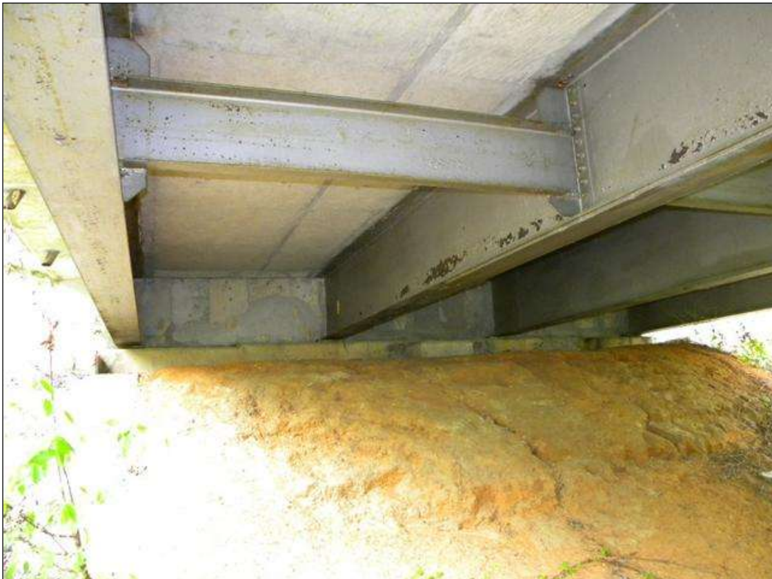
END BENT 1 OVERVIEW
