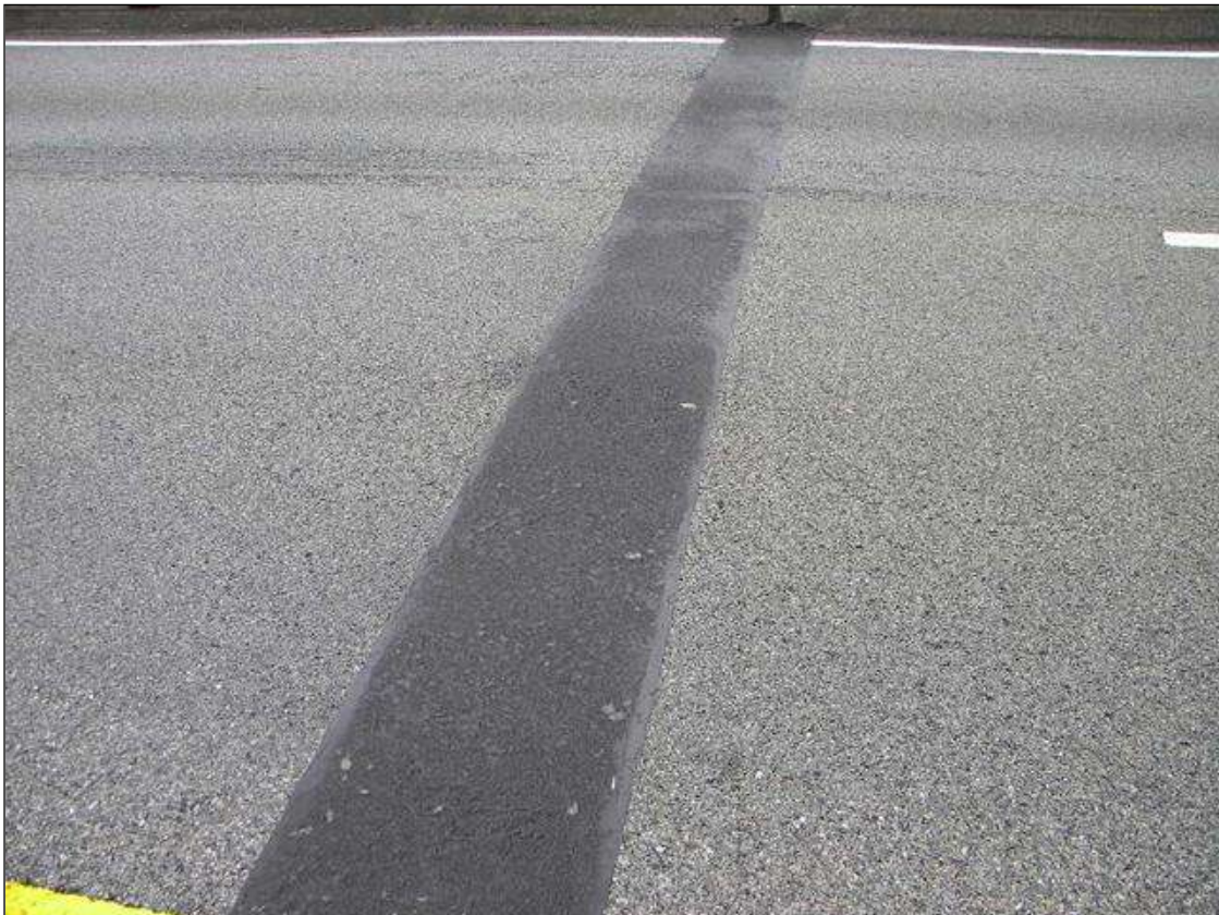
JOINT AT BENT 1
