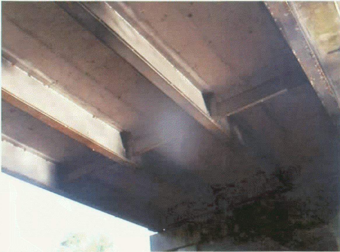
SPAN 2 UNDERSIDE. (ALL SPANS SIMILAR)
