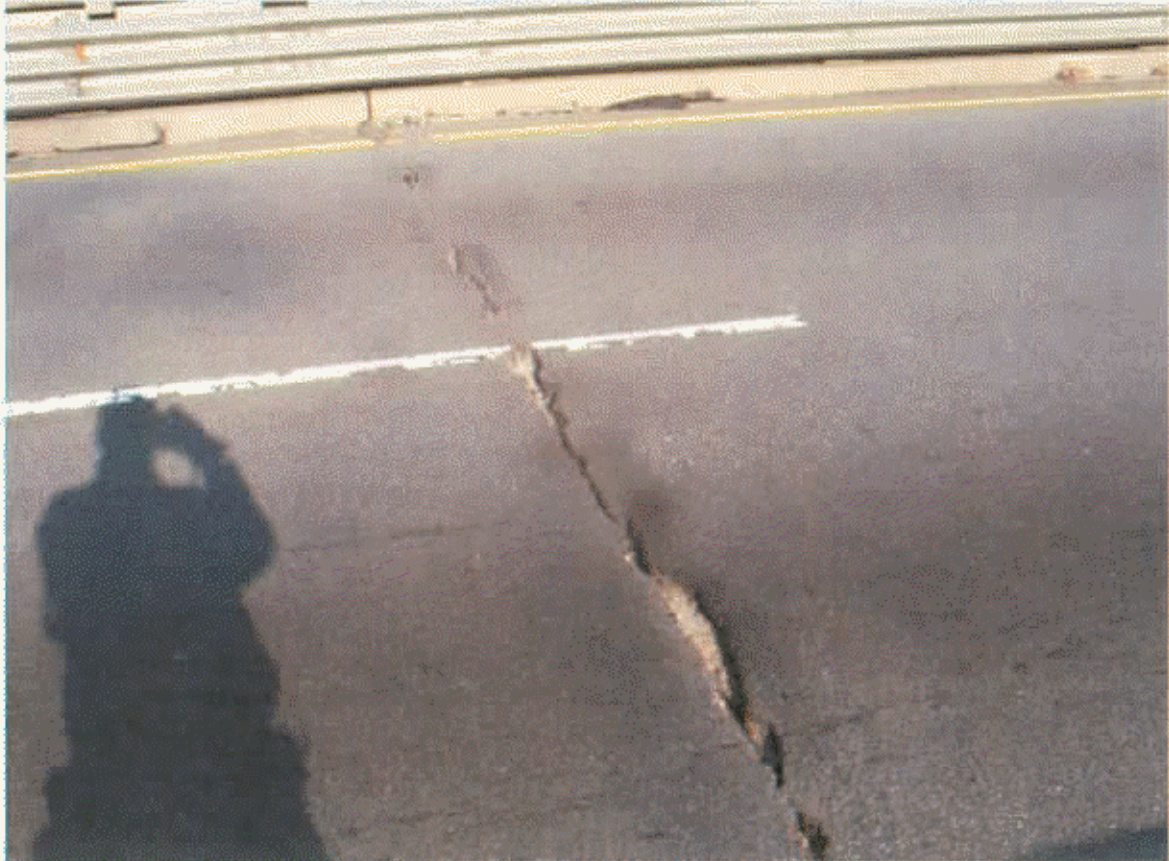
ASPHALT WEARING SURFACE AT BENT 3 JOINT
