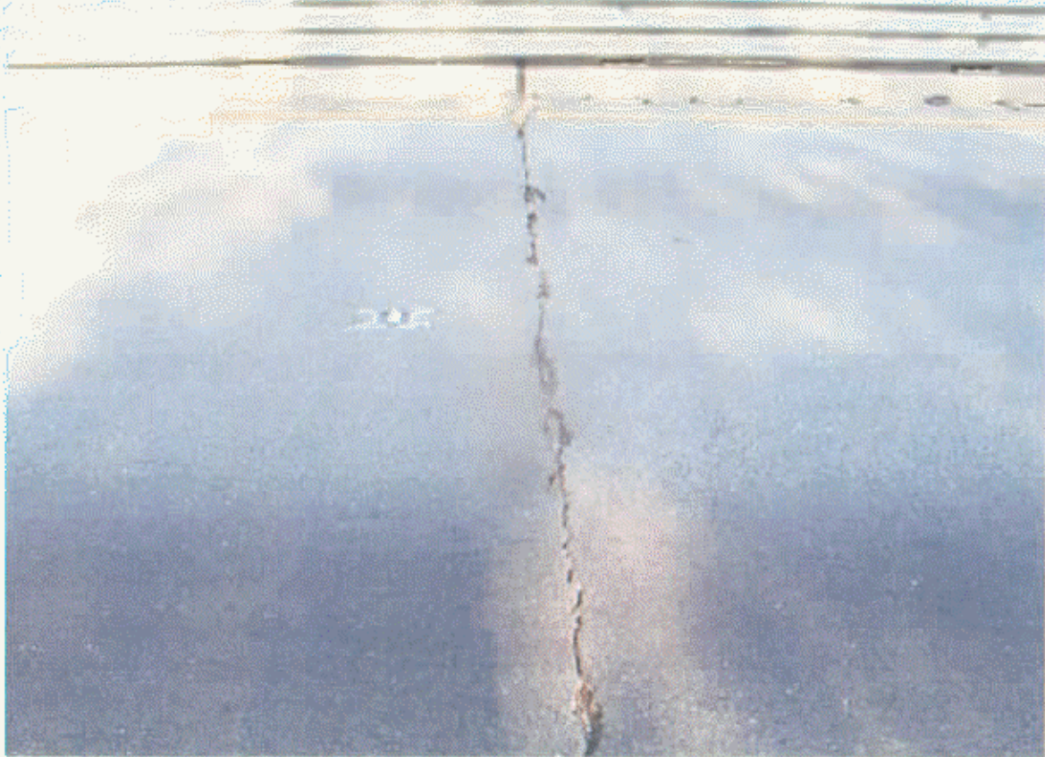
ASPHALT WEARING SURFACE AT BENT 1 JOINT
