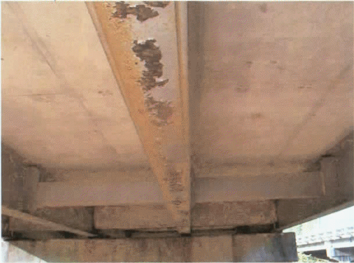
BEAM 2, SPAN 4 PAINT CONDITION SIMILAR
