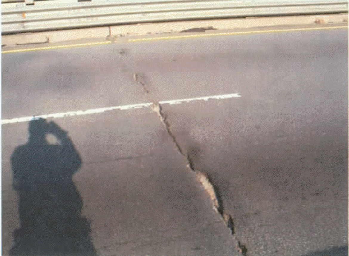
ASPHALT WEARING SURFACE AT BENT 3 JOINT
