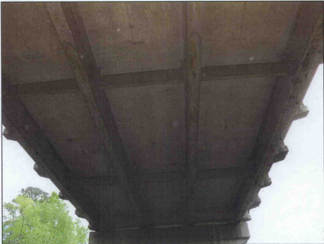
SUPERSTRUCTURE OVERVIEW, ALL SPANS SIMILAR
