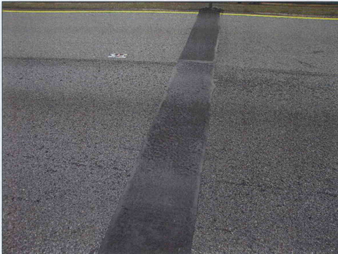
JOINT AT BENT 1
