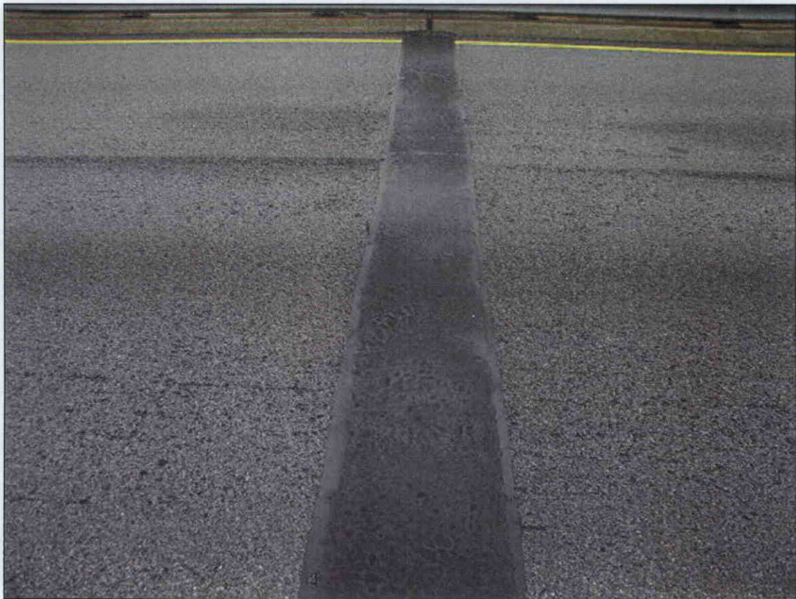
JOINT AT BENT 2
