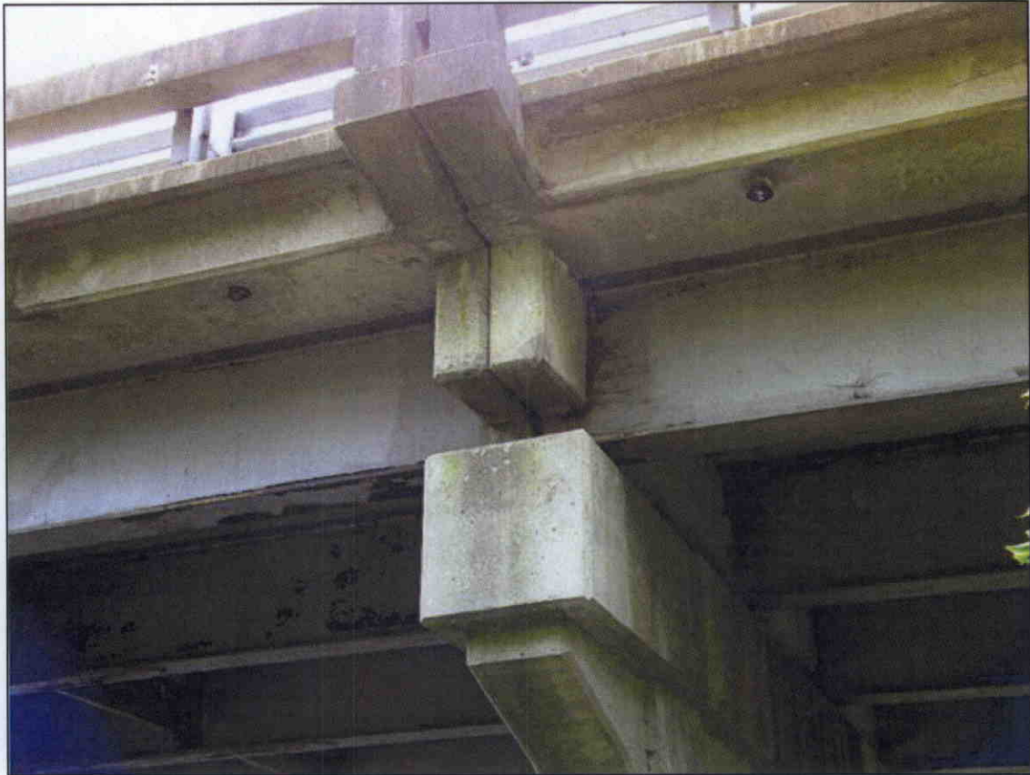
SUPERSTRUCTURE OVER BENT 1 END OF CAP, OTHER BENTS SIMILAR
