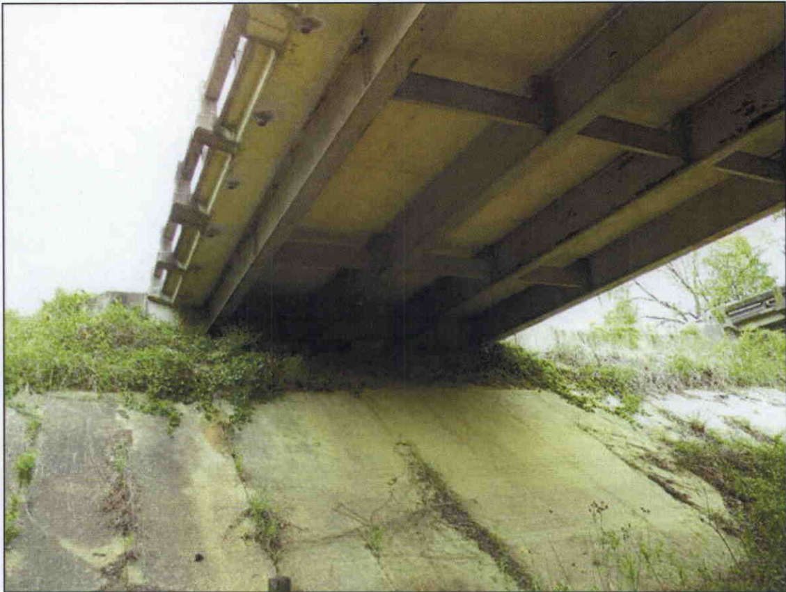
END BENT 2 OVERVIEW
