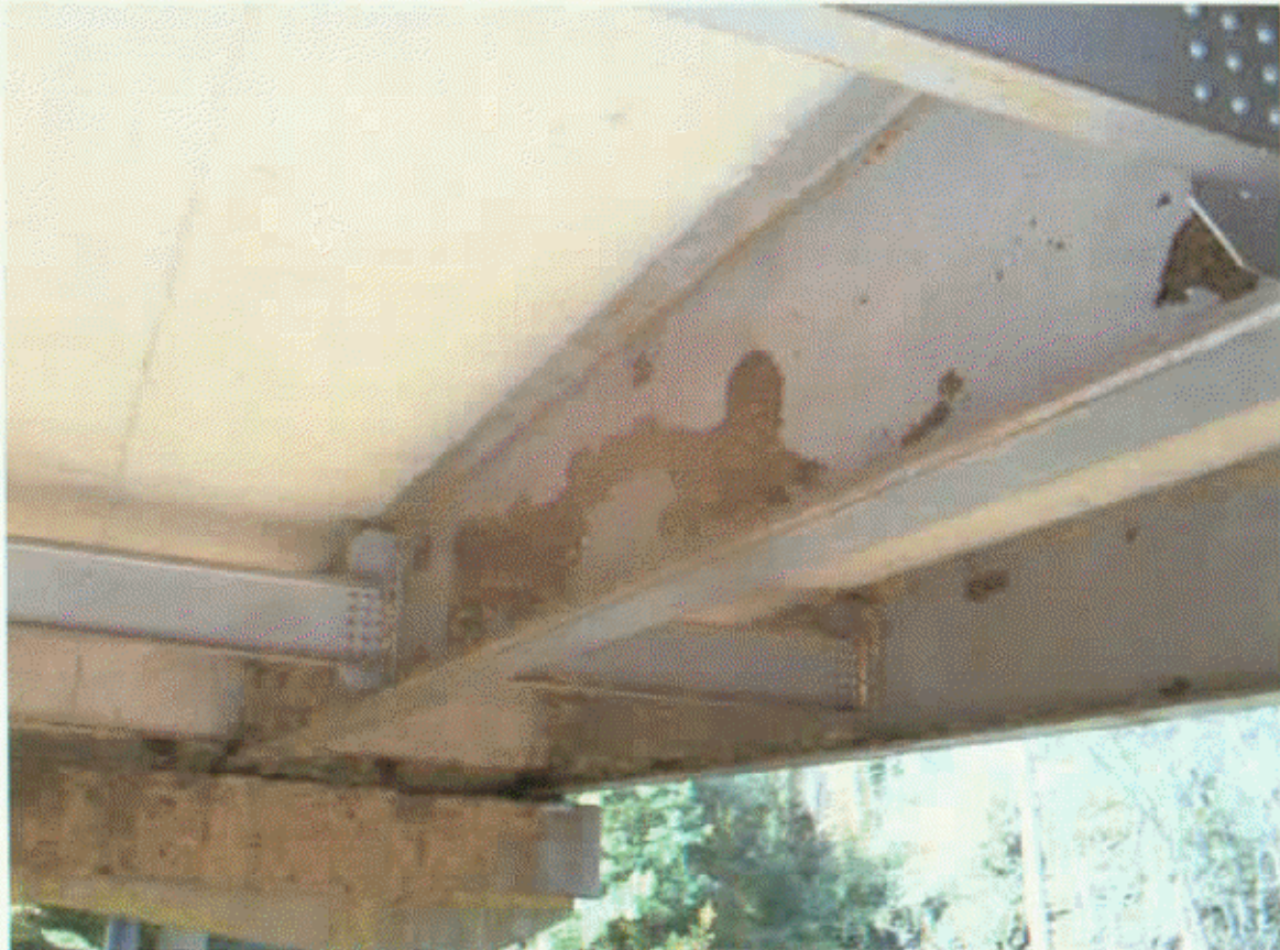
BEAM 2 IN SPAN 4 PAINT CONDITION SIMILAR
