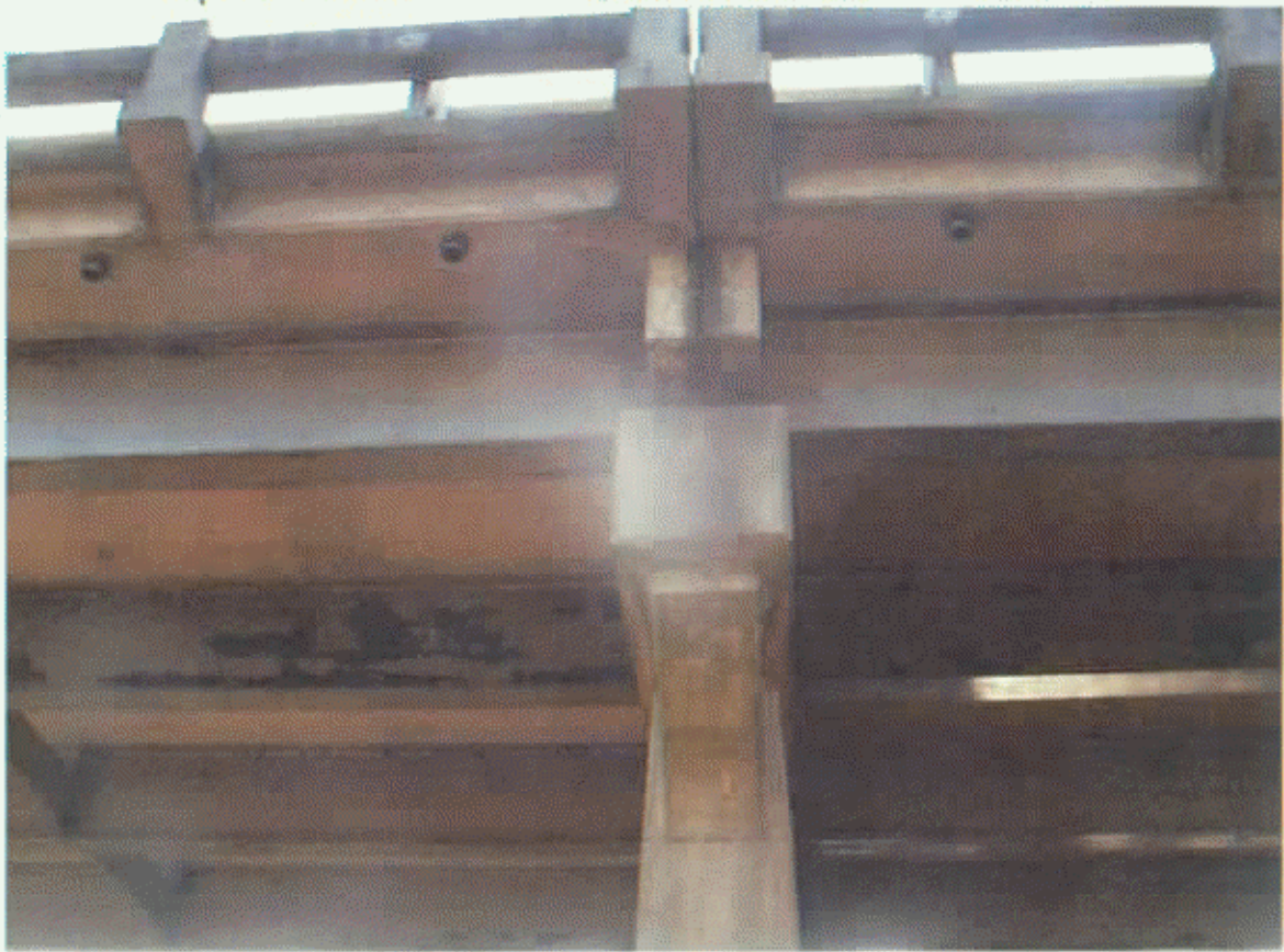
WEST END OF BENT 2
