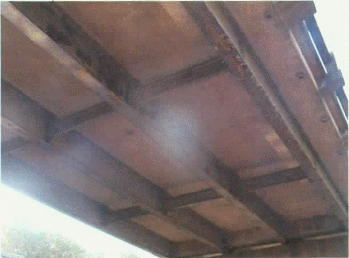
SPAN 2 UNDERSIDE (ALL SPANS SIMILAR)
