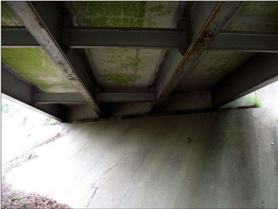
END BENT 2 OVERVIEW
