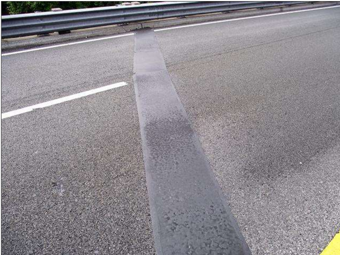
JOINT AT BENT 3
