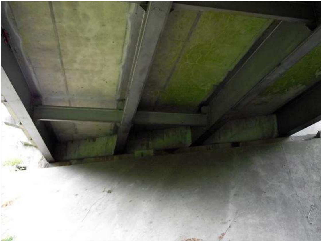
END BENT 1 OVERVIEW
