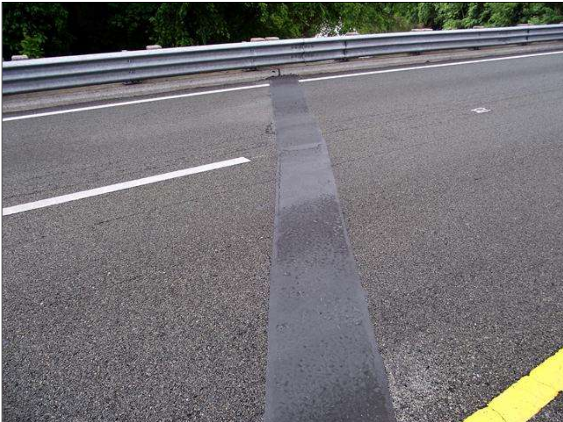
JOINT AT BENT 7
