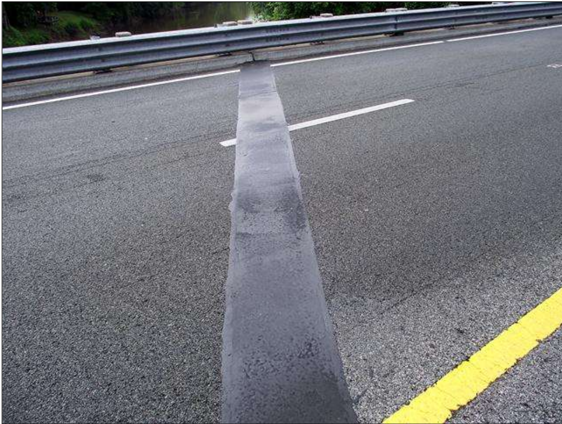
JOINT AT BENT 4
