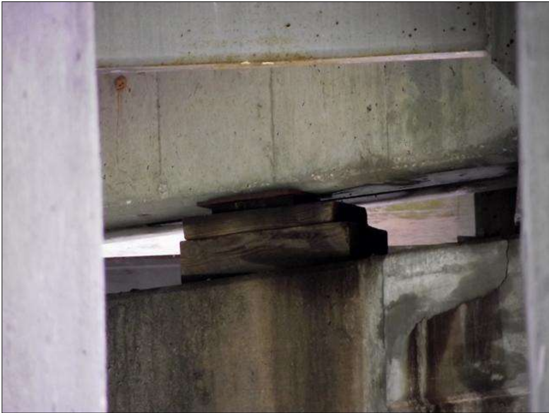
SHORING ADDED AT BENT 4 BAY 2
