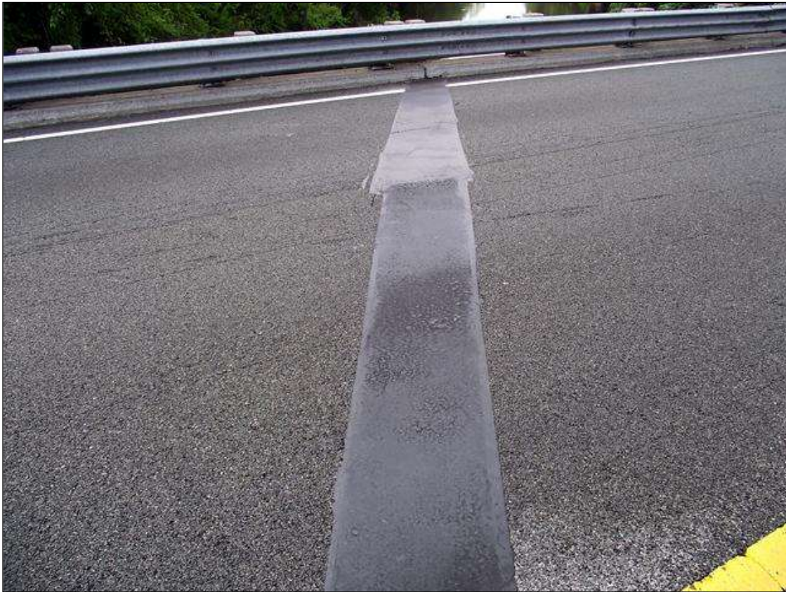
JOINT AT BENT 6
