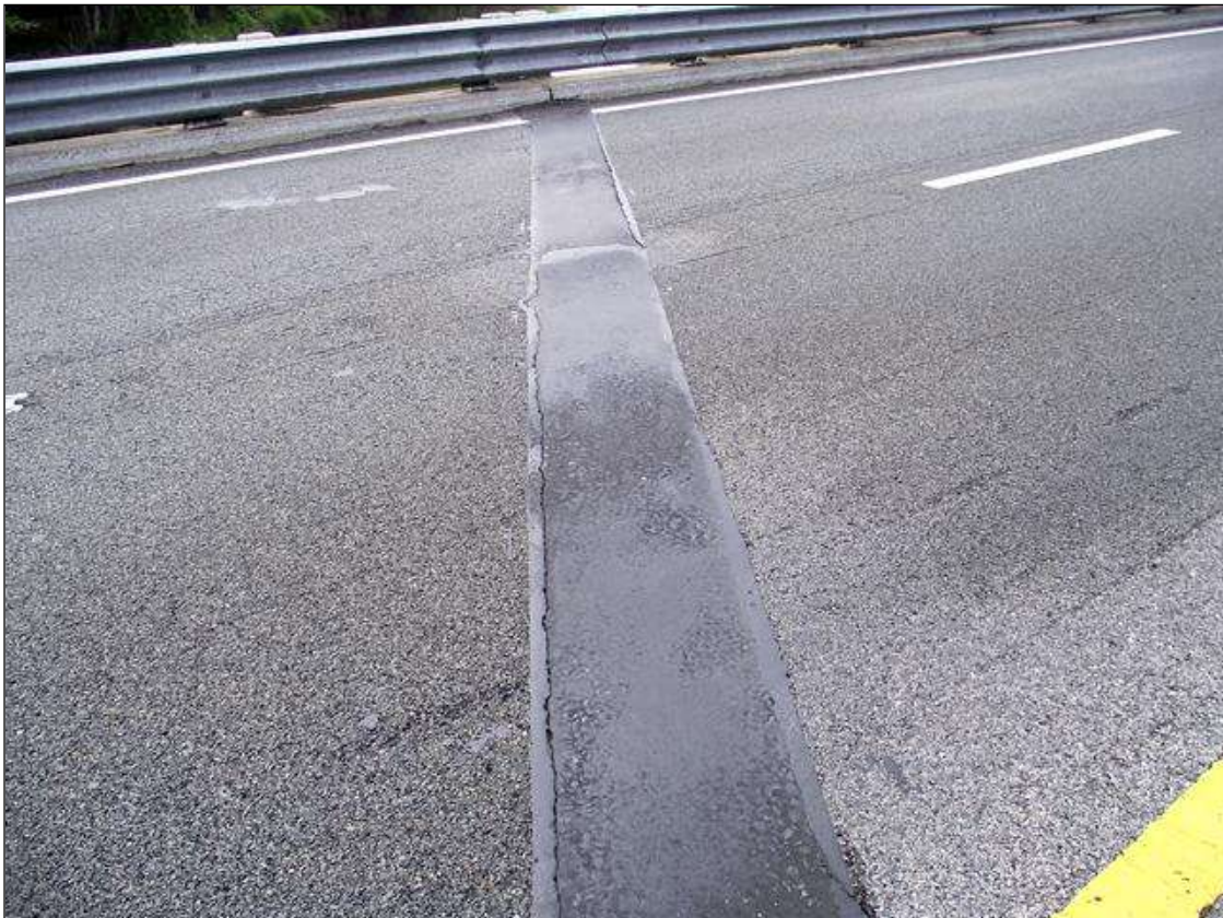
JOINT AT BENT 5
