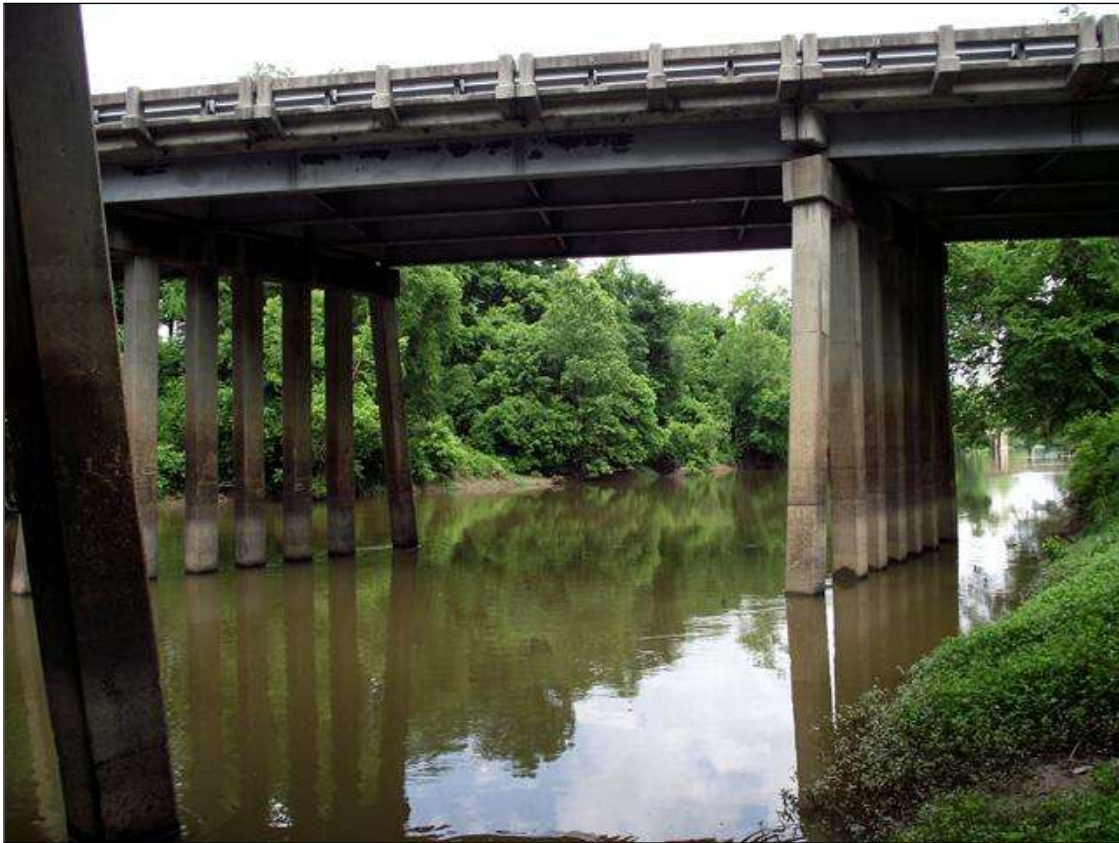
LOOKING WEST UPSTREAM UNDER THE SOUTHBOUND STRUCTURE
