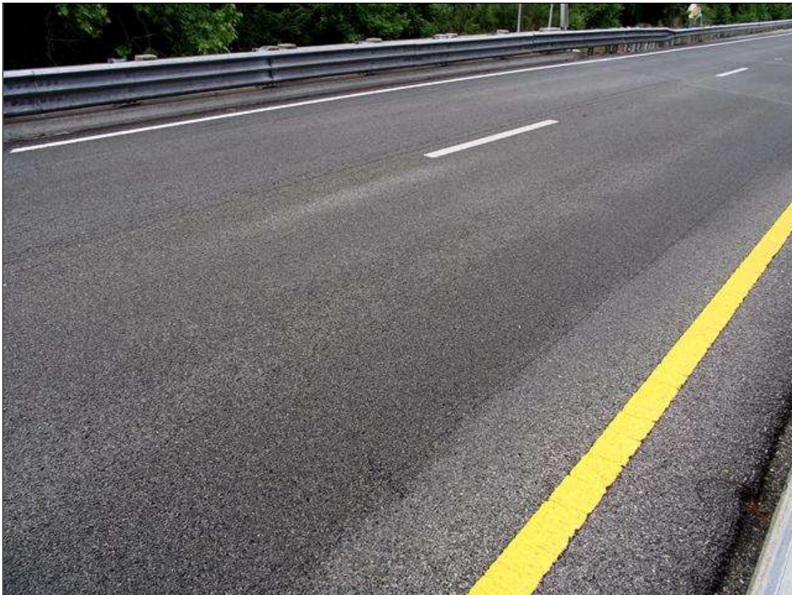
SPAN 1 OVERVIEW - ALL SPANS SIMILAR
