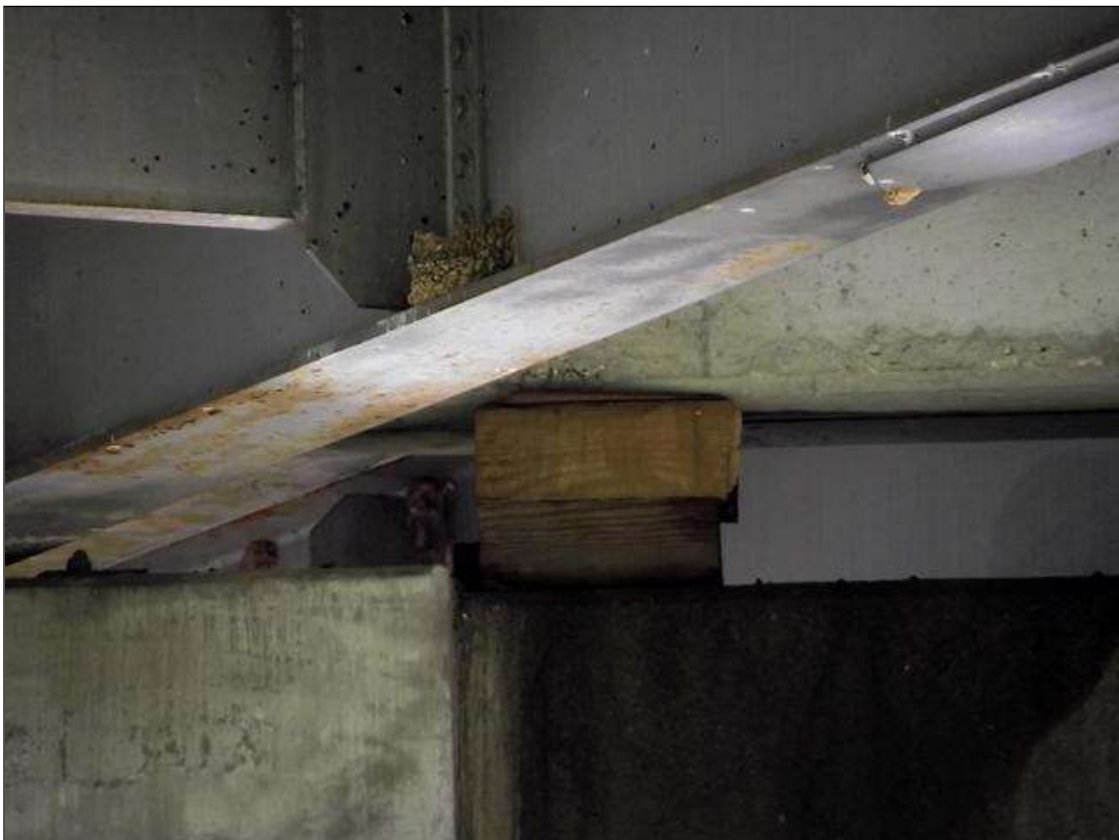
SHORING ADDED AT BENT 4 BAY 3
