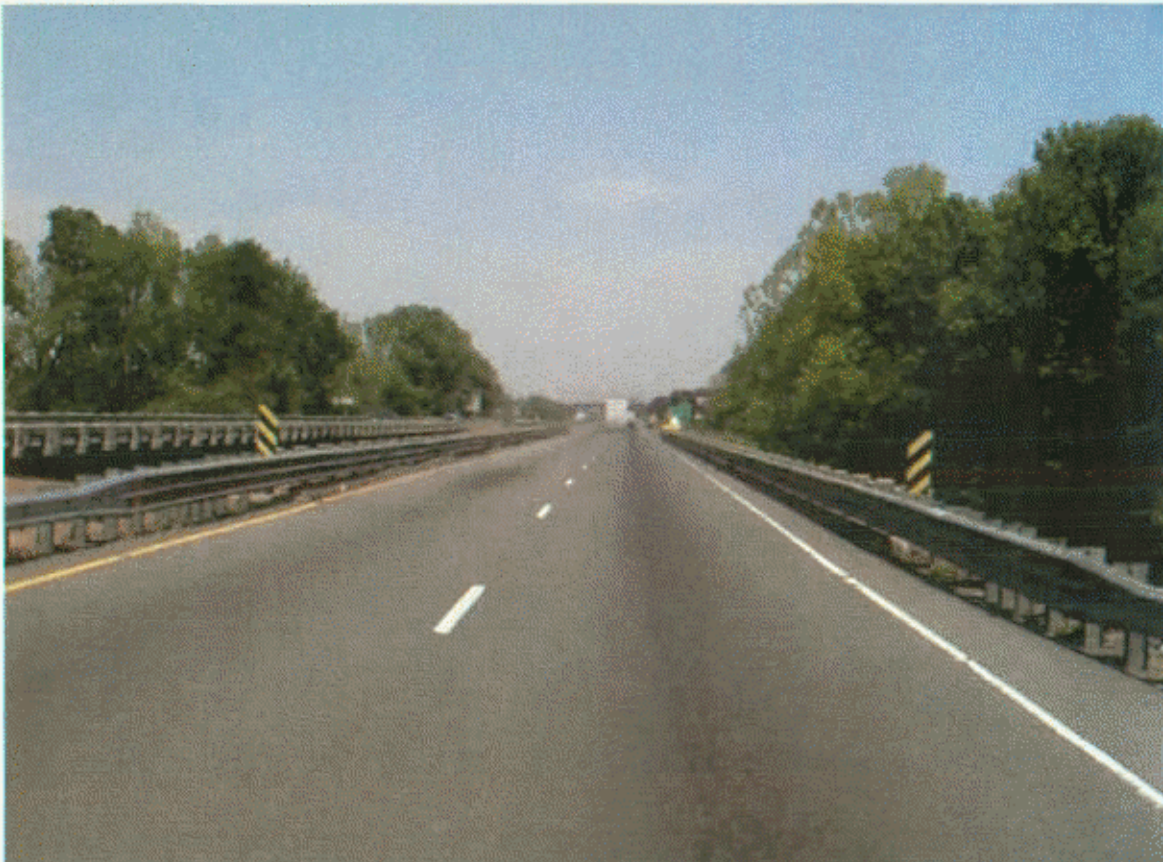
NORTH & RAIL TRANSITIONS @ SOUTH END OF BRIDGE
