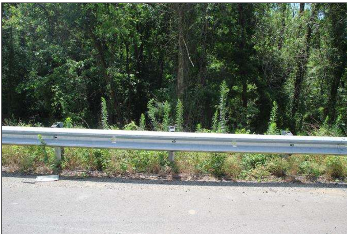
POST SPACING MID LENGTH NORTHEAST CORNER
