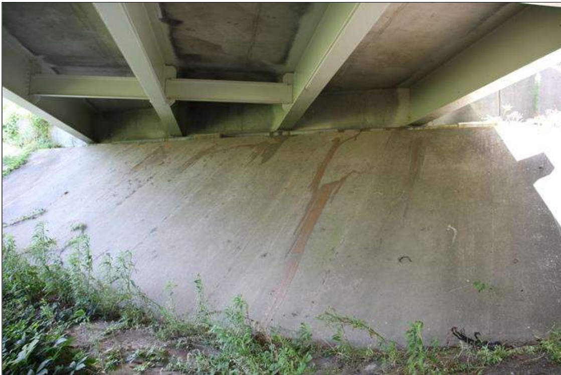
SLOPE PROTECTION AT END BENT 2
