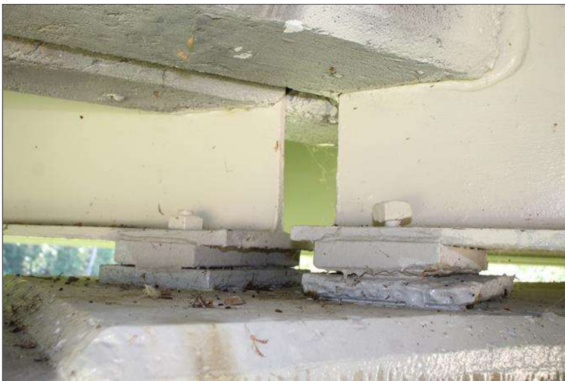
BEARINGS AT BENT 1 BEAM 2
