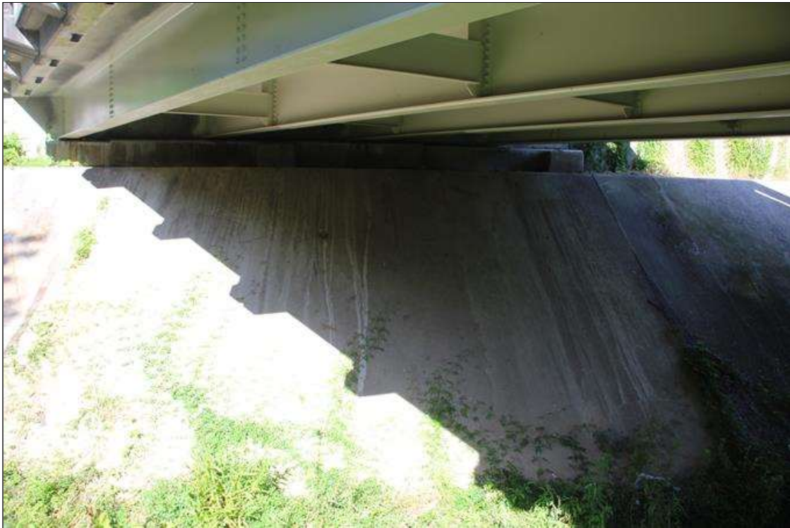
SLOPE PROTECTION AT END BENT 1
