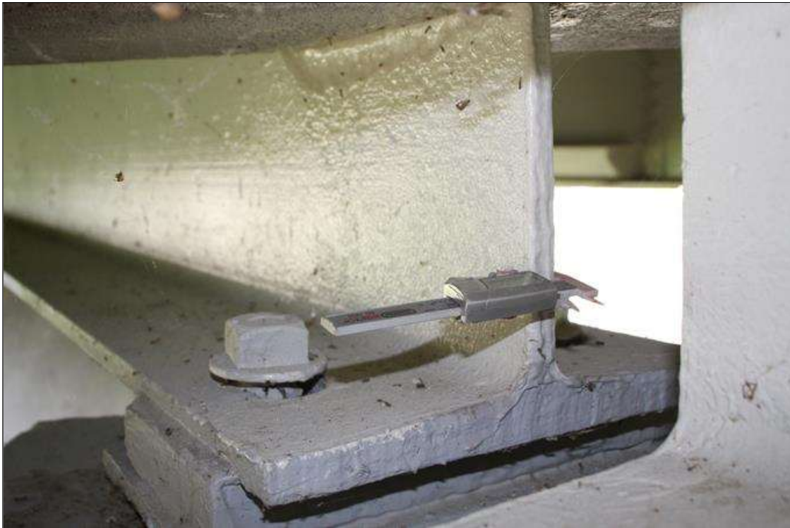
WEB THICKNESS SPAN 8 BEAM 2
