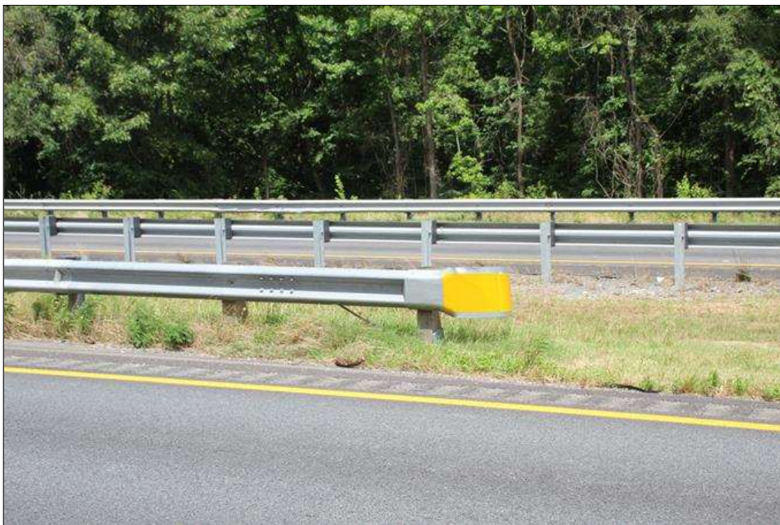
GUARDRAIL END TERMINAL NORTHWEST CORNER
