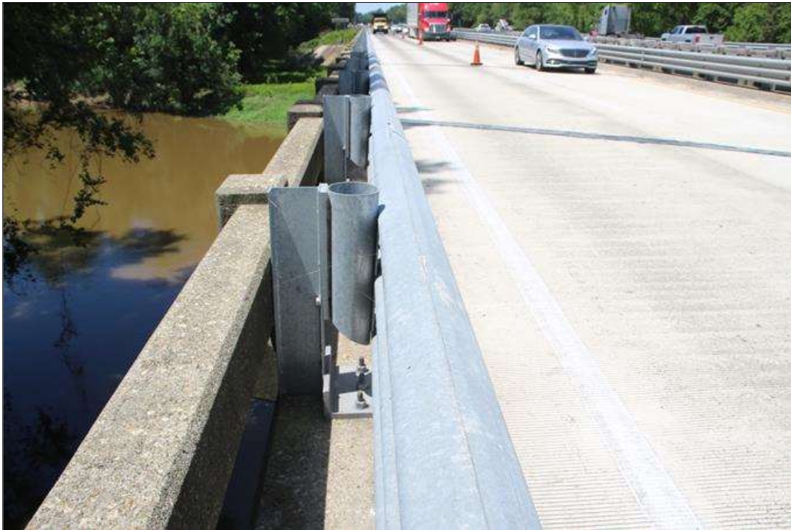
LEFT BRIDGE RAIL LOOKING SOUTH
