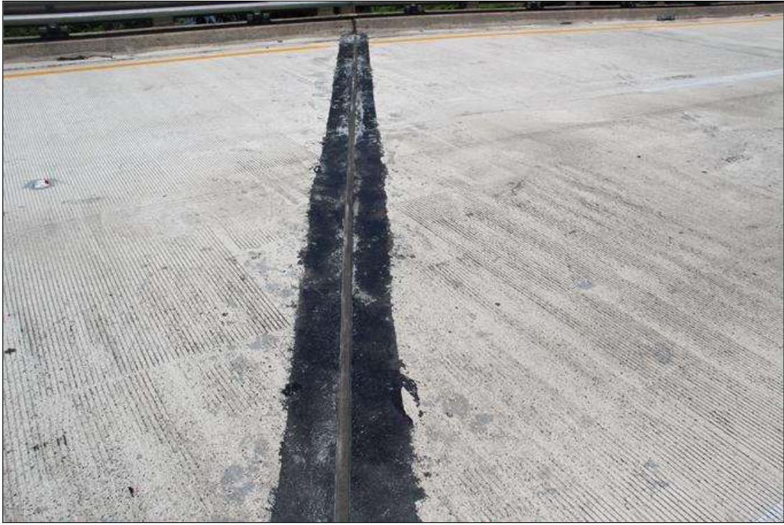
DECK JOINT ALONG BENT 7. OTHER BENTS SIMILAR.
