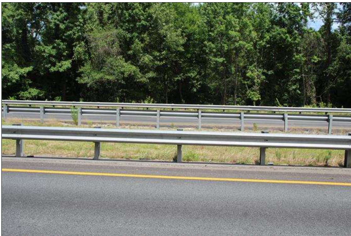
POST SPACING MID LENGTH NORTHWEST CORNER
