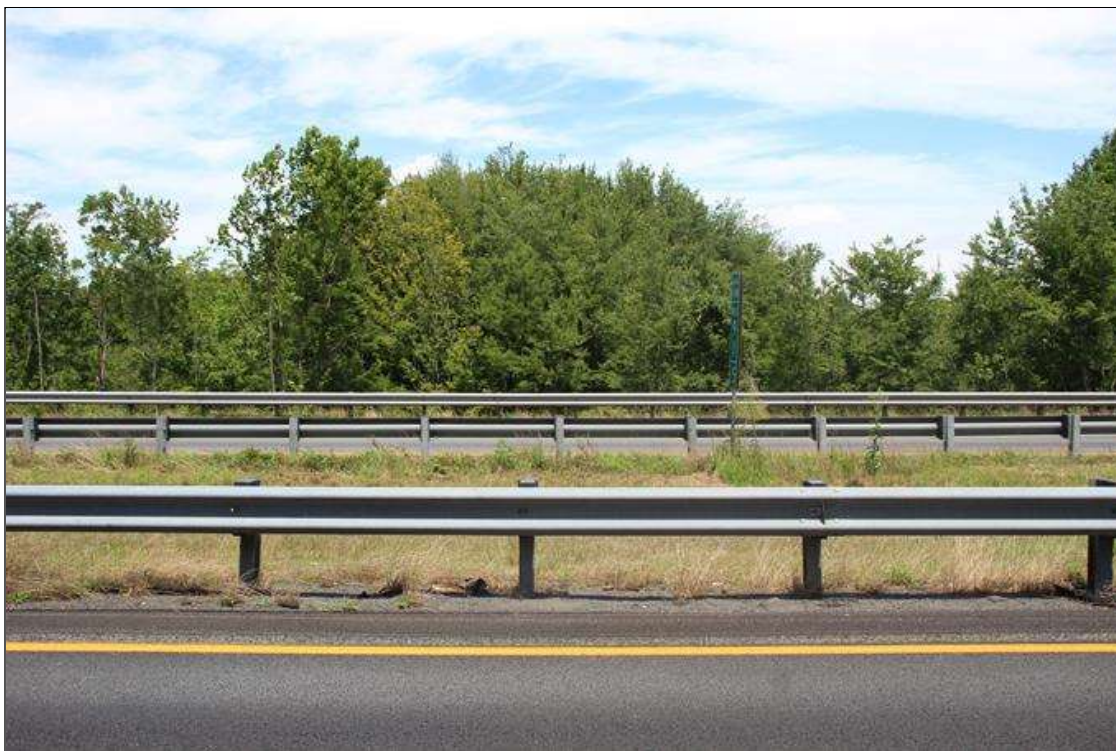
POST SPACING MID LENGTH SOUTHWEST CORNER
