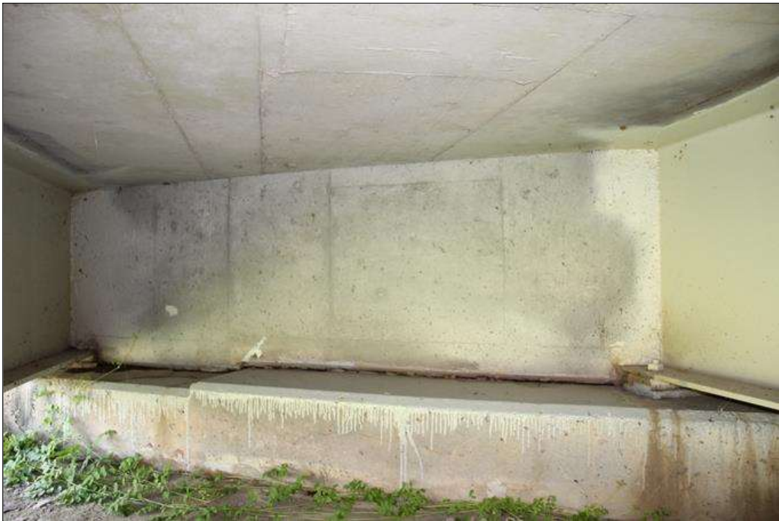
CAP AND BACKWALL AT END BENT 1 BAY 1
