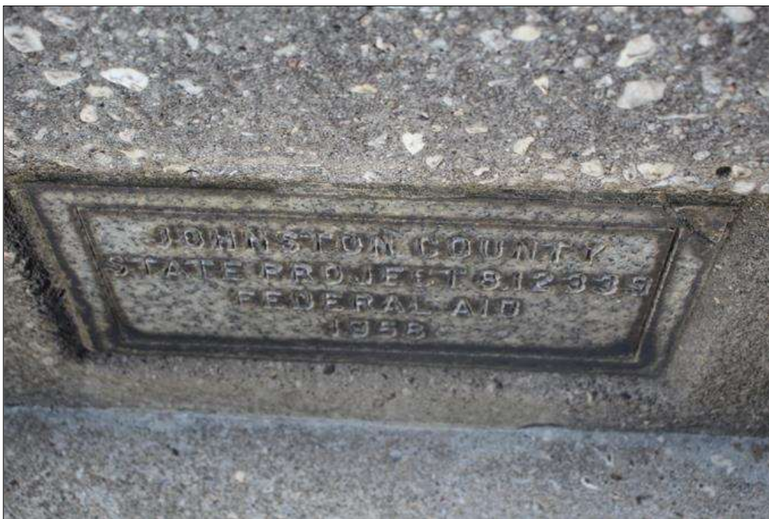
BRIDGE PLAQUE AT SOUTHEAST CORNER. TYPICAL AT NORTHWEST CORNER.
