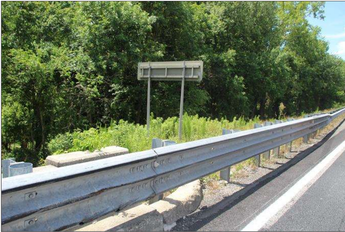
POST SPACING AT BRIDGE SOUTHEAST CORNER
