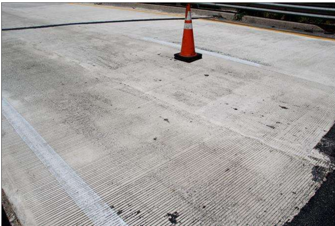
NORTH APPROACH SLAB. NEW SINCE PREVIOUS INSPECTION.
