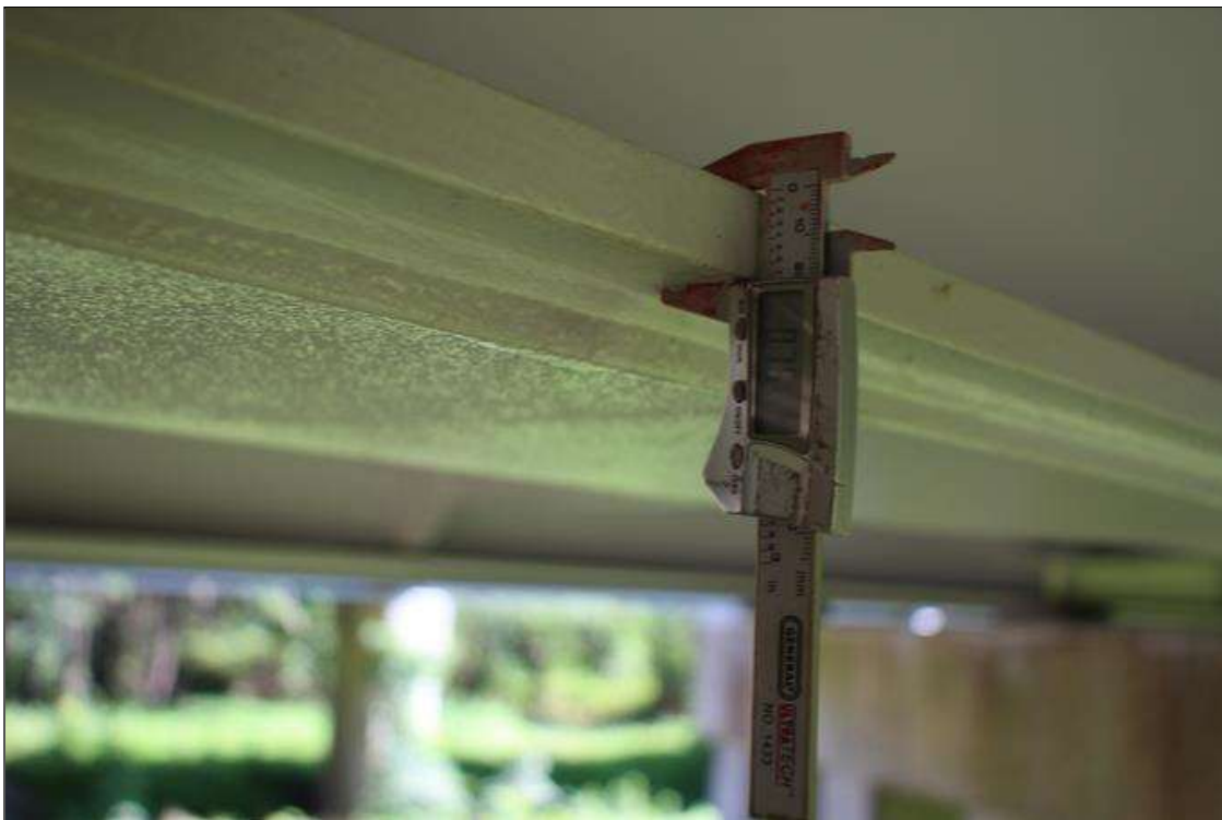
BOTTOM FLANGE THICKNESS SPAN 1 BEAM 3
