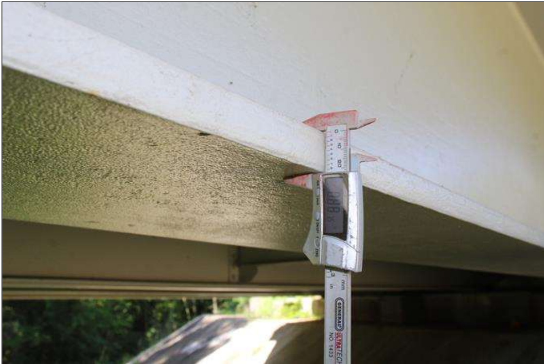
BOTTOM FLANGE THICKNESS IN SPAN 1, BEAM 1.
