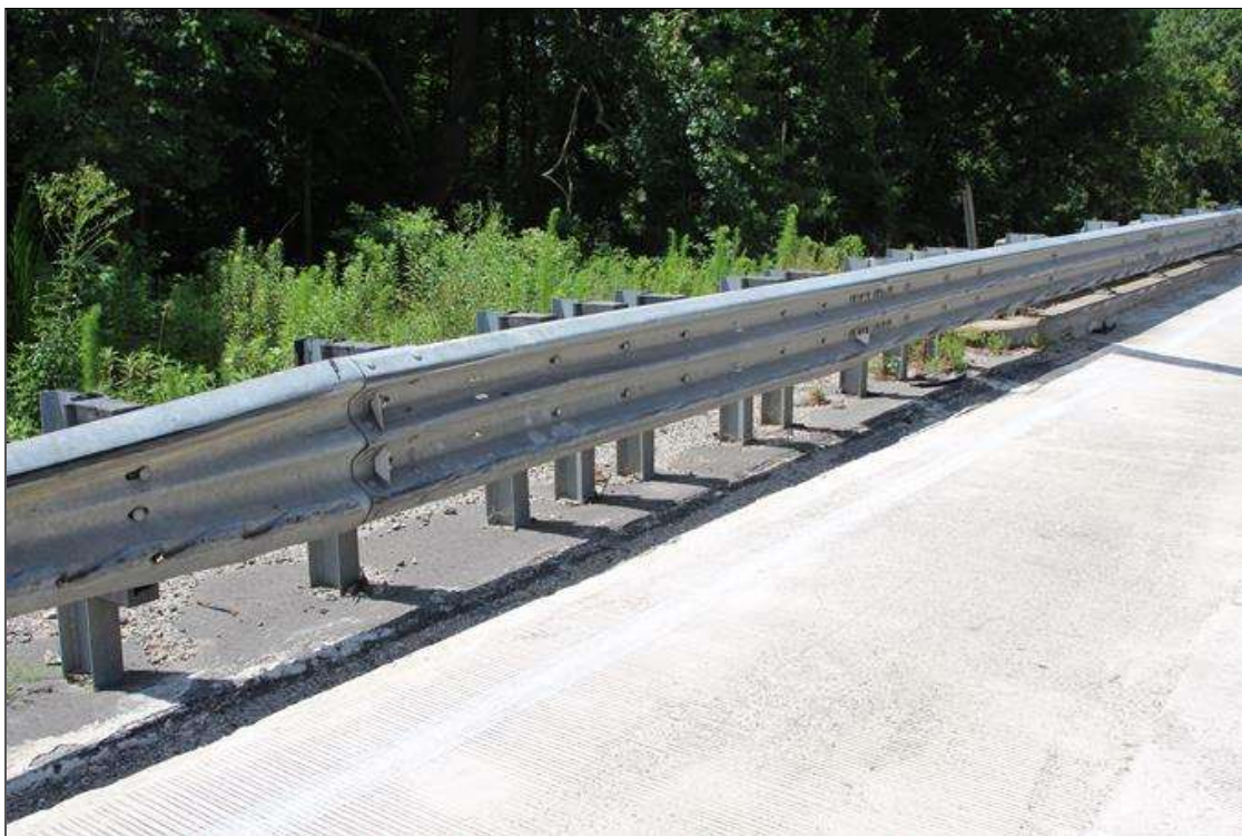
POST SPACING AT BRIDGE NORTHEAST CORNER
