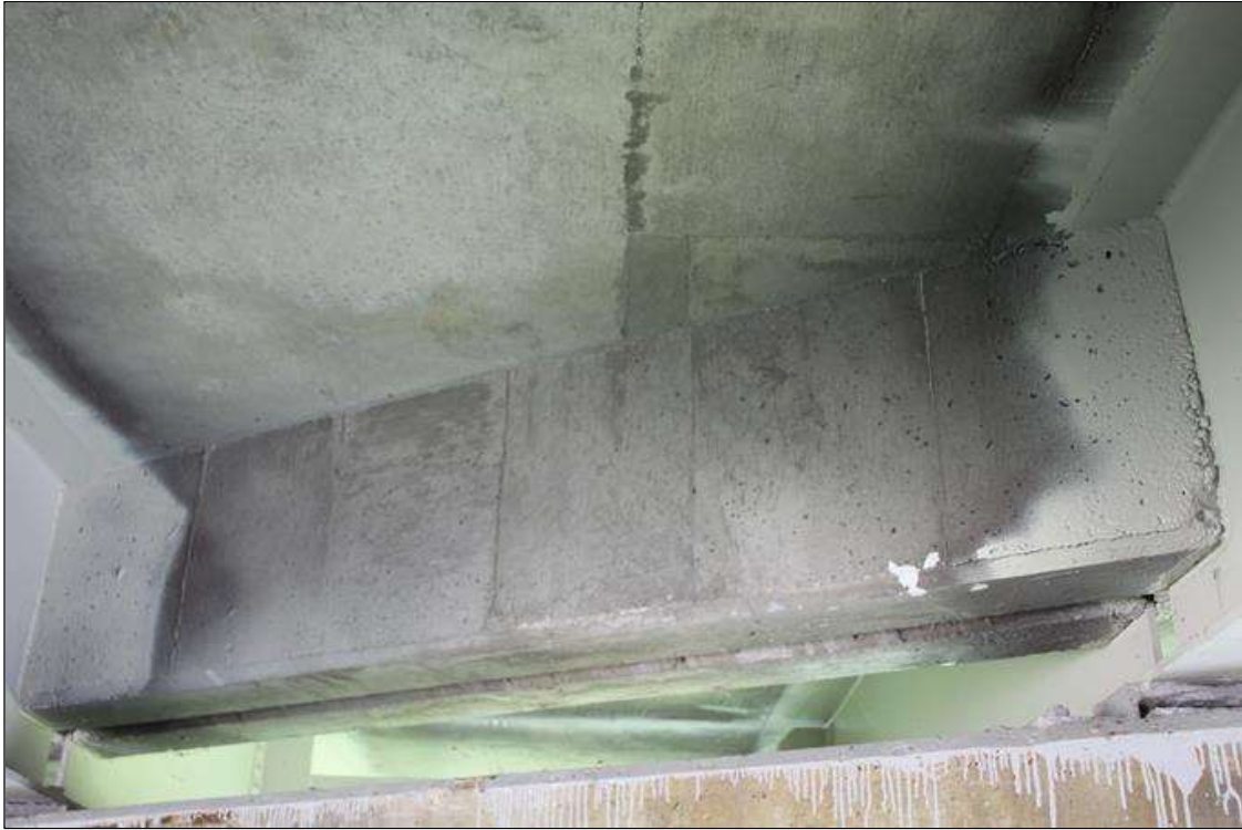
END DIAPHRAGM AT BENT 1 BAY 2
