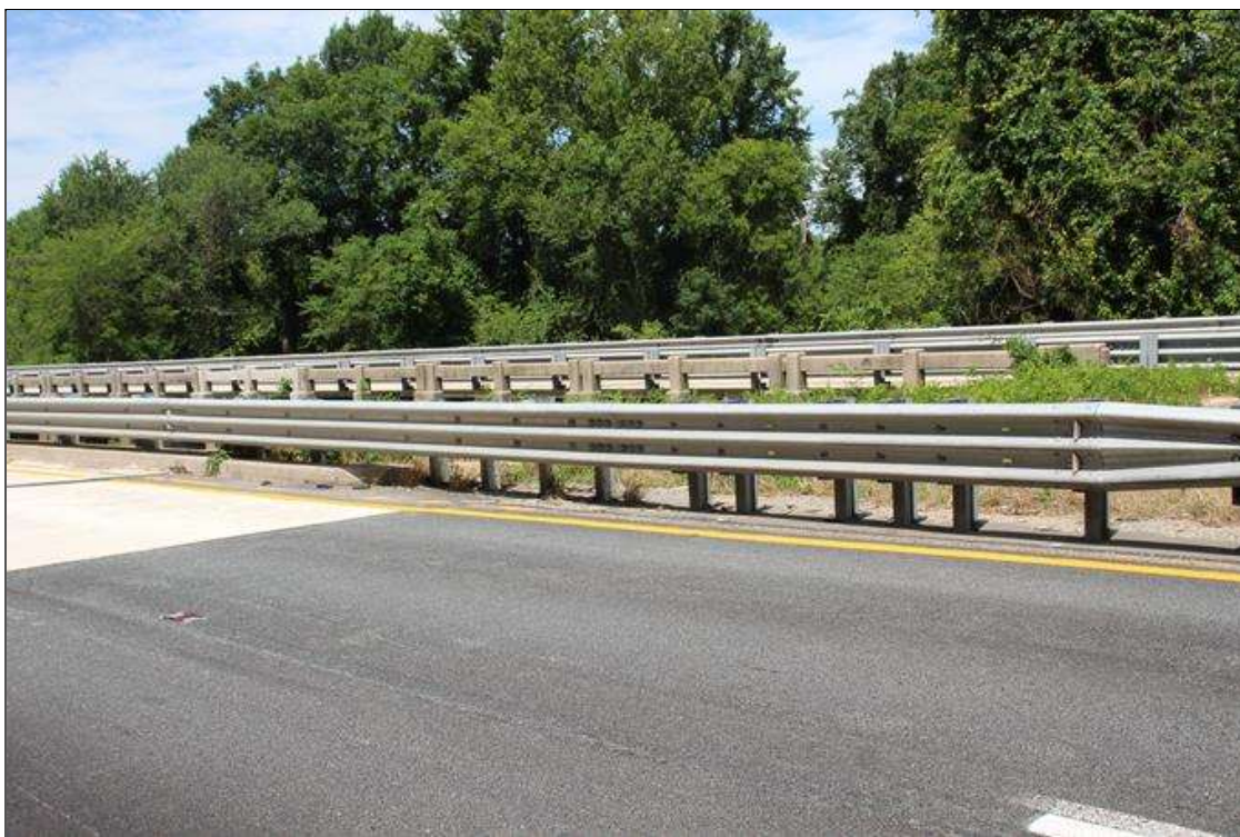
POST SPACING AT BRIDGE NORTHWEST CORNER
