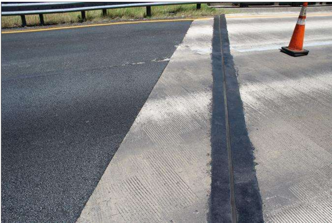
DECK JOINT OVER END BENT 1
