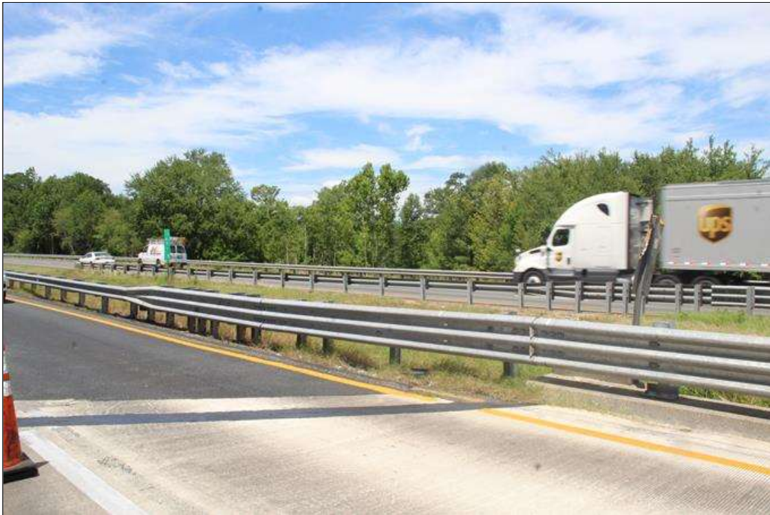
POST SPACING AT BRIDGE SOUTHWEST CORNER
