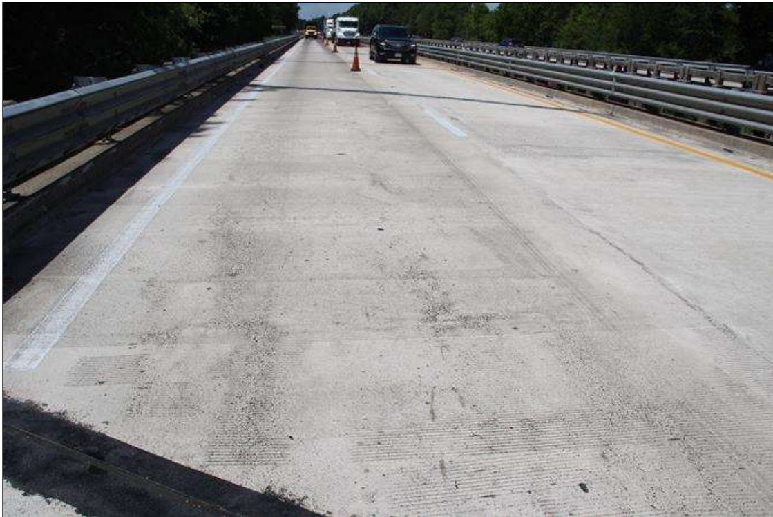
TOP OF DECK. NOTE NEW DECK SINCE PREVIOUS INSPECTION.
