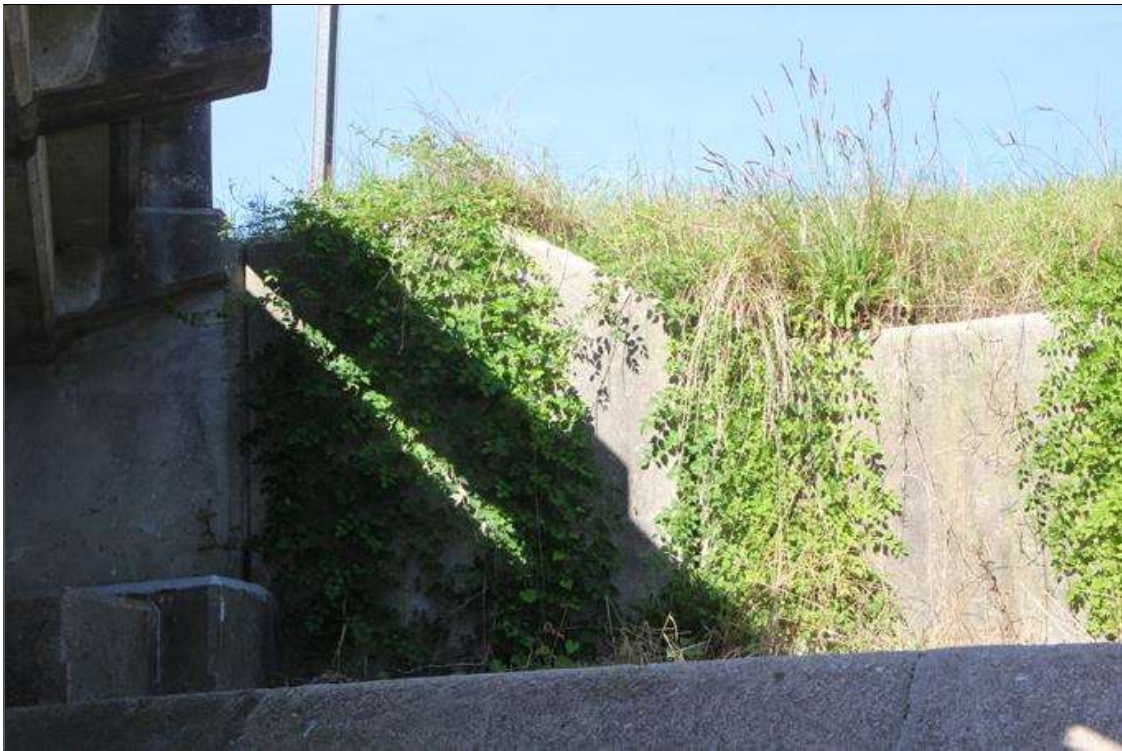
SOUTHWEST WINGWALL. NOTE HEAVY VEGETATION.
