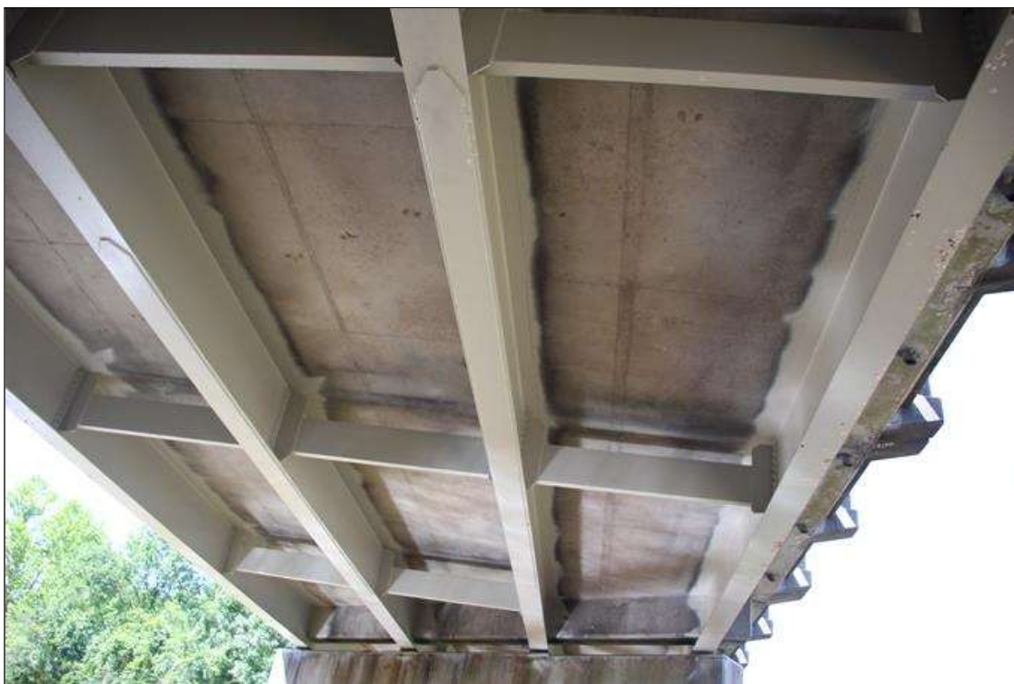
SUPERSTRUCTURE UNDERSIDE SPAN 5. NOTE NEW PAINT REPAIRS SINCE PREVIOUS INSPECTION.
