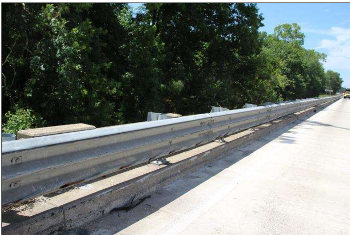
LEFT BRIDGE RAIL
