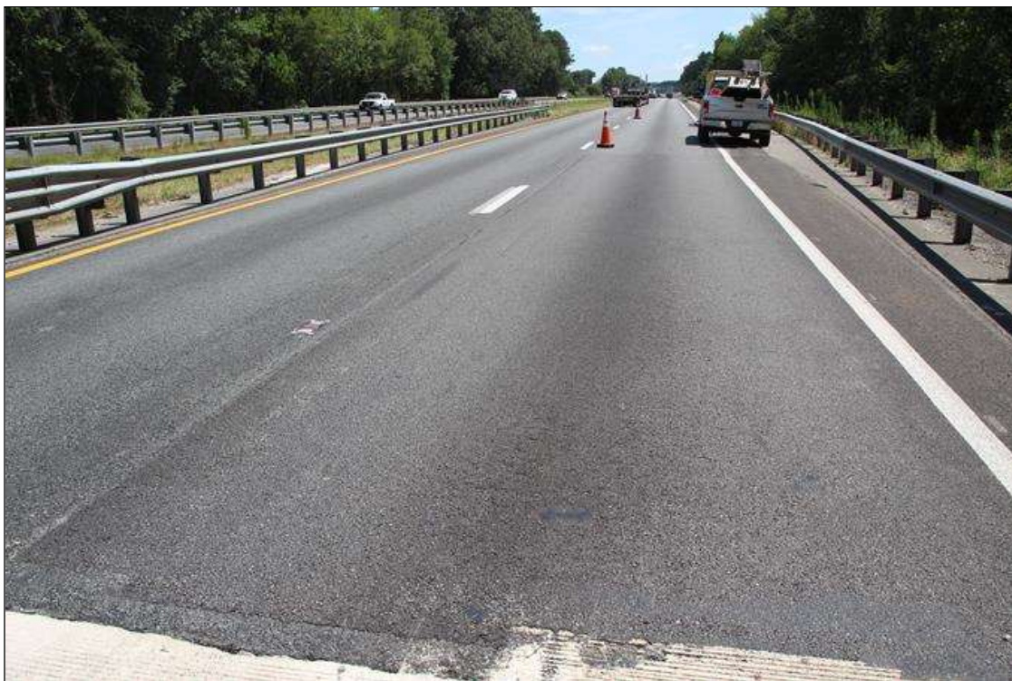
NORTH APPROACH. NOTE NEW APPROACH PAVEMENT.
