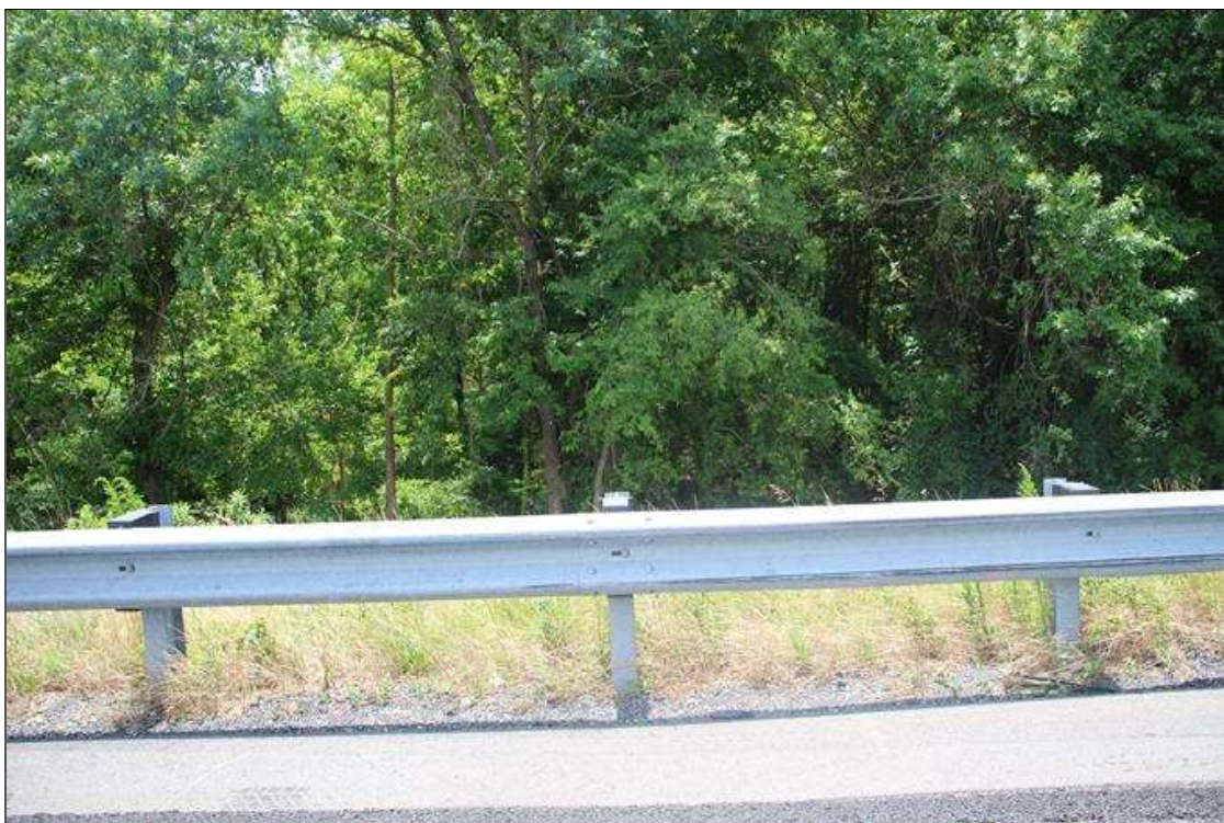
POST SPACING MID LENGTH SOUTHEAST CORNER
