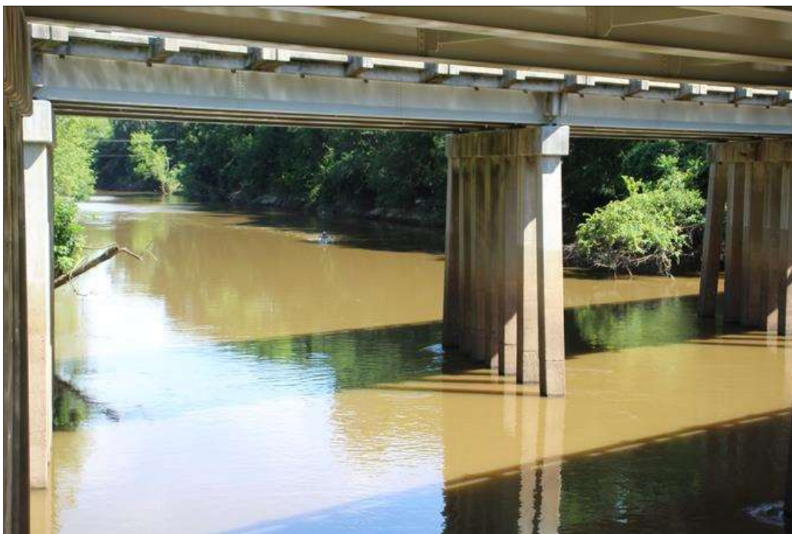
UPSTREAM FROM UNDER THE BRIDGE
